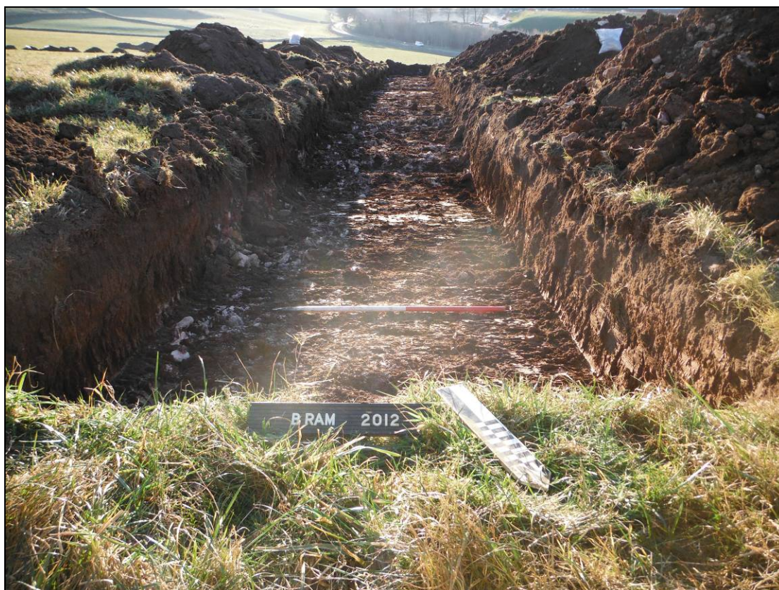
Figure 20. Trench 5, looking south-west. Scale 1x1m
