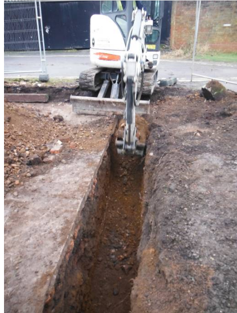
General view of excavation area, looking south
