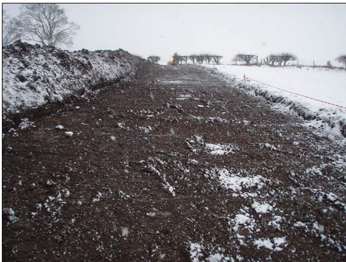
Figure 3: The stripped easement in Field 1, looking south.
