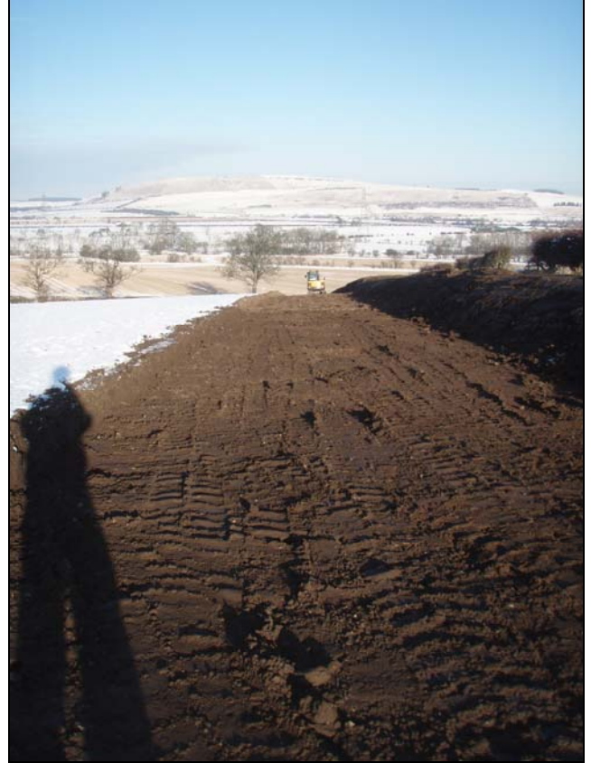
The stripped easement, looking northeast
