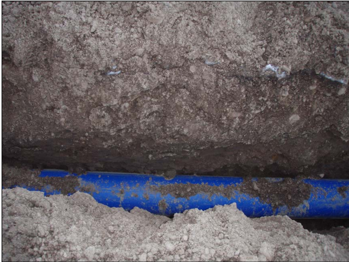
Figure 4: Looking into the pipeline trench once the pipe had been laid.
