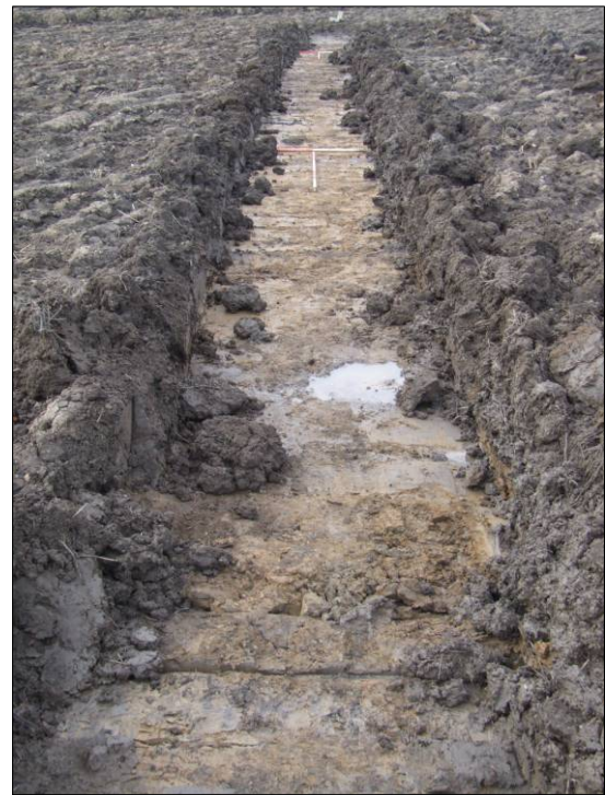
Figure 13: Trench 8, looking northeast
