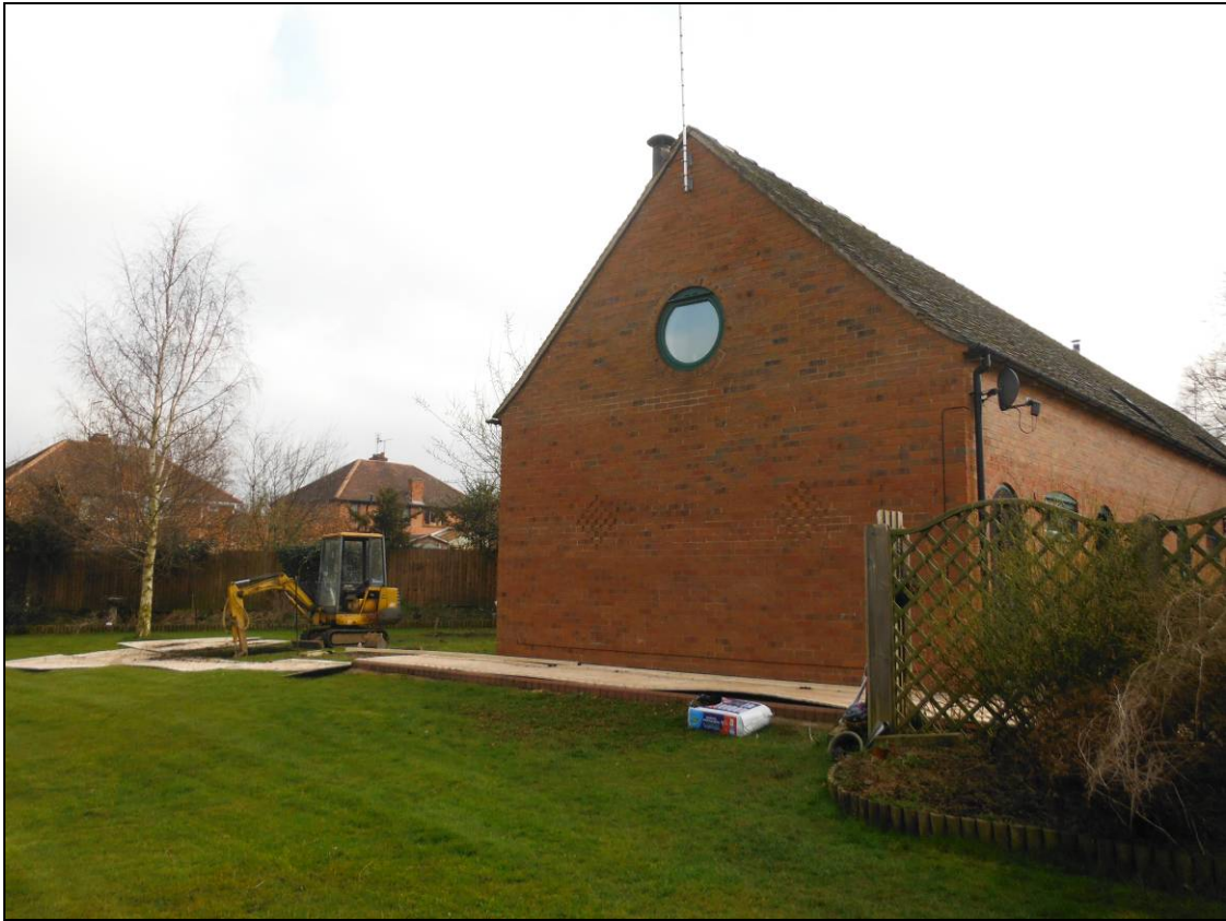
Figure 5: General view of the excavated area, looking north
