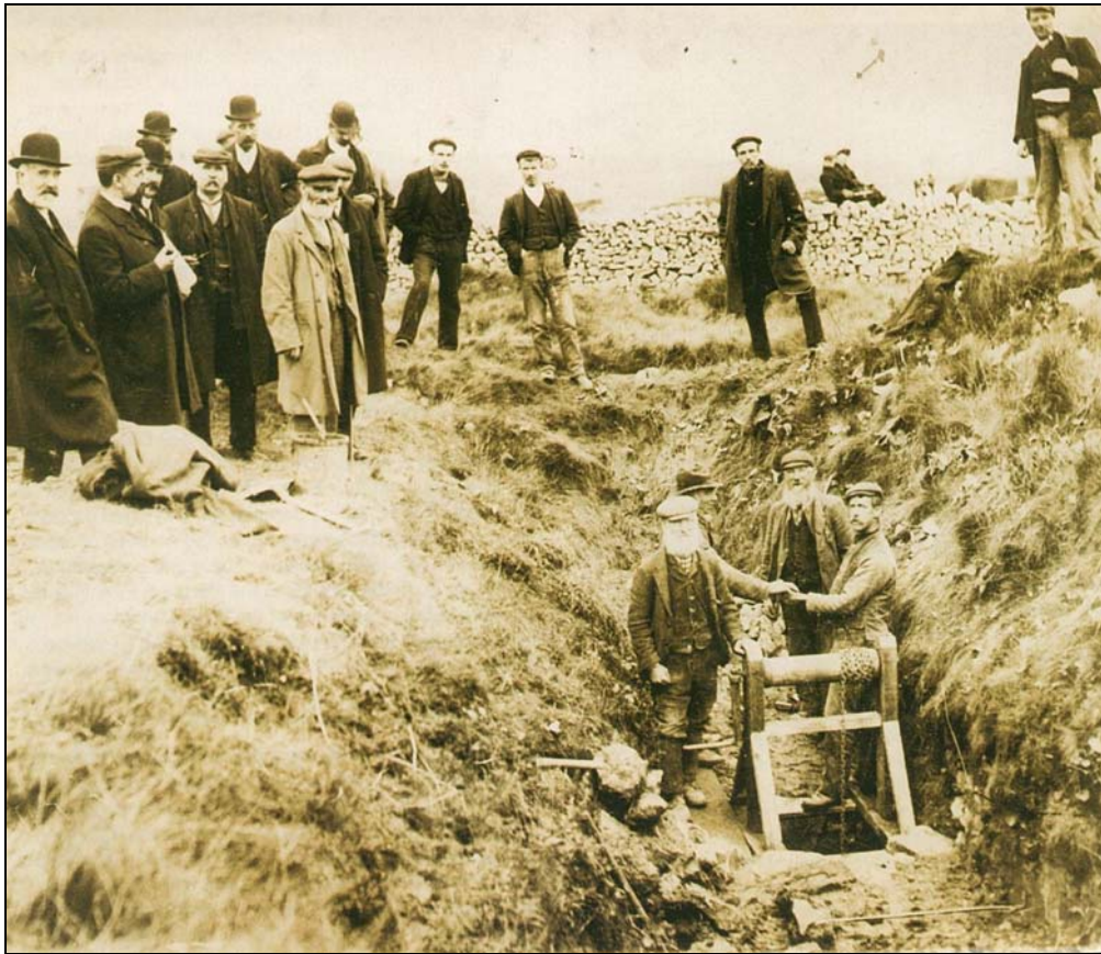
Figure 14. Mine workings at Moss Rake, Bradwell in 1906. The small shaft entrance with the hand windlass in the foreground is comparable in shape and dimension to feature [103] observed in trench 1. (After Barnatt and Penny 2004, chapter 2.10)
