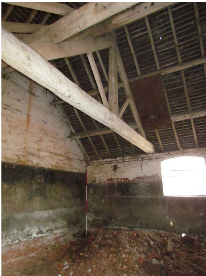
Figure 66: View Across Bay 3, Looking North-east (Scale = 2m).
