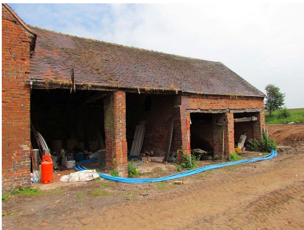
Figure 44: Bays 3 to 5 of Barn 2, Looking North (Scale = 2m).
