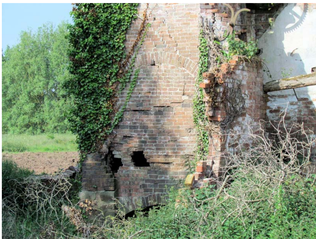
Figure 22: Detail of Double Archway Over Wheelpit.
