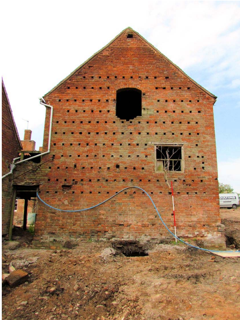
Figure 37: Barn 1, North-East Elevation, Looking South-west (Scale = 2m).
