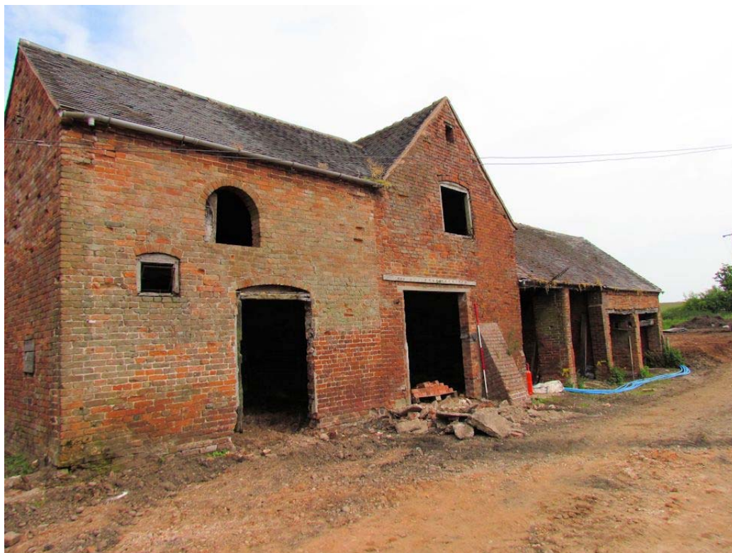
Figure 43: South-east Elevation of Barn 2, Looking North (Scale = 2m).
