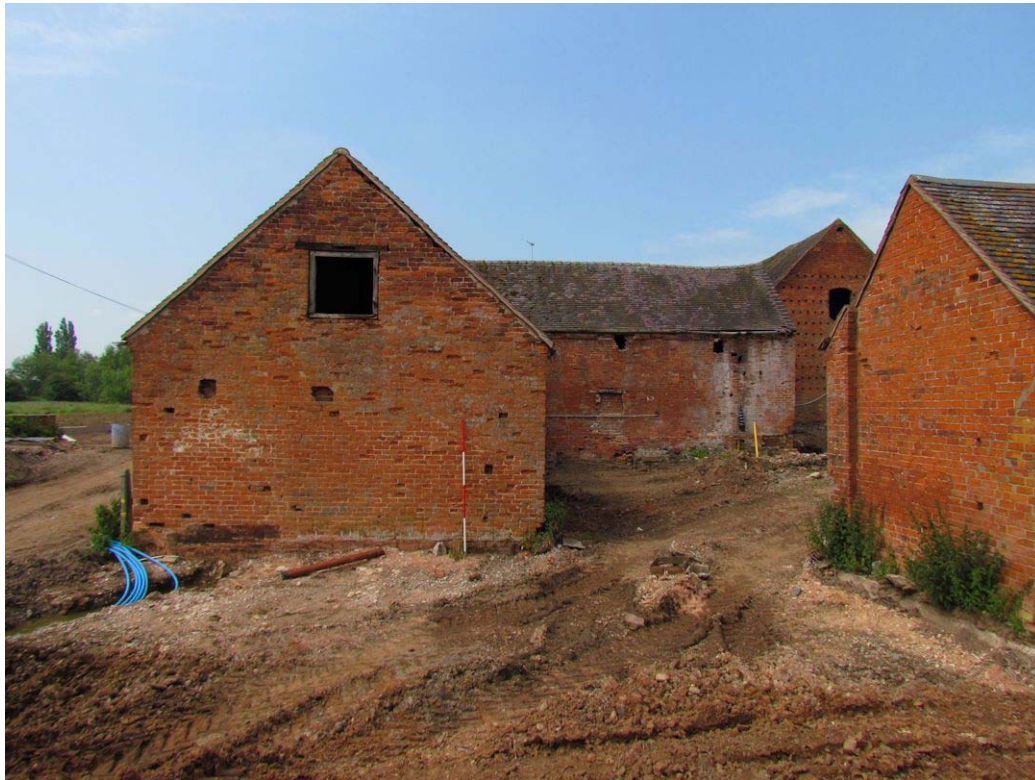
Figure 45: North-east Elevation of Barn 2, Looking South-west (Scale = 2m).
