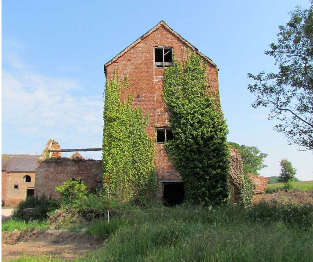
Figure 19: South Elevation, Looking North (Scale=2m).
