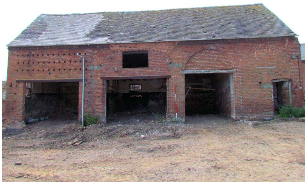
Figure 35: North-west Elevation, Looking South-east (Scale = 2m).
