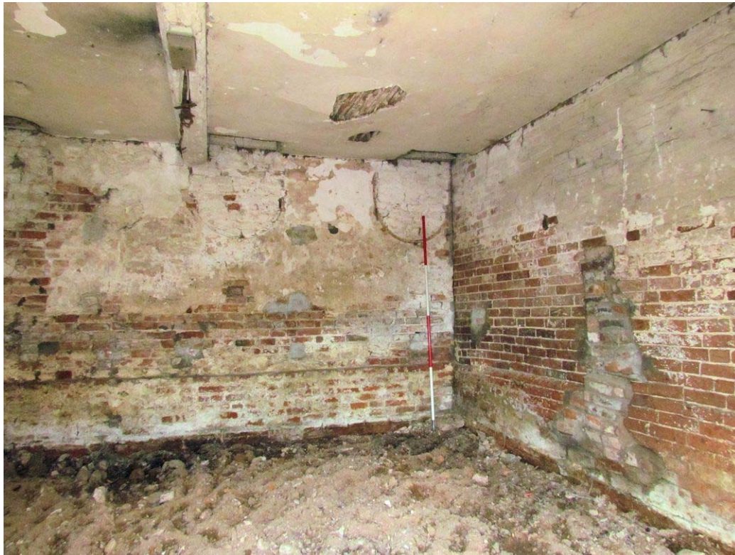
Figure 52: Bay 1, Looking North (Scale = 2m).
