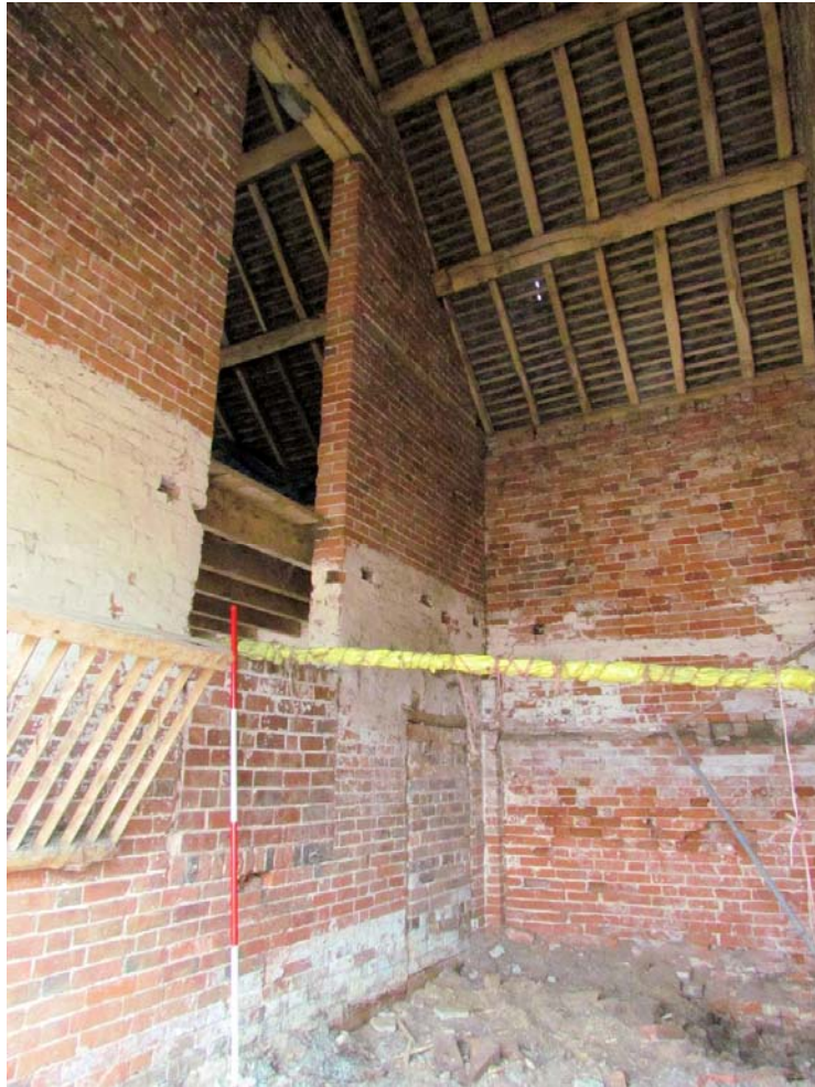
Figure 39: Interior of Bay 2, Looking East (Scale = 2m).
