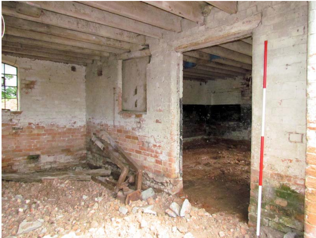
Figure 65: View Across Bays 1 and 2, Looking East (Scale = 2m).
