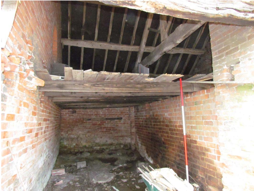
Figure 55: Bay 4, Looking North (Scale = 2m).
