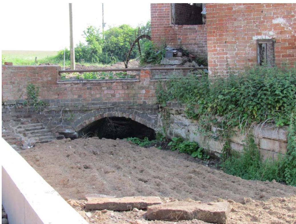
Figure 18: Detail of Bridge Over Northern Mill Race.
