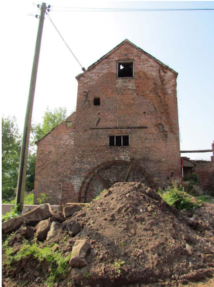
Figure 15: North Elevation of Mill, Looking South-east (scale = 2m).
