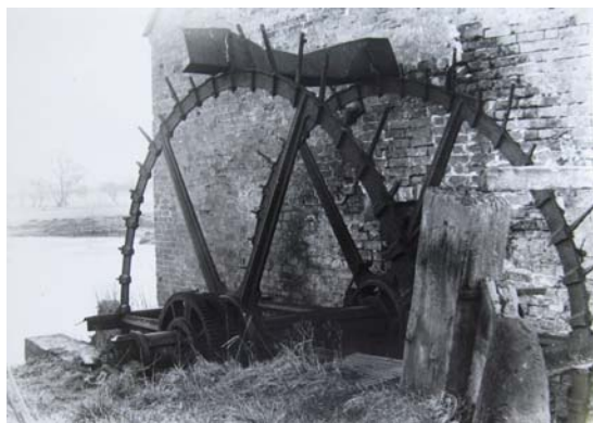
Figure 8: Waterwheel from West.
