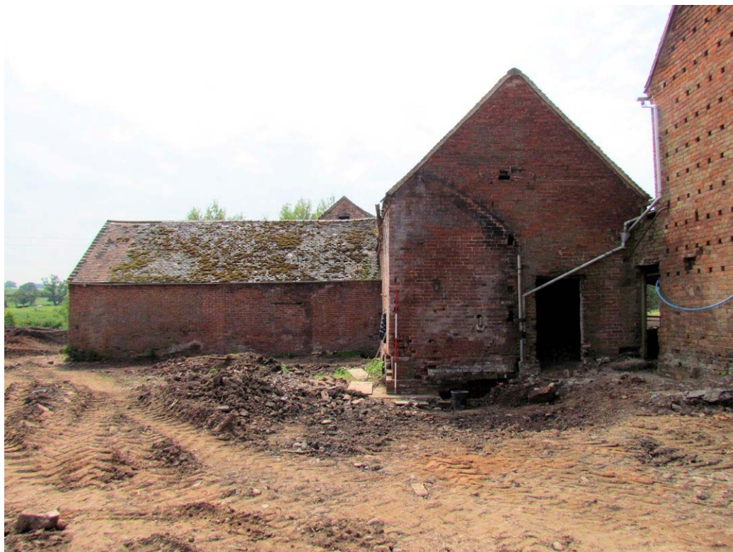
Figure 47: North-west Elevation of Barn 2, Looking South-east (Scale = 2m).
