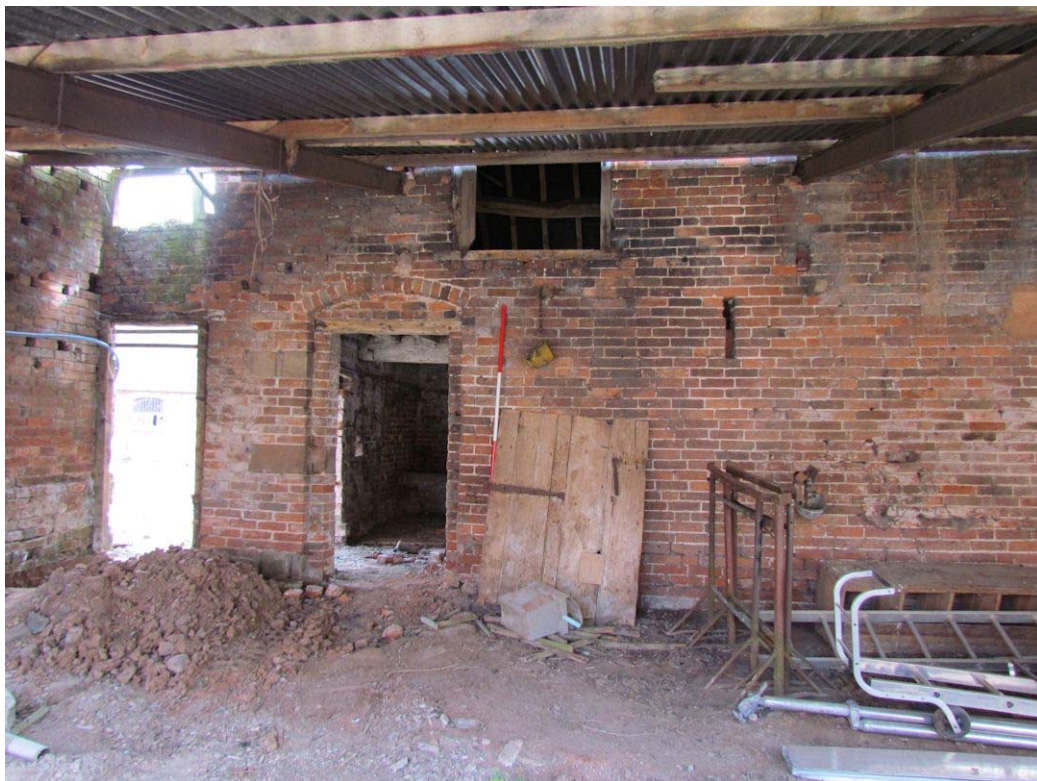
Figure 51: South-west Elevation of North Bay, Looking North (Scale = 2m).
