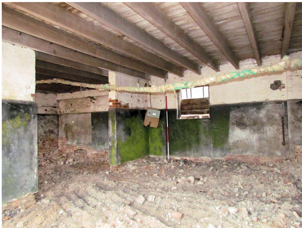
Figure 40: Interior of Bay 3, Looking East (Scale = 2m).
