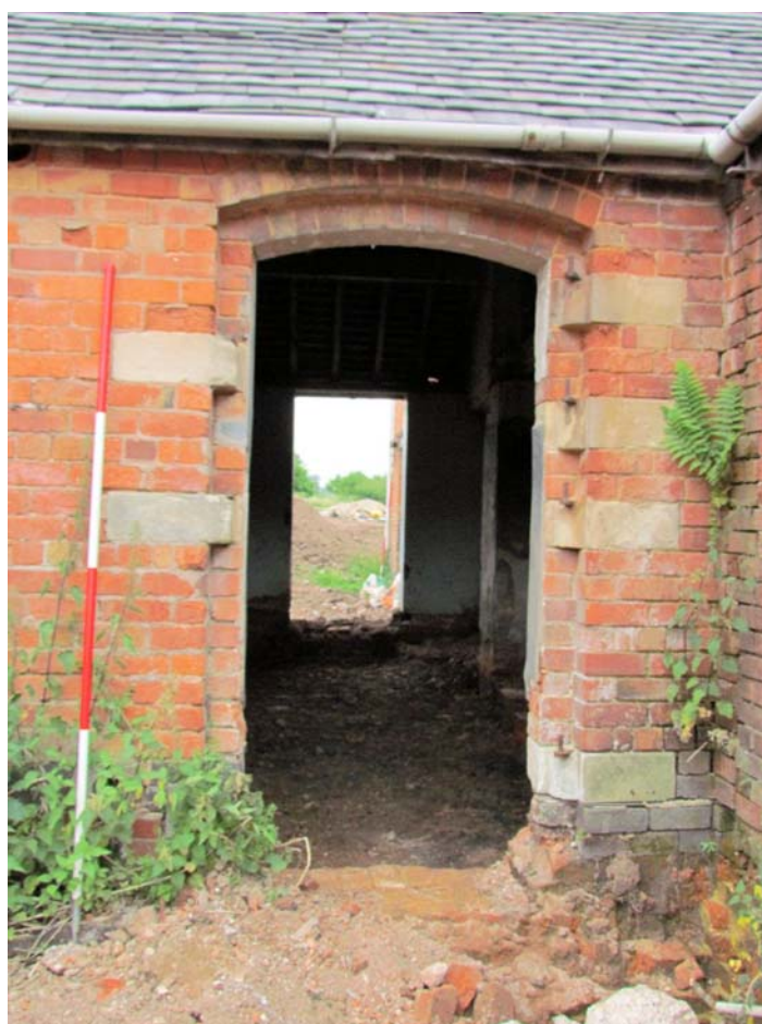
Figure 61: Detail of Door In Western Bay (Scale = 2m).
