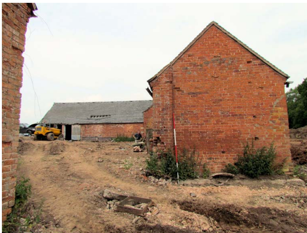
Figure 60: South-east Elevation of Barn 3, Looking North-west (Scale = 2m).
