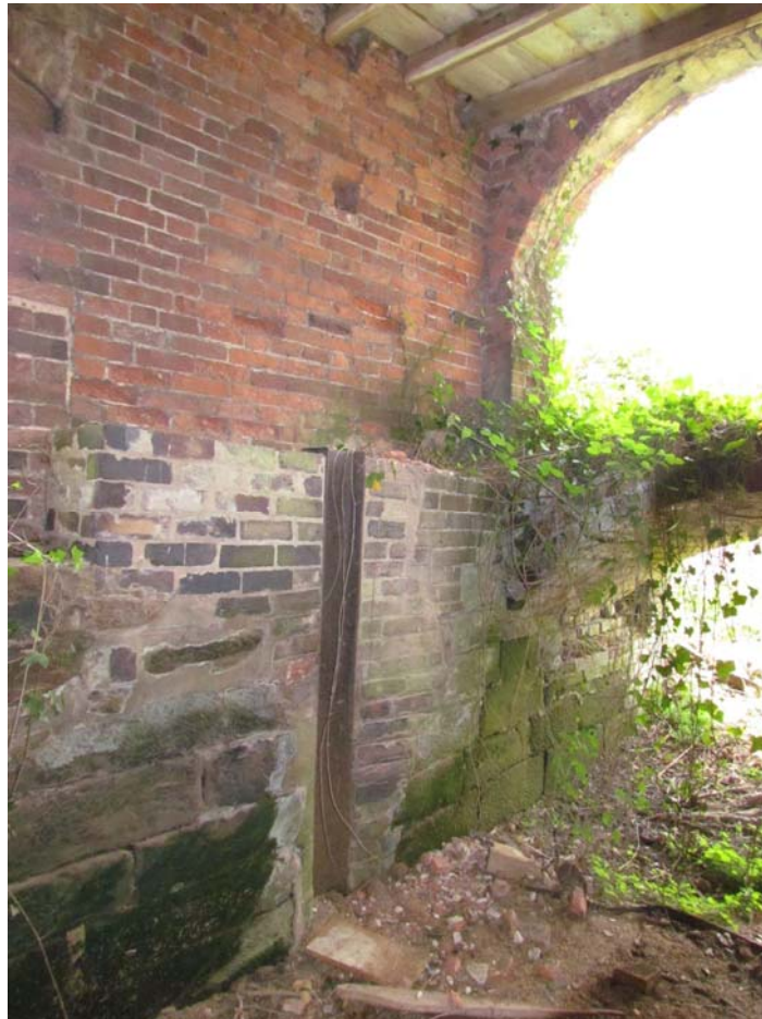
Figure 26: Detail of Southern Wheelpit, Looking South.
