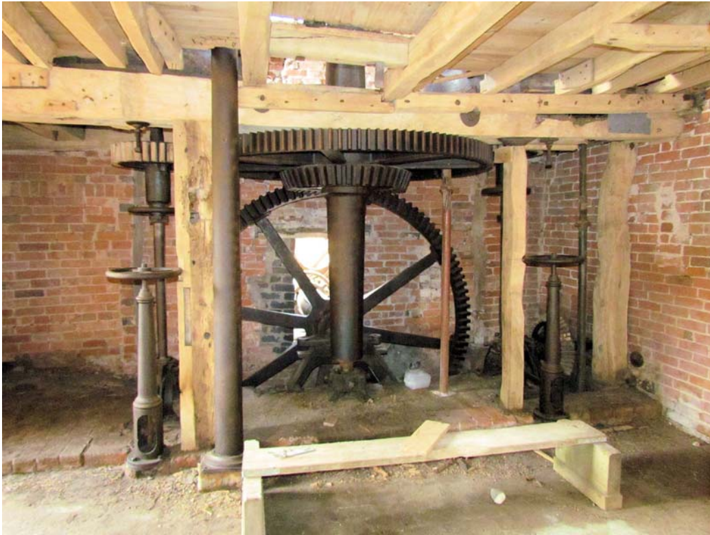
Figure 27: Detail of North Wheel Gearing, Looking North-west.
