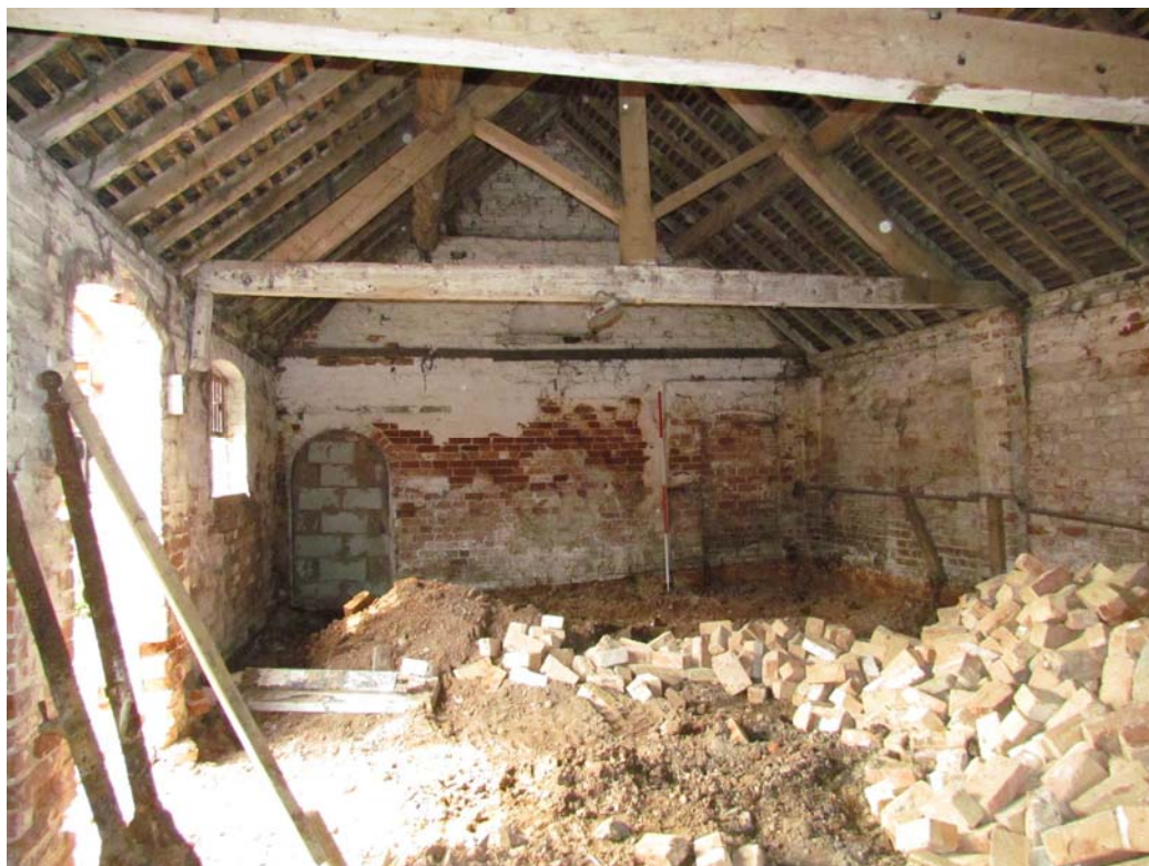
Figure 68: View Across Bay 2, Looking North-west (Scale = 2m).
