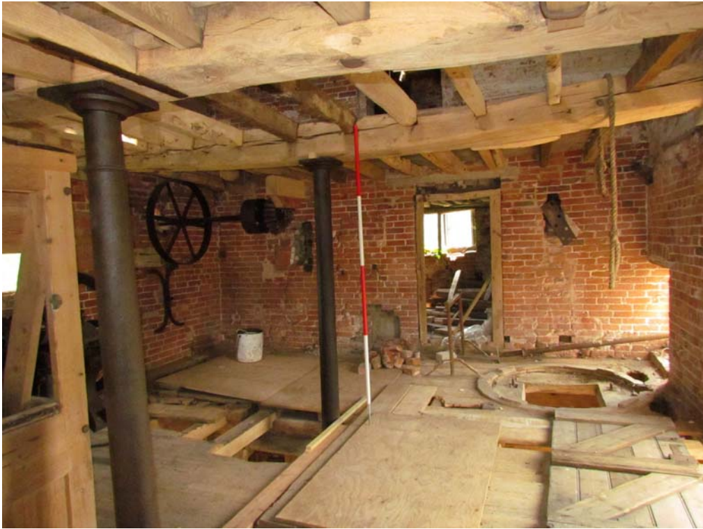
Figure 30: View Across Stone Floor, Looking South-east (Scale=2m).
