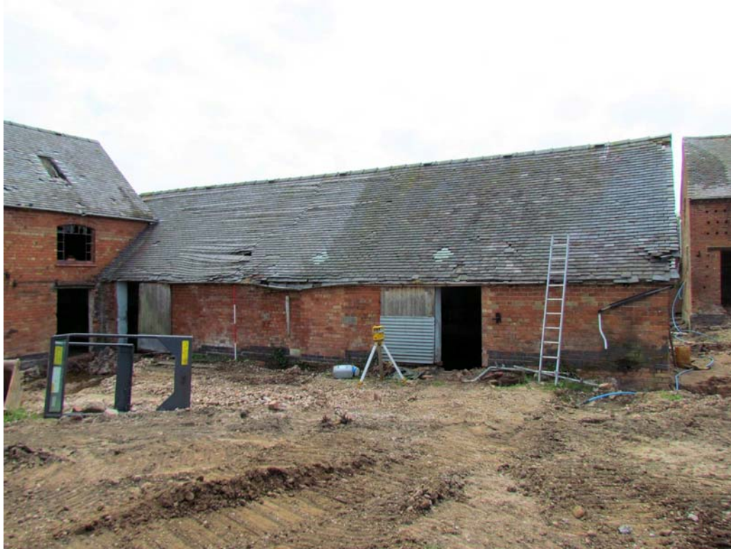
Figure 62: North-West Elevation of Barn 3, Looking South-east (Scale = 2m).
