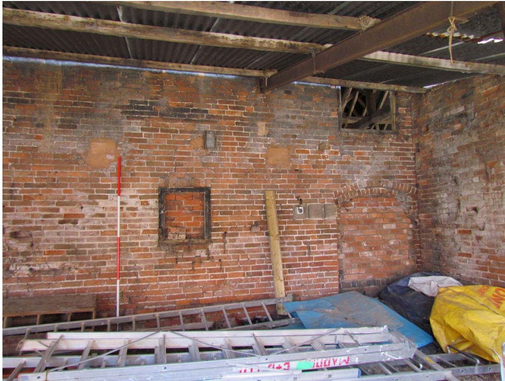
Figure 50: South-west Elevation of Bay 2, Looking North-east (Scale = 2m).
