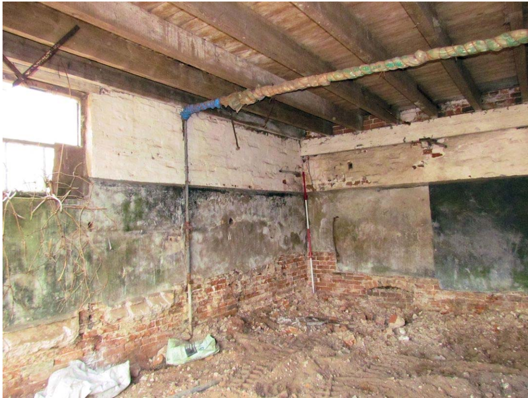
Figure 42: Interior of Bay 4, Looking East (Scale = 2m).
