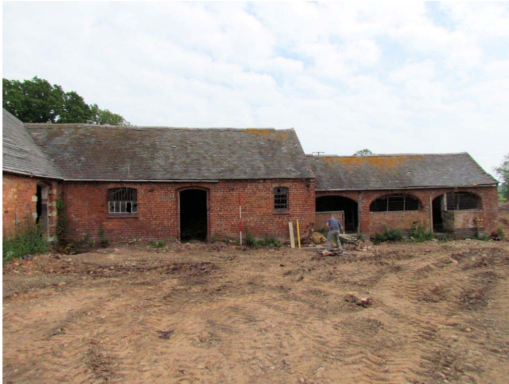
Figure 59: South-west Elevation of Bays 4 and 5, Looking North-east (Scale = 2m).
