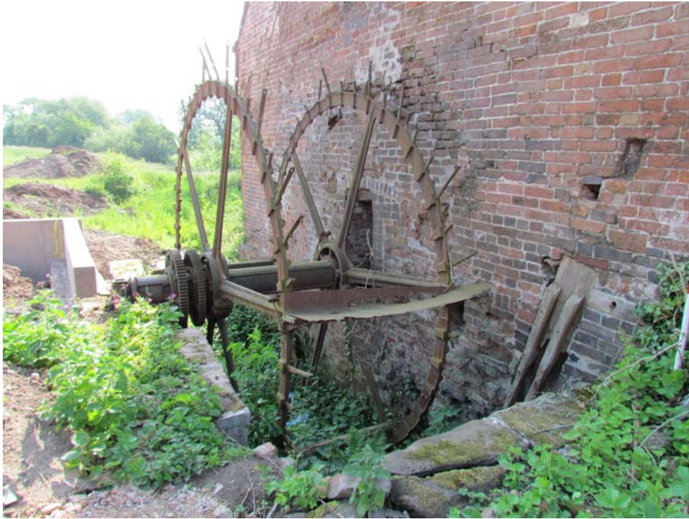
Figure 16: Detail of Waterwheel and Pit (Scale = 2m).
