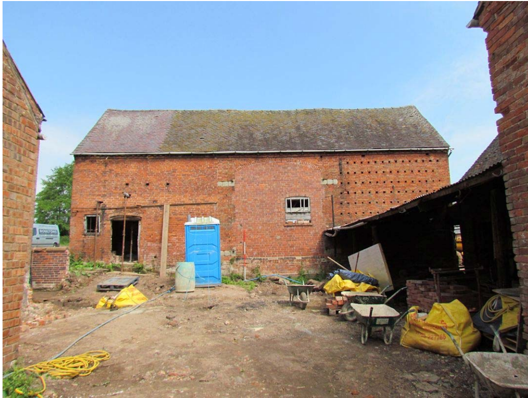
Figure 34: South-east Elevation of Barn 1, Looking North-west (Scale = 2m).
