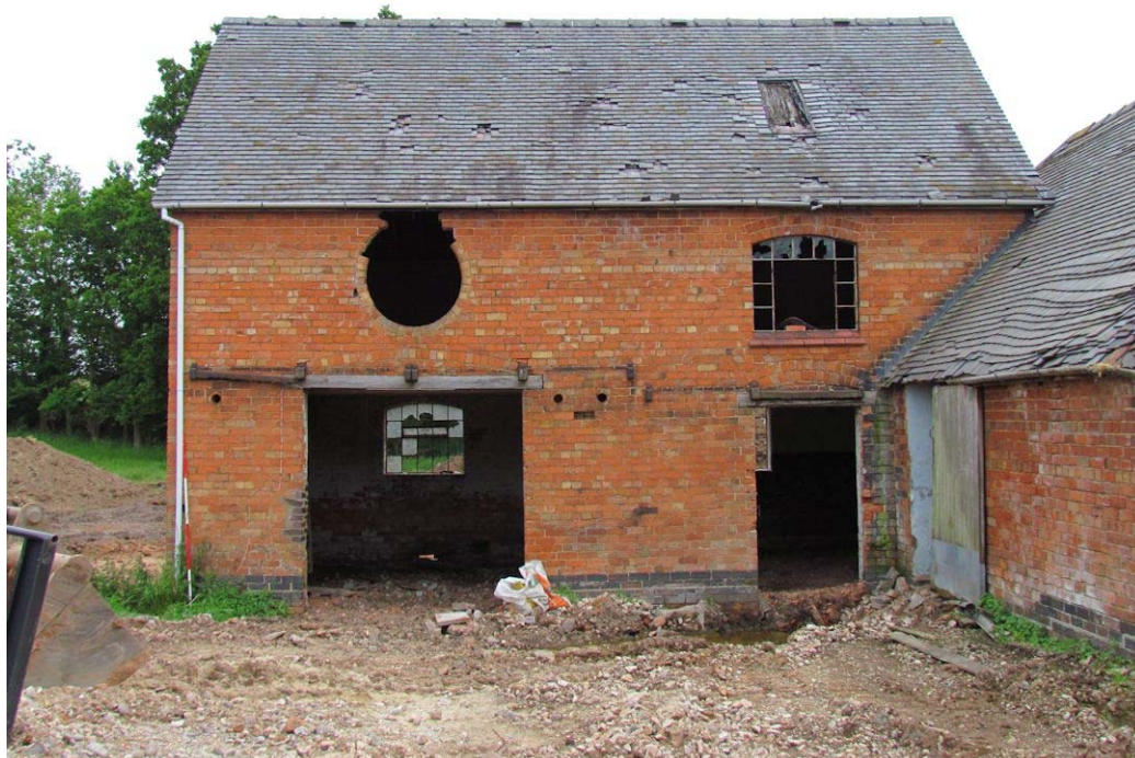
Figure 57: South-west Elevation of Bays 1 and 2, Looking North-east (Scale = 2m).
