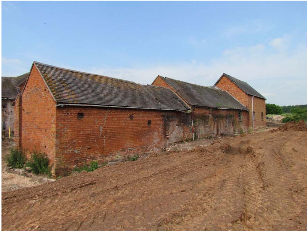
Figure 63: North-East Elevation of Barn 3, Looking North-west (Scale = 2m).
