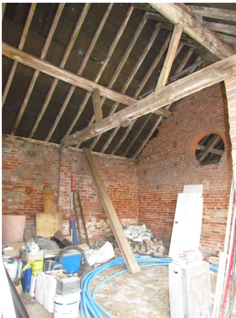
Figure 54: Bay 3, Looking North (Scale = 2m).
