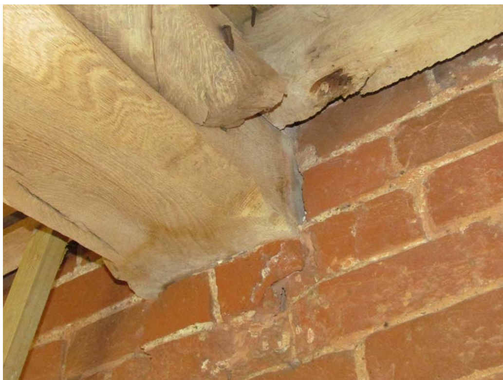
Figure 25: Detail of Chamfered and Stopped Beam.
