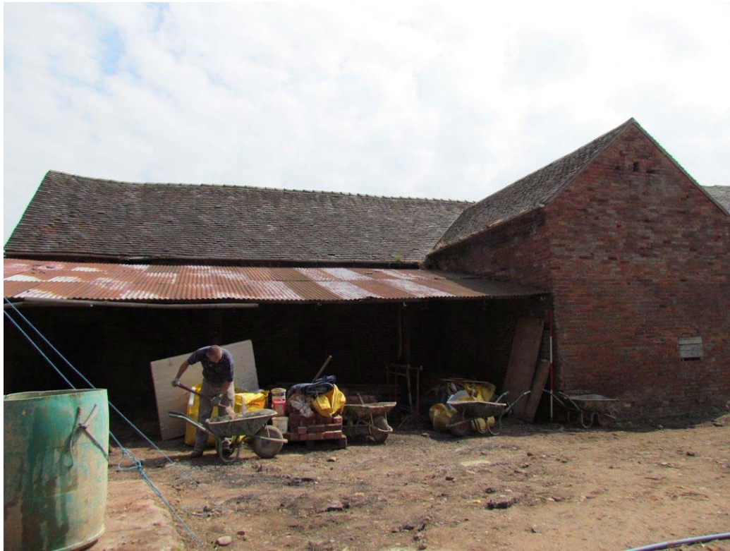
Figure 49: South-west Elevation of Barn 2, Looking North-east (Scale = 2m).
