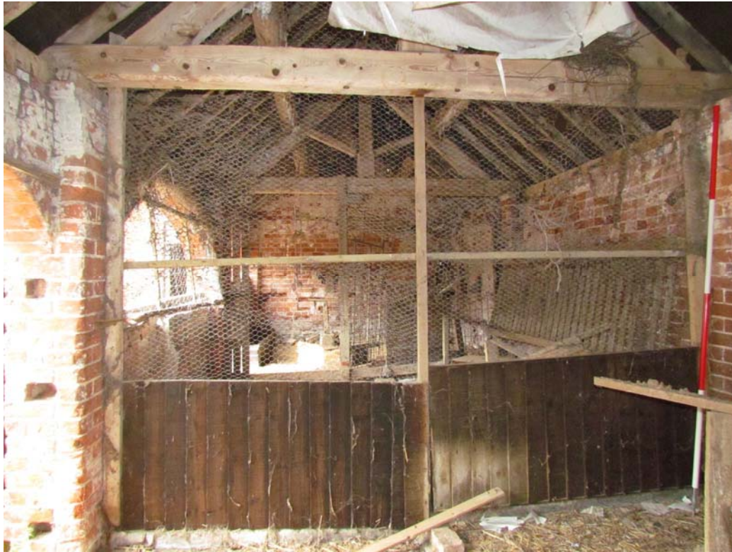
Figure 69: View Across Bay 1, Looking North-west (Scale = 2m).
