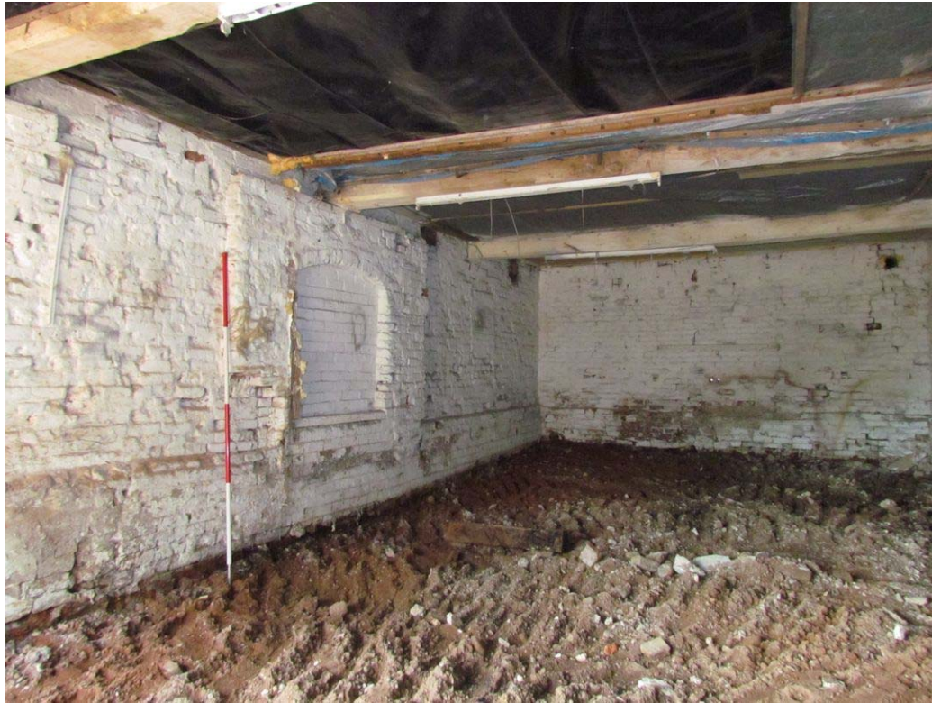
Figure 53: Bay 2, Looking West (Scale = 2m).
