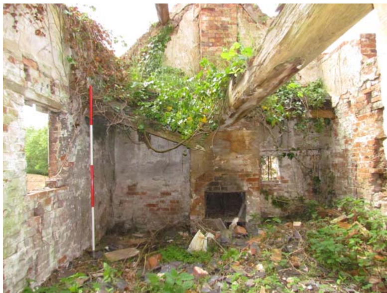
Figure 28: Office Building, Looking South-West (Scale=2m).
