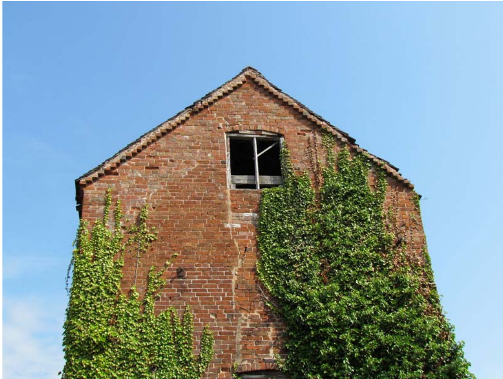
Figure 20: Detail of Upper Section Showing Changes in Brickwork.
