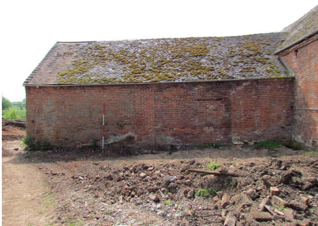
Figure 48: North-west Elevation of Bays 3 to 5, Looking South-east (Scale = 2m).
