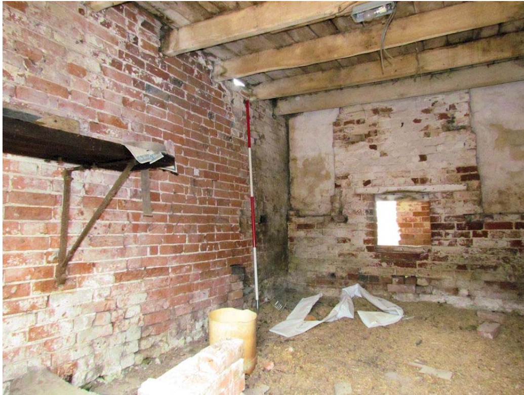
Figure 38: Interior of Bay 1, Looking West (Scale = 2m).
