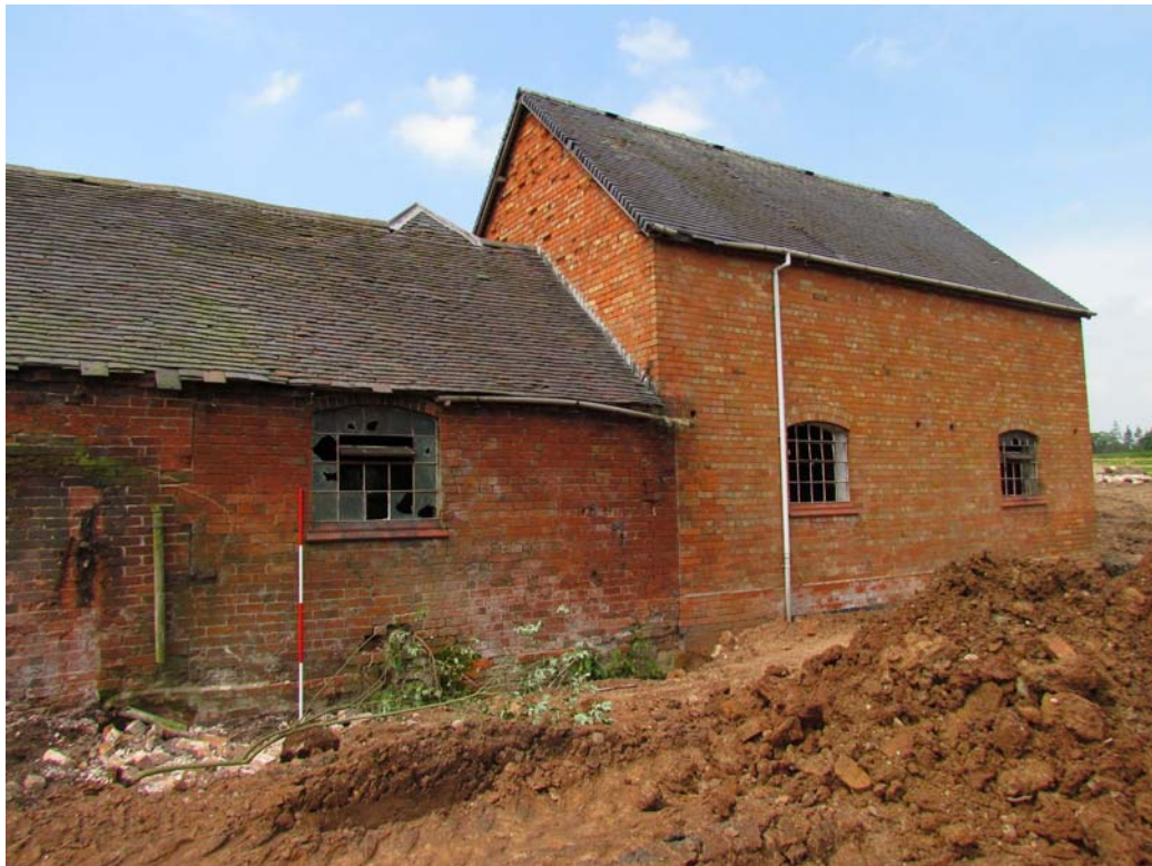
Figure 64: North-East Elevation of Bays 1 to 3, Looking North-west (Scale = 2m).
