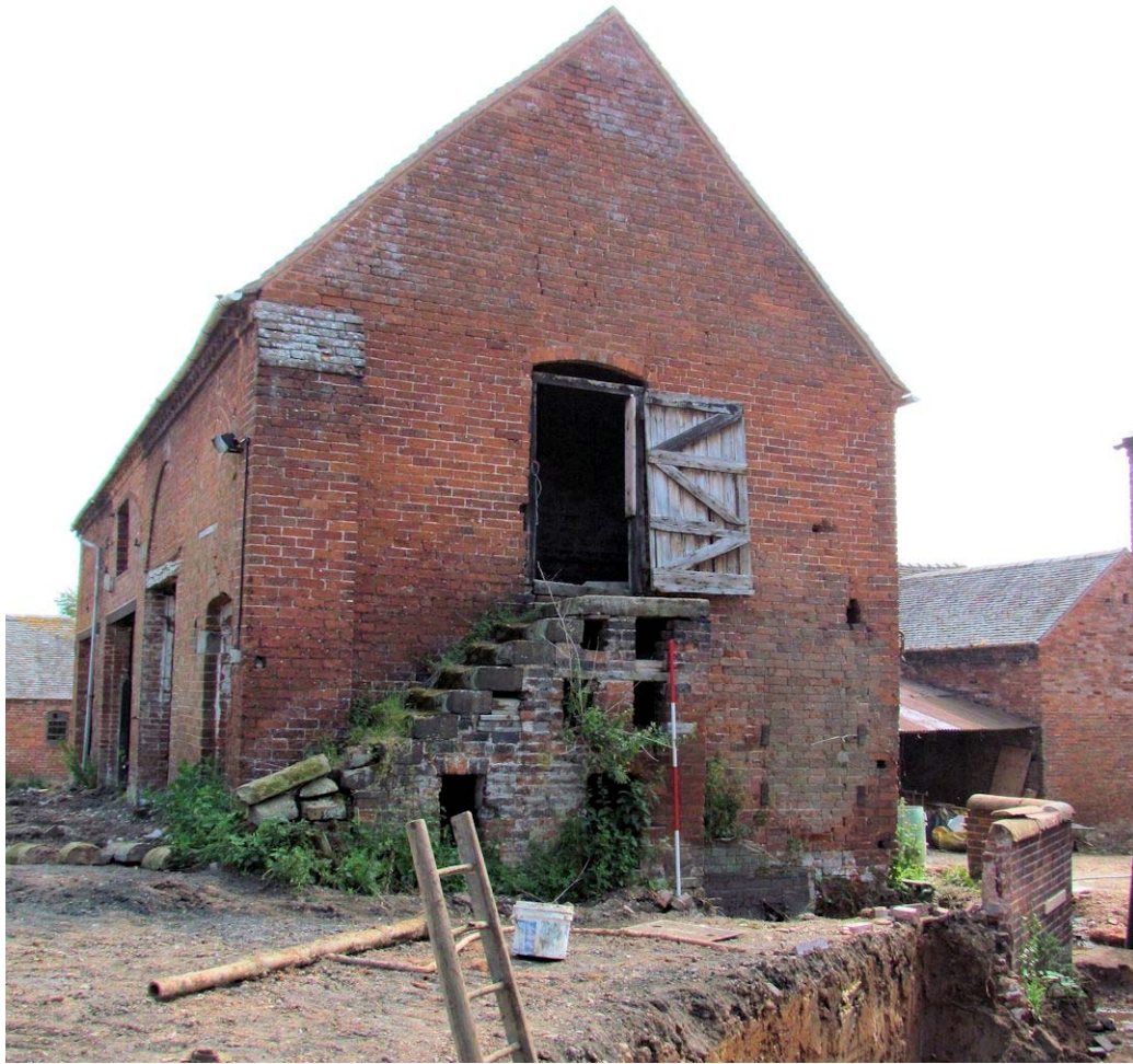
Figure 36: South west Elevation, Looking North-east (Scale = 2m).
