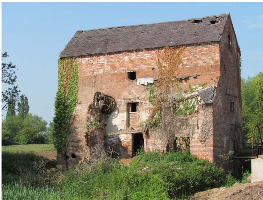
Figure 21: East Elevation, Looking West (Scale=2m).
