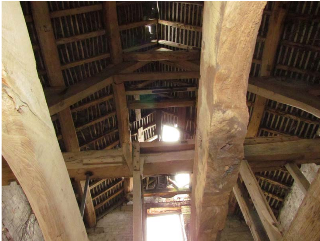
Figure 32: View of Roof Structure from Stone Floor, Looking North.
