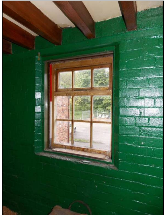
Figure 127: Detail of window, looking south-west (scale 1m).
