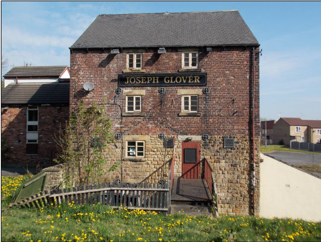
Figure 15: South elevation of Building A (scale 2m).
