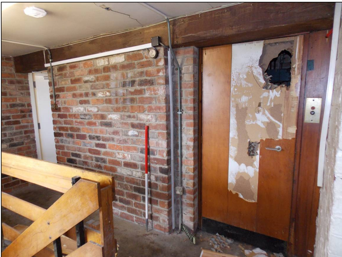
Figure 54: Lobby S6, looking west (scale 1m).
