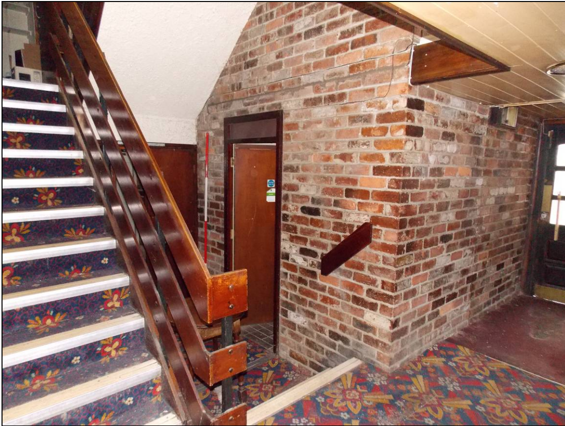
Figure 167: Staircase well within the ground floor, looking north-west (scale 2m).
