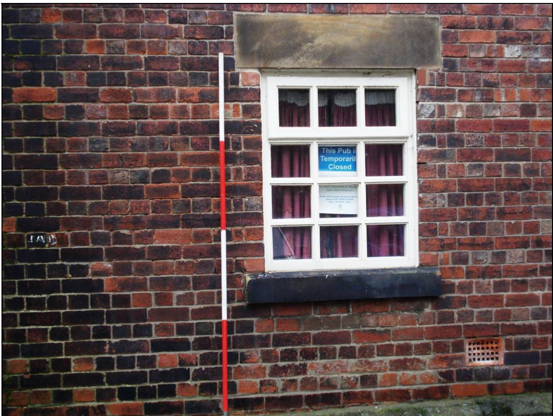
Figure 88: Detail of window opening, looking east (scale 2m).
