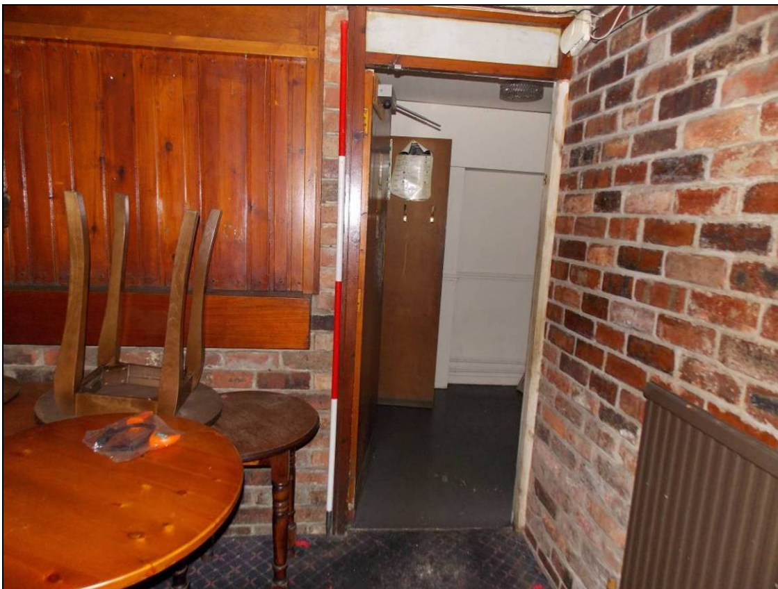
Figure 168: Doorway to the gents lavatory within the ground floor, looking west (scale 2m).
