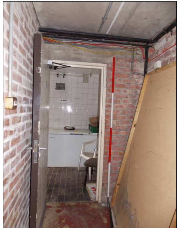
Figure 155: Doorway to the kitchen, looking east (scale 2m).
