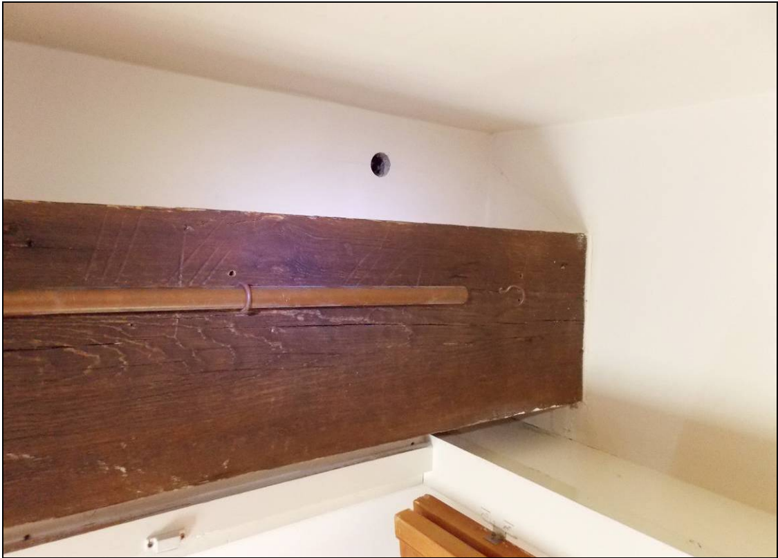
Figure 59: Detail of carpenter's marks on the underside of the central beam.
