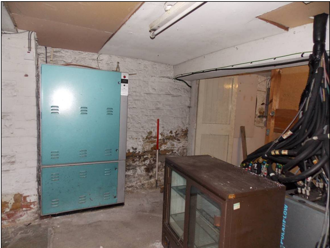
Figure 25: South-east room, looking south (scale 1m).
