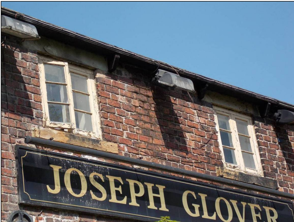
Figure 16: Window openings within the second floor.
