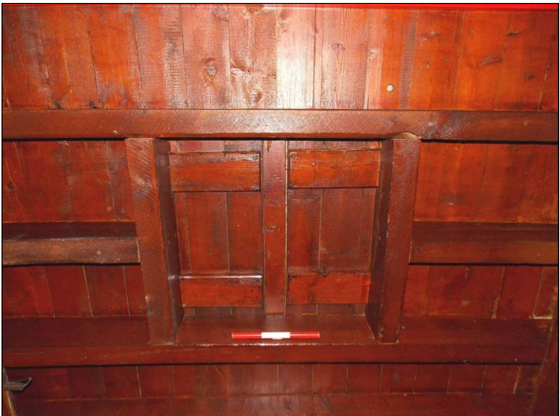
Figure 101: Detail of ceiling hatch, looking east (scale 300mm).
