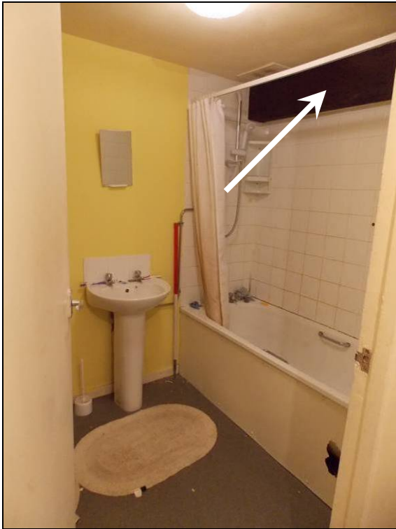
Figure 67: Lavatory S5 with eastern tie-beam containing carpenter's marks (arrow) (scale 1m).
