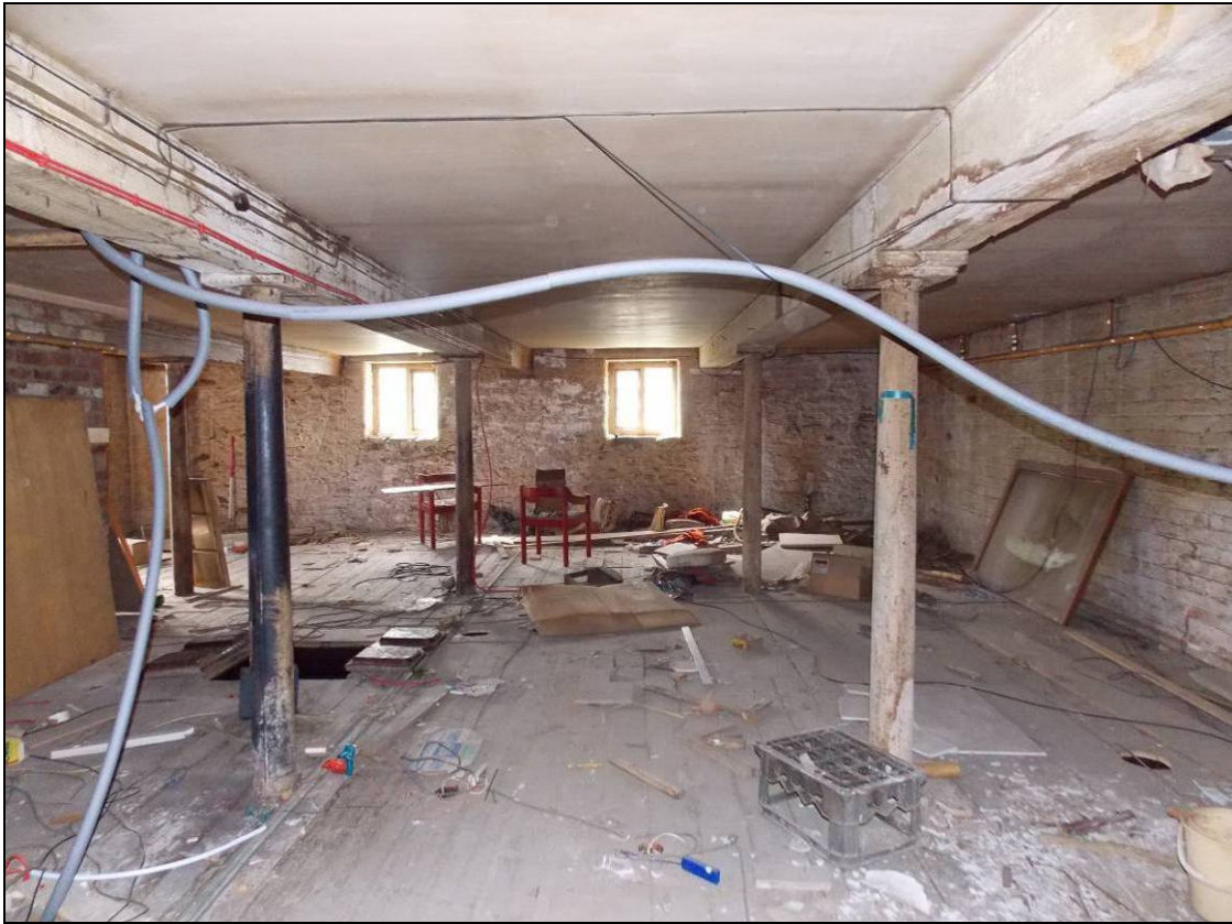
Figure 41: General view of the first floor, looking south (scale 1m).
