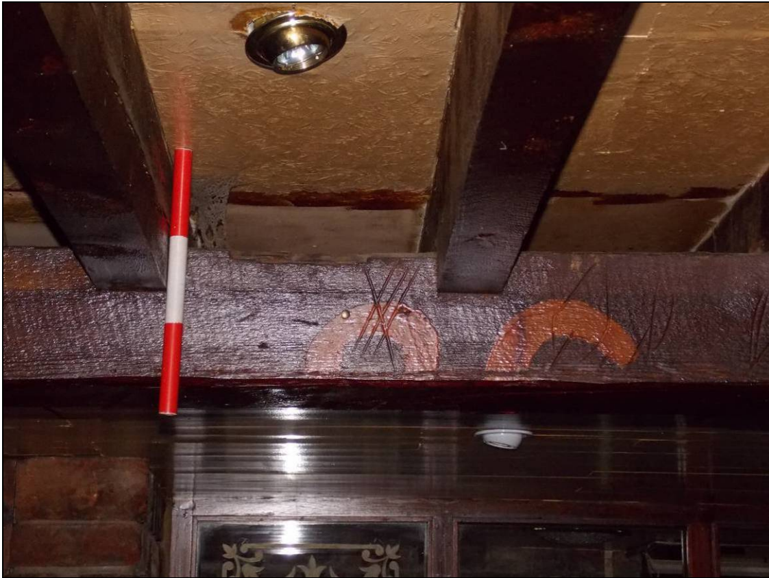
Figure 38: Carpenter's marks within the northern section of the western beam (scale 300mm).
