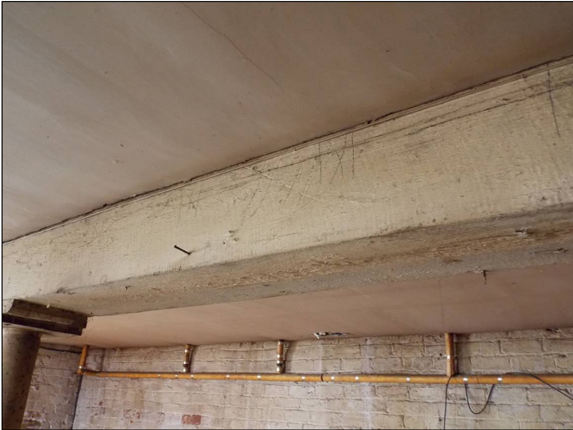
Figure 52: Carpenter's marks within the western beam, looking south-west.
