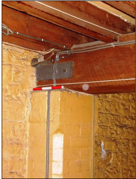
Figure 114: Detail of plate attaching longitudinal beams, looking south-west (scale 300mm).
