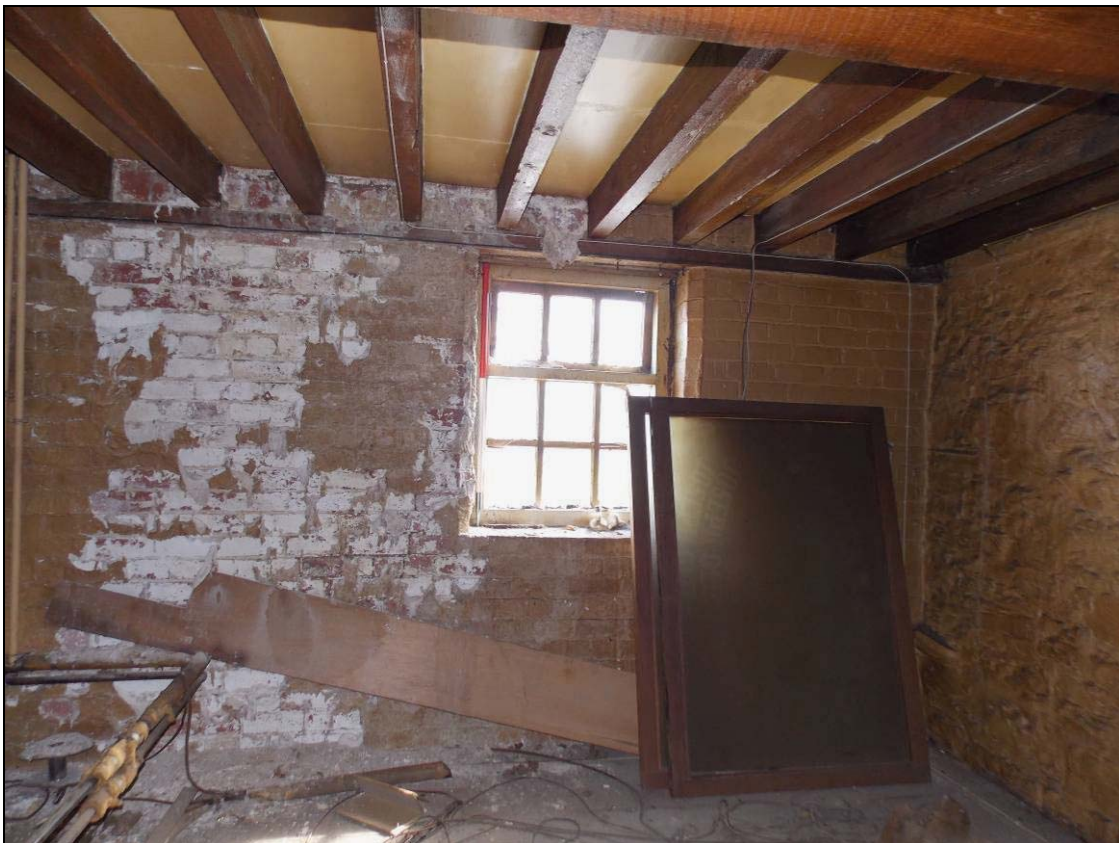
Figure 110: Southern bay of the first floor, looking east (scale 1m).
