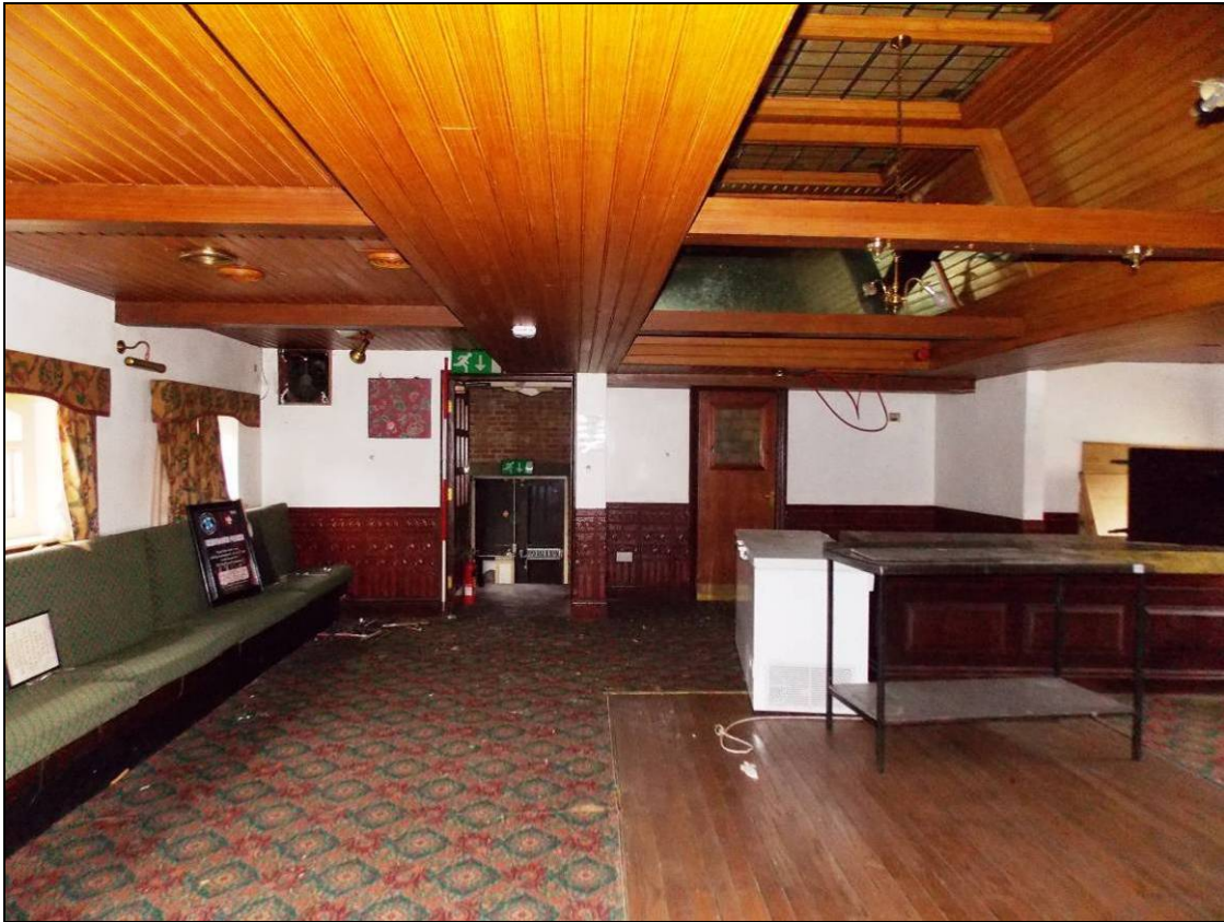
Figure 159: Ground floor, looking north (scale 2m).
