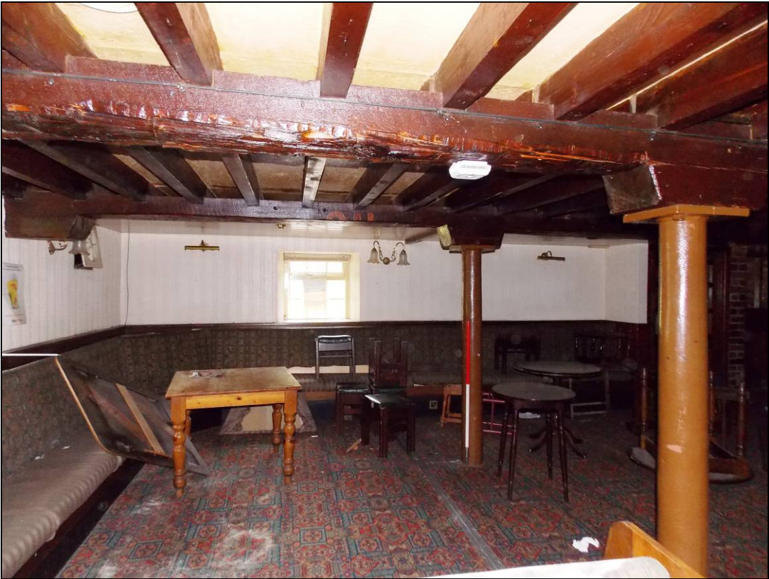
Figure 30: Ground floor, looking west (scale 1m).
