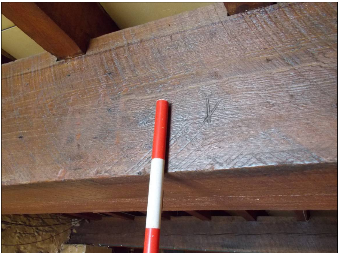
Figure 112: Detail of carpenter's marks within the eastern beam (scale 200mm).
