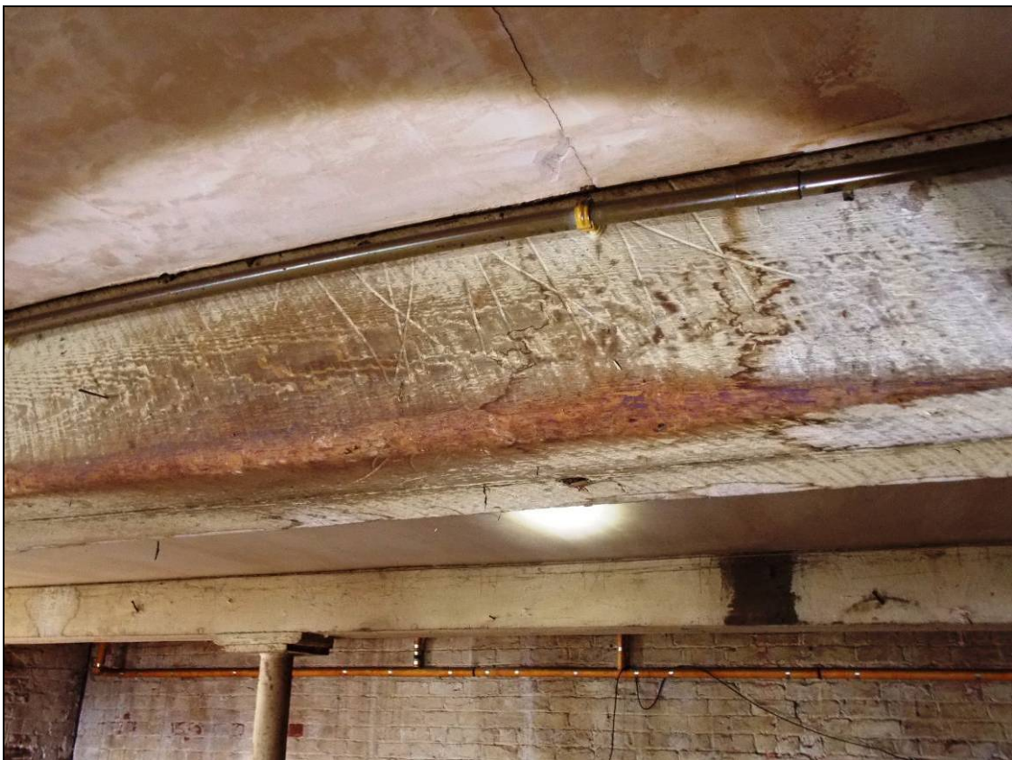
Figure 51: Carpenter's marks within the central beam, looking west.
