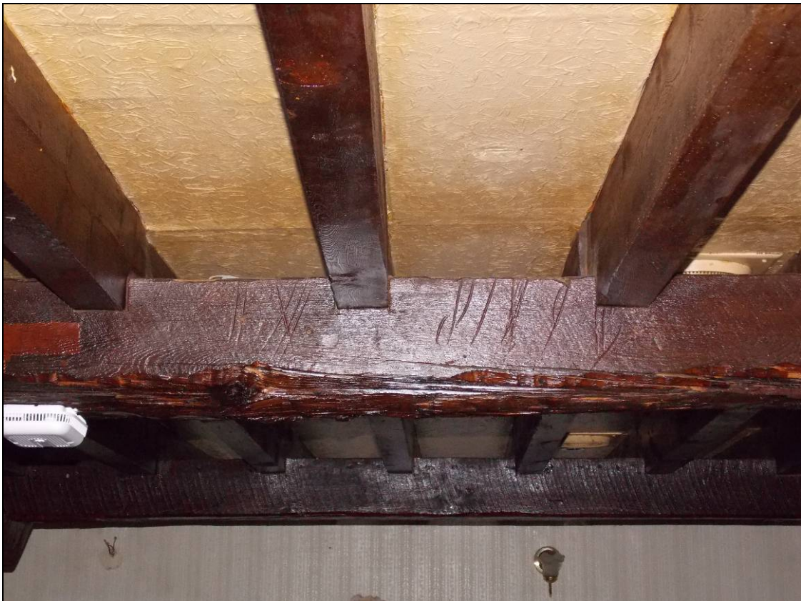
Figure 35: Carpenter's marks within southern section of the central beam, looking east.
