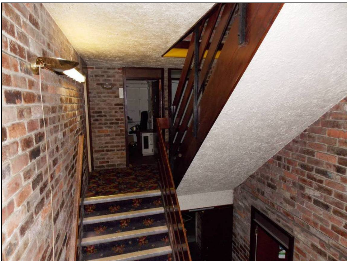
Figure 170: Staircase to the upper floors, looking west.
