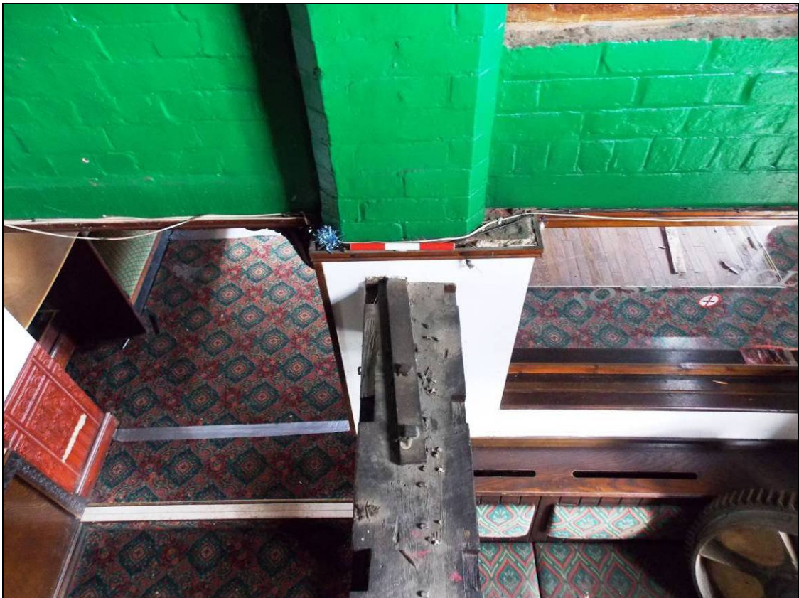
Figure 134: Detail of tie-plate attached to the eastern beam, looking north (scale 300mm).
