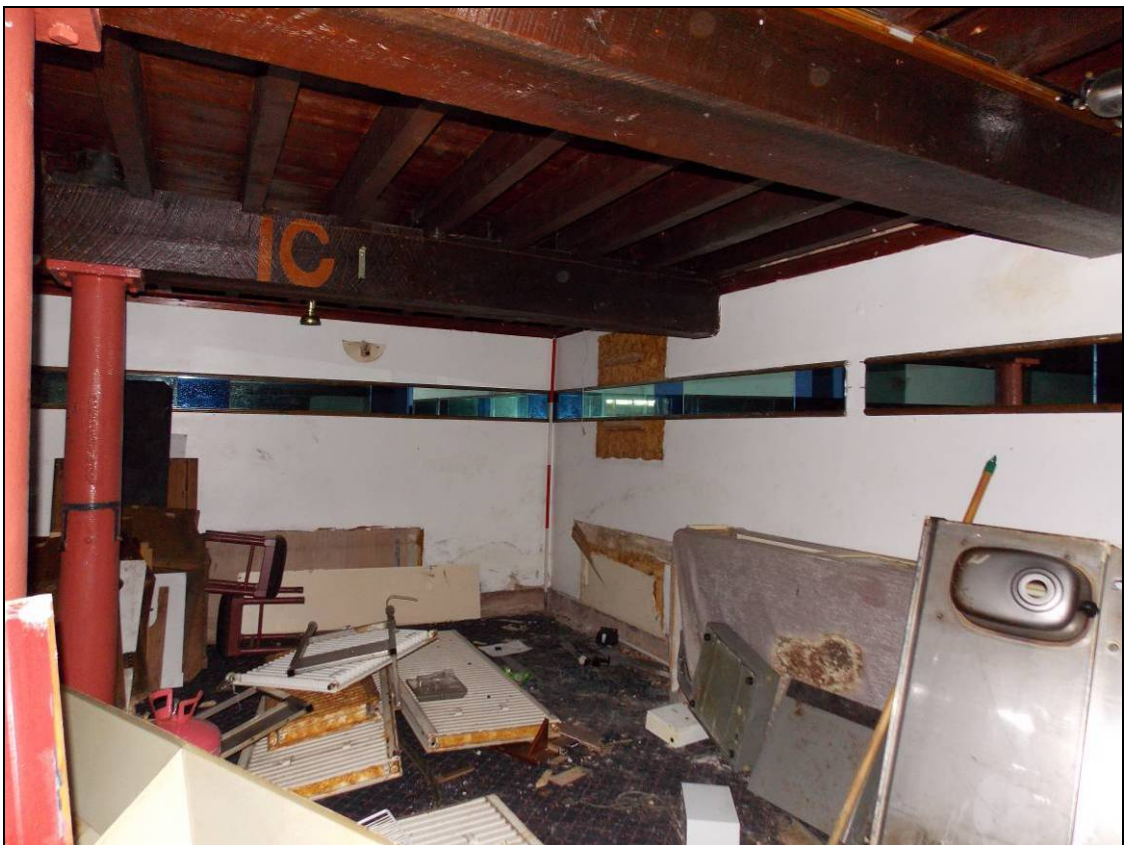
Figure 99: North wall after soft-stripping, looking north-west (scale 2m).
