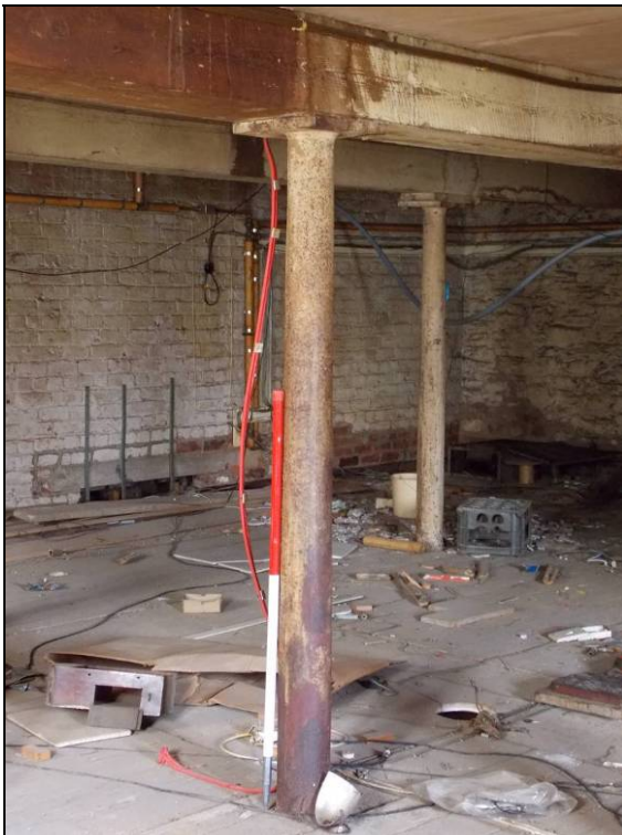
Figure 46: Detail of cast-iron column, looking north-west (scale 1m).
