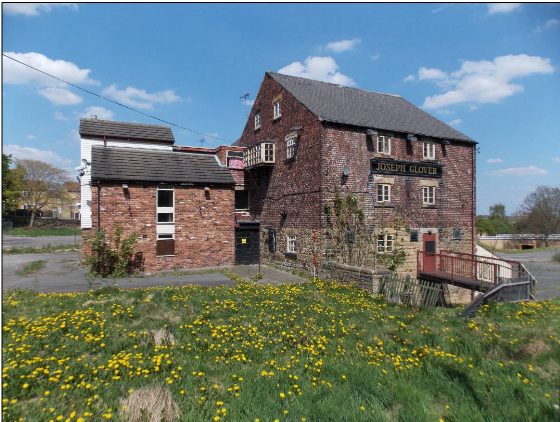
Figure 14: General view of the south elevation of Building A with later Building D to the left (scale 2m).
