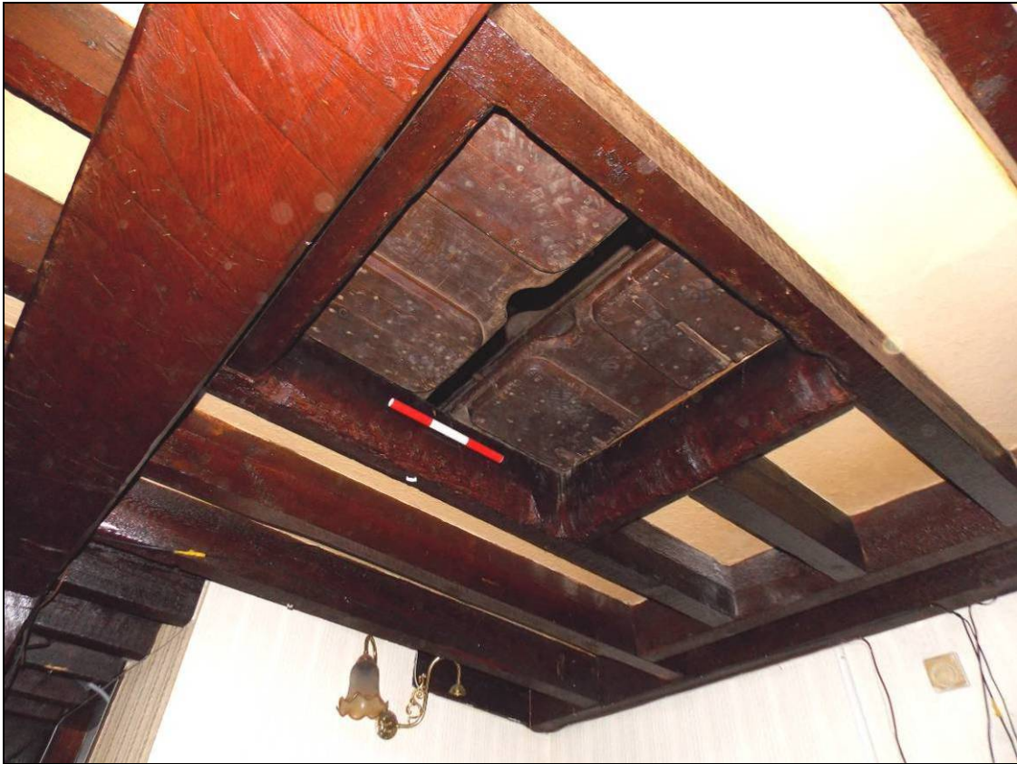
Figure 34: Ceiling hatch, looking north-east (scale 300mm).
