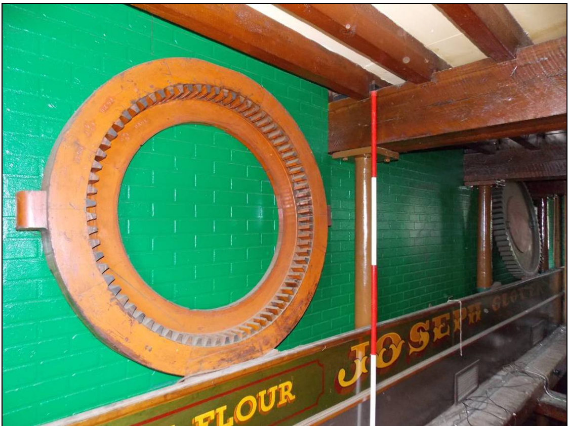
Figure 119: Fake brick stud panel with bevelled gears (scale 2m).
