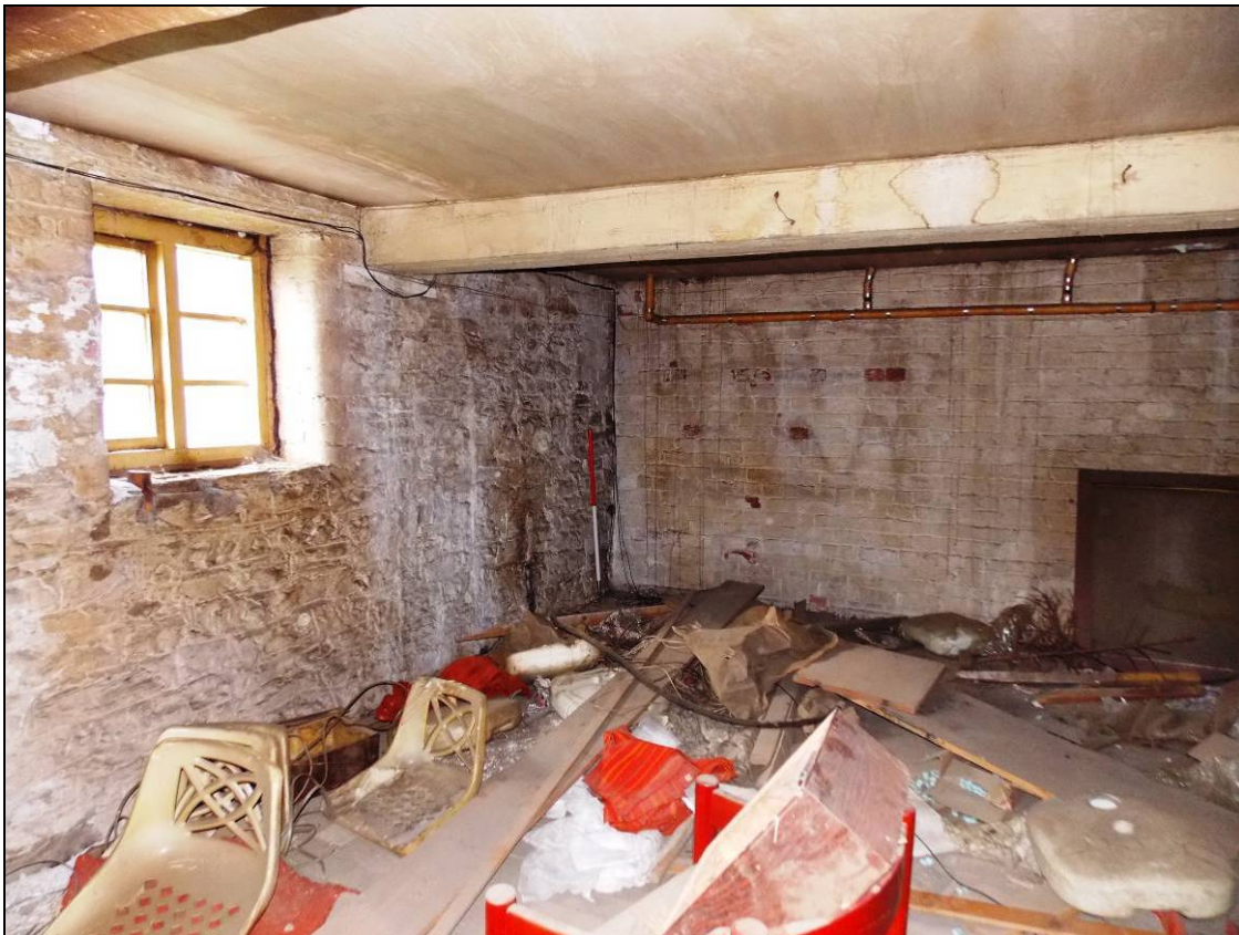
Figure 42: South-western corner of the first floor (scale 1m).
