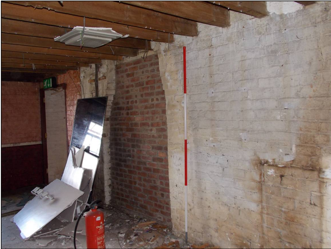
Figure 142: Former opening within the south wall, looking south-east (scale 2m).
