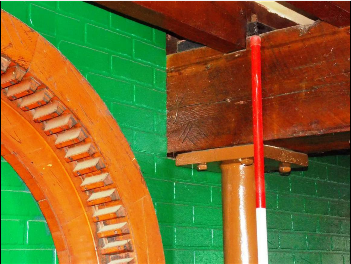
Figure 122: Carpenter's marks within the eastern beam and above the southernmost column (scale 500mm).
