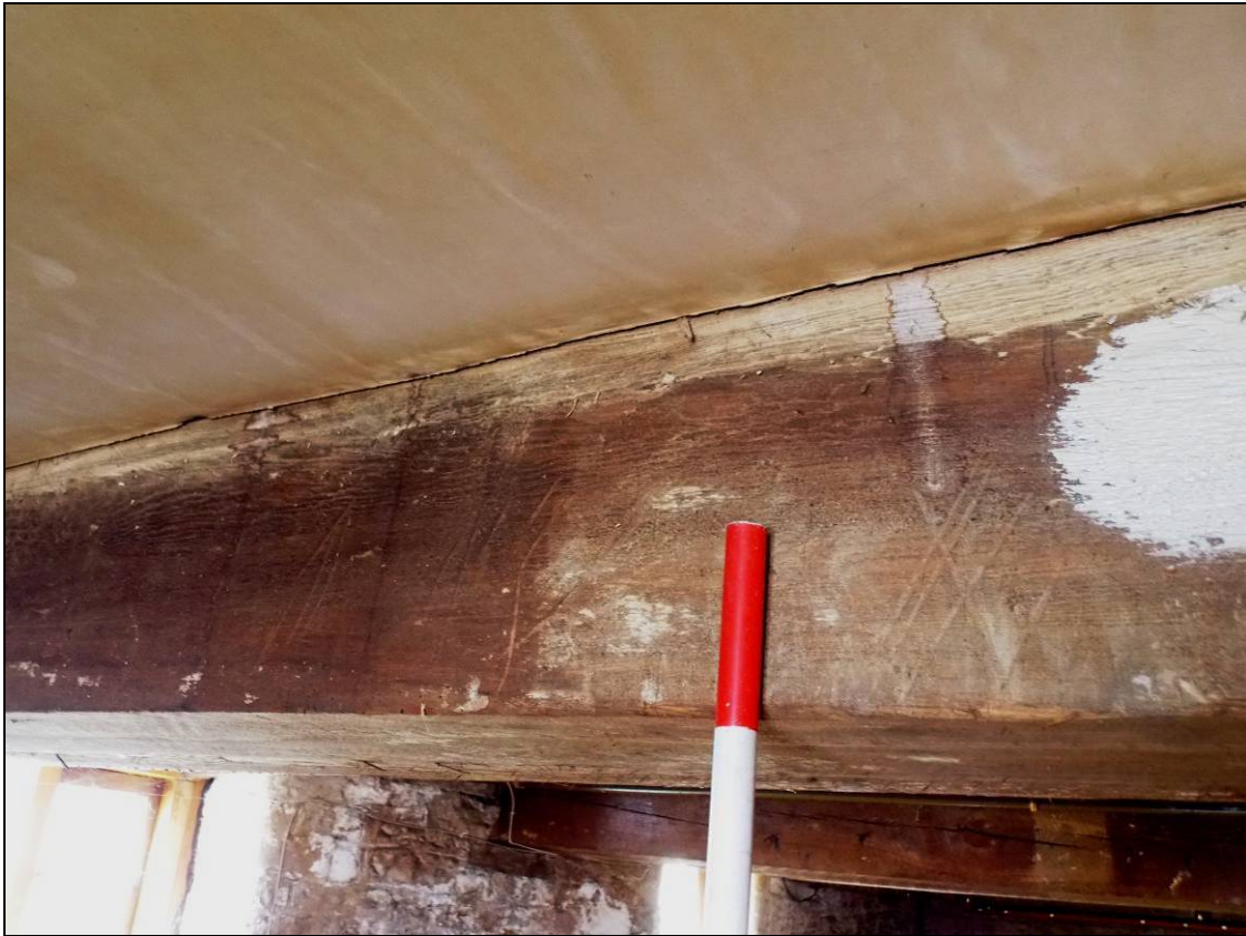
Figure 50: Carpenter's marks within the eastern beam, looking south-west (scale 200mm).
