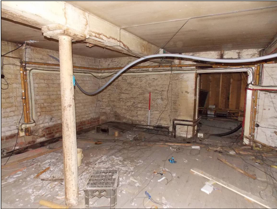
Figure 45: Inserted doorway within the north wall providing access to Building B (scale 1m).
