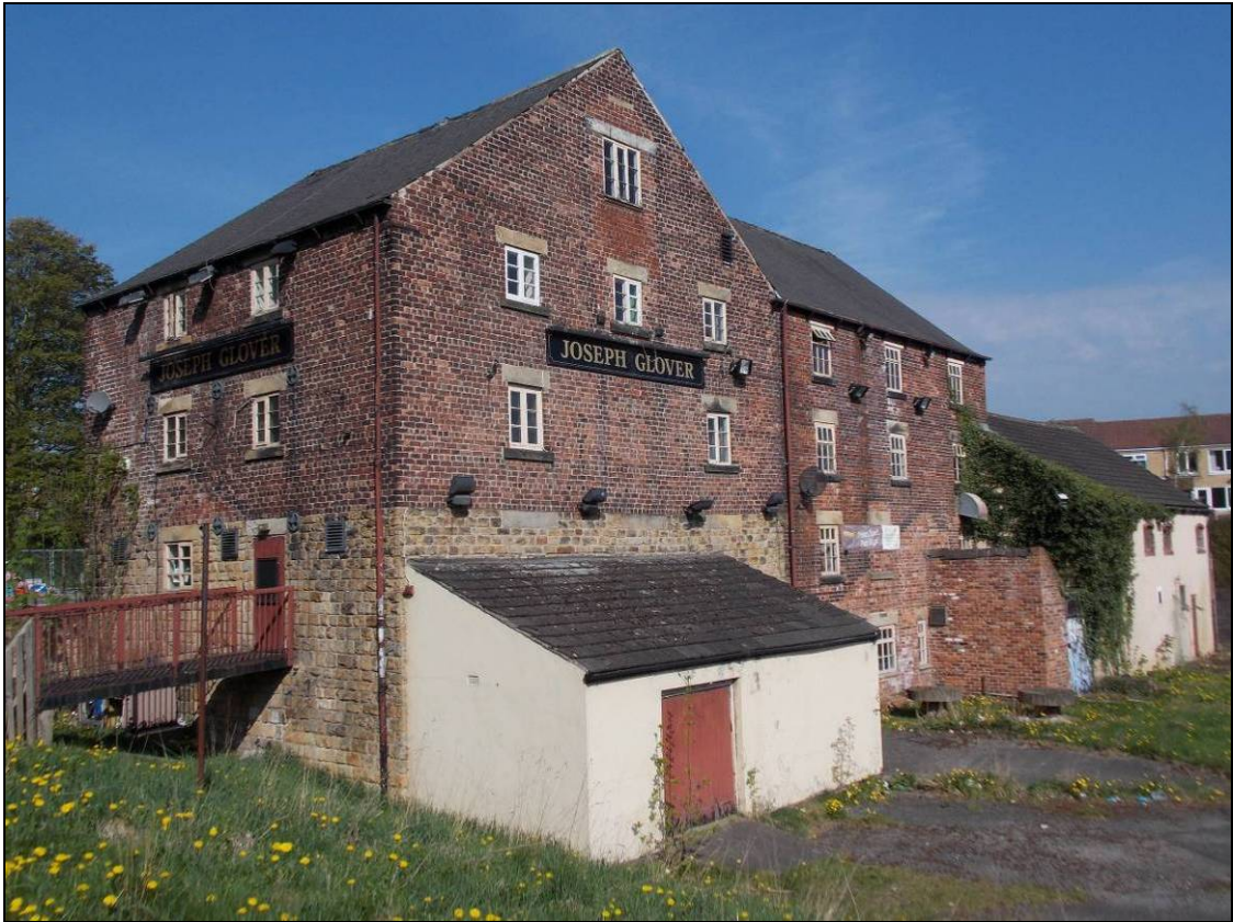
Figure 6: General view of the east elevation of Building A, looking north-west.
