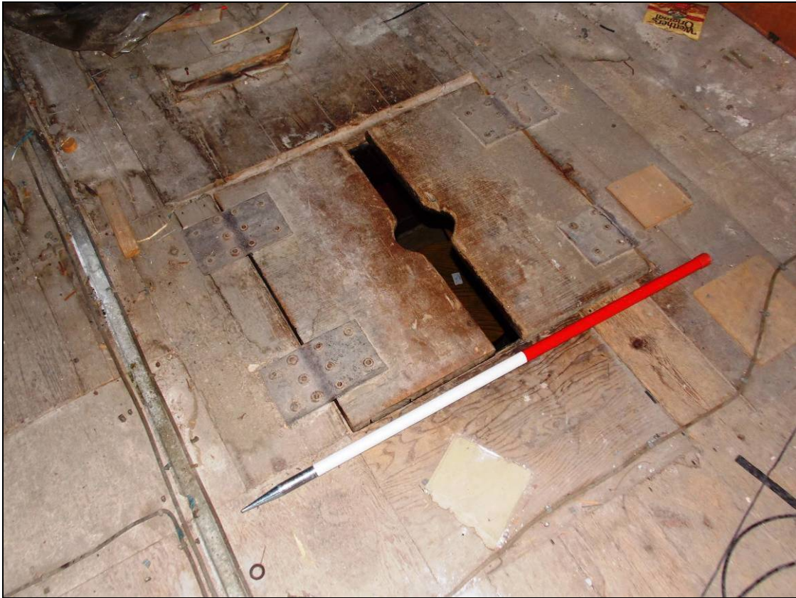
Figure 43: Detail of hatch within the floor boards, looking north-east (scale 1m).
