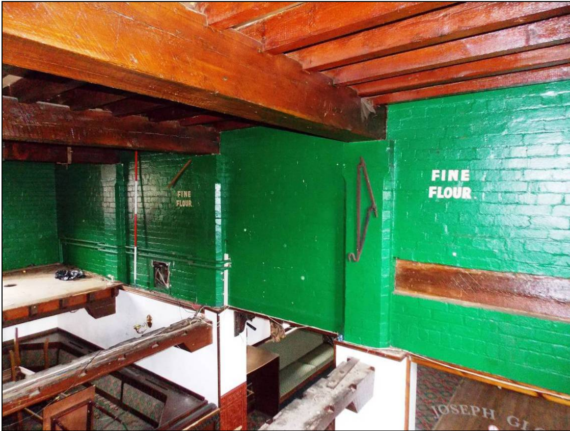
Figure 131: North wall with timber lintel within the eastern bay (scale 2m).
