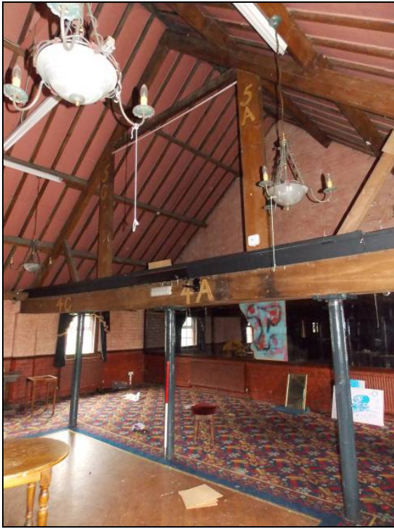
Figure 136: First floor, looking north-west (scale 1m).
