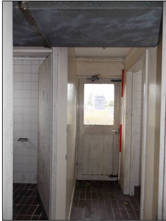
Figure 157: Passageway to lavatories and external doorway, looking east (scale 2m).
