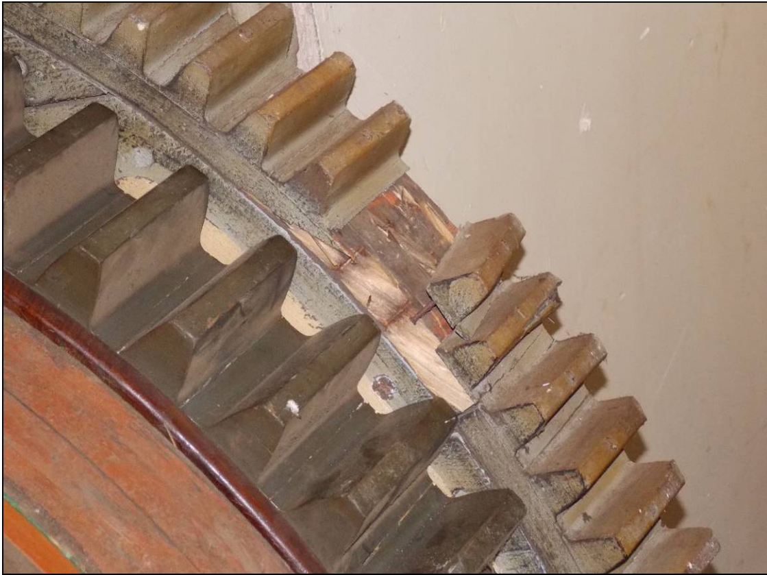
Figure 120: Detail of fake gear recorded during the soft-stripping watching brief.
