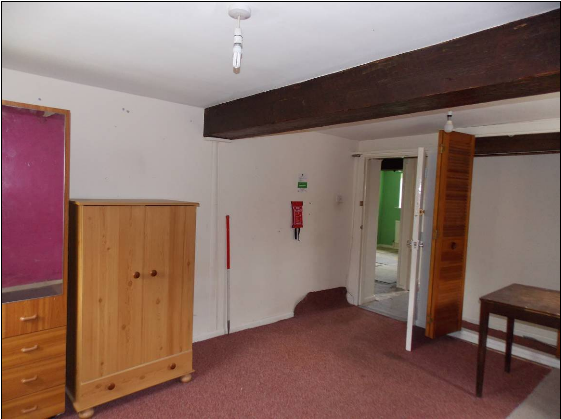
Figure 57: Room S2, looking north-east (scale 1m).
