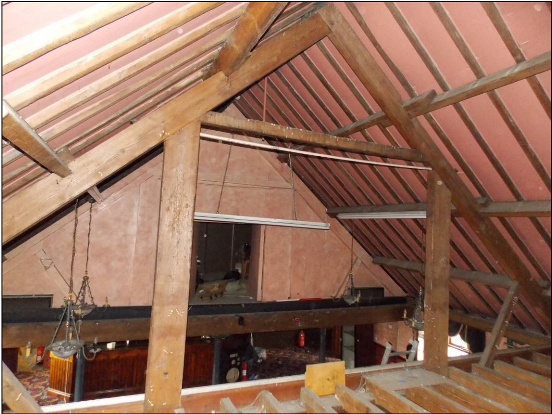
Figure 143: General view of the loft, looking south (scale 1m).
