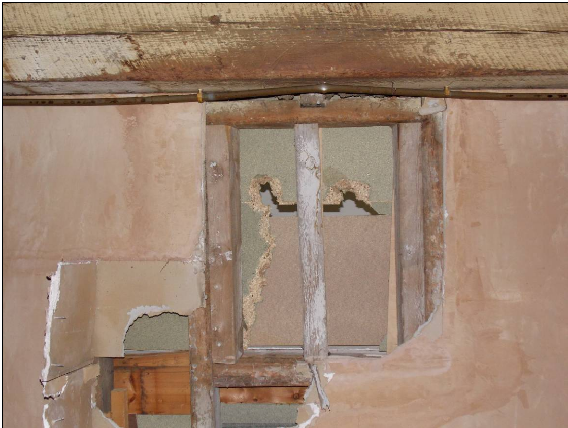
Figure 49: Remnants of ceiling hatch identified during the soft-stripping watching brief.
