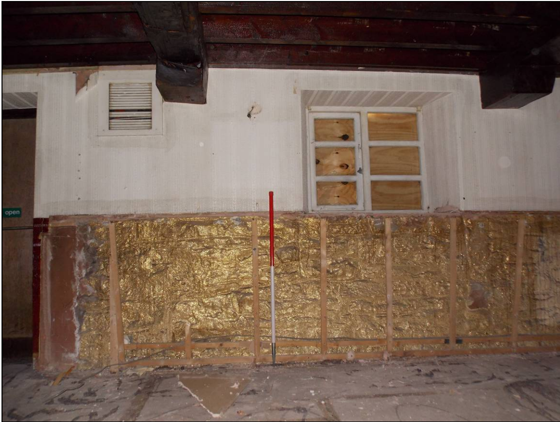
Figure 28: Stone wall revealed after soft-stripping watching brief (scale 1m).
