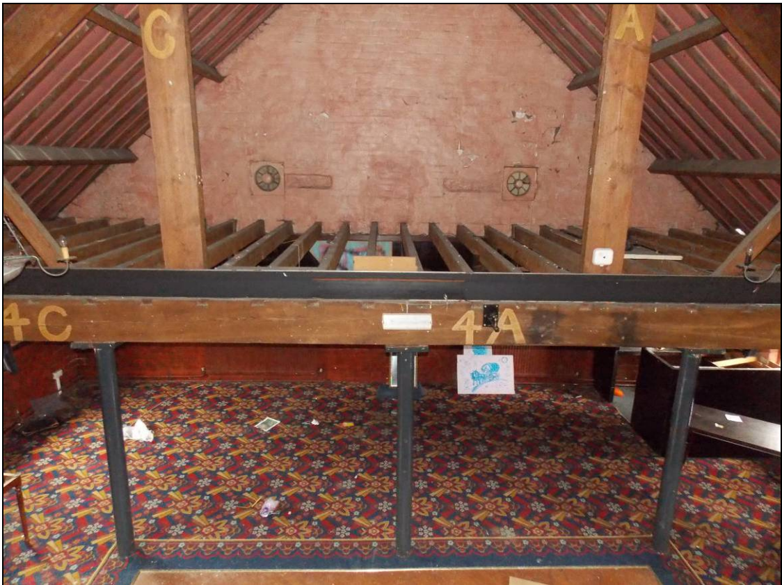
Figure 144: Central and northern bays, looking north.
