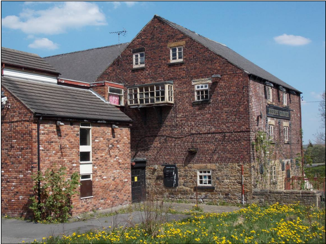
Figure 11: General view of the west elevation of Building A (scale 2m).
