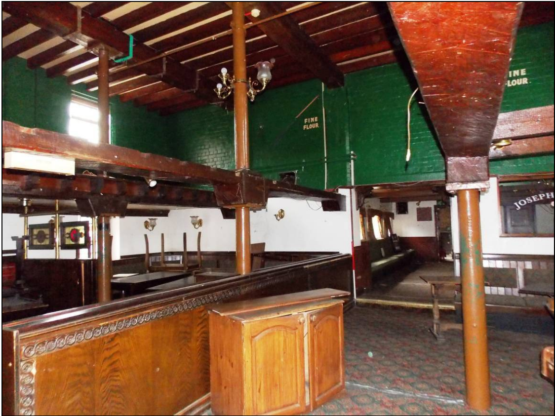
Figure 105: Ground floor, looking north-west (scale 1m).
