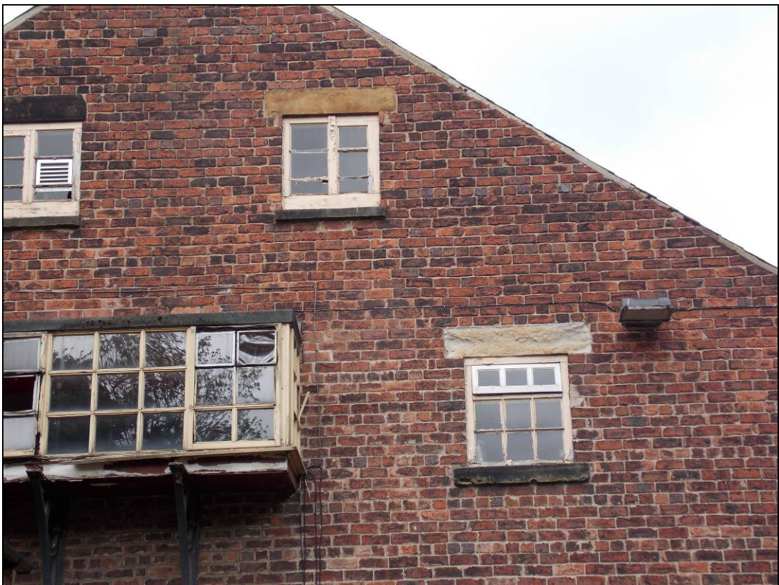
Figure 12: Detail of different brickwork within the gable.
