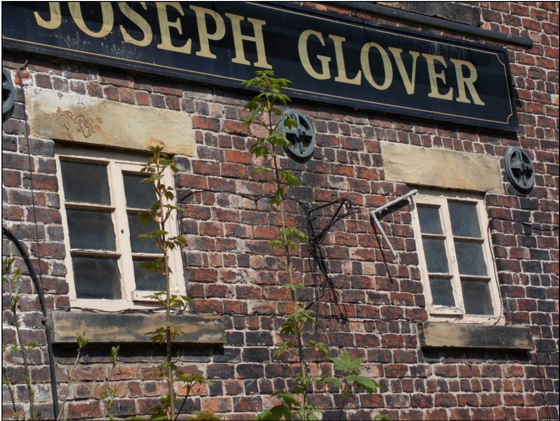
Figure 17: Window openings within the first floor.
