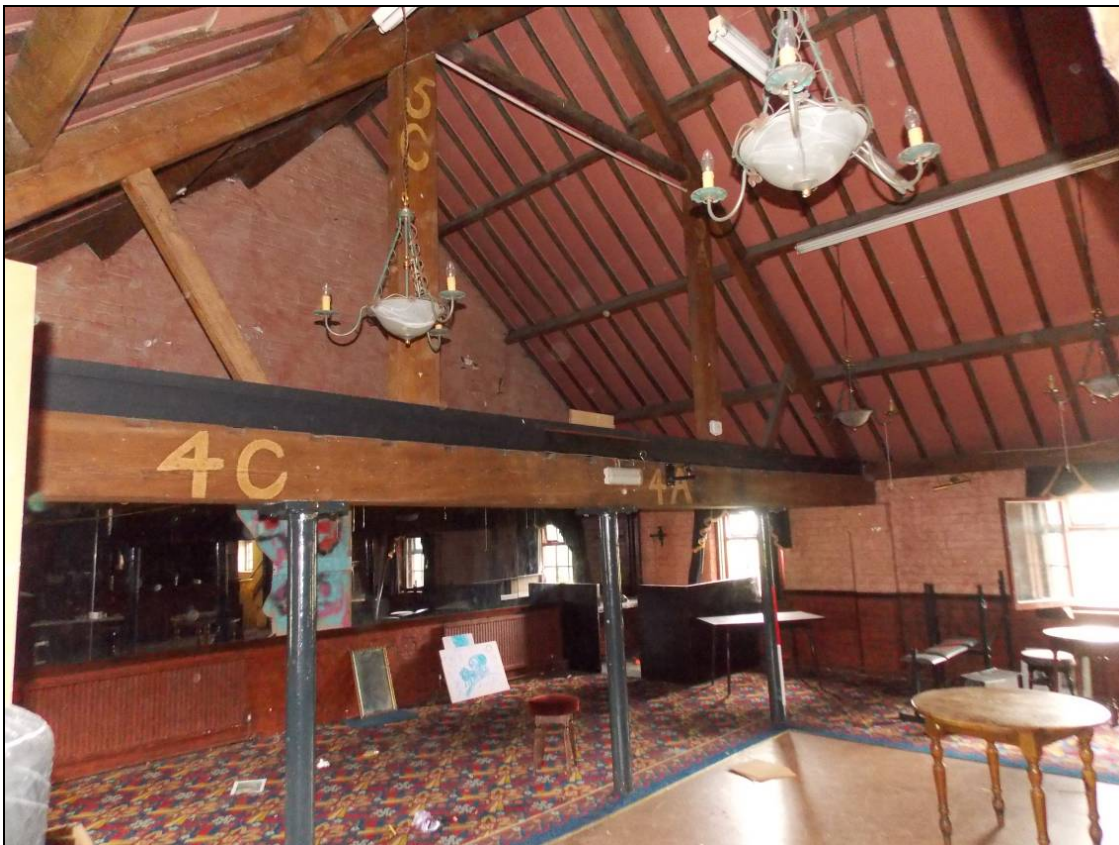
Figure 135: General view of the second floor, looking north-east (scale 1m).
