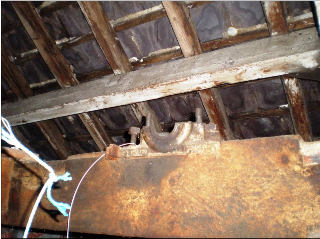
Figure 81: Remnants of former bearing housing, looking south.
