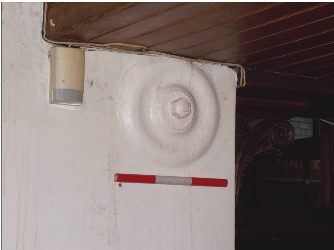
Figure 92: Detail of wall plate, looking south (scale 300mm).
