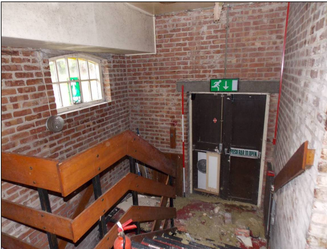
Figure 152: Staircase to the basement of Building C, looking north-west (scale 2m).
