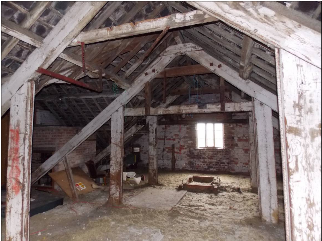
Figure 76: General view of the loft, looking east (scale 2m).
