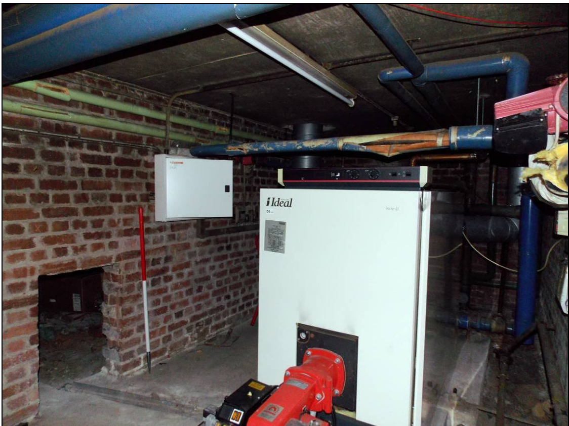
Figure 166: Boiler room within the basement, looking west (scale 1m).
