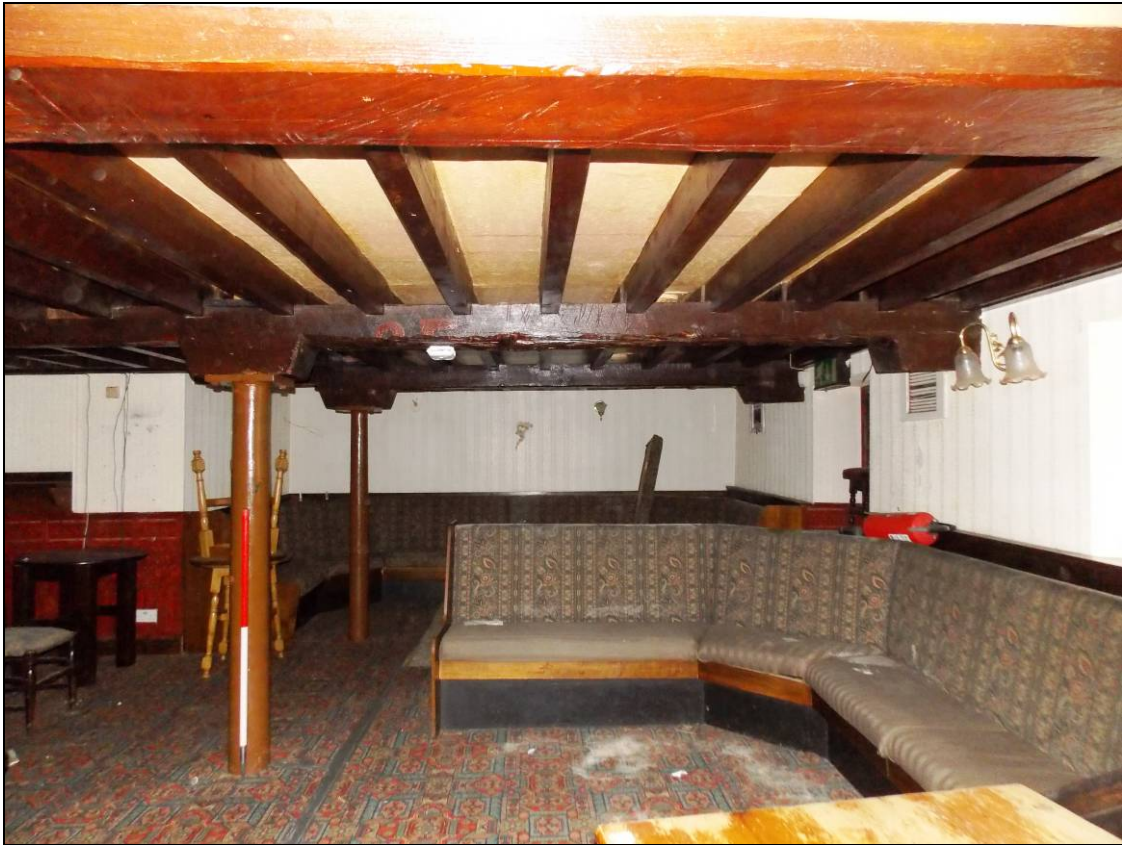
Figure 32: Ground floor, looking east (scale 1m).
