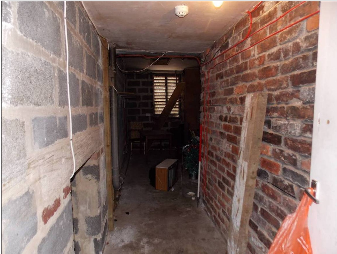
Figure 174: Second floor of Building D, looking west (scale 1m).
