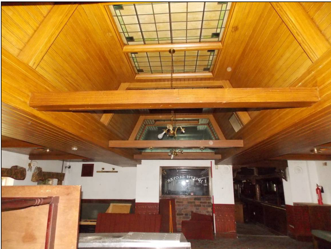
Figure 158: General view of the ground floor of Building C, looking south (scale 2m).
