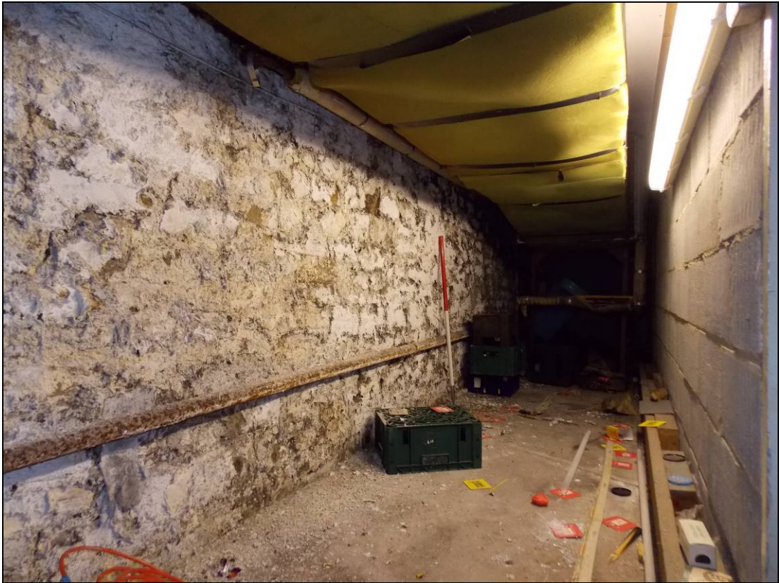
Figure 24: West wall of the basement, looking north (scale 1m).
