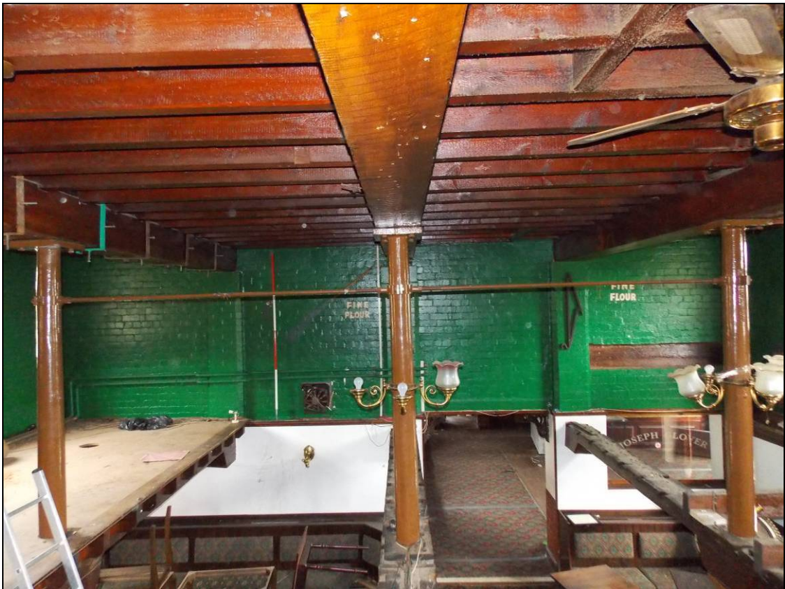
Figure 130: General view of the north wall, looking north-west (scale 2m).
