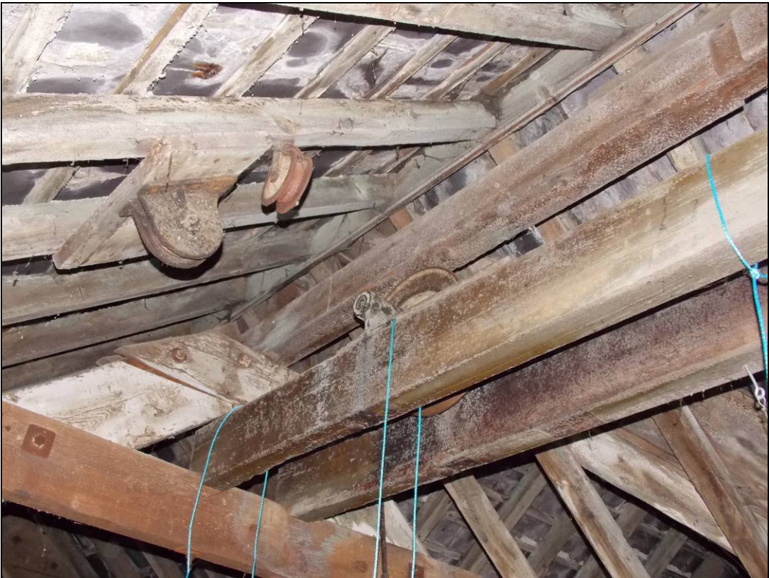
Figure 80: Detail of the pulley wheels, looking east.
