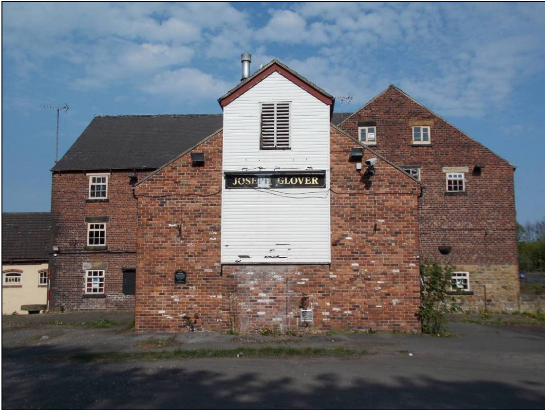
Figure 162: West elevation of Building D (scale 2m).
