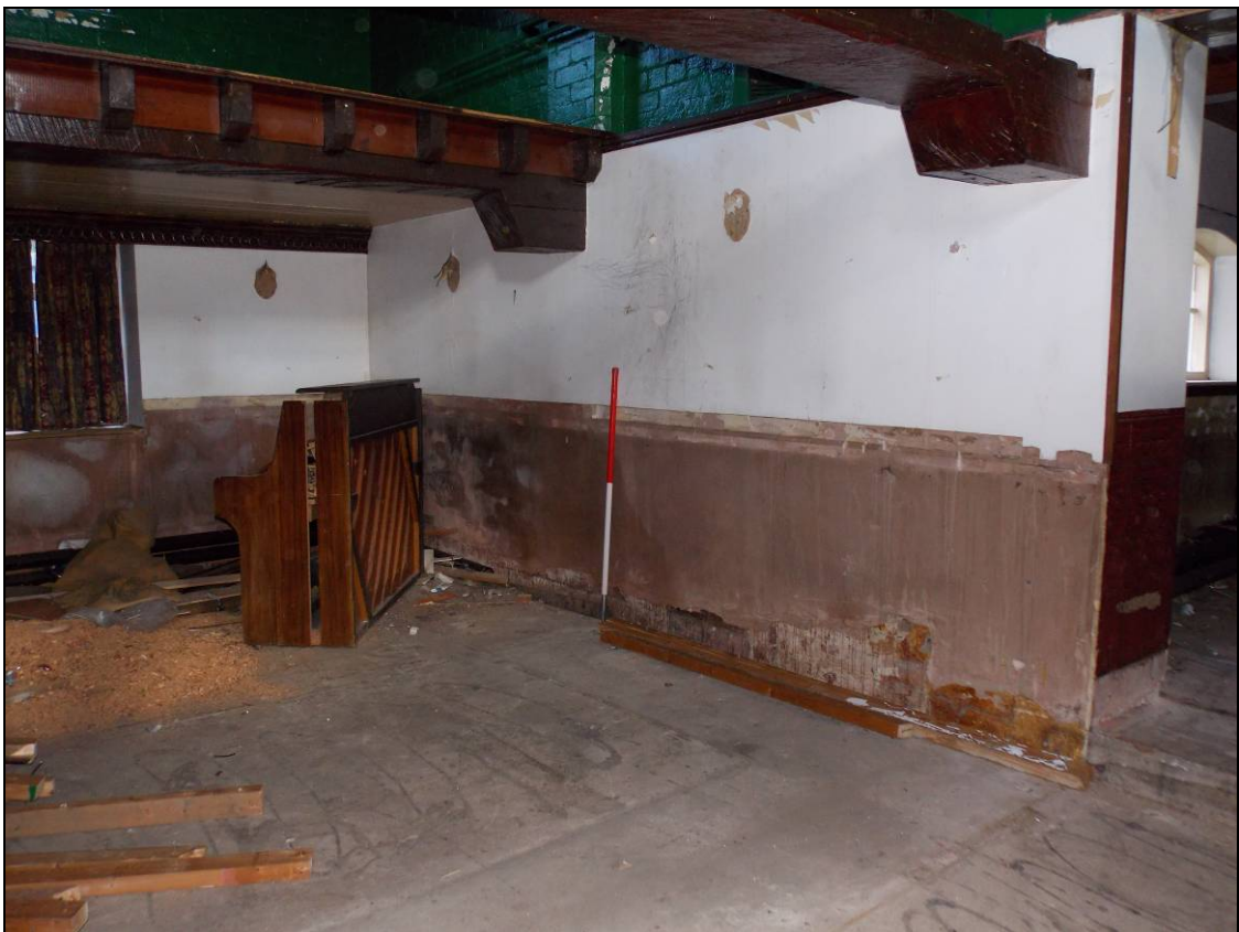
Figure 106: North wall following soft-stripping (scale 1m).
