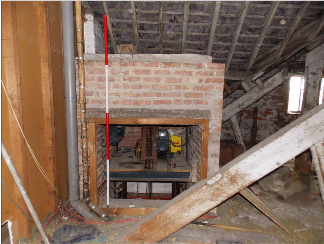
Figure 73: Upper section of the inserted lift, looking east (scale 2m).
