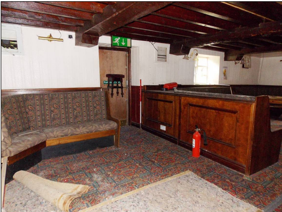
Figure 27: Ground floor of Building A, looking south-west (scale 1m).
