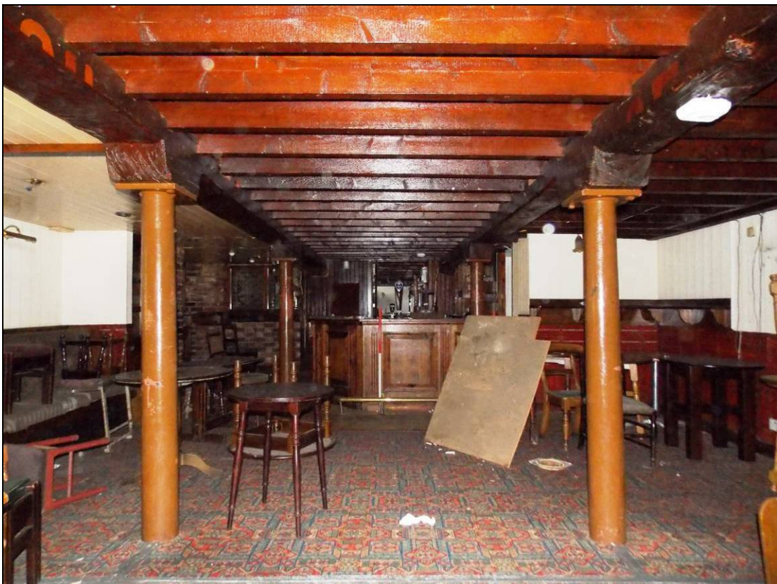
Figure 33: Ground floor, looking north (scale 1m).
