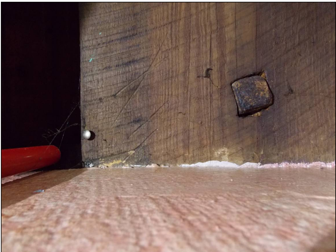
Figure 141: Detail of carpenter's marks within the southern tie-beam.
