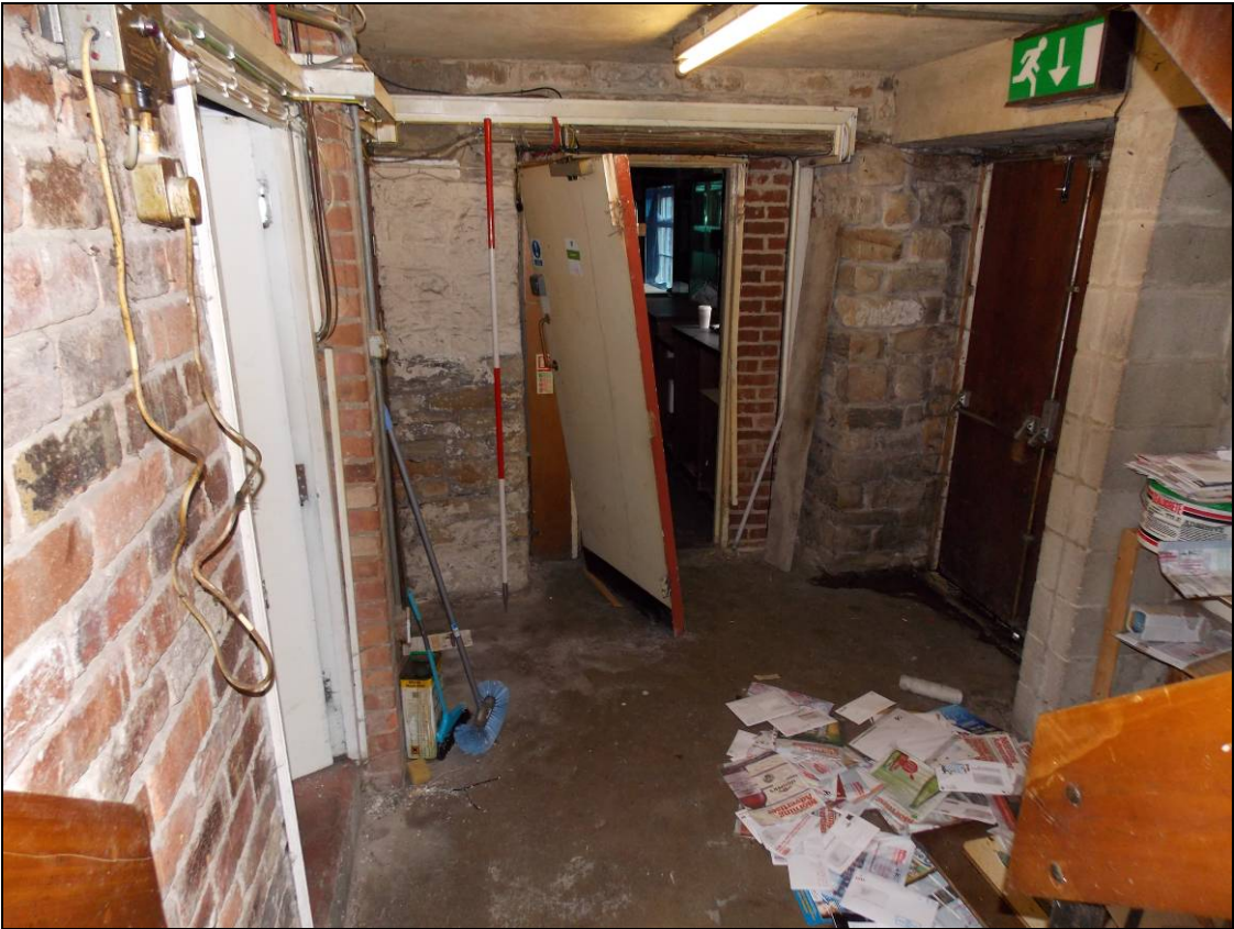
Figure 20: Basement's lobby with inserted doorways within the east and north walls, looking north (scale 2m).
