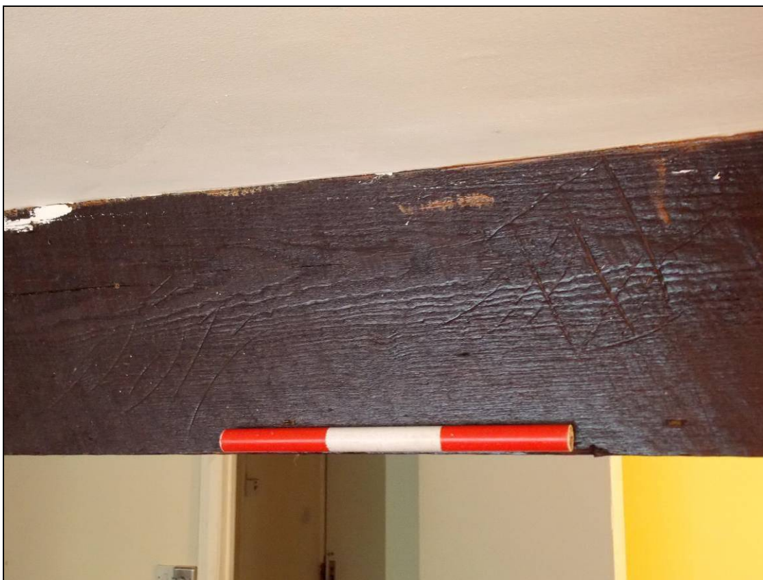
Figure 70: Detail of carpenter's marks, looking east (scale 300mm).
