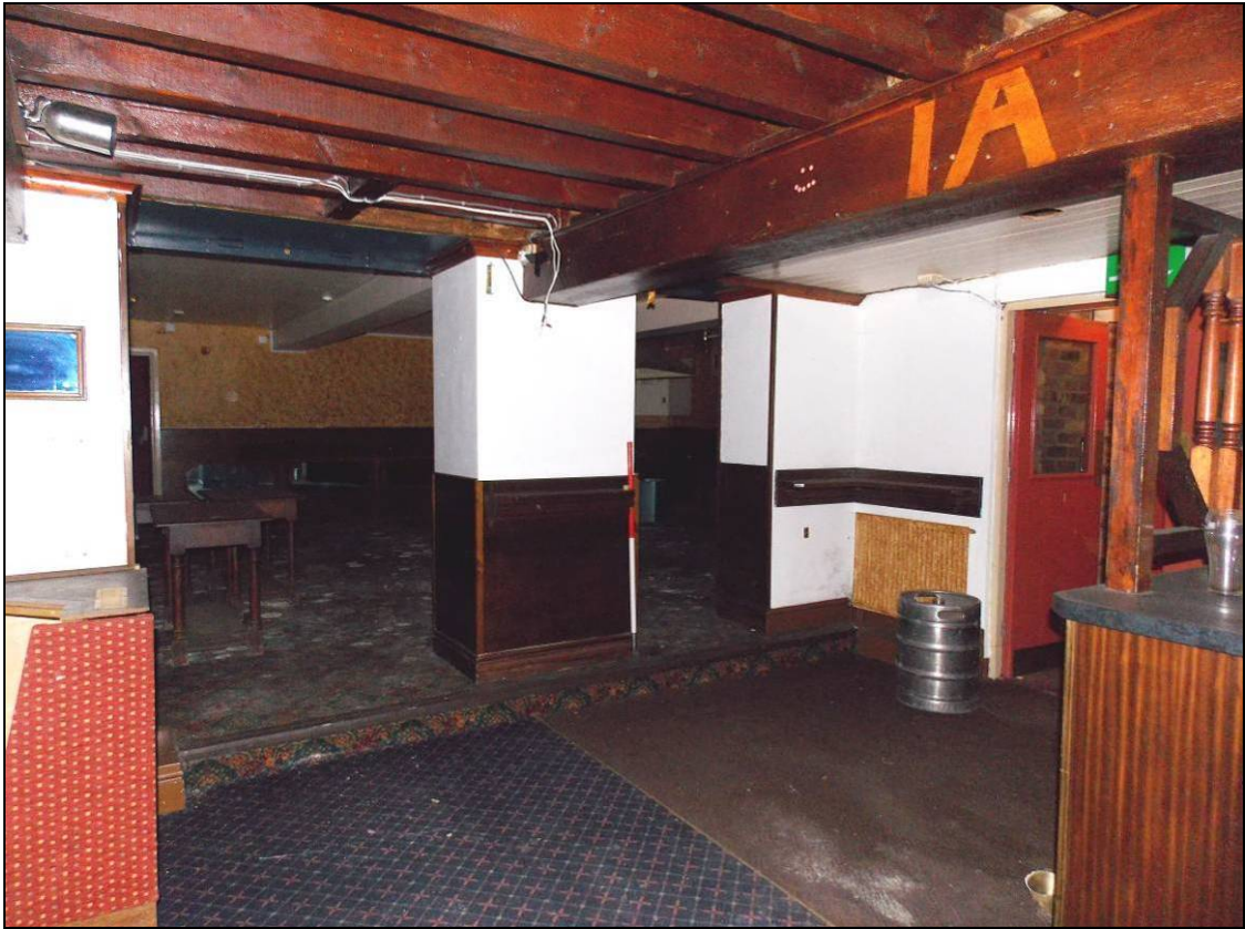
Figure 96: Inserted doorways within the north wall (scale 1m).
