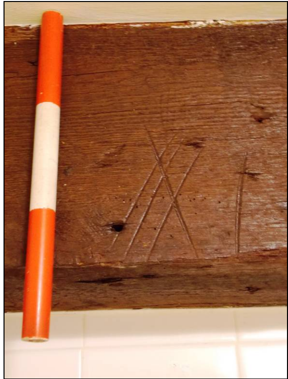
Figure 68: Detail of carpenter's marks, looking east (scale 300mm).
