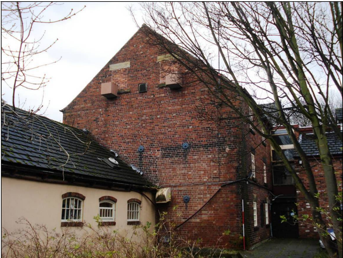
Figure 90: North elevation of Building B (scale 2m).
