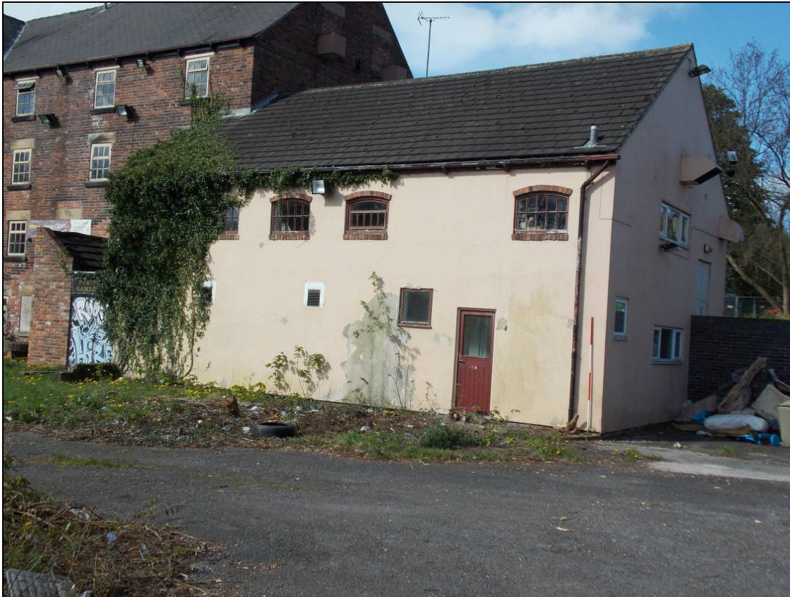
Figure 147: East elevation of Building C (scale 2m).
