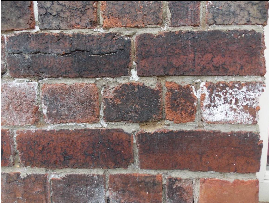
Figure 93: Detail of re-pointed brickwork.
