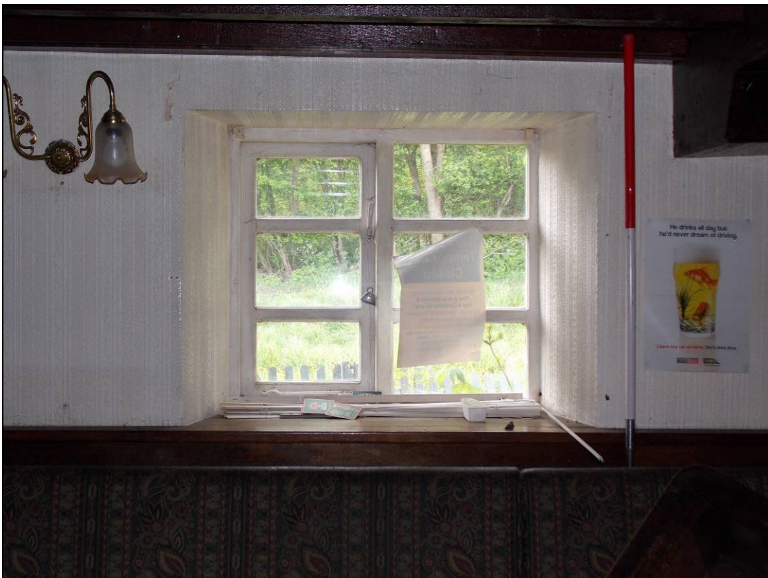
Figure 29: Detail of window within the south wall (scale 1m).
