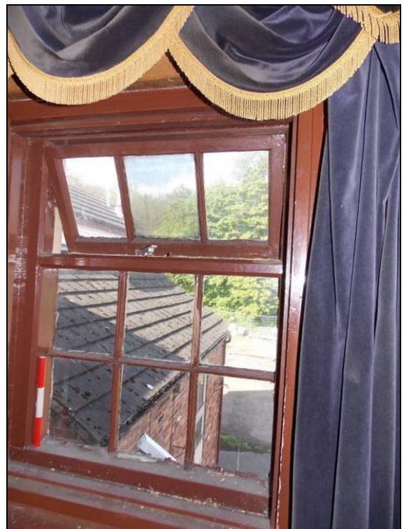
Figure 139: Detail of window, looking west (scale 300mm).
