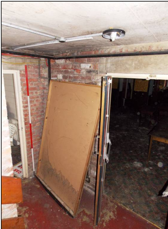
Figure 154: Doorway to the basement, looking south-east (scale 2m).
