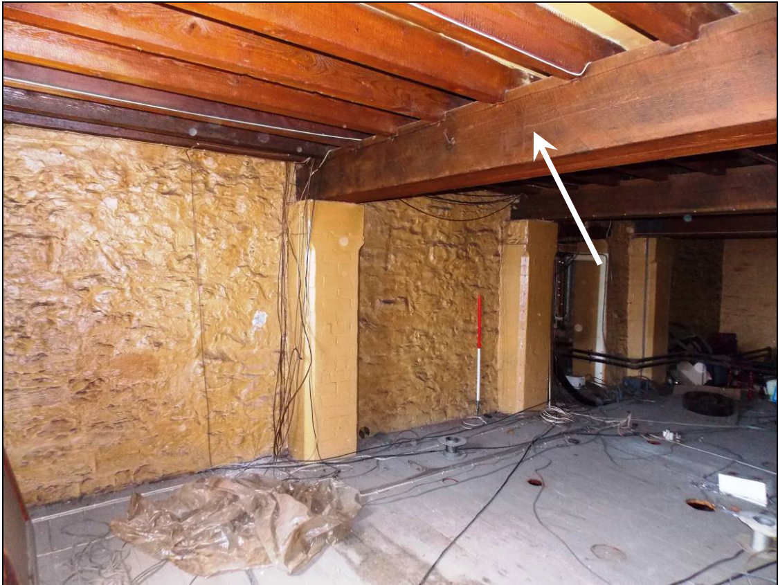
Figure 111: First floor with beam containing carpenter's marks (arrow) (scale 1m).
