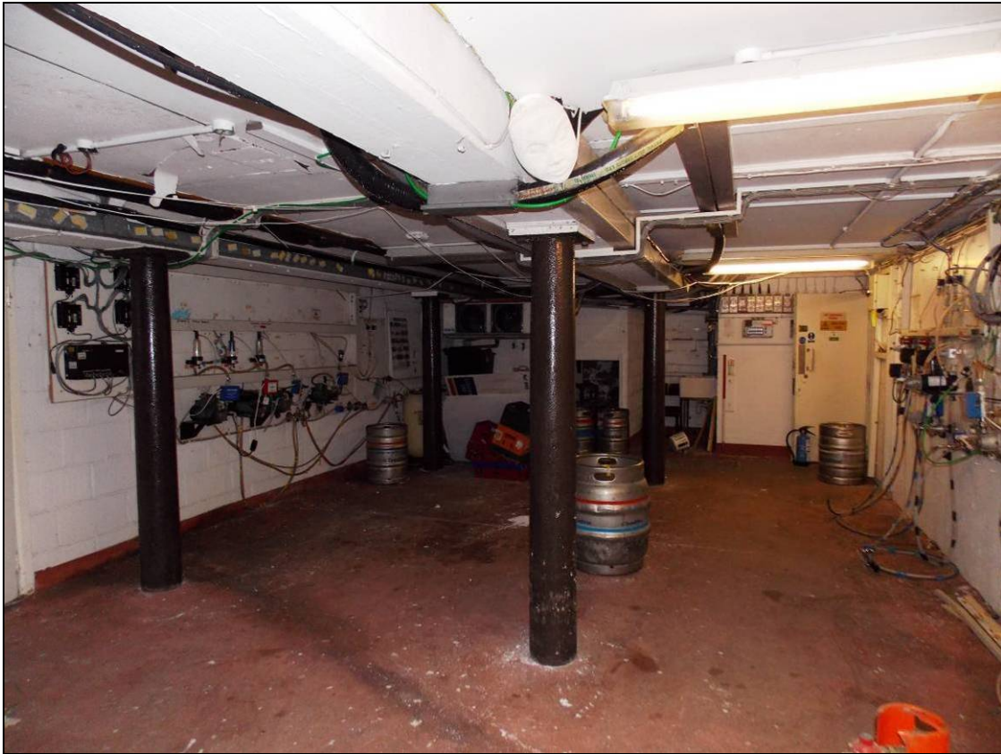
Figure 22: General view of the beer cellar, looking north (scale 1m).
