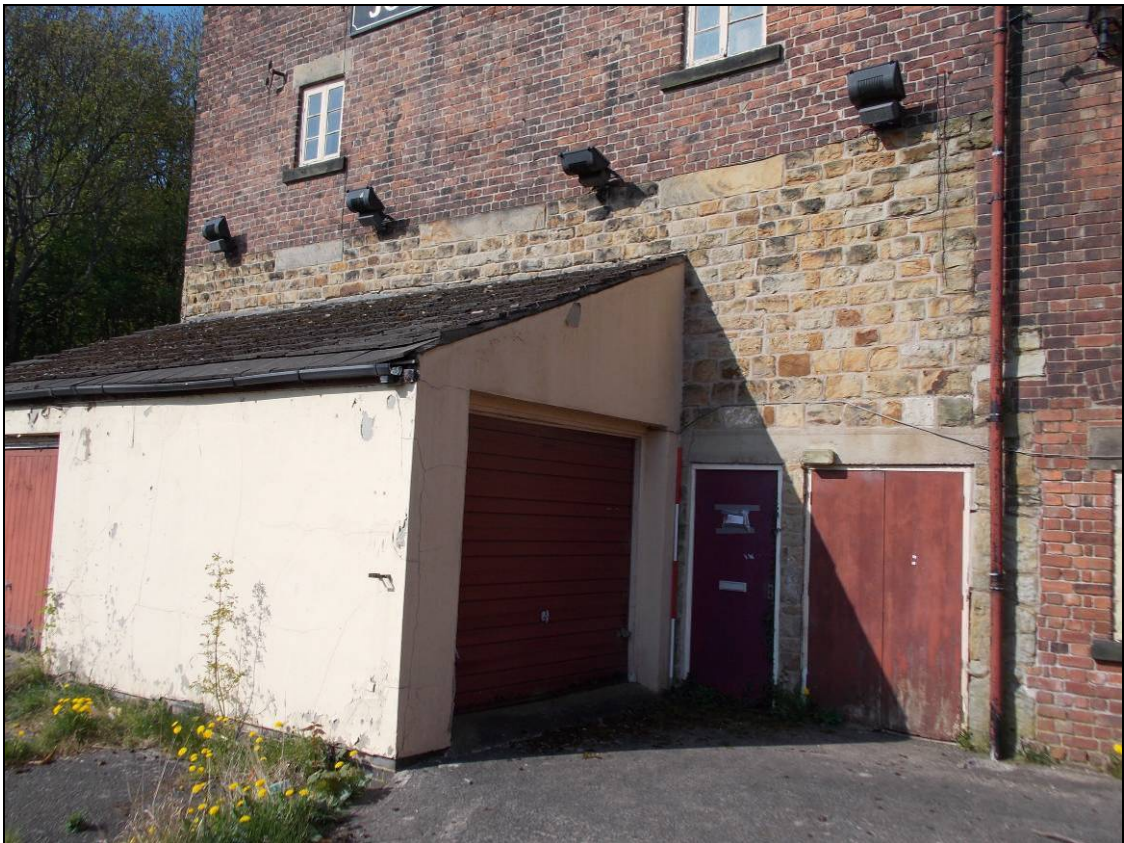
Figure 10: Detail of blocked-up window openings, looking south-west (scale 2m).
