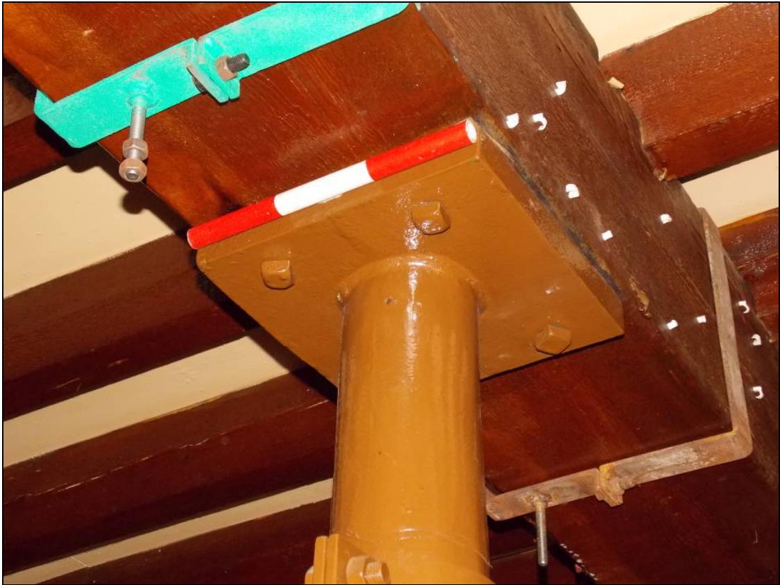
Figure 129: Detail of column capital and bolted brace (scale 300mm).
