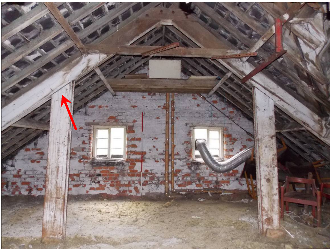
Figure 74: Western truss III with carpenter's assembly marks (arrow) (scale 2m).
