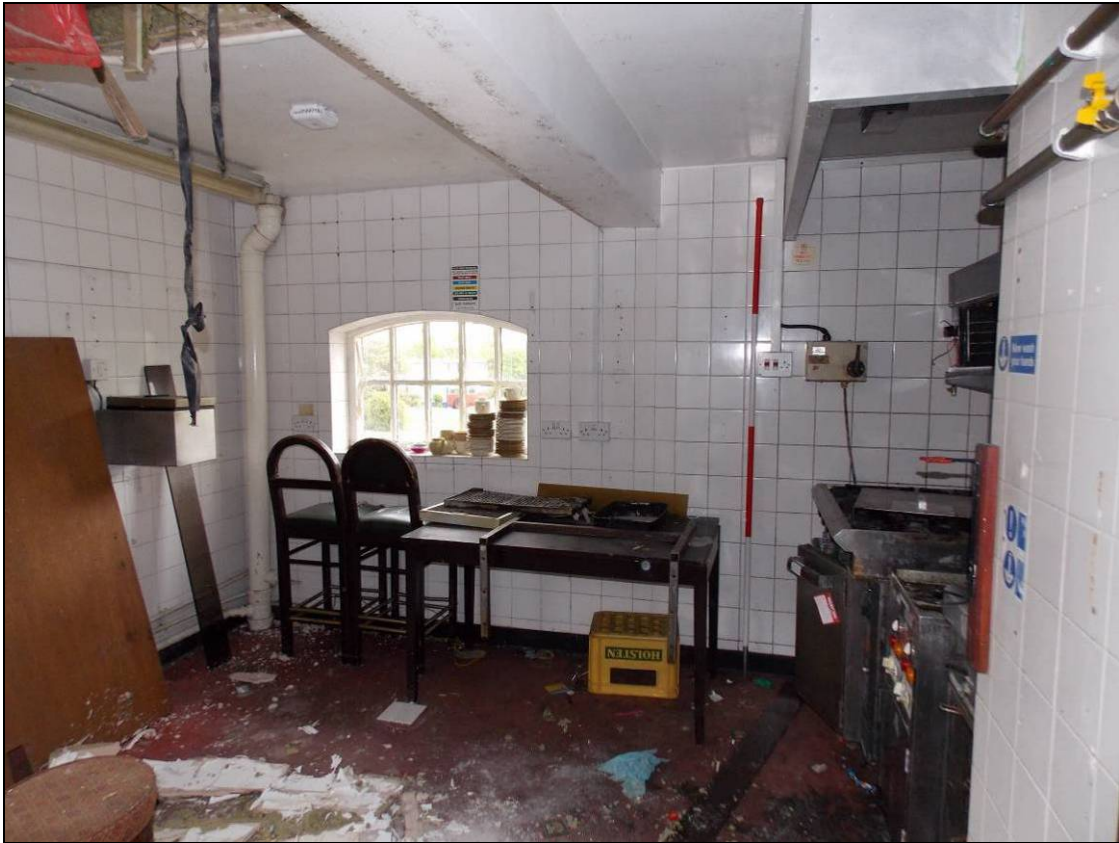
Figure 161: Kitchen, looking east (scale 2m).
