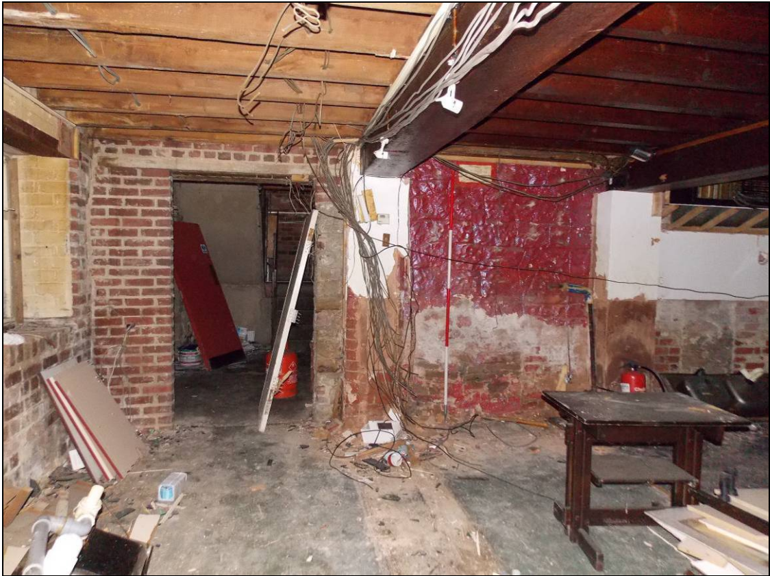
Figure 98: South wall after soft-stripping (scale 2m).
