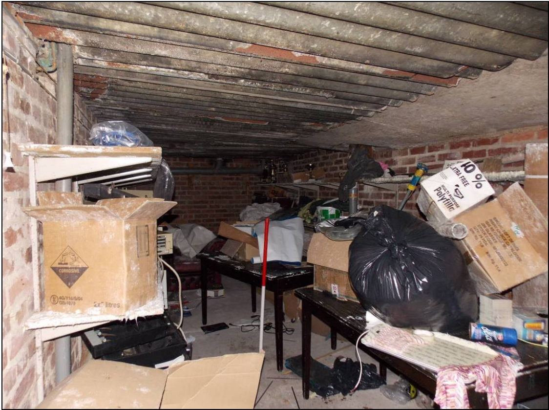
Figure 165: General view of the basement, looking west (scale 1m).
