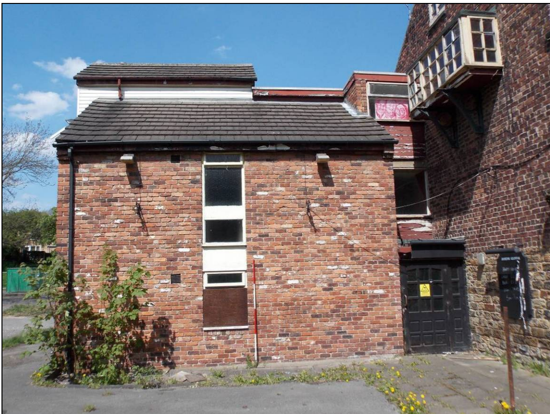
Figure 163: South elevation of Building D (scale 2m).
