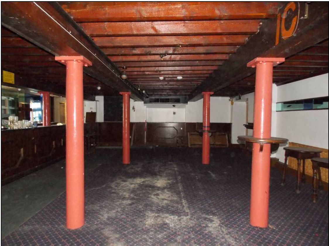
Figure 97: General view of the basement, looking south (scale 1m).
