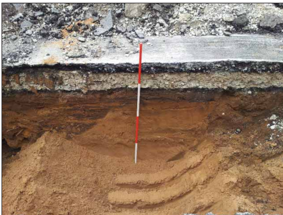
Figure 3. Original excavation depth of trench 1. Note the cut for a water pipe on the left, and the smaller cut for an unknown service trench on the right. Scale 2m.
