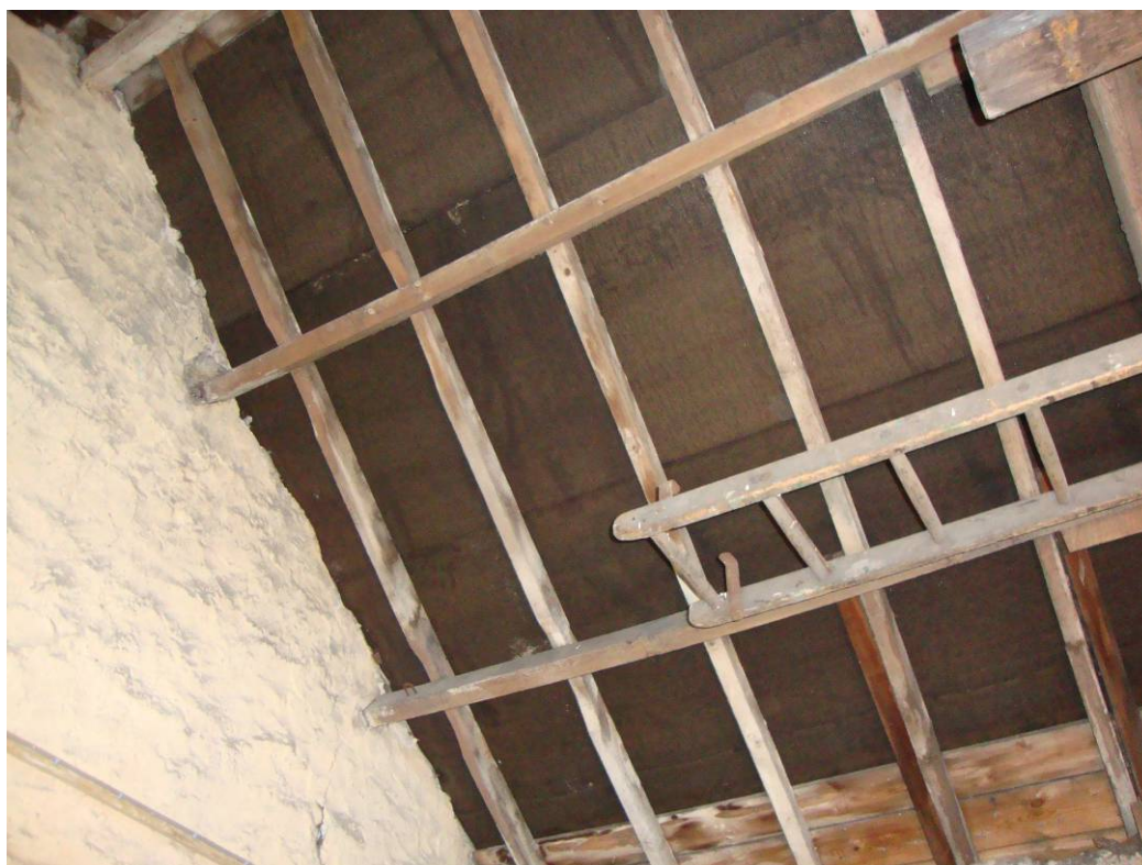
Figure 6. Internal view of the former farm building showing modern re-roofing.
