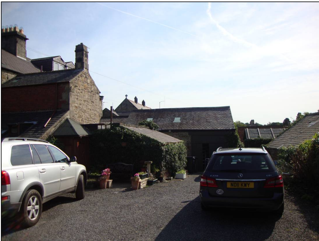
Figure 2. General view of the west elevation of the former farm building looking east.
