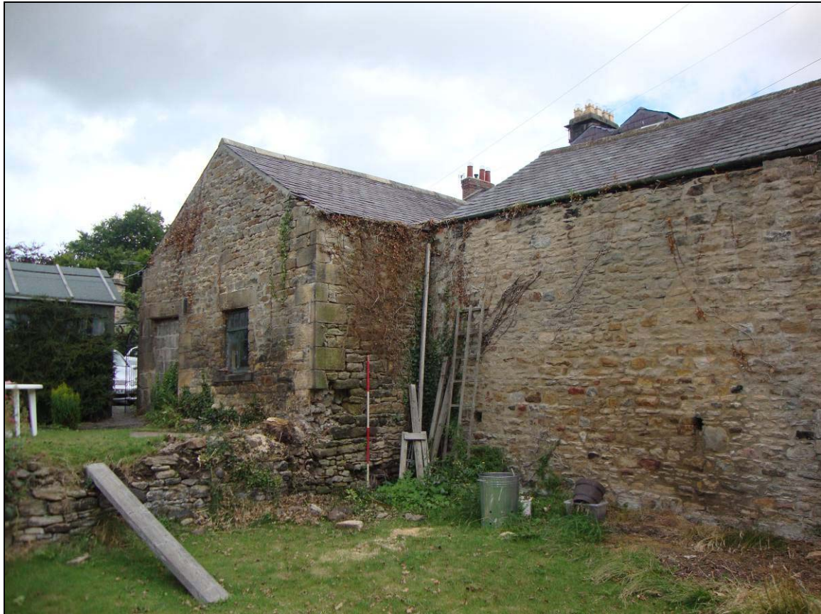
Figure 3: East elevation of Building A, with adjoining building (scale=2m).
