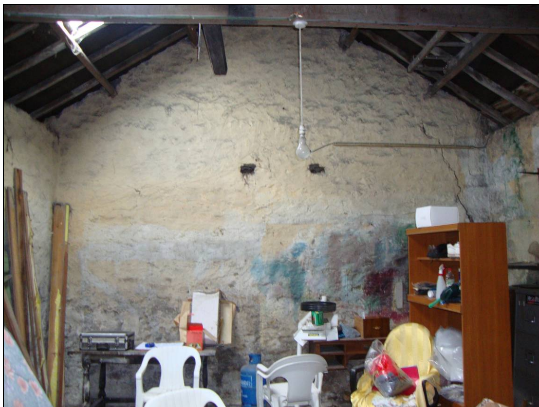
Figure 7: North wall of Room A1, Building A.
