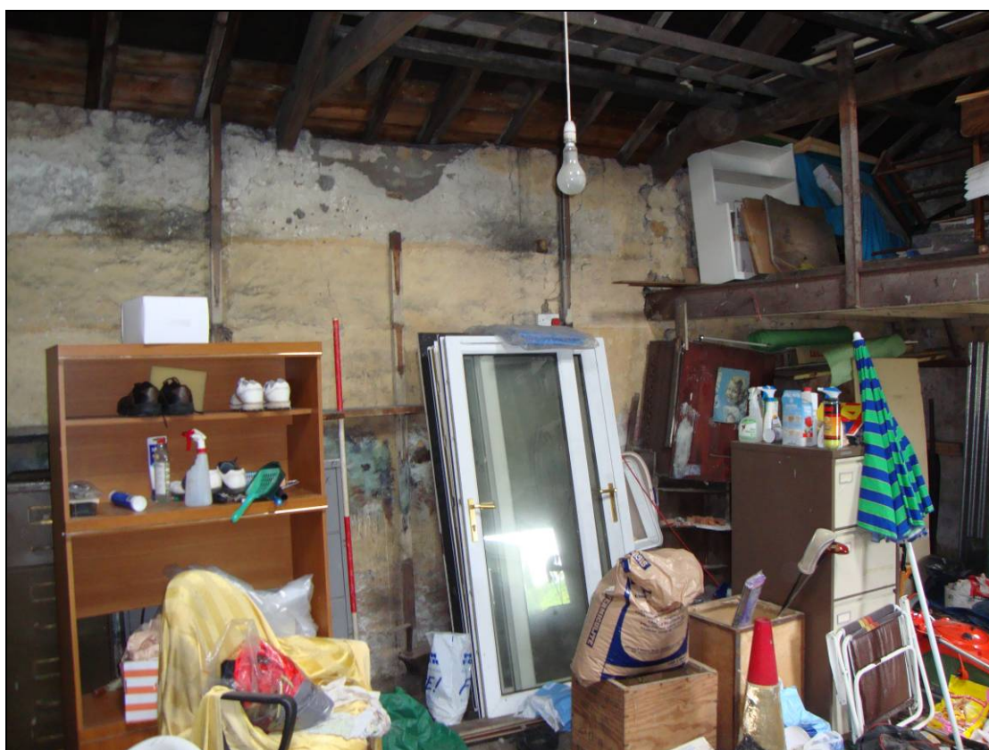
Figure 9: East wall of Room A1, Building A. (scale=2m).
