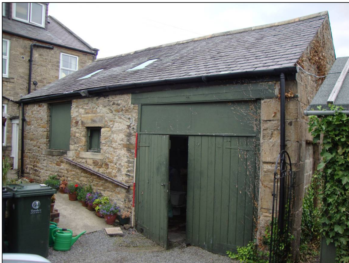
Figure 4: West elevation of Building A (scale=2m).
