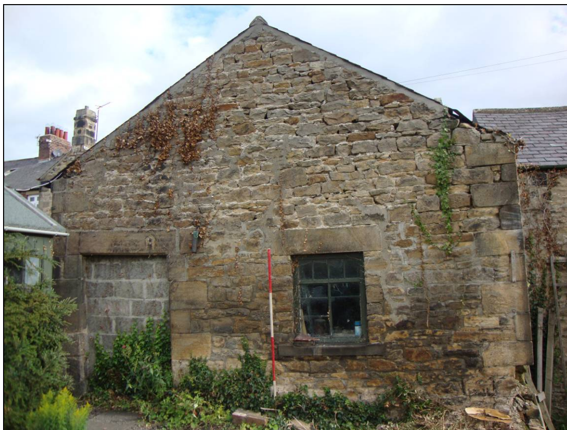
Figure 6: South elevation of Building A (scale=2m).
