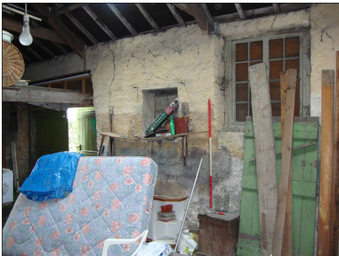
Figure 8: West wall of Room A1, Building A. (scale=2m).
