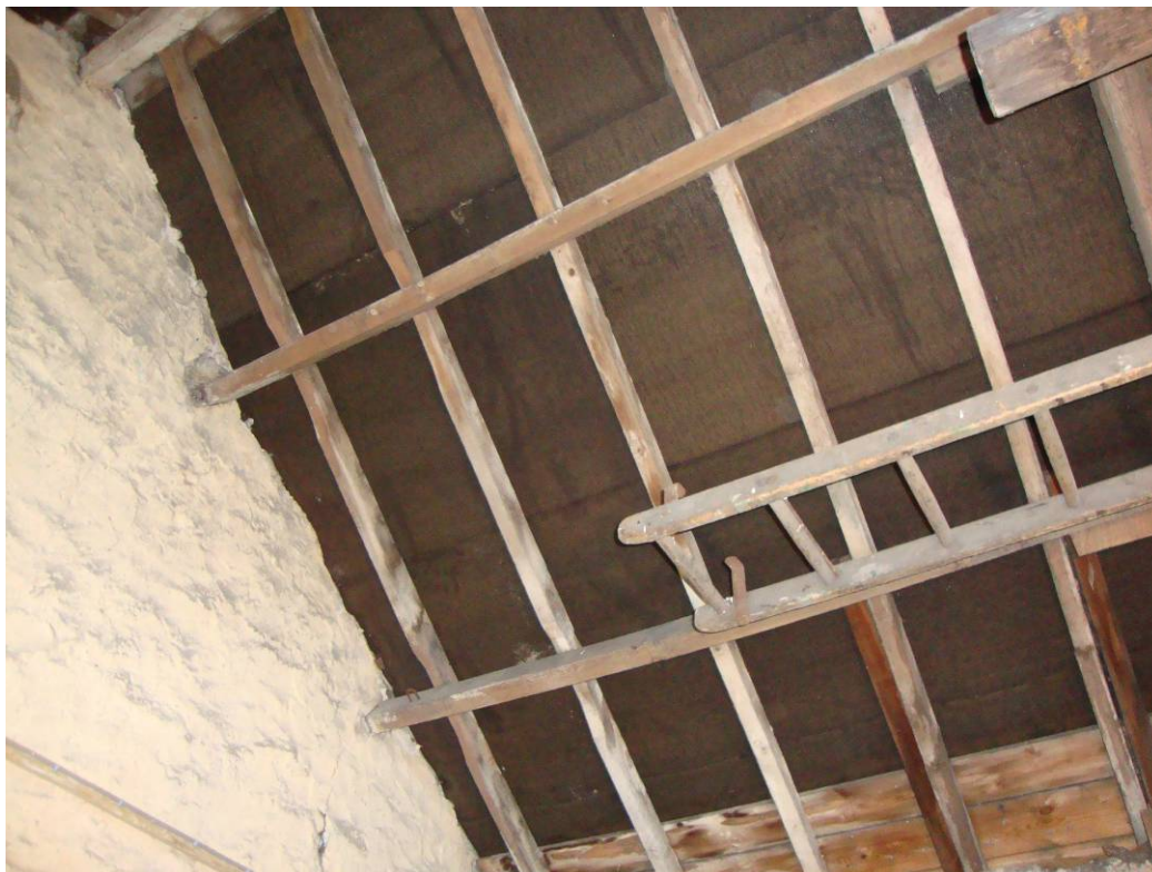
Figure 12: Internal view of the former farm building showing modern re-roofing.
