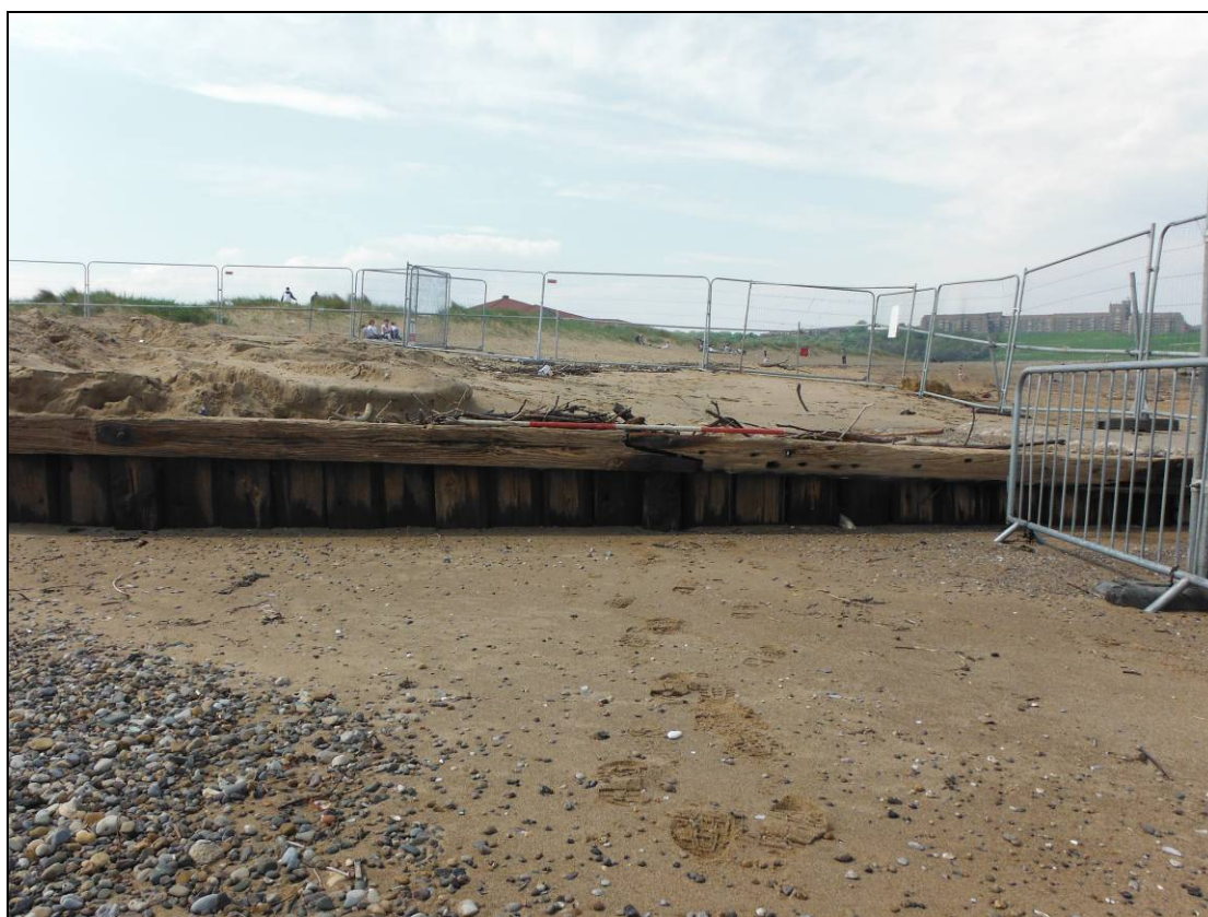
Figure 3. North facing view of seaplane ramp
