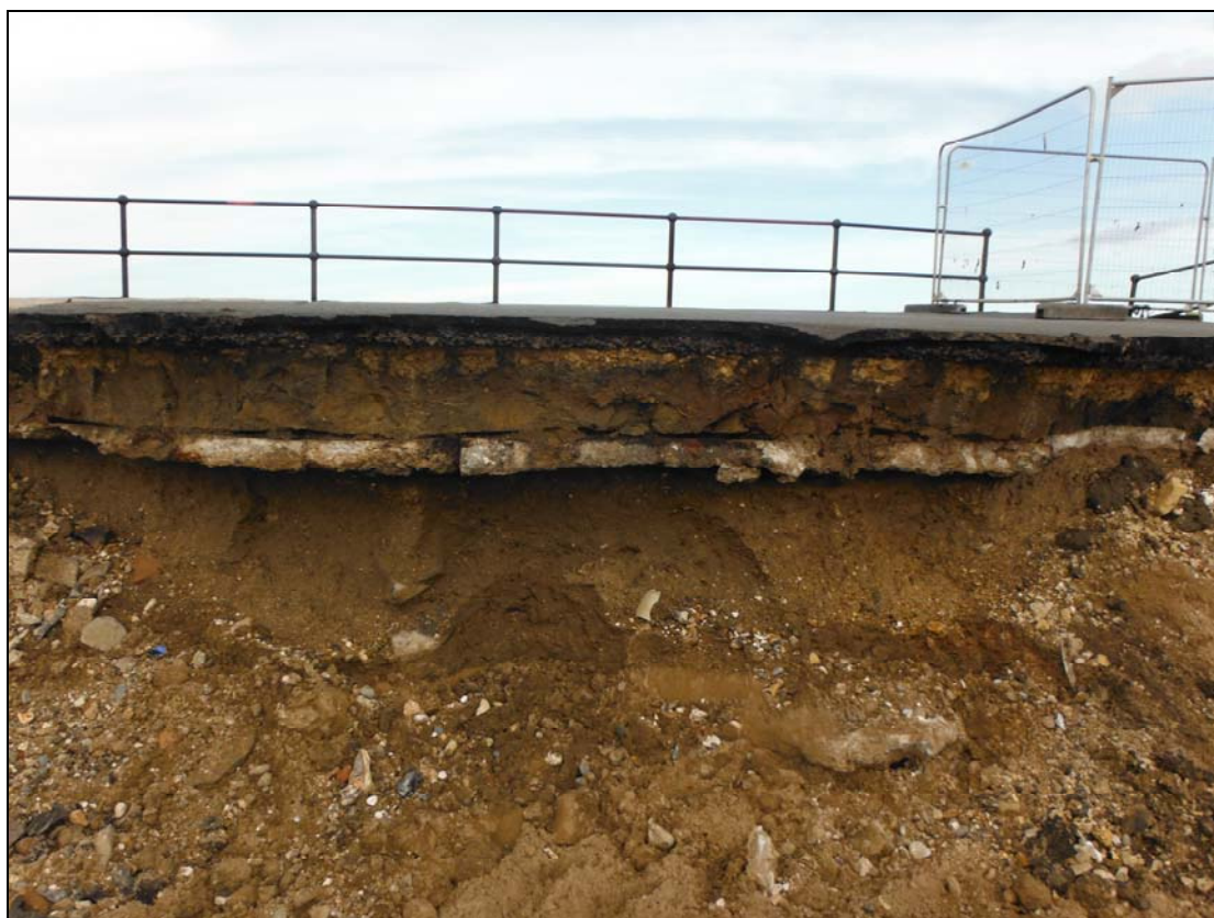
Figure 16. Image showing composition of old sea wall.
