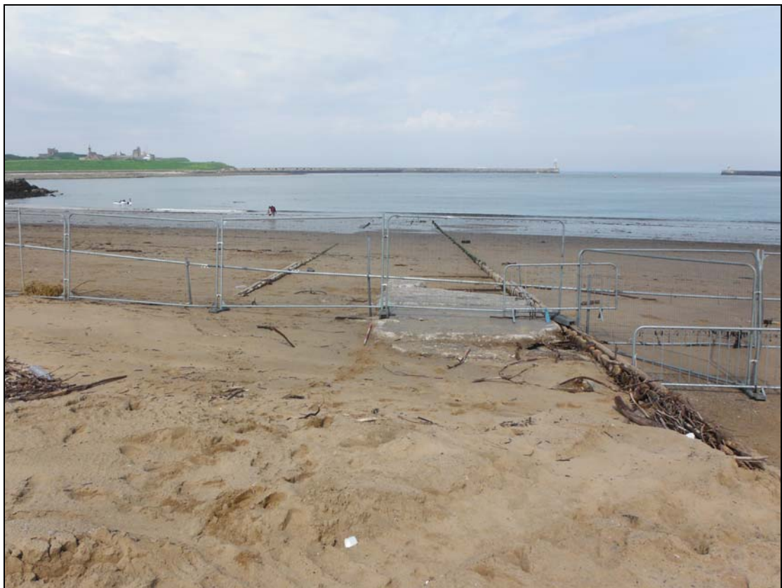
Figure 5. Eastern view of seaplane ramp, showing inset concrete surface.
