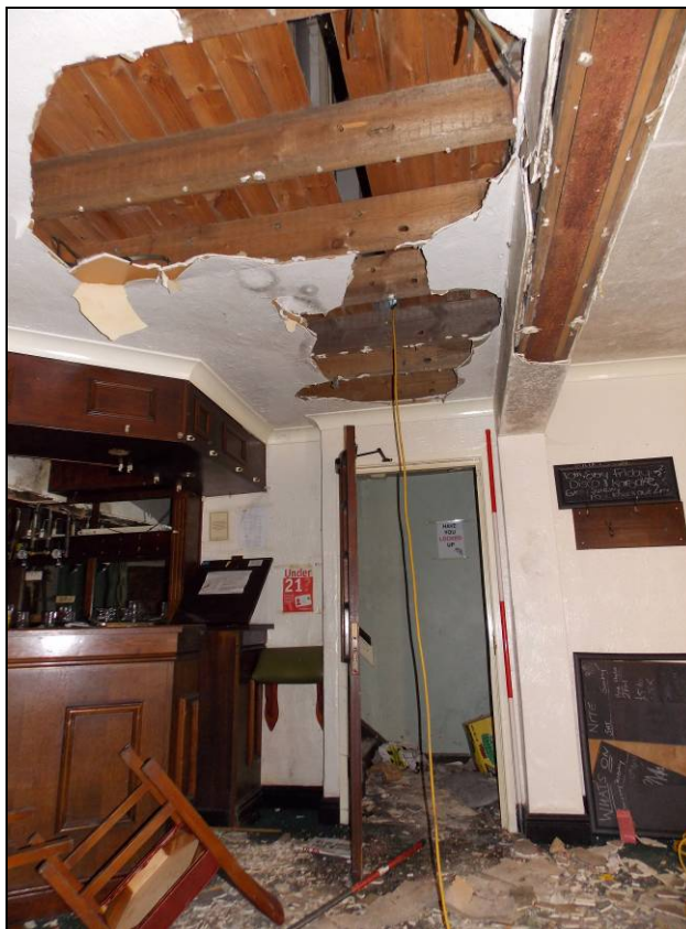
Plate 12: Southern room, looking north (scale 2m)
