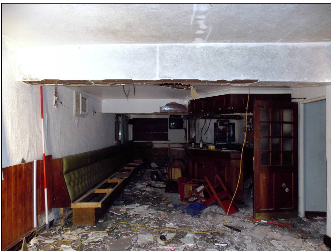
Plate 11: Southern room of the ground floor, looking west (scale 2m)
