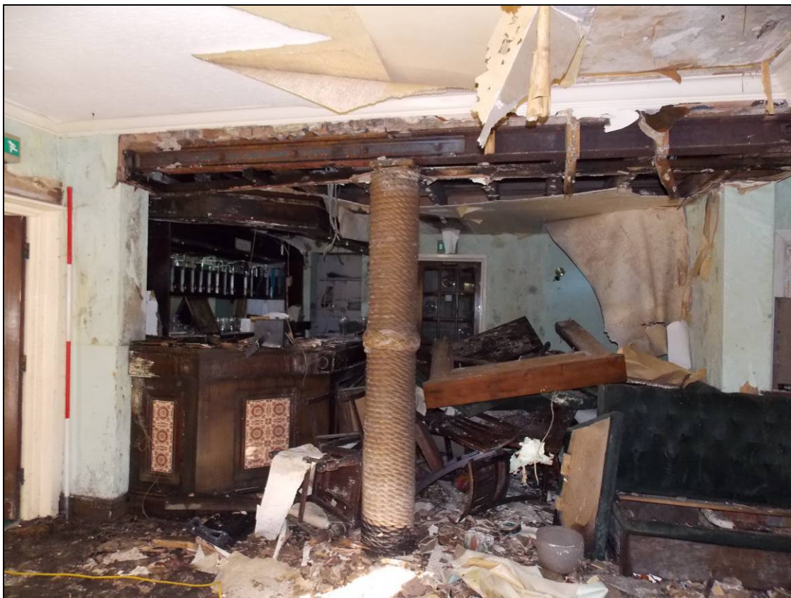
Plate 14: Northern room of the ground floor, looking west (scale 2m)
