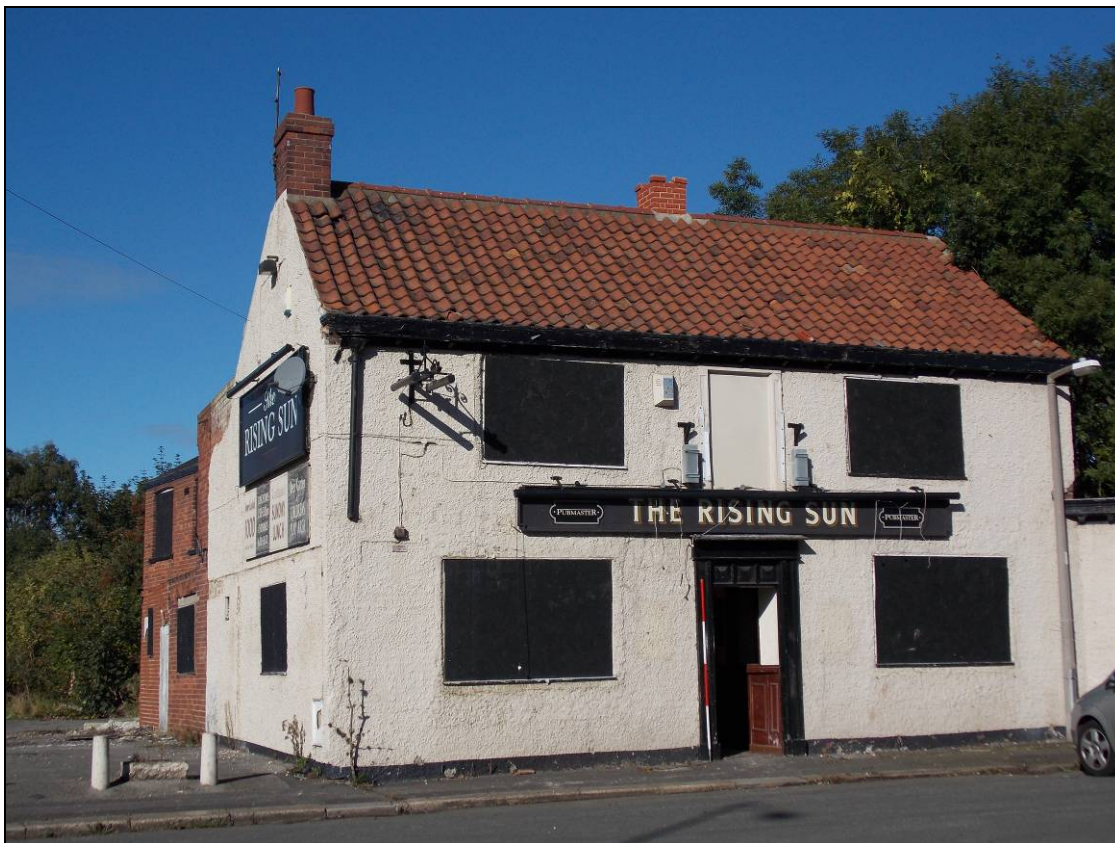
Plate 3: East elevation of the main range (scale 2m)
