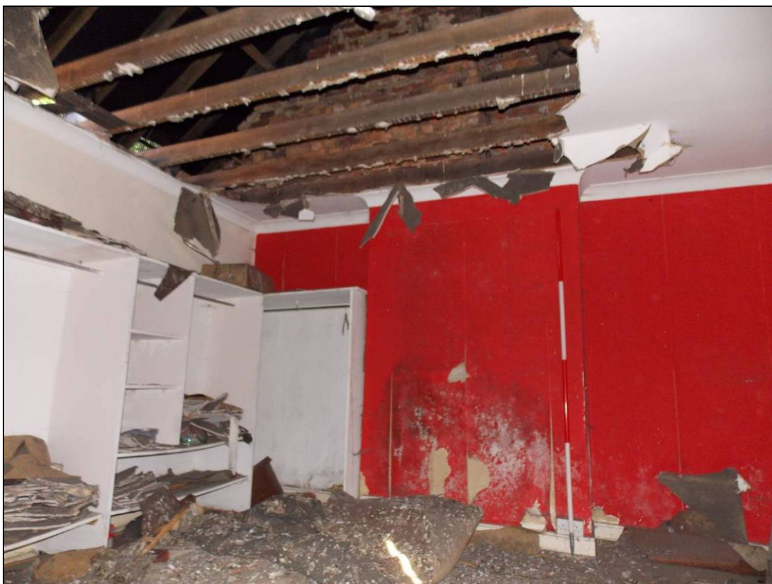
Plate 20: Northern room of the first floor, looking north (scale 2m)
