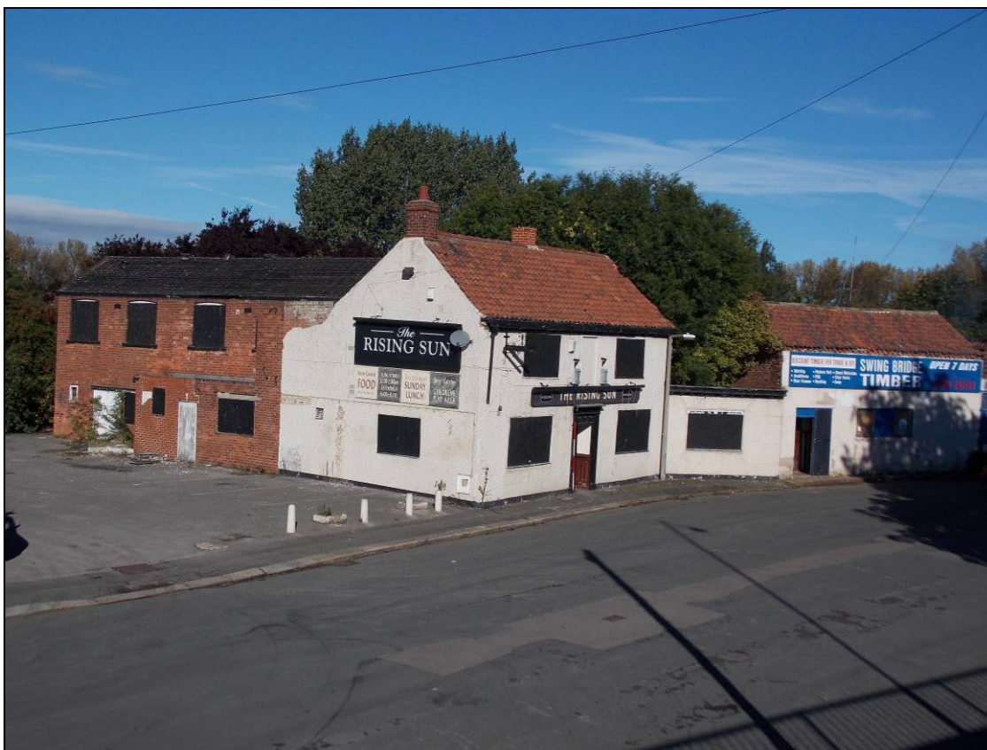
Plate 1: General view of the Rising Sun, looking north-west
