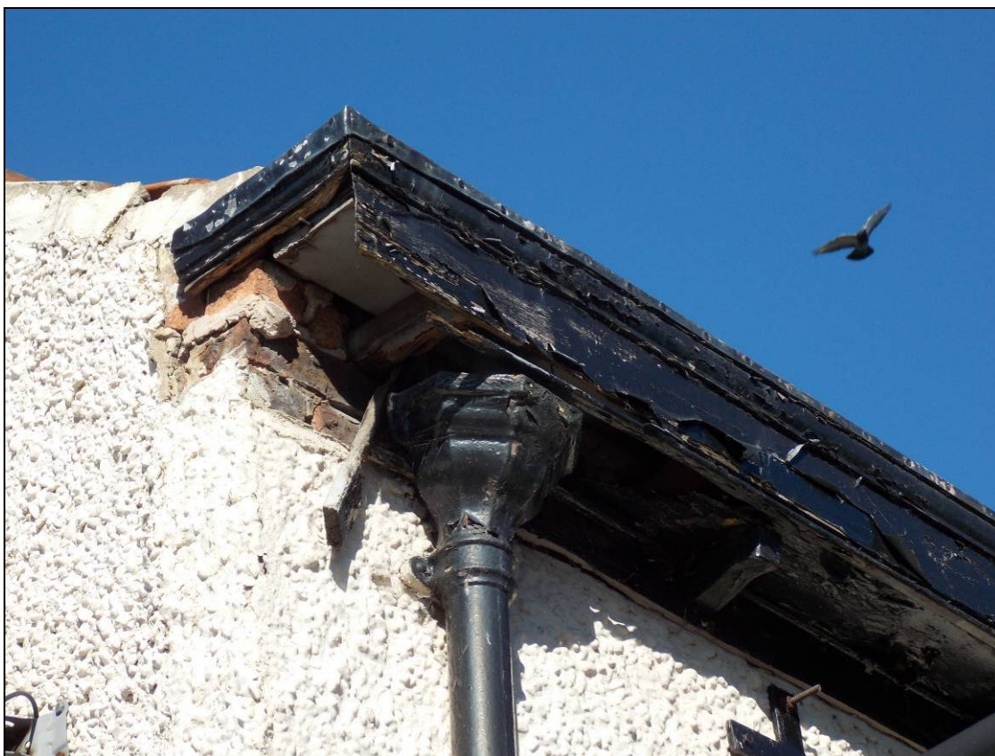
Plate 4: Detail of exposed brickwork beneath the gutter, looking north-west
