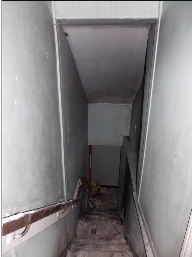
Plate 17: Staircase to the first floor, looking east (scale 2m)
