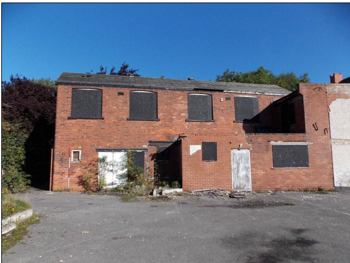
Plate 7: South elevation of the cross-wing (scale 2m)
