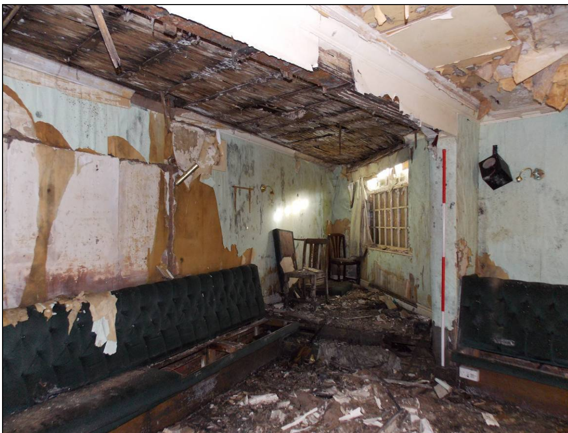
Plate 15: Later north-east extension, looking east (scale 2m)
