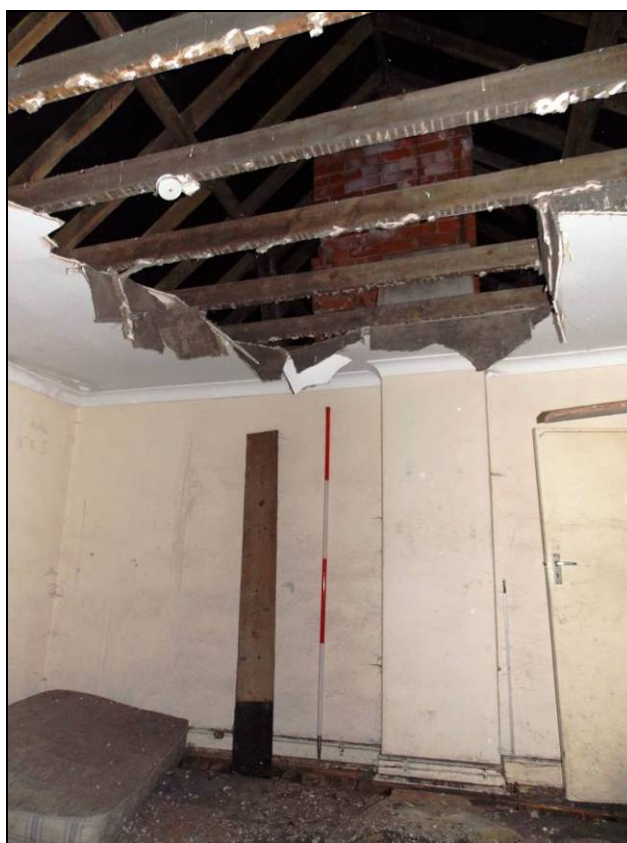
Plate 21: Northern room of the first floor, looking south (scale 2m)
