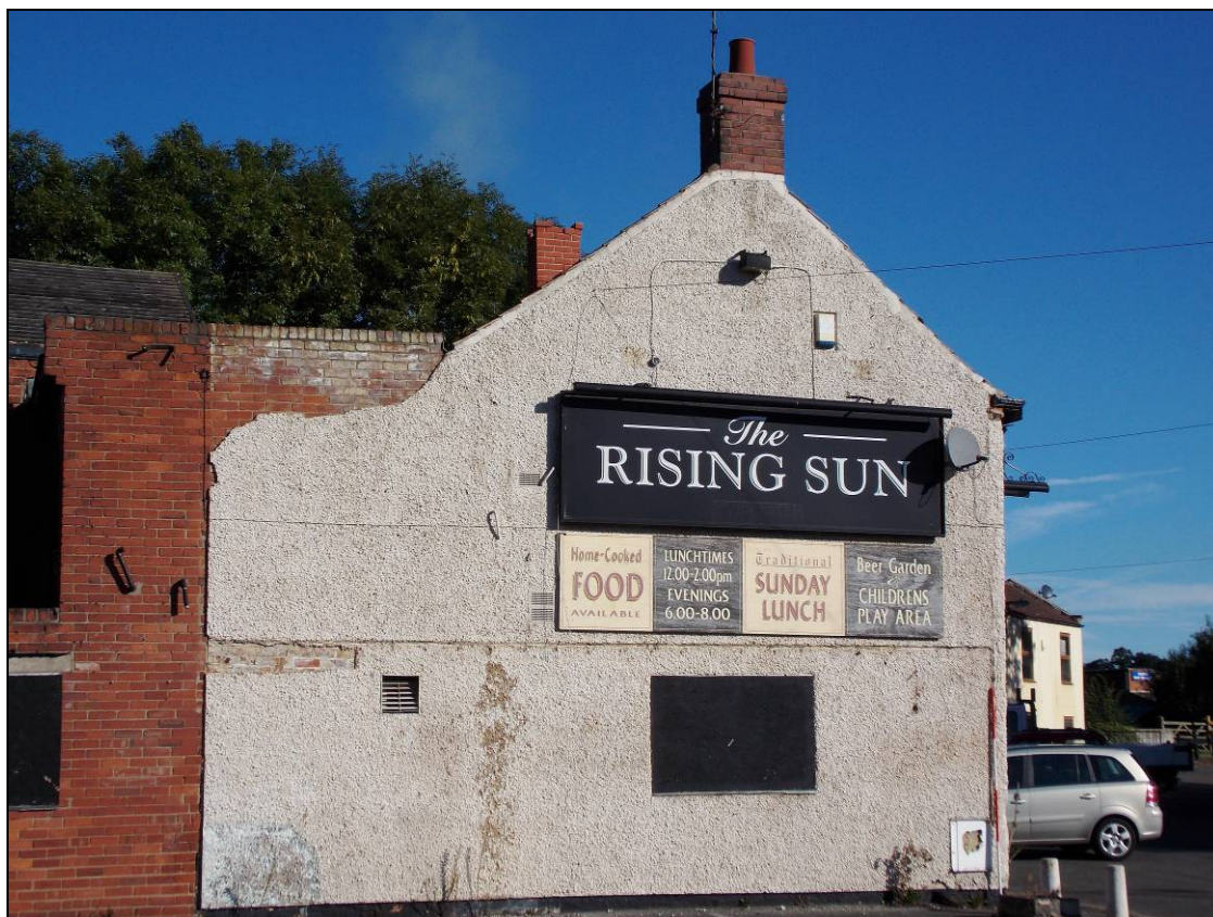
Plate 5: South elevation of the main range (scale 2m)
