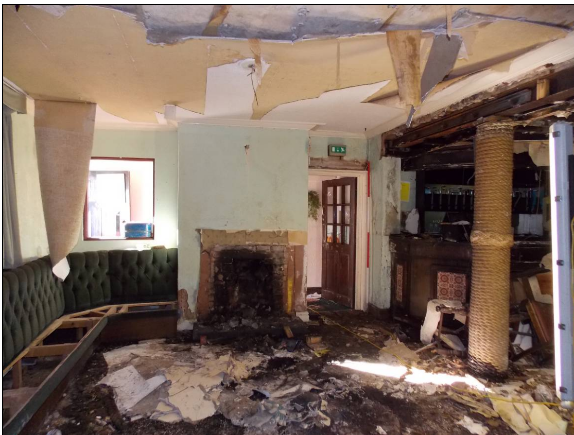
Plate 13: Northern room of the ground floor, looking south (scale 2m)
