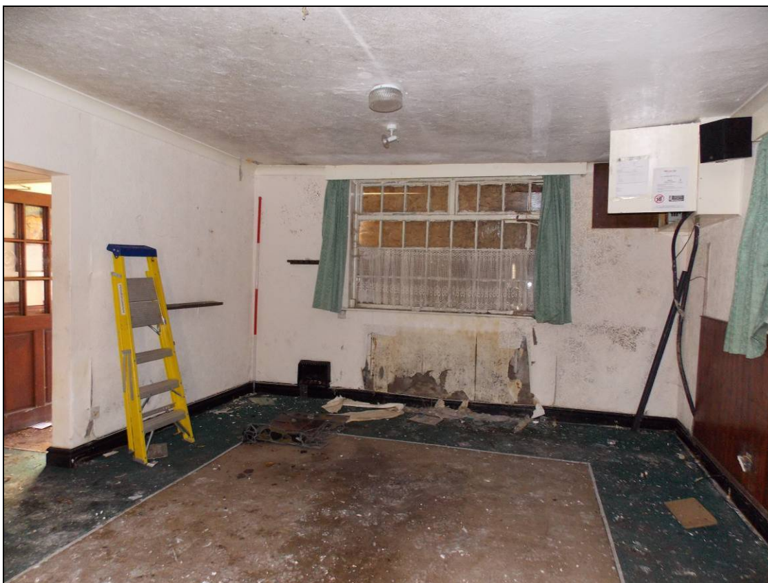
Plate 10: Southern room of the ground floor, looking east (scale 2m)
