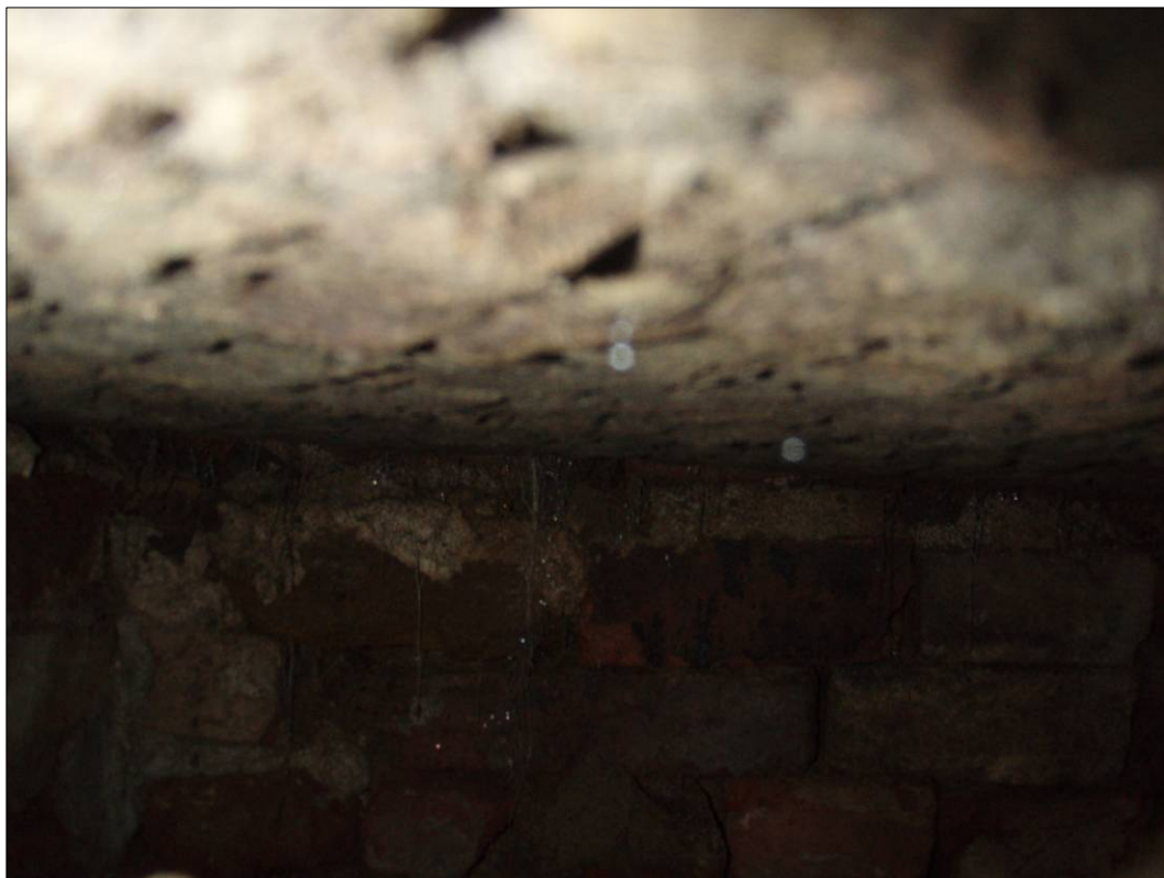
Figure 7: View into the void space within (403) showing brick-built construction, looking north.
