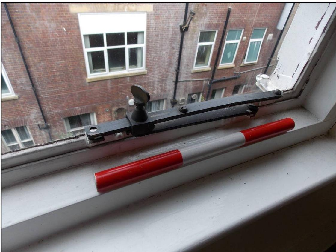
Plate 111: Detail of window sliding stay, looking south-east (scale 300mm).
