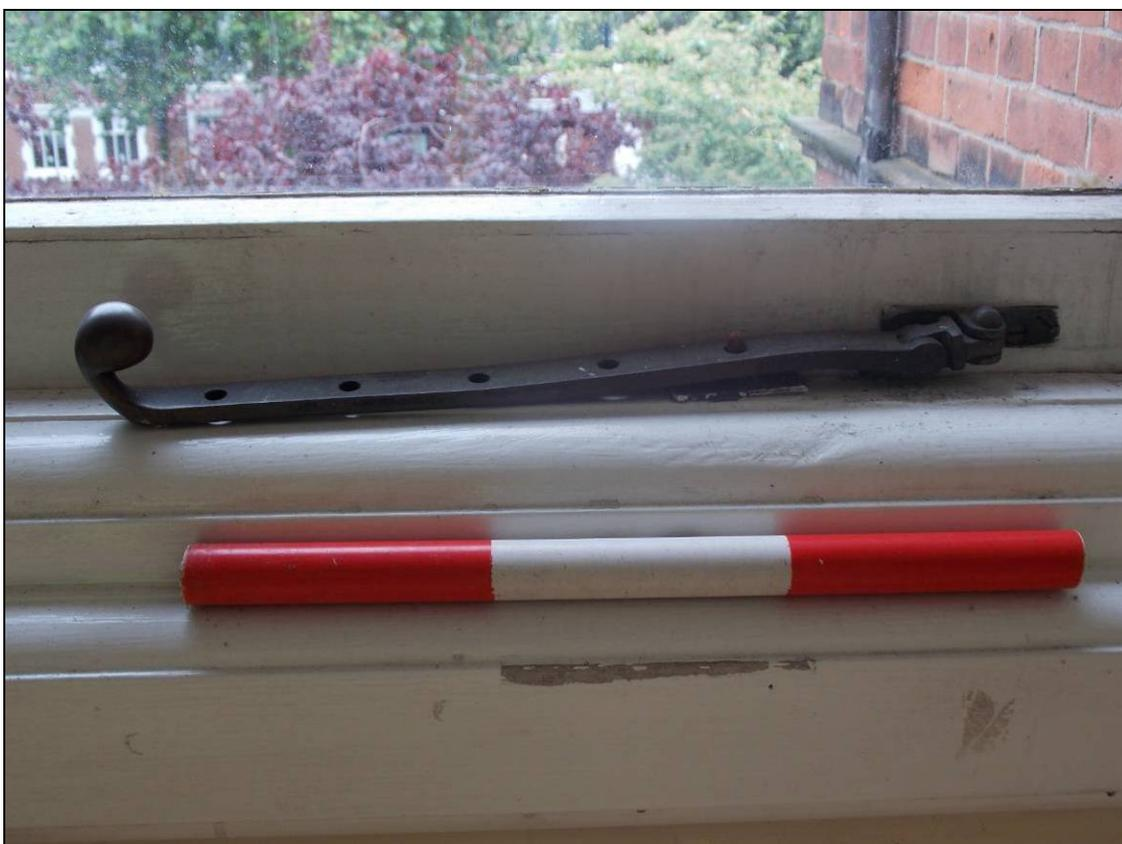
Plate 298: Detail of bronze window stay, looking north (scale 300mm).
