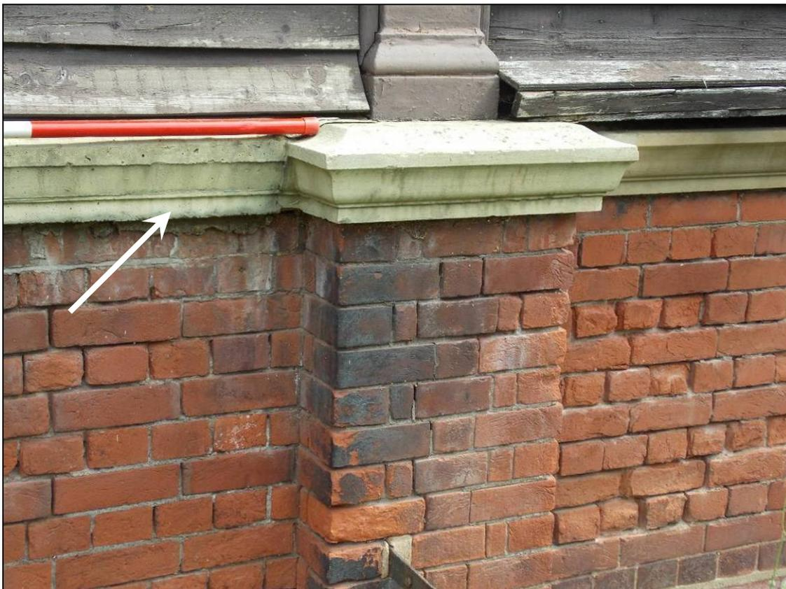
Plate 10: Concrete repair (arrow) of the coping stone, looking north (scale 500mm).
