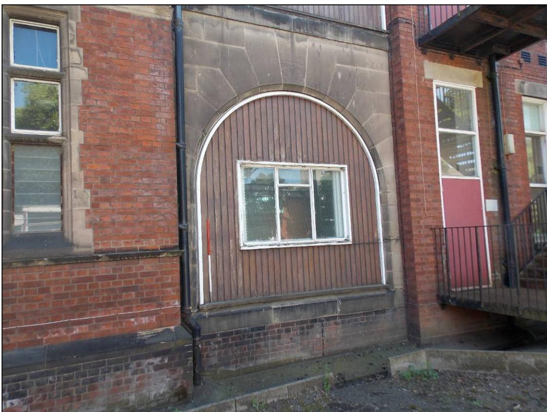
Plate 54: Semi-circular arched opening with stepped arch *voussoirs*, looking south-east (scale 1m).
