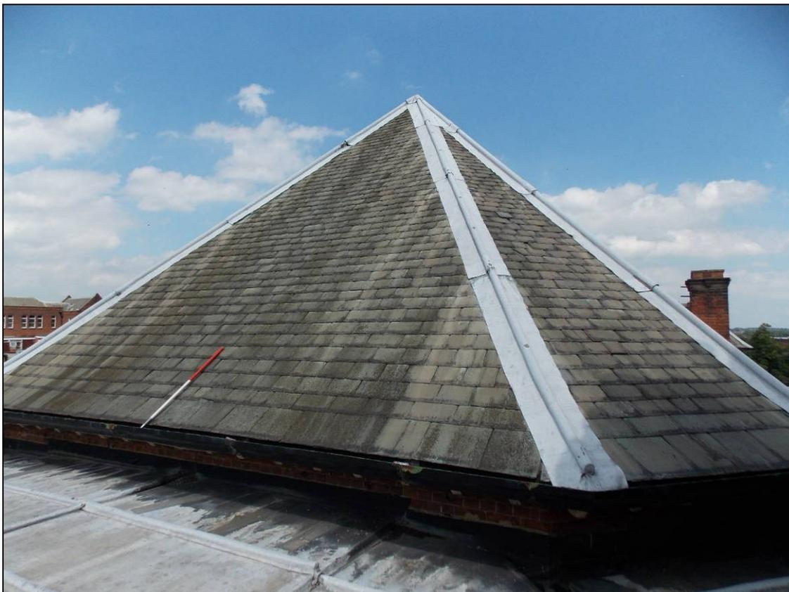
Plate 192: Detailed view of the slated hipped roof between the towers, looking west (scale 1m).
