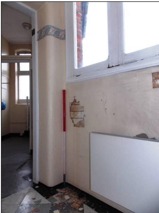
Plate 301: Original glazed brickwork exposed within the lavatory link-way, looking east (scale 1m).
