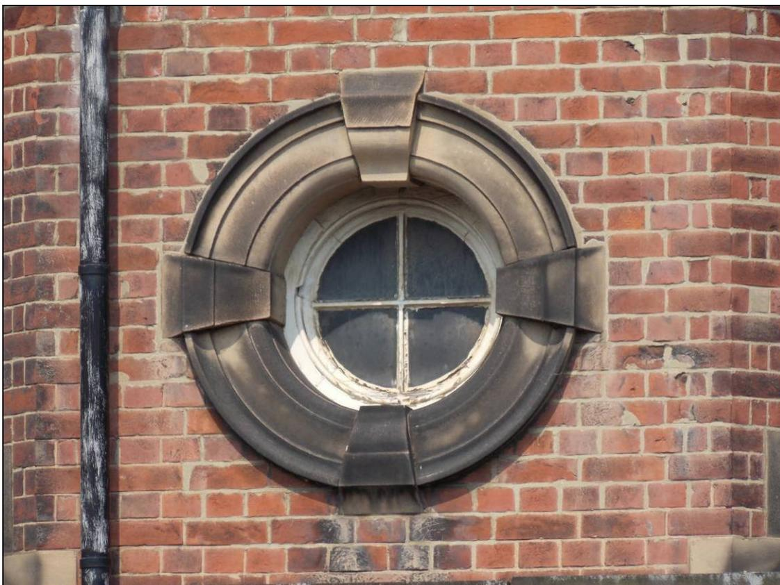
Plate 42: Oculus with moulded architraves and cruciform key-stones, looking north-east.
