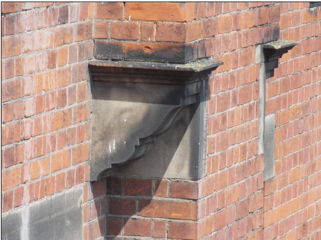
Plate 204: Detail of moulded bracket, looking north-west.
