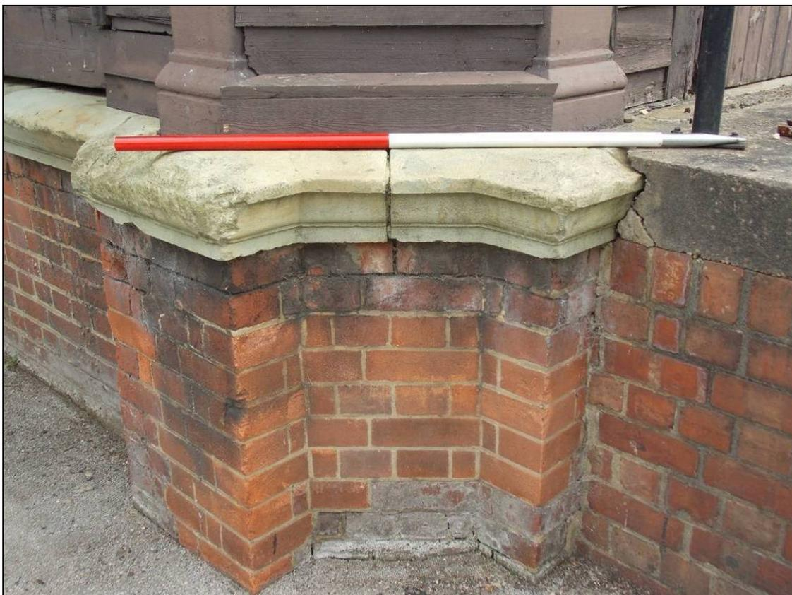
Plate 9: Detail of angled moulded coping stone, looking north-east (scale 1m).
