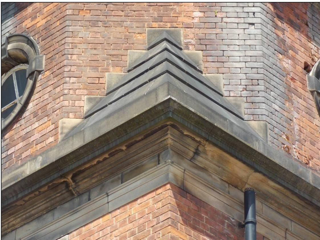
Plate 195: Detail of masonry mitre joint of the string-course, looking north-west.
