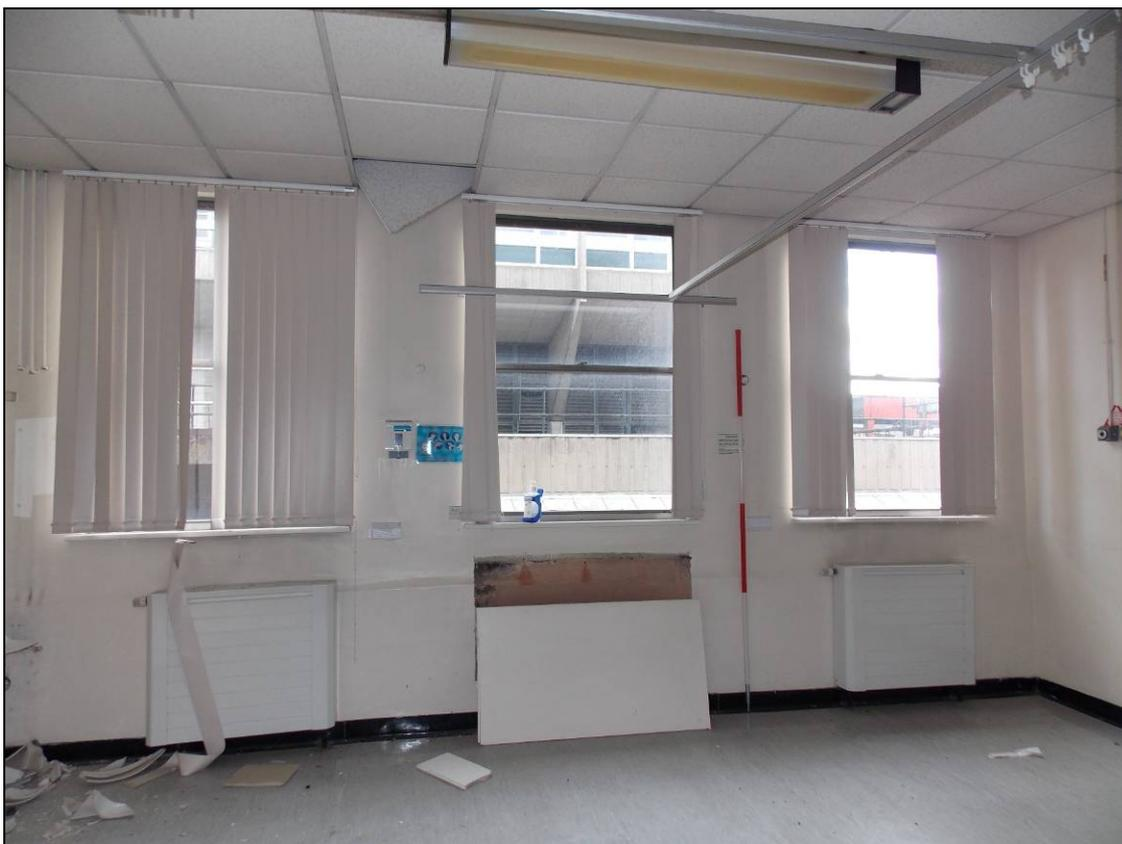
Plate 168: Modern aluminium windows behind the eastern arcade, looking east (scale 2m).
