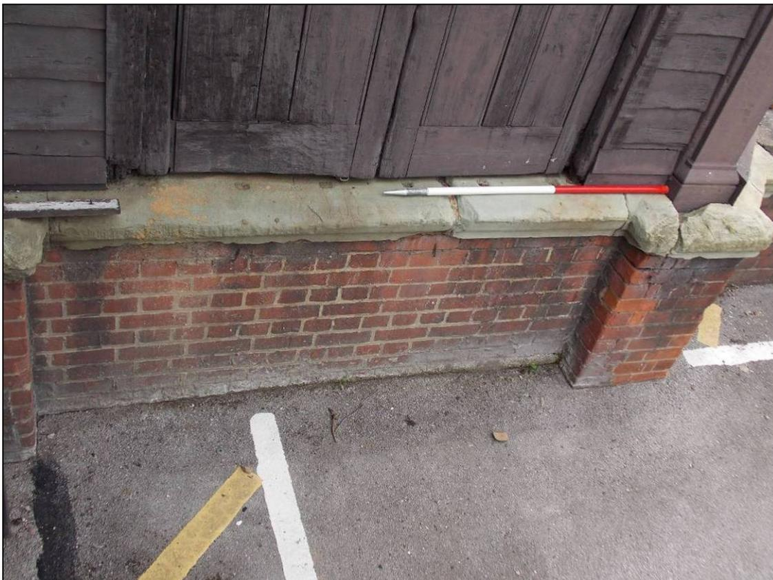
Plate 8: Detail of sandstone coping with sockets of former railings, looking east (scale 1m).
