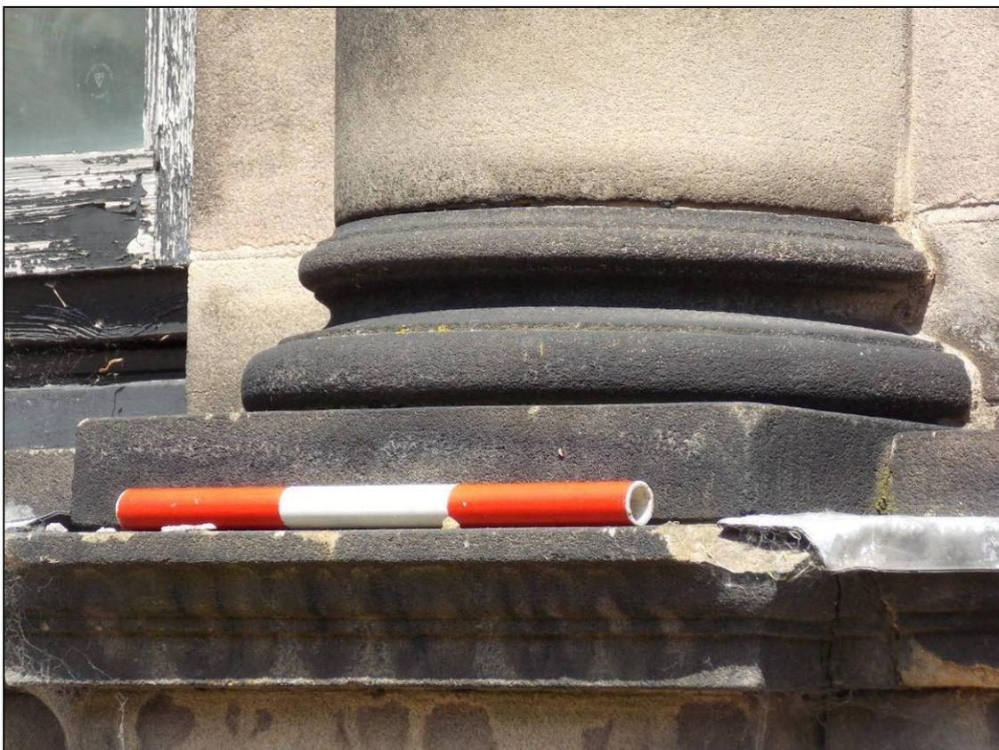
Plate 183: Detail of attic base of engaged column, looking north (scale 300mm).
