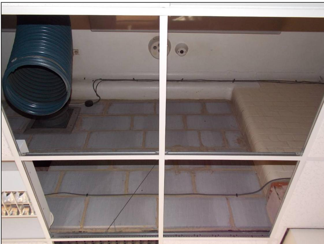
Plate 164: Detail of block-work filling the upper area of the original windows, looking west.
