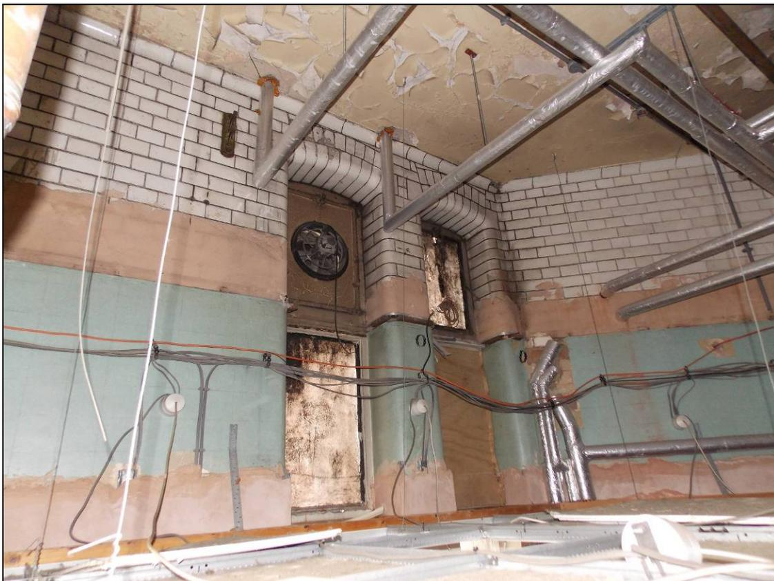
Plate 150: Original brickwork and later rendering over the false ceiling, looking south.
