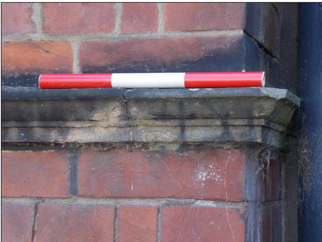
Plate 53: Detail of moulded string-course around the domed tower, looking east (scale 300mm).
