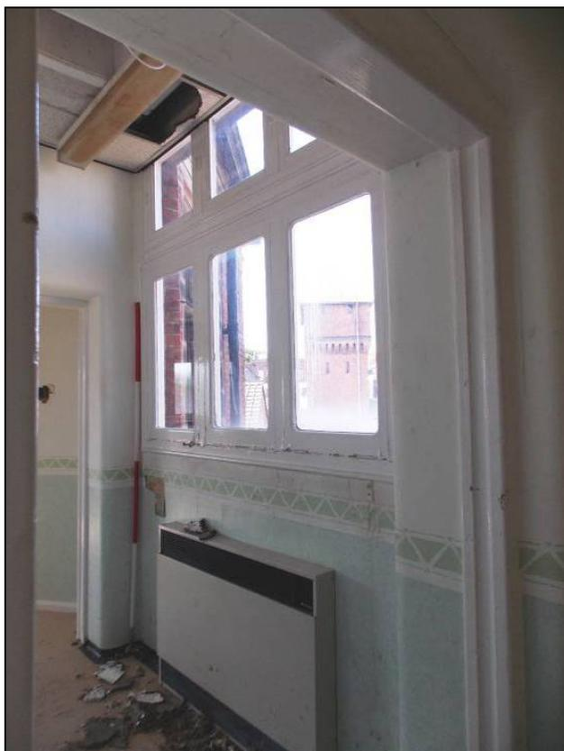
Plate 250: Architrave of former double-action door, looking west (scale 2m).
