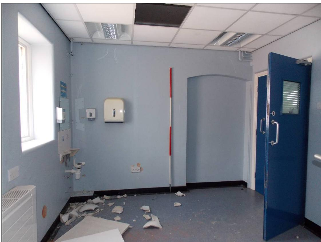
Plate 161: Resus Room with inserted doorway blocked up, looking north (scale 2m).
