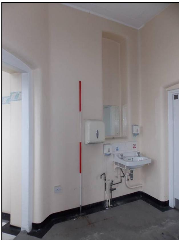
Plate 300: Lobby of lavatory with blocked-up window opening, looking west (scale 2m).
