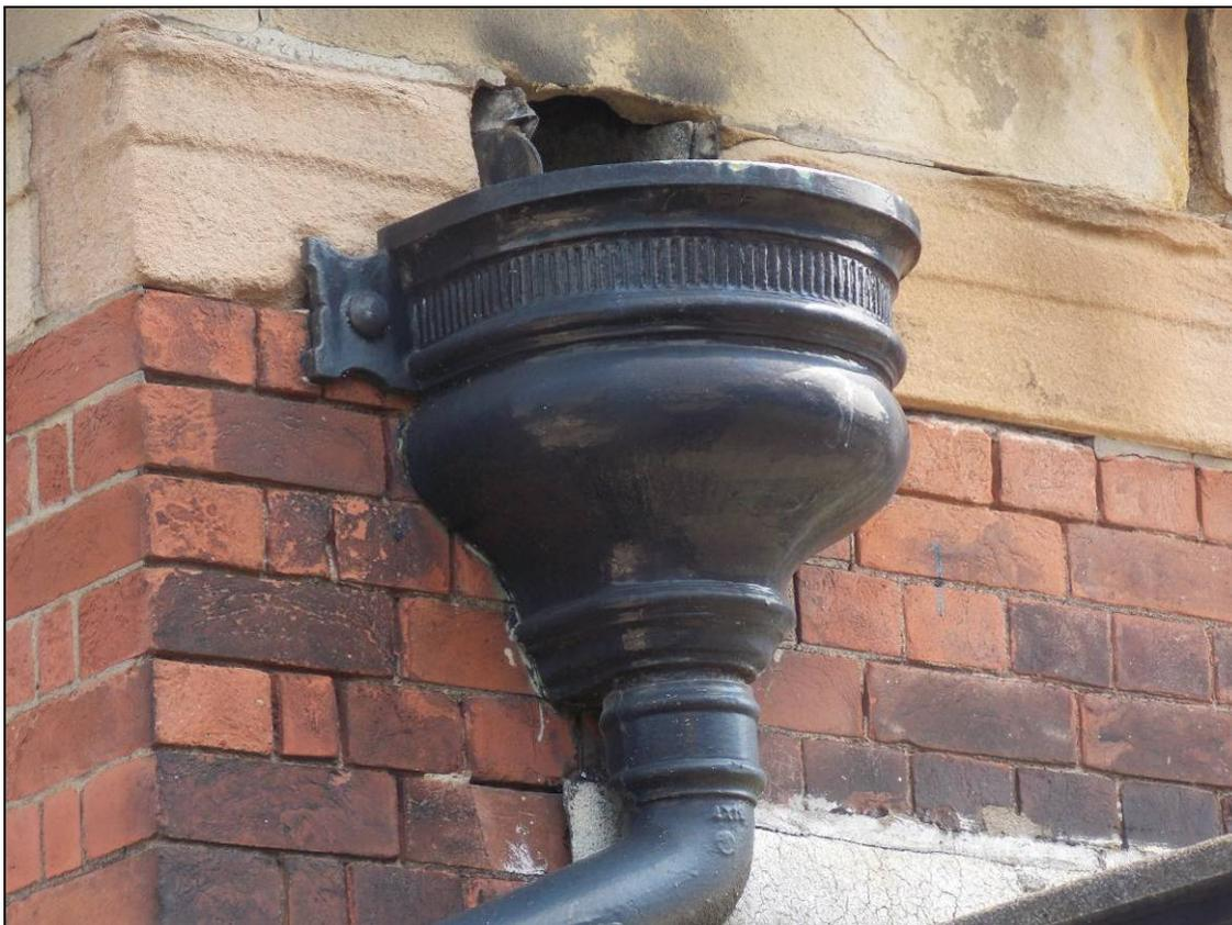
Plate 41: Detail of guttering hopper, looking north-east.
