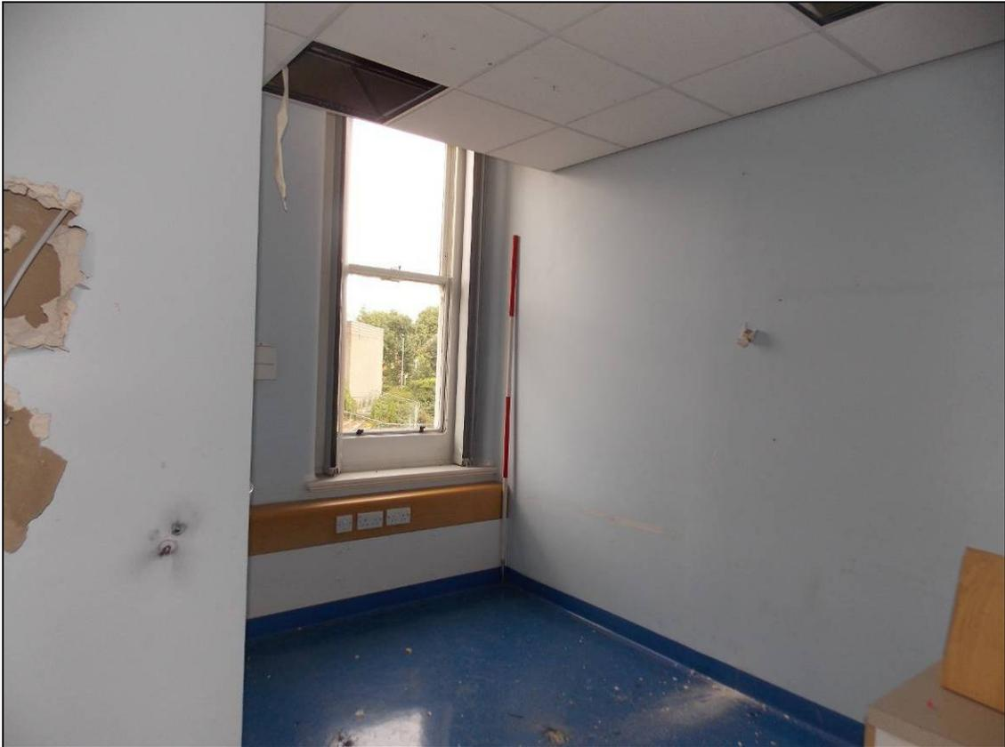
Plate 37: Stud partition wall creating separate rooms, looking north-west (scale 2m).
