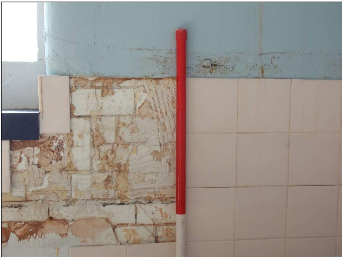
Plate 252: Original glazed brickwork revealed beneath the present tiles, looking south (scale 500mm).
