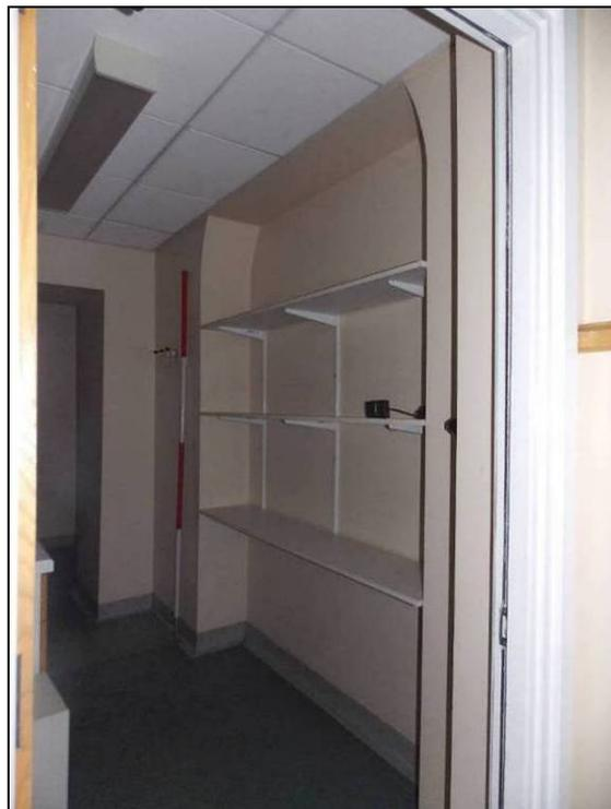
Plate 18: Detail of blocked-up arched doorway inside the small office, looking south-east (scale 2m).
