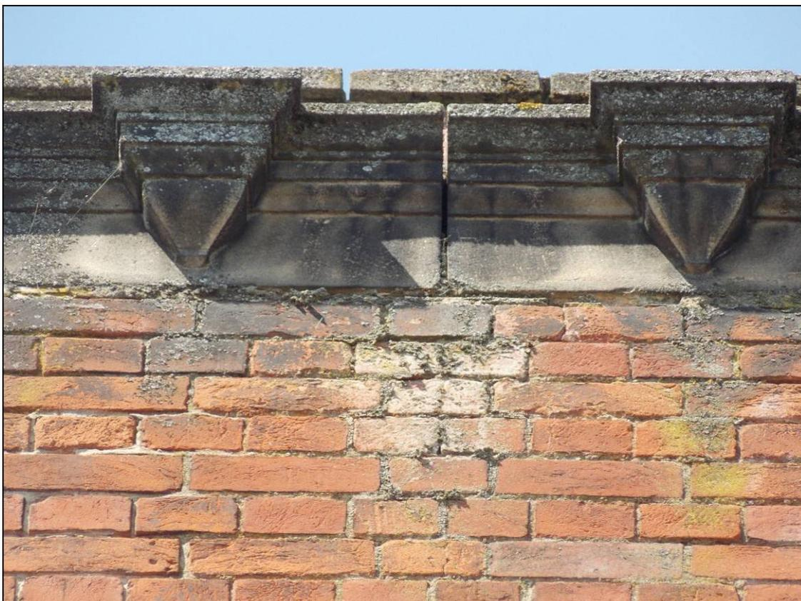
Plate 203: Detail of moulded string-course around the stack, looking west.
