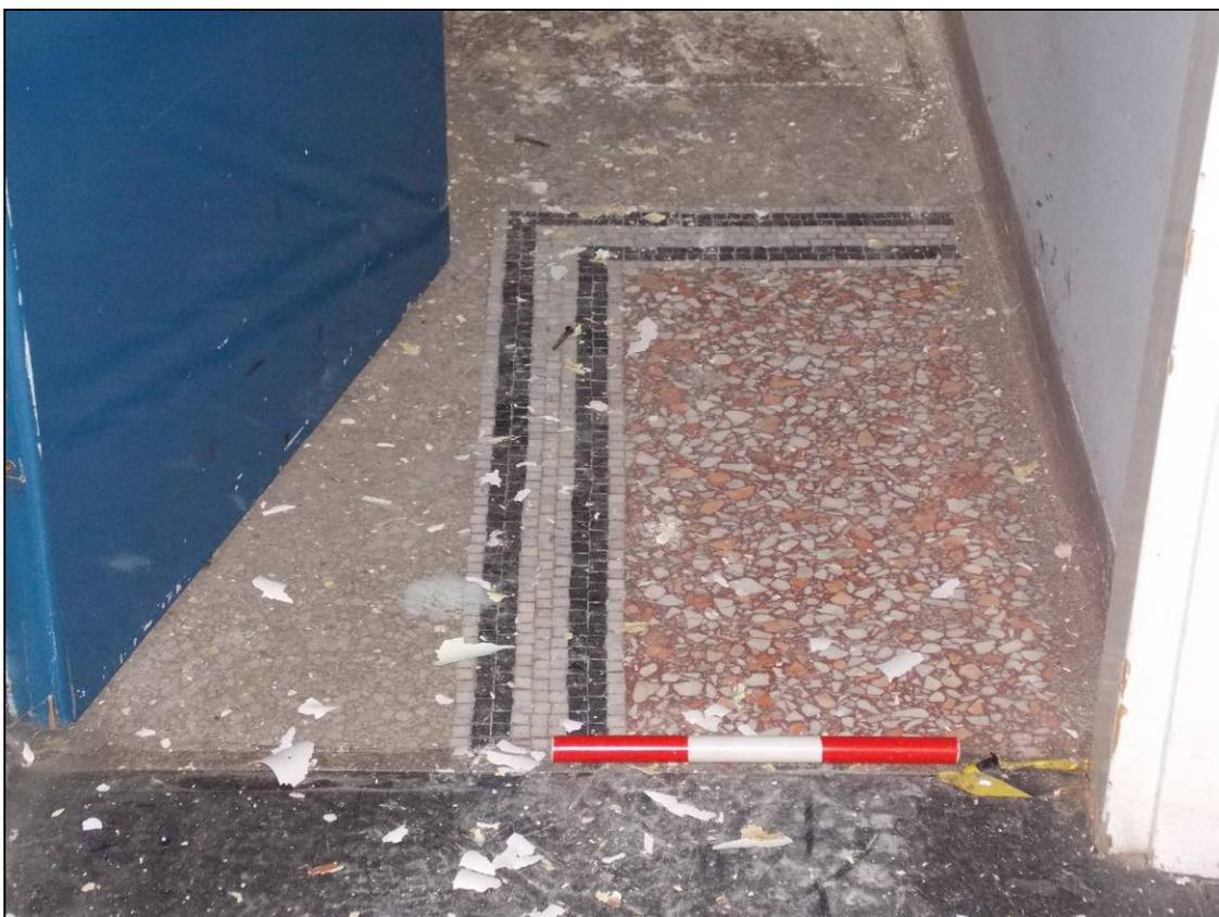
Plate 159: Detail of patterned screed floor with mosaic band, looking west (scale 300mm).
