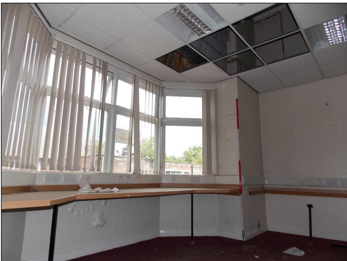
Plate 163: Inserted bay window and blocked-up original windows over the false ceiling, looking north (scale 2m).
