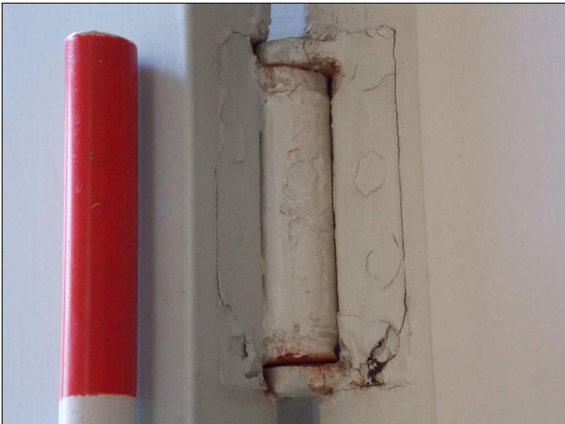
Plate 93: Detail of double action hinge of single door, looking east (scale 100mm).
