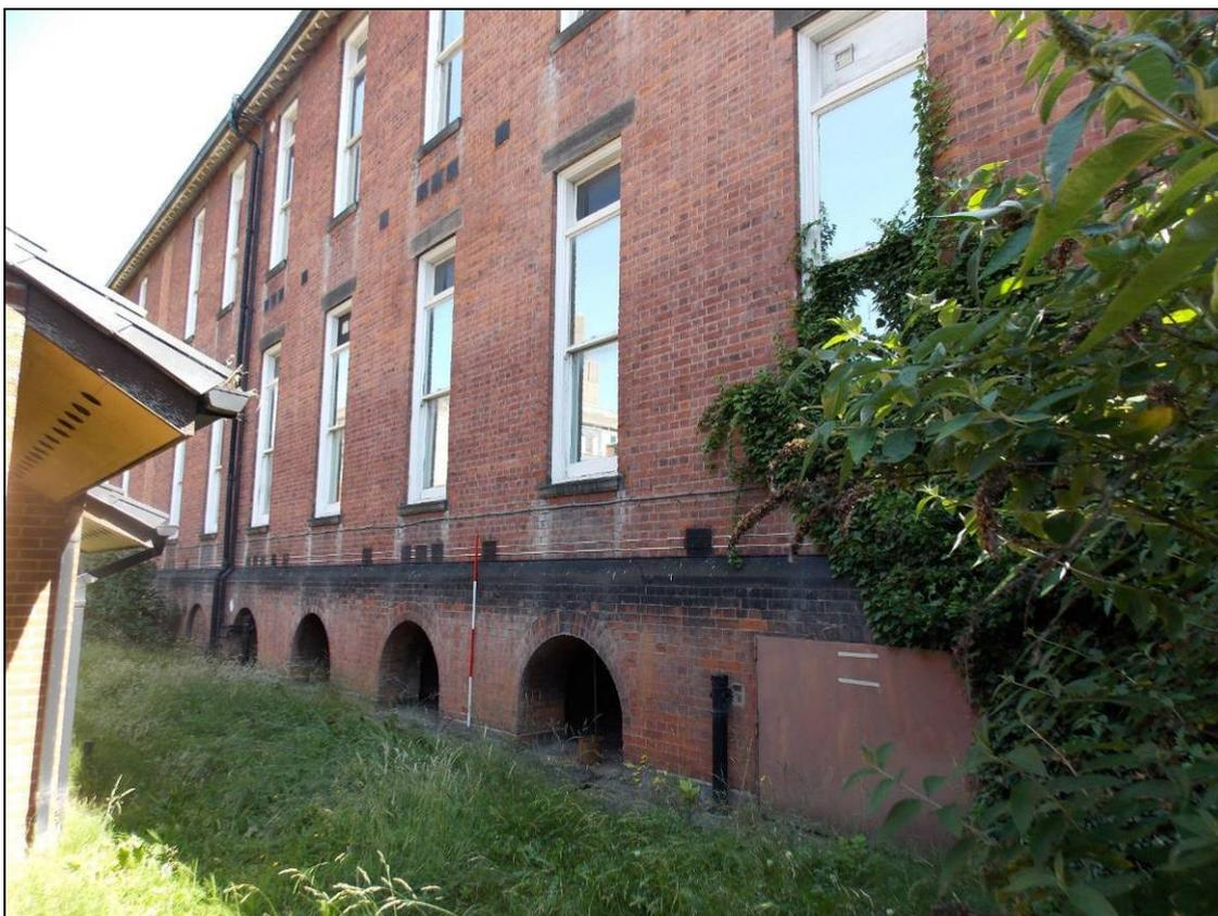
Plate 216: West elevation with arcaded opened basement, looking north-east (scale 2m).
