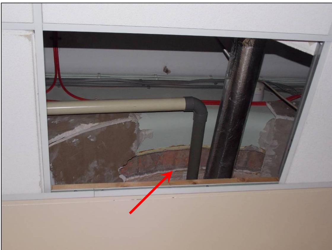
Plate 19: Detail of bullnosed brick *intrados* and scars of former architrave (arrow), looking south.
