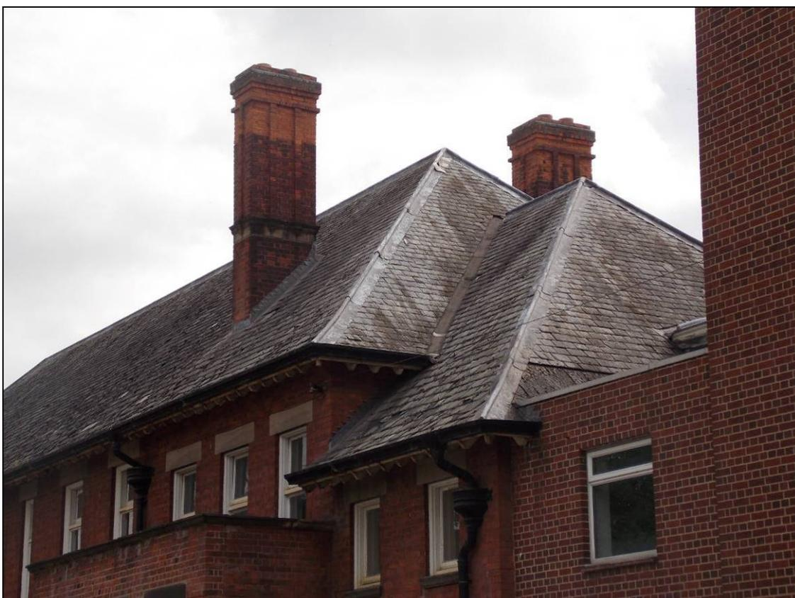
Plate 56: Stepped hipped roof with full-height chimney stacks, looking north-east.
