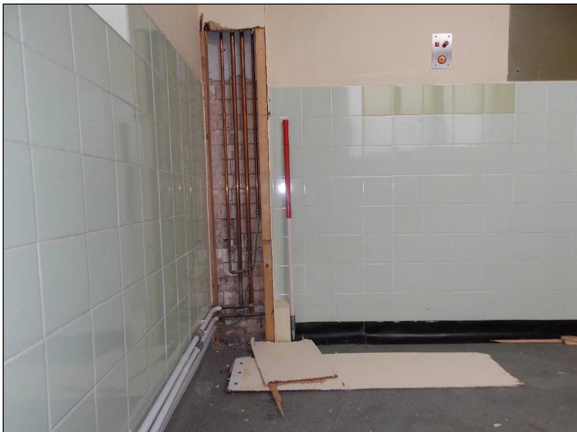
Plate 235: Original glazed brickwork behind copper pipes, looking north (scale 1m).
