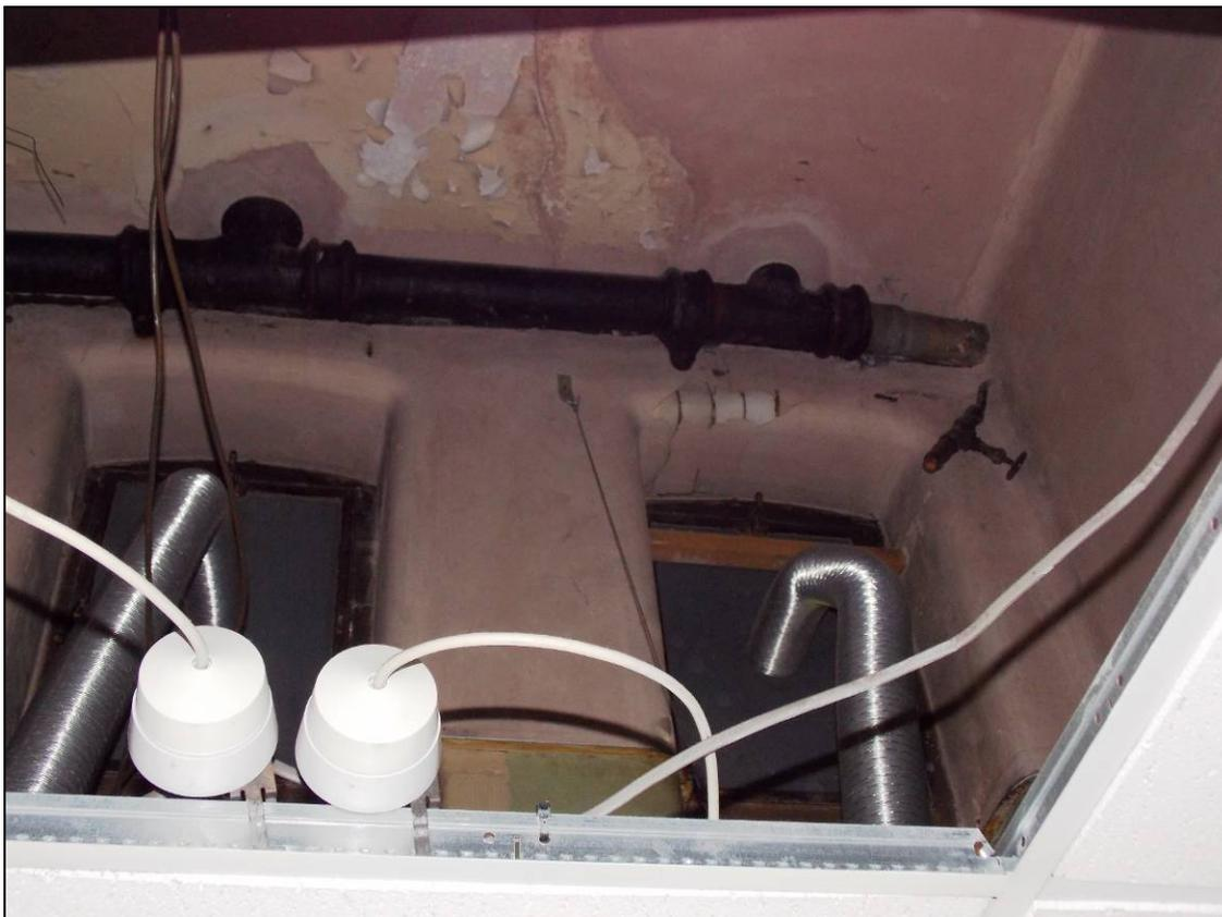
Plate 154: Original glazed brickwork with later rendering over the false ceiling, looking west.
