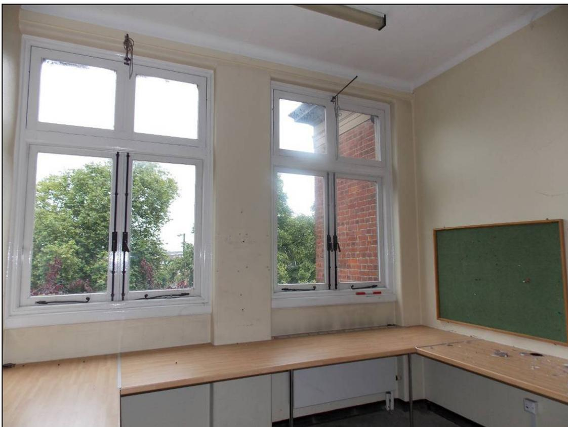
Plate 297: Office with late casement windows, looking north-east (scale 300mm).
