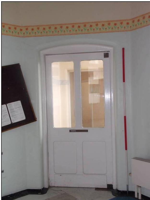
Plate 299: Original glazed double-action door, looking north-east (scale 2m).
