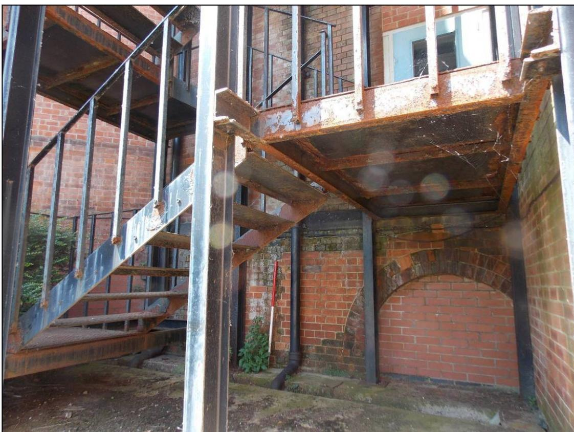
Plate 199: Blocked-up arched opening and fire escape staircase, looking west (scale 1m).
