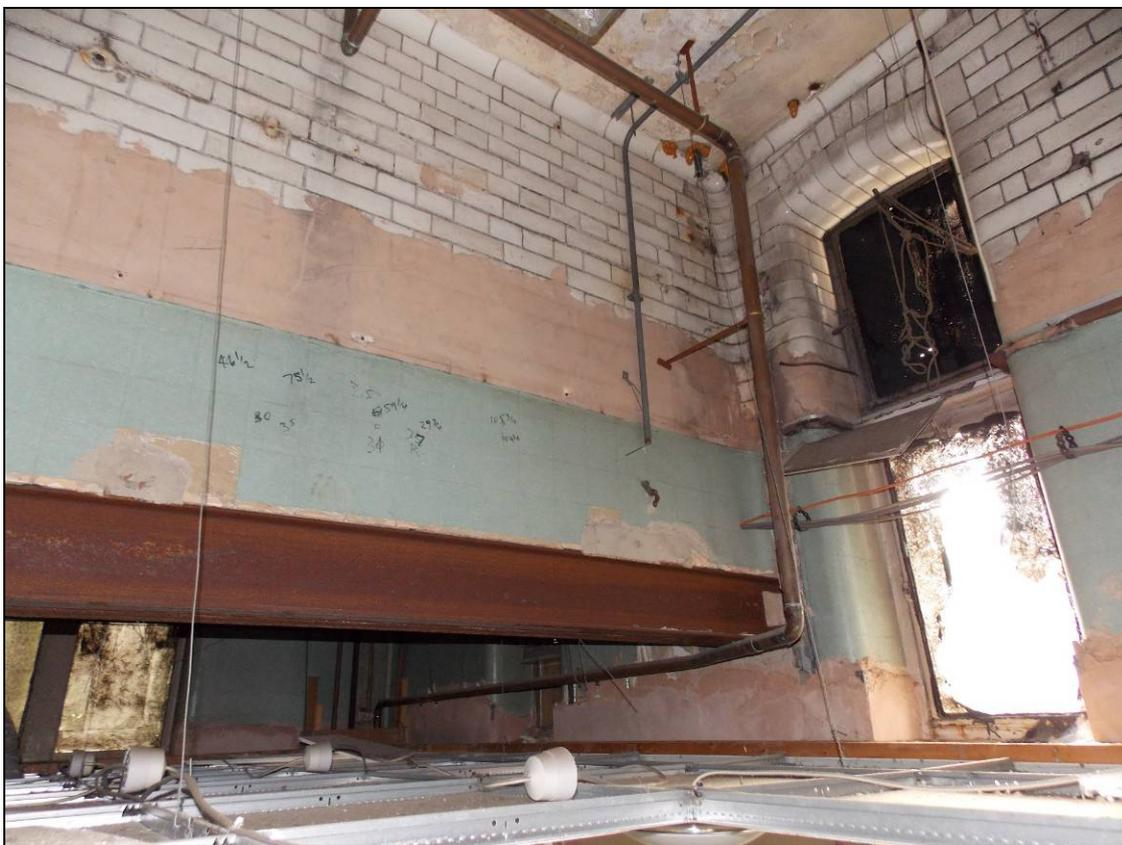
Plate 149: Partially removed partition wall carried by an RSJ, looking south-west.
