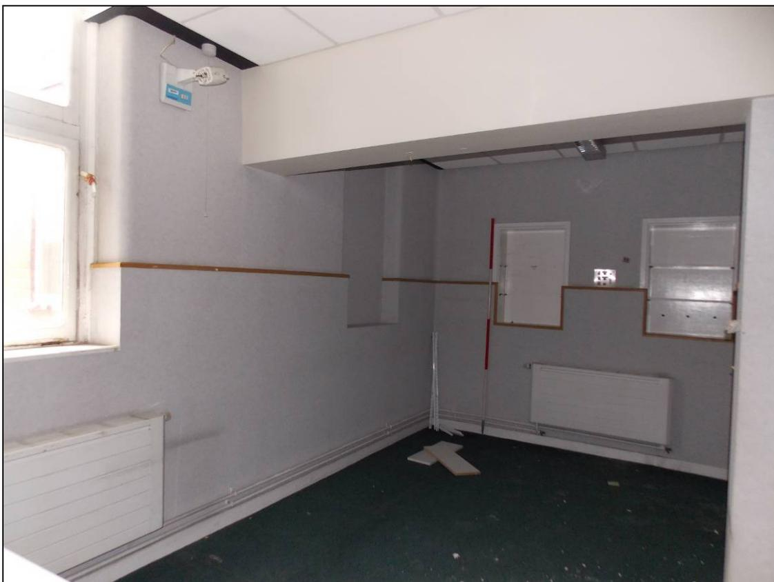
Plate 140: Reception Room with blocked-up window openings, looking south-east (scale 2m).
