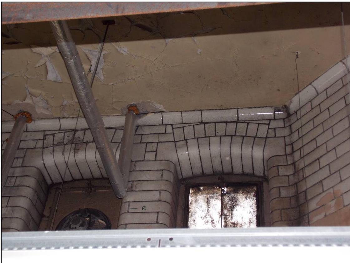
Plate 148: Original glazed brickwork over the false ceiling, looking south.
