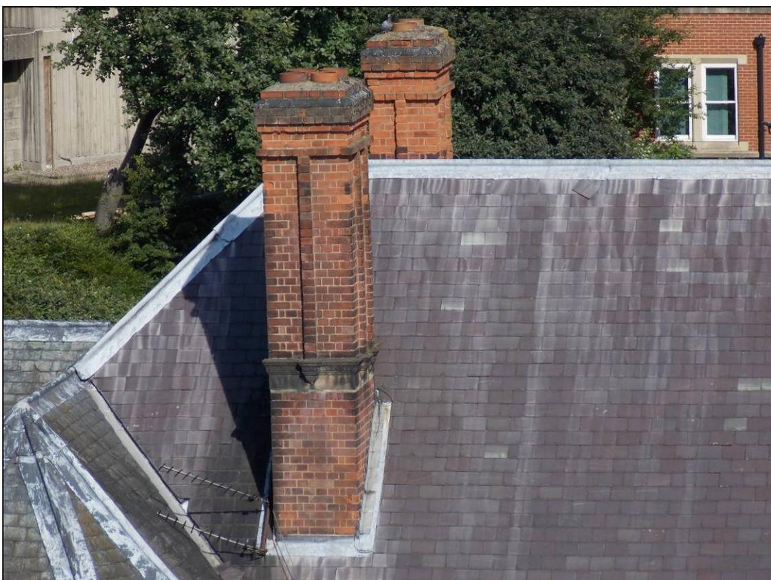
Plate 50: Full-height southern stacks containing pots, flaunching and crown, looking west.
