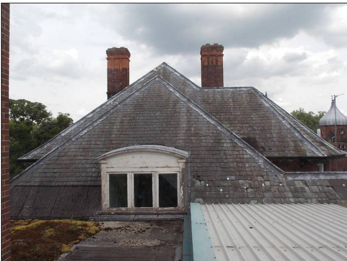
Plate 58: Southern end of the hipped roof with a central dormer window, looking north.
