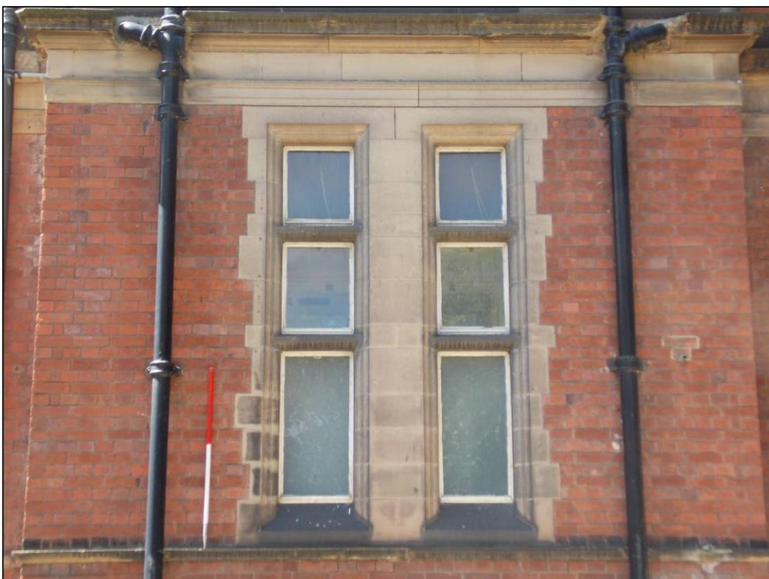
Plate 44: Detail of mullion window within the domed tower, looking west (scale 1m).
