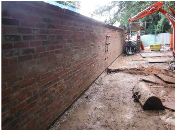
The new wall construction, looking south.
