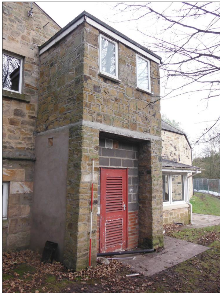
Figure 52: Northwest and southwest elevation of Building E (scale=2m).
