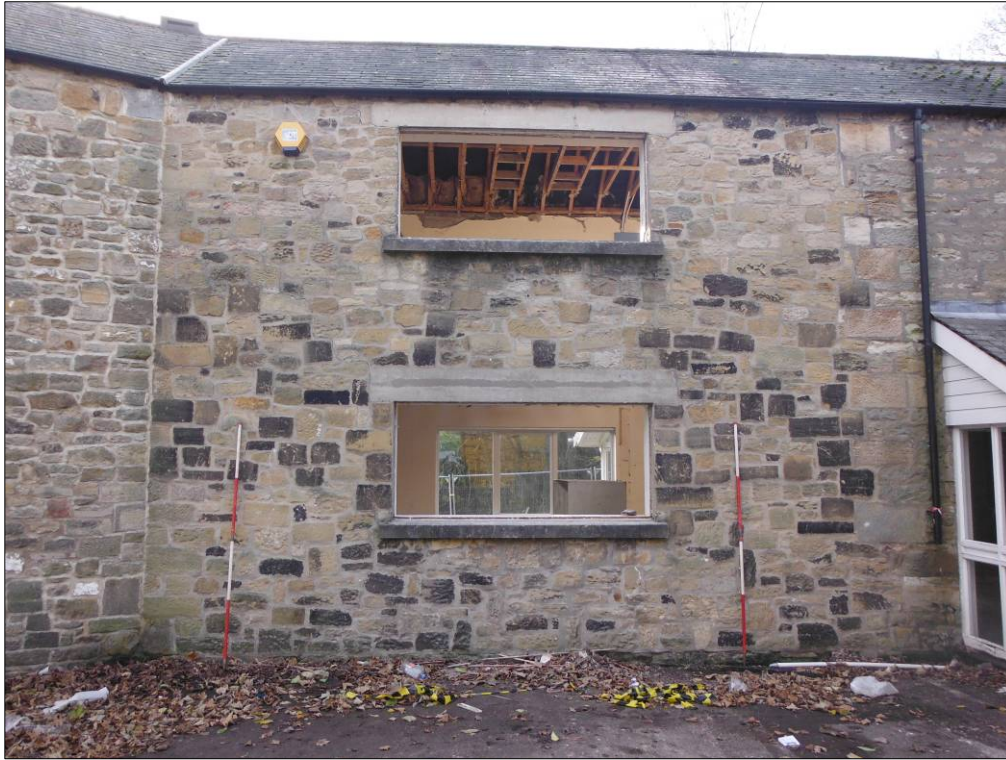
Figure 6: Northeast elevation of Building B (scale=2 x 2m).
