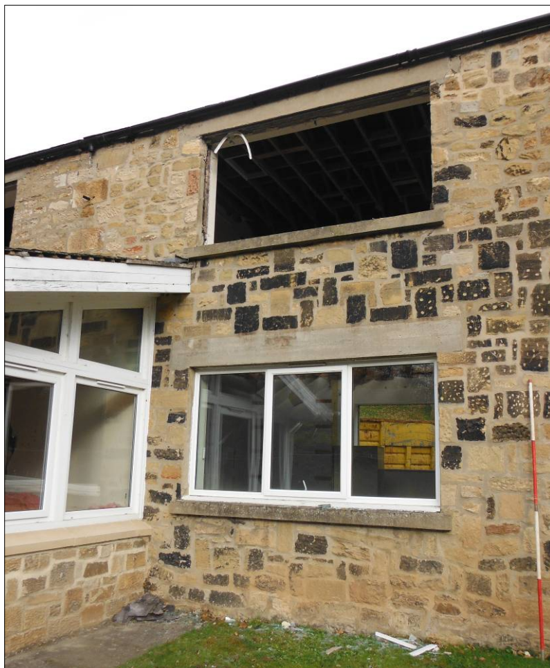
Figure 7: Southwest elevation of Building B (scale=2m).
