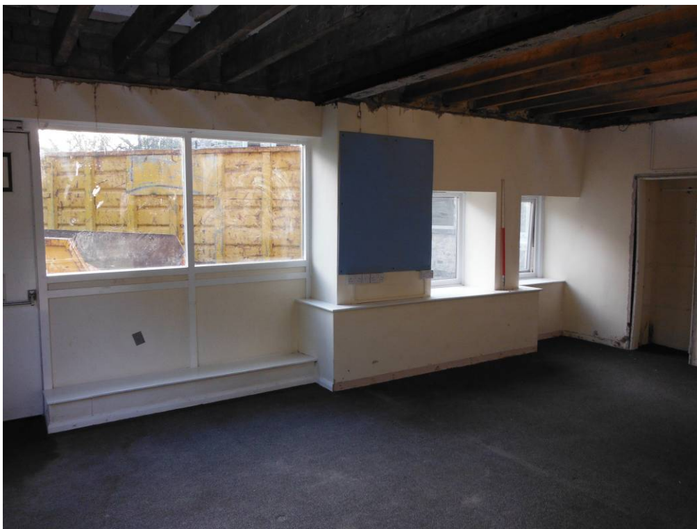
Figure 35: Southeast wall of Room C3 (scale=2m).
