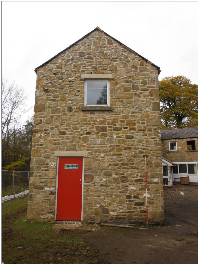
Figure 3: Southeast elevation of Building A (scale= 2m).
