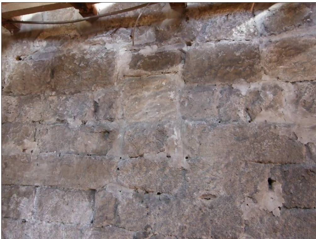
Figure 41: Rectangular slot in the northeast wall of Room C4 marking the location of a possible drive shaft.
