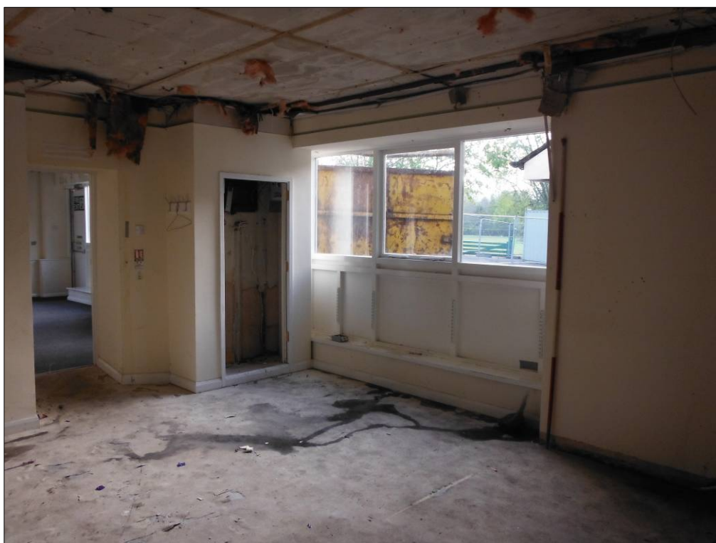
Figure 33: Northeast and southeast walls of Room C2 (scale=2m).
