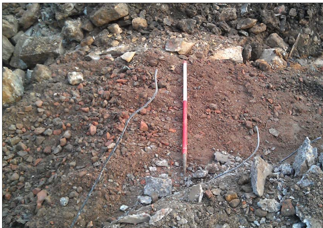
Figure 86: Brick and concrete chippings (004) beneath the concrete pad (003) in Building C, Room C4.
