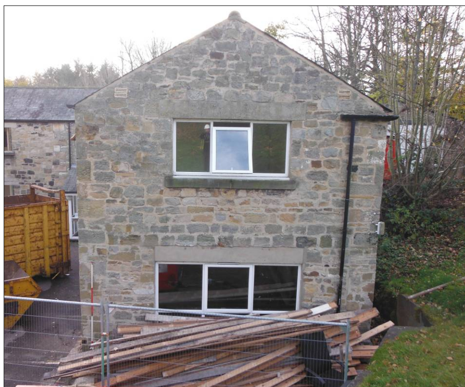
Figure 10: Northeast elevation of Building C Part 2 (scale=2m).
