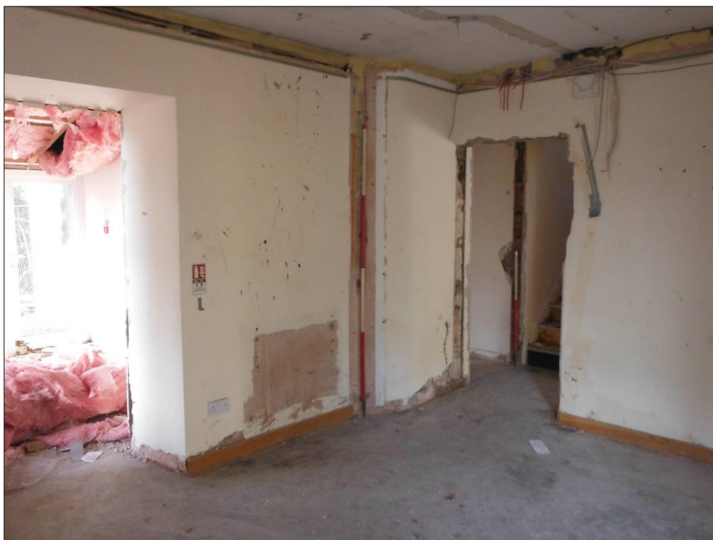
Figure 28: Northwest and southwest walls of Room C1 (scale=2m + 1m).
