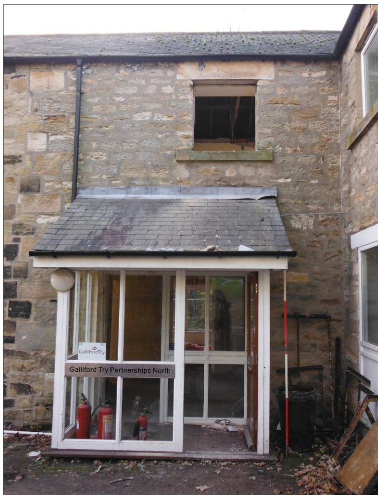
Figure 9: Northeast elevation of Building C Part 1 (scale=2m).
