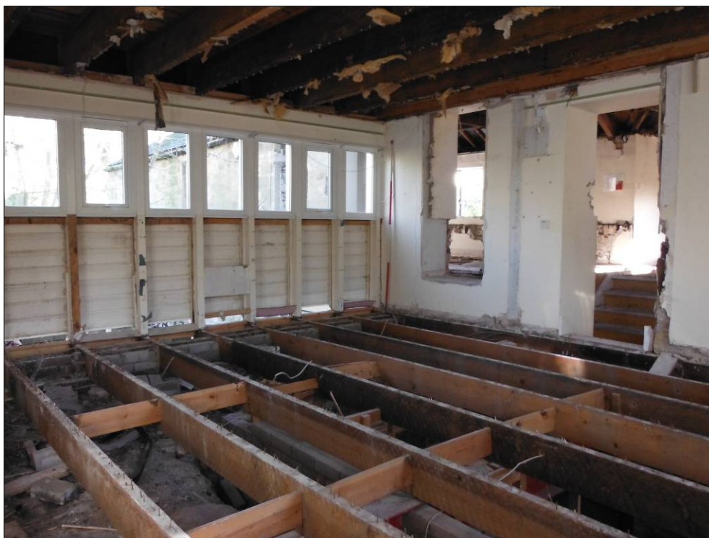
Figure 22: Inserted doorways on the northwest elevation of Building C contained within Building F (scale=2m).
