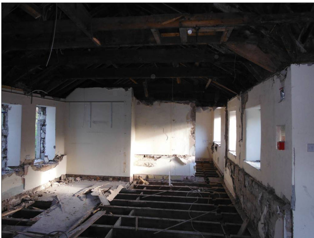
Figure 46: First floor over Room C2.
