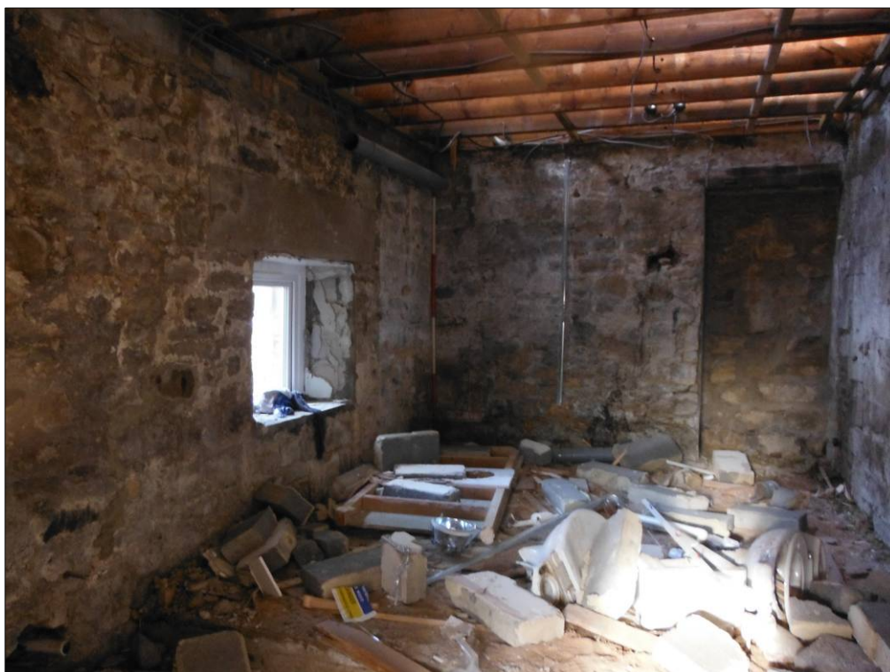
Figure 38: Southwest and northwest walls of Room C4 (scale=2m).
