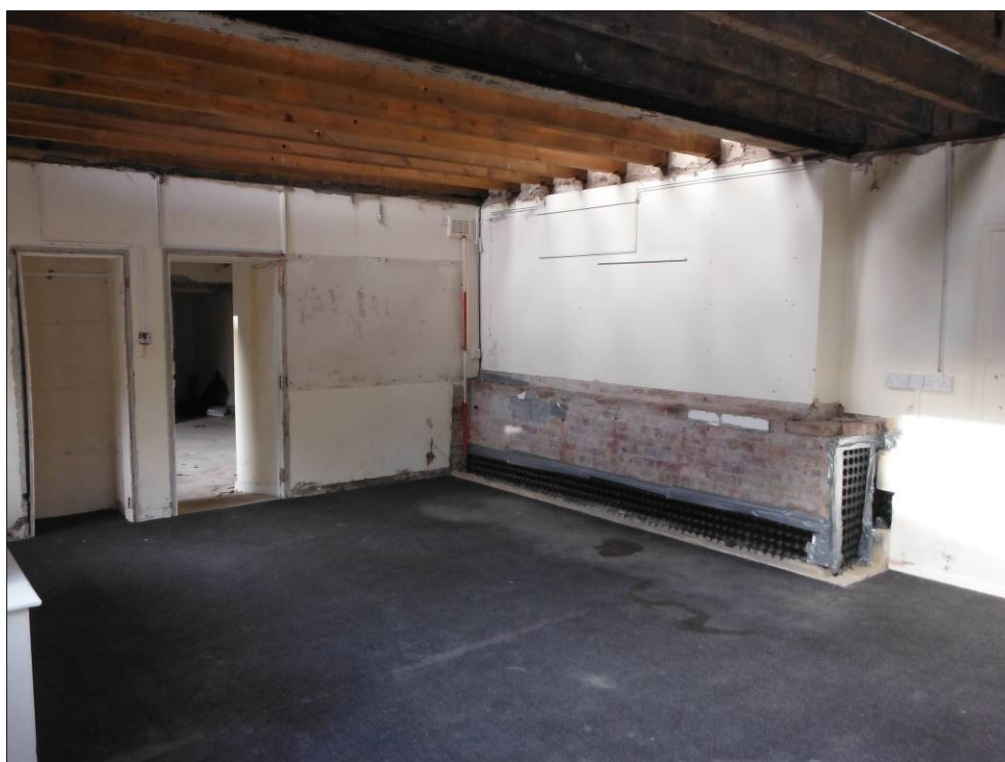
Figure 34: Southwest and northwest walls of Room C3 (scale=2m).
