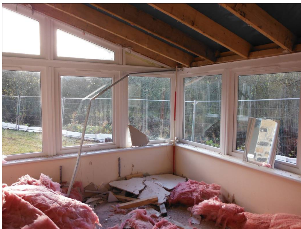
Figure 51: Southeast and southwest walls of Building D (scale=2m).
