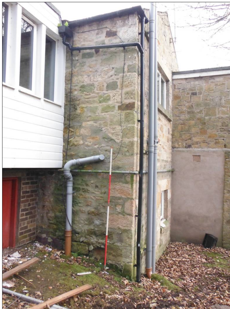
Figure 24: Western end of the northwest elevation of Building C (scale=1m).
