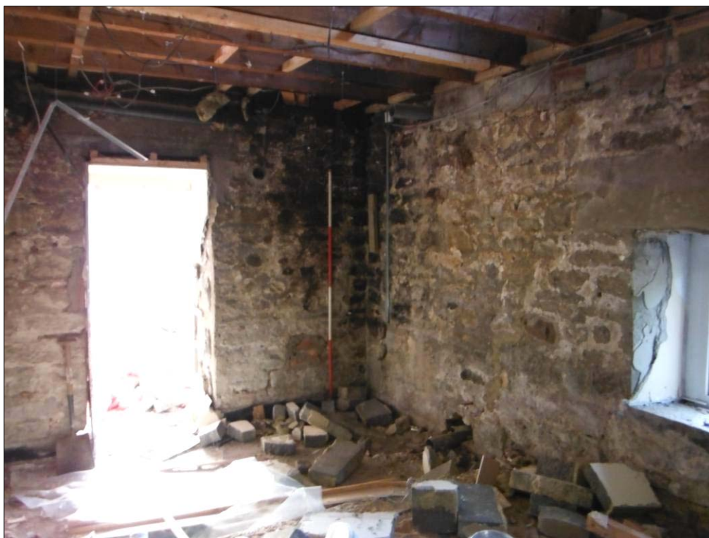
Figure 37: Southeast wall of Room C4 (scale=2m).
