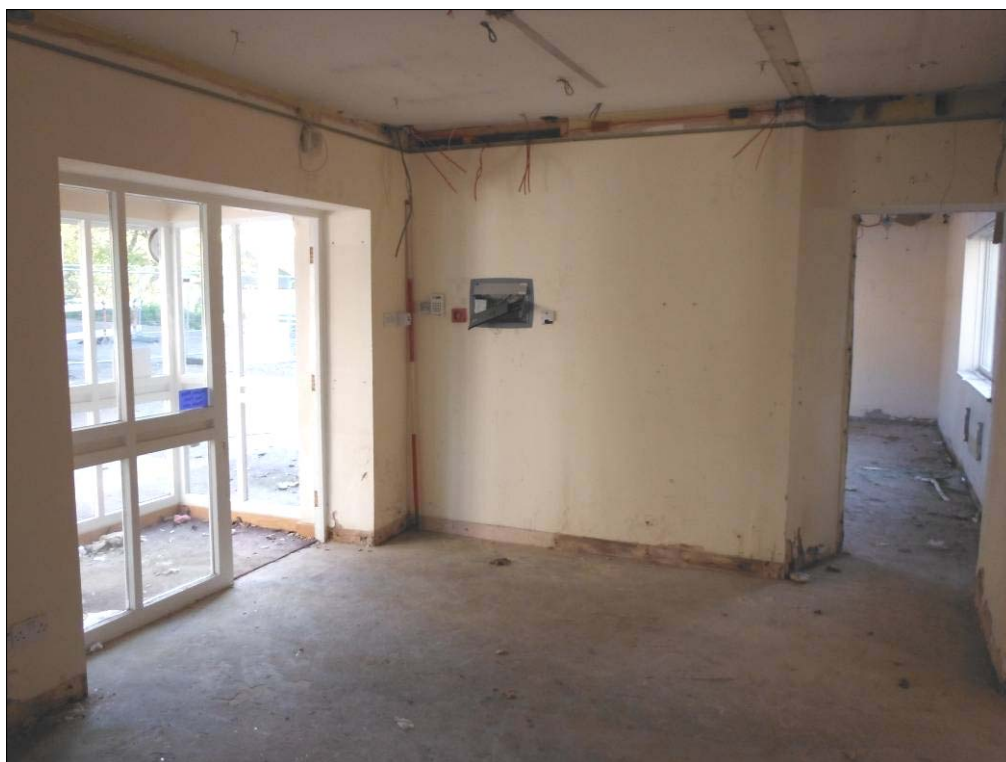
Figure 27: Northeast and southeast walls of Room C1 (scale=2m).
