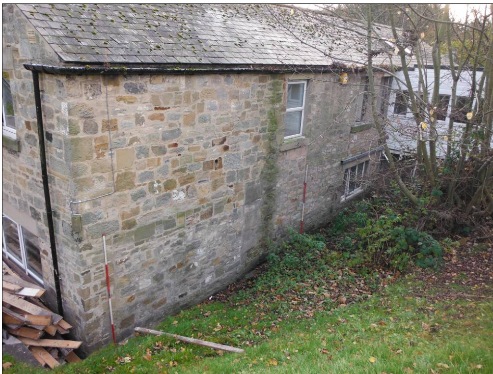
Figure 17: Northwest elevation of Building C (scale=2 x 2m).
