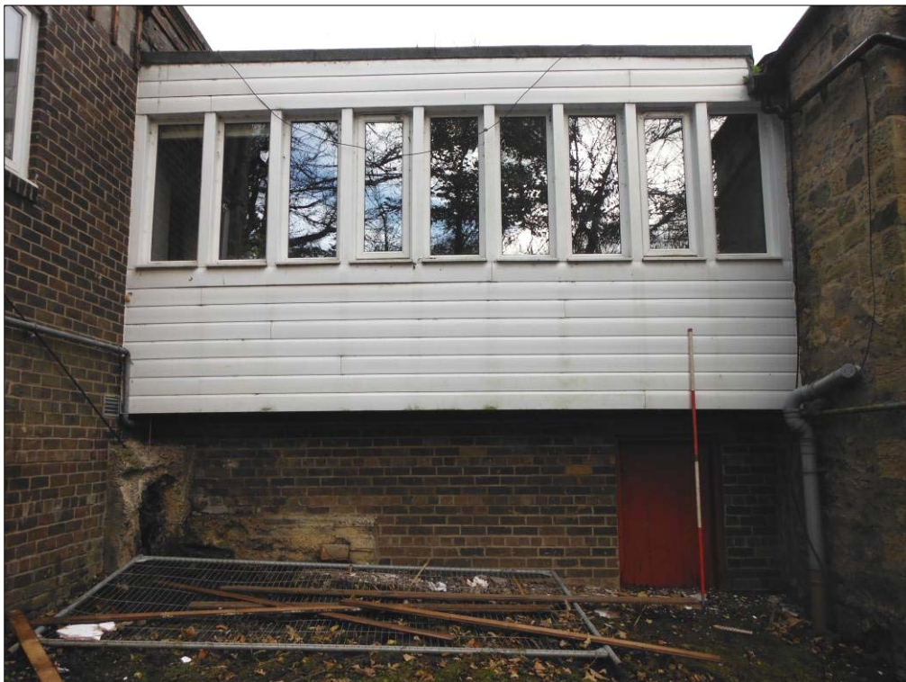
Figure 53: Southwest elevation of Building F (scale=2m).
