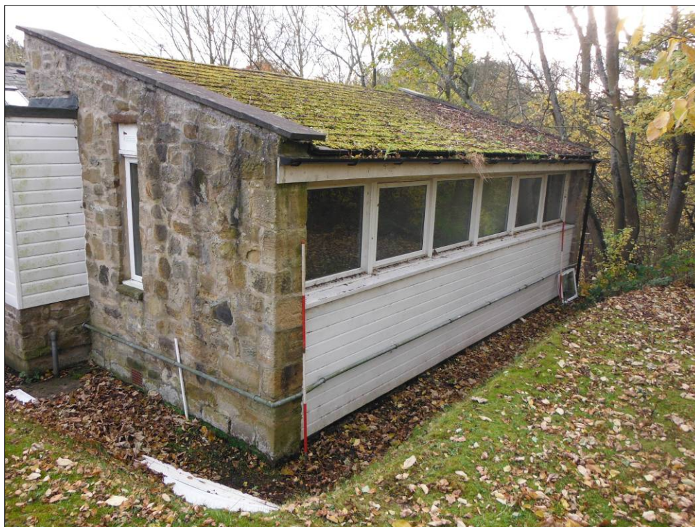
Figure 58: Northeast and northwest elevation of Building G (scale=2 x 2m).
