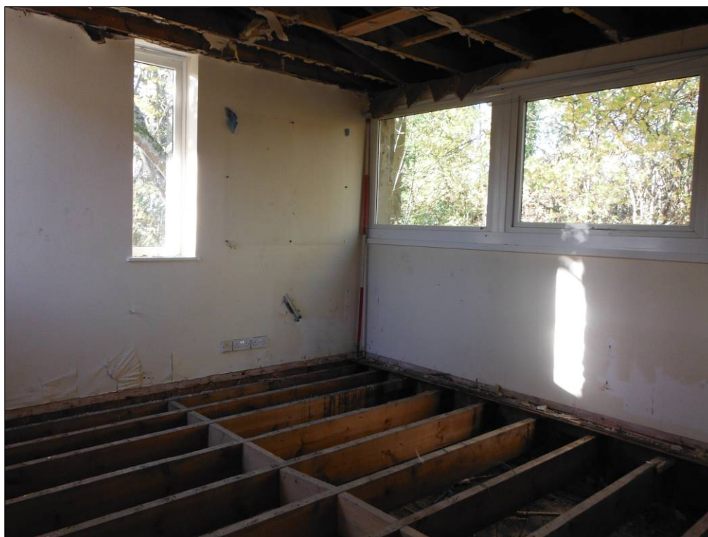
Figure 59: Southwest and Northwest walls of Room G1 (scale=2m).
