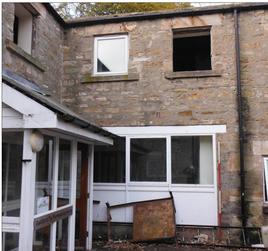
Figure 13: Westernmost section of the southeast elevation of Building C (scale=2m).
