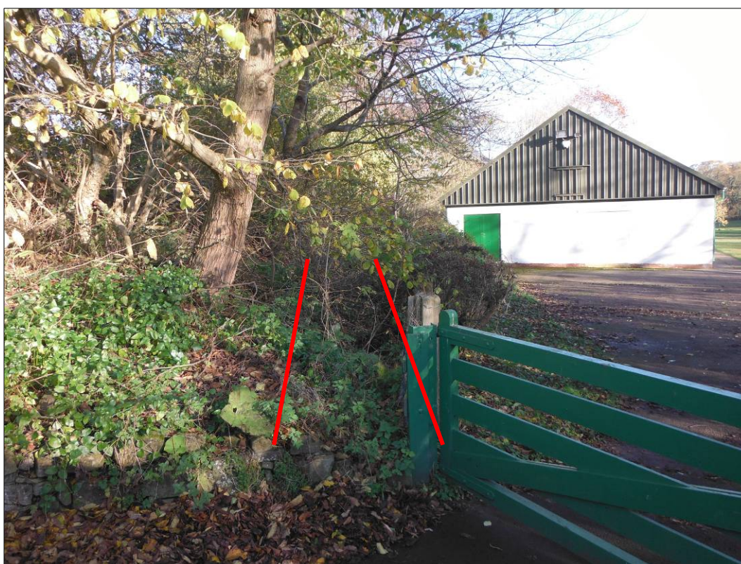
Figure 63: Length of surviving tail race to the east of the building (highlighted in red), surviving in use as a property boundary ditch at the centre of the picture. The earthwork is greatly obscured by foliage.
