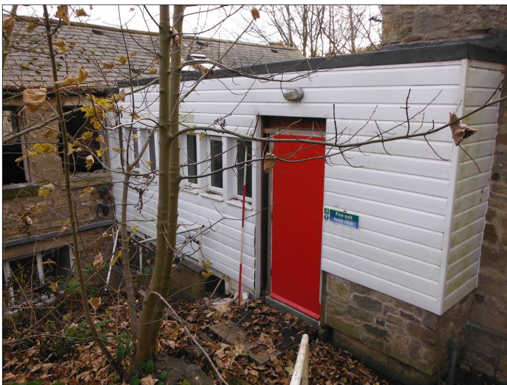
Figure 54: Northeast elevation of Building F (scale=2m).
