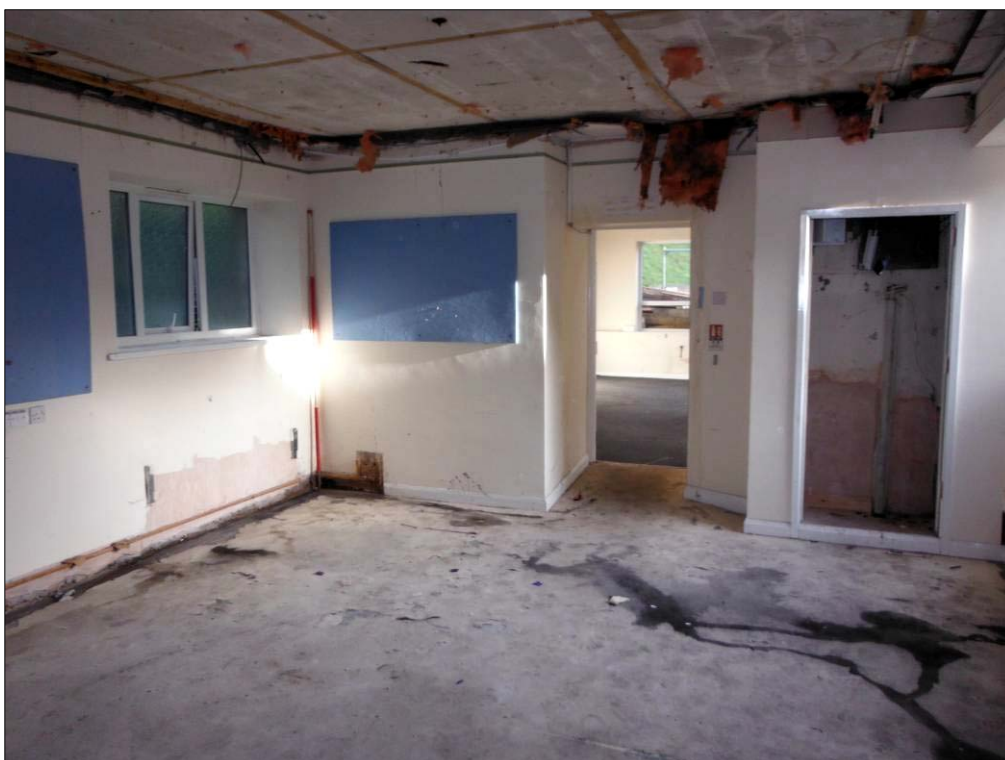
Figure 30: Northwest and northeast walls of Room C2 (scale=2m).
