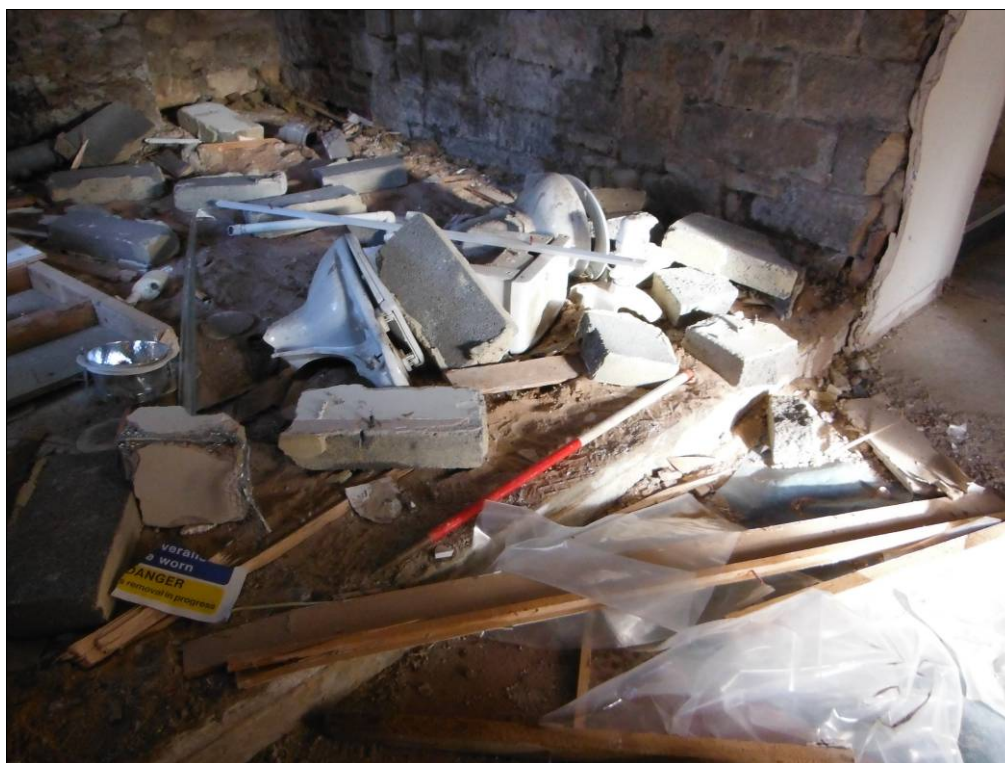
Figure 43: Concrete platform covering the probable location of the wheel pit in Room C4 (scale 1m).
