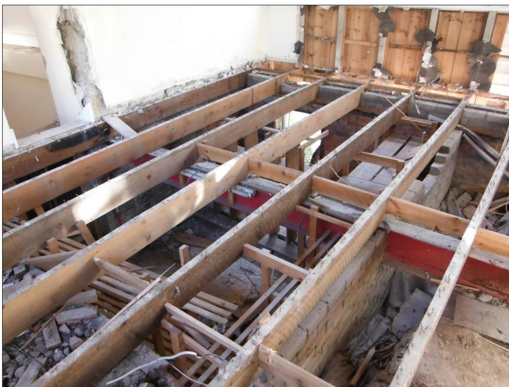
Figure 55: Basement room beneath the floor of Building F.
