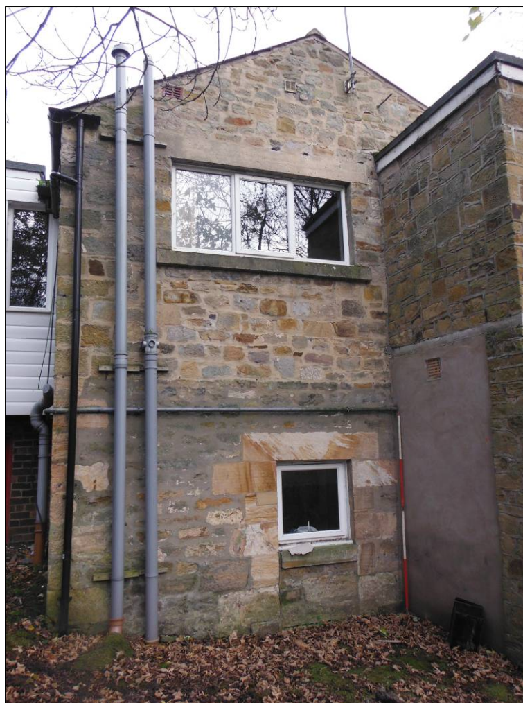
Figure 26: Southwest elevation of the main range of Building C (scale=2m).
