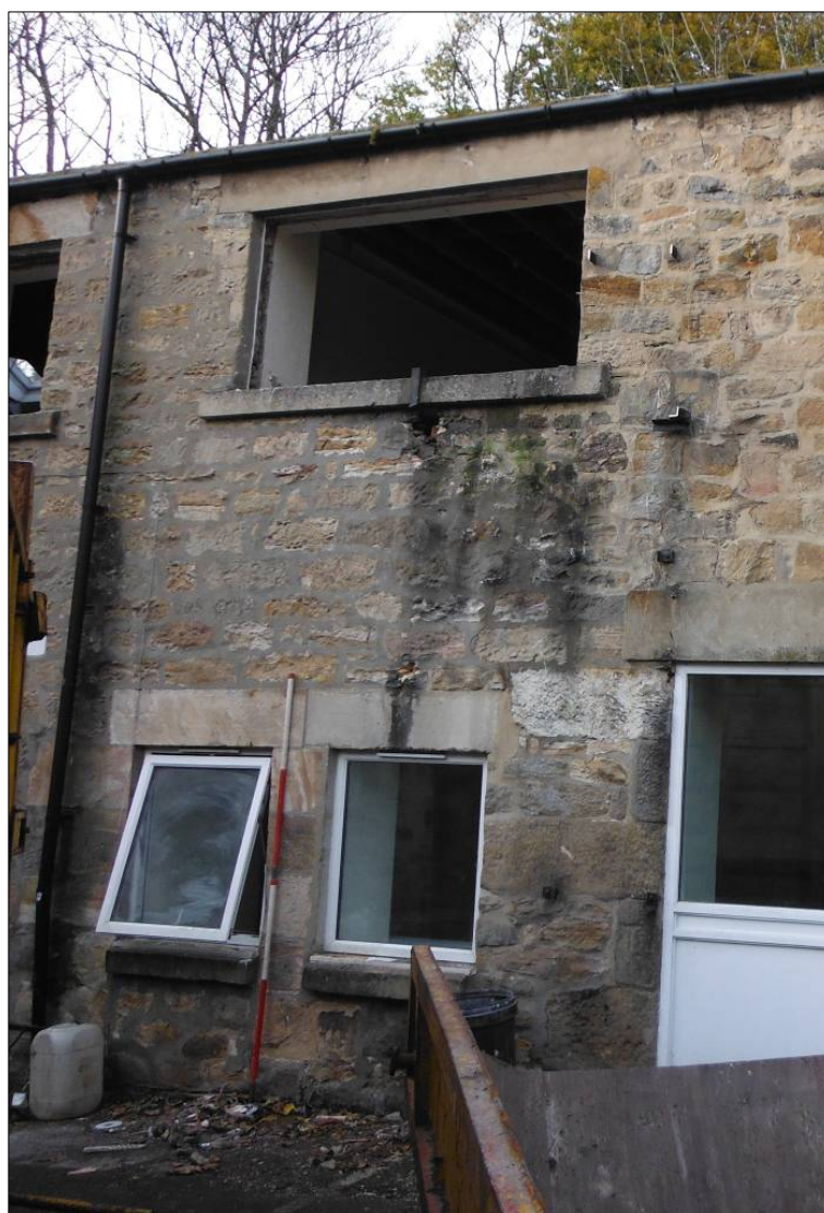
Figure 14: Middle section of the southeast elevation of Building C (scale=2m).
