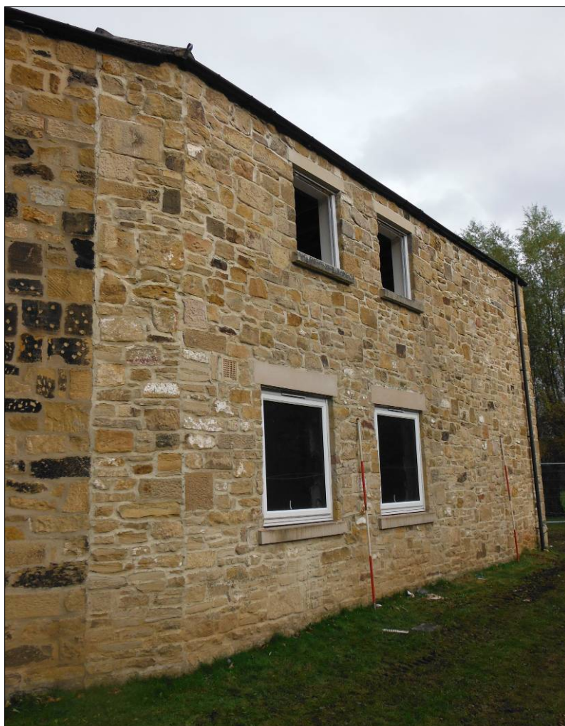
Figure 4: Southwest elevation of Building A (scale=2 x 2m).
