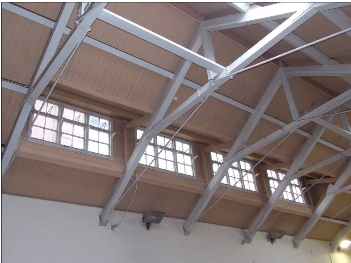
Plate 45: Glazed clerestory along the western side of the pitched roof.
