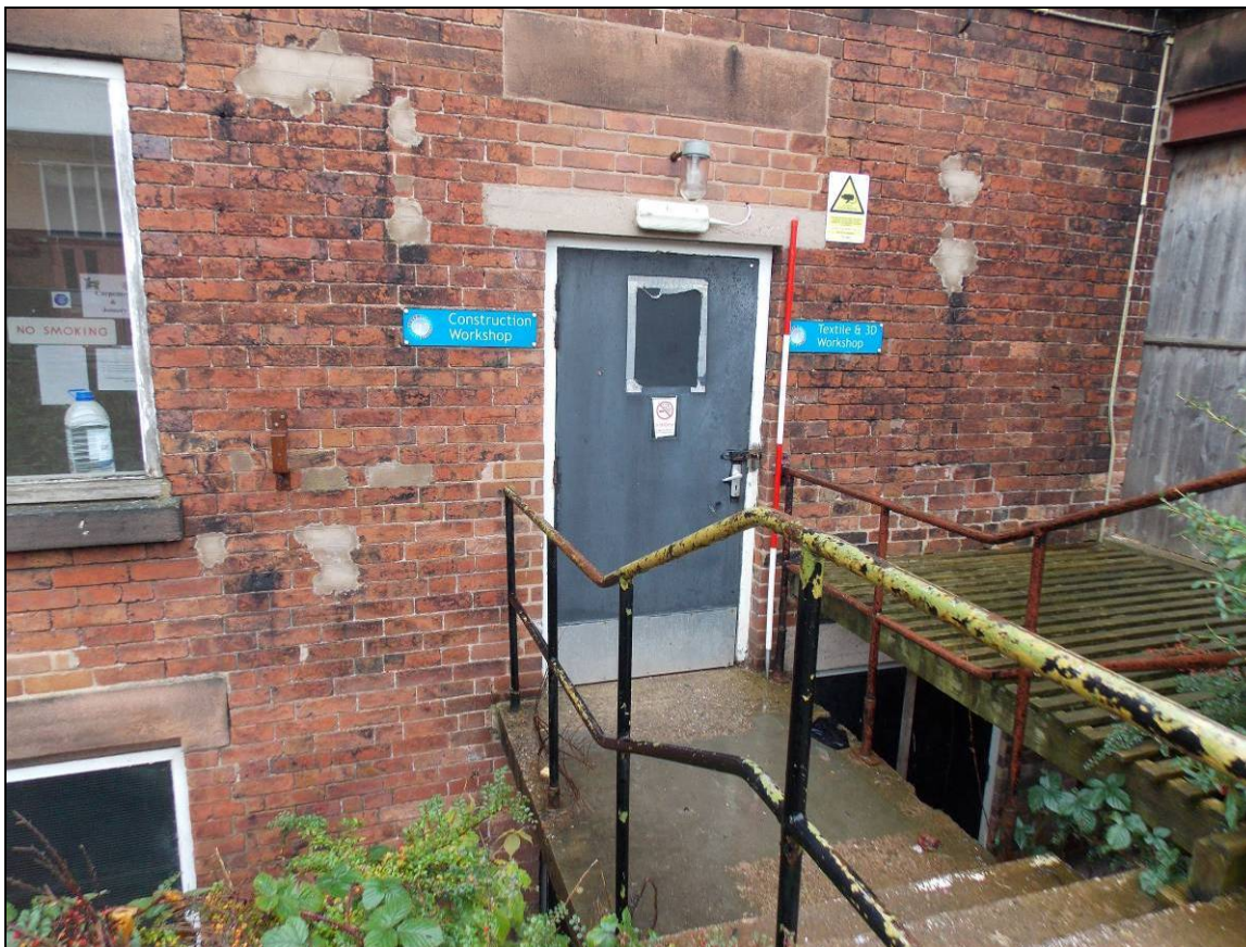
Plate 57: First floor's entrance, looking east (scale 2m).
