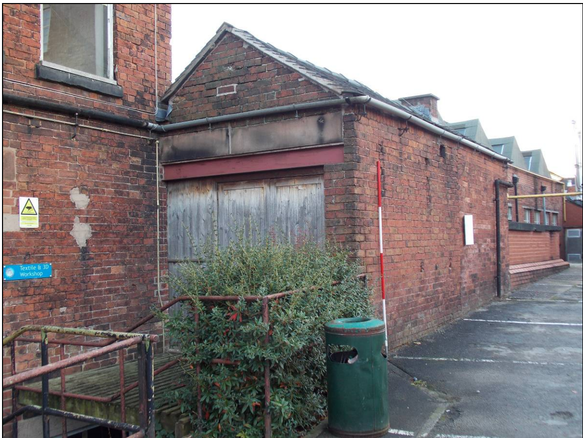
Plate 59: Later southern extension, looking south (scale 2m).
