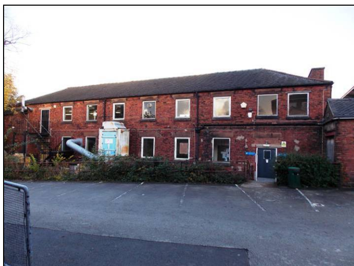
General view of the former Mill
