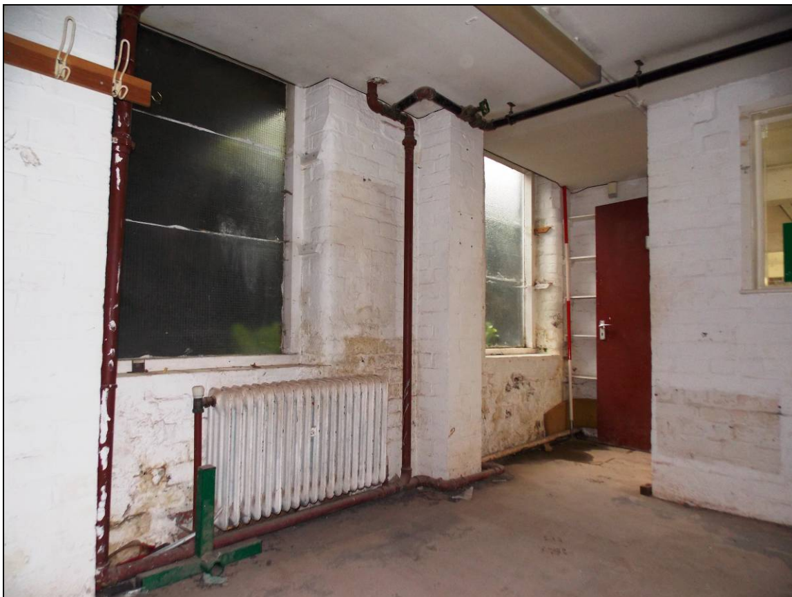
Plate 78: South-western room, looking north-west (scale 2m).
