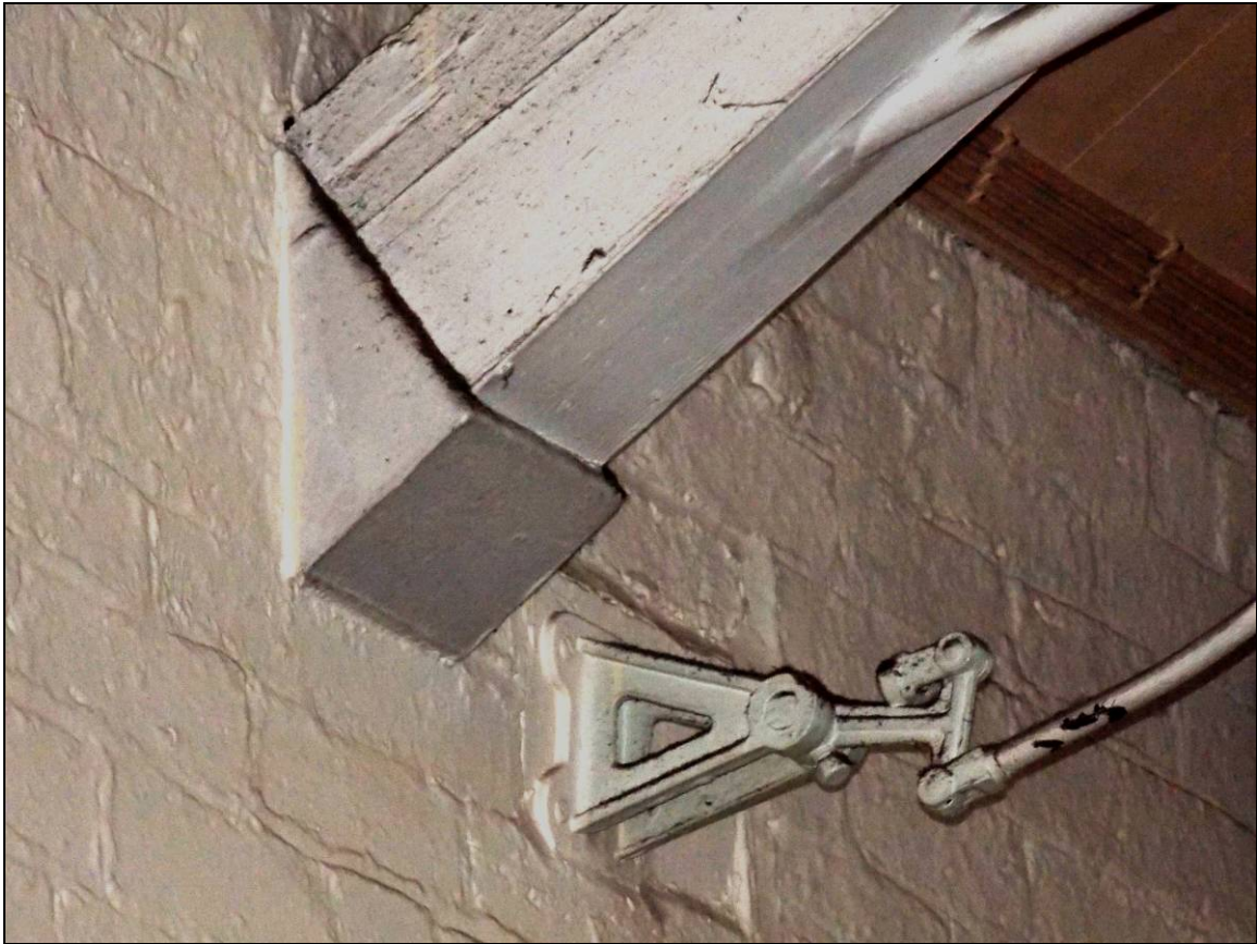
Plate 44: Detail of principal rafter's shoe and fitting for the opening of the glazed clerestory.
