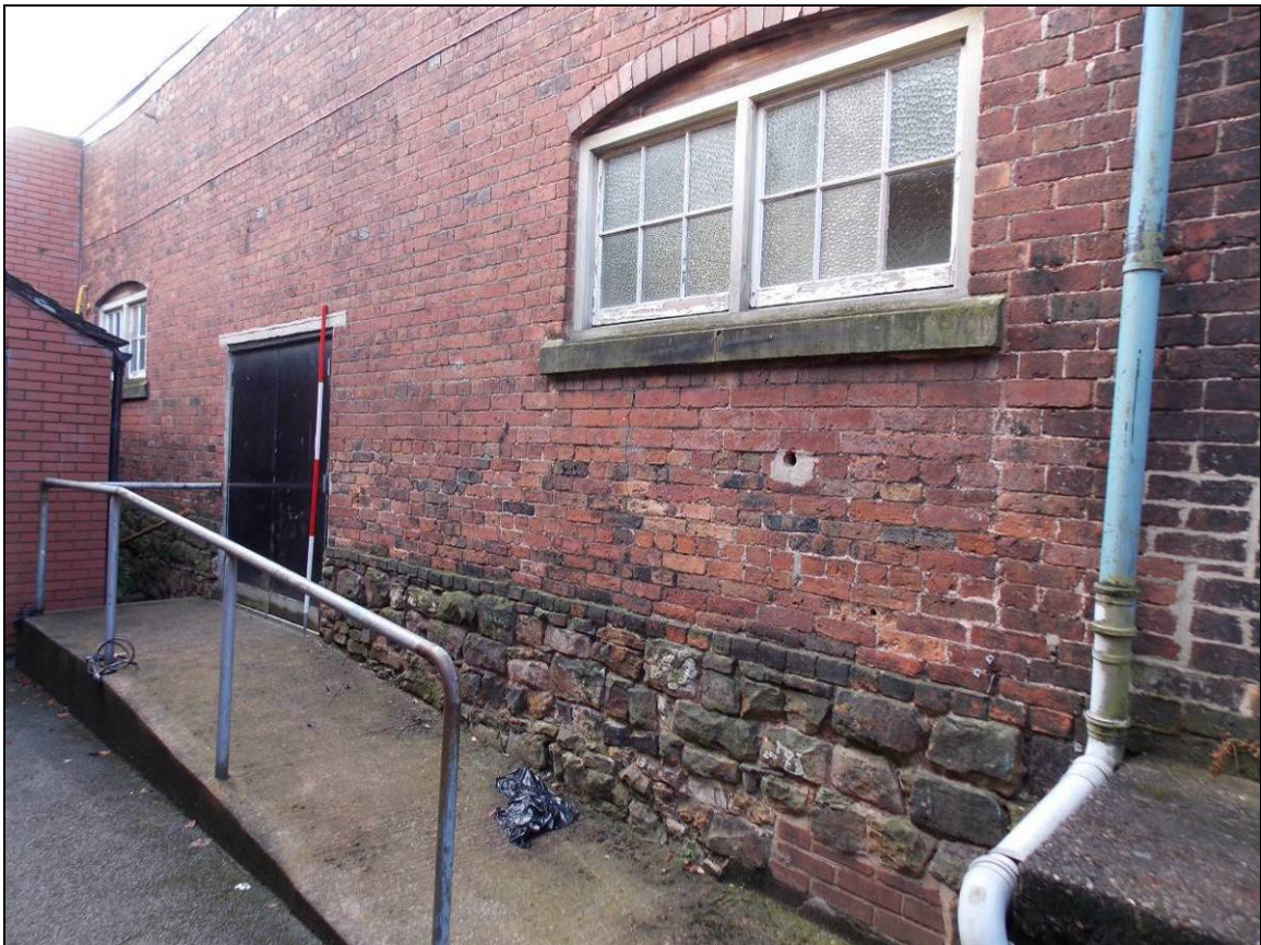
Plate 17: Northern side of the east elevation, looking south (scale 2m).
