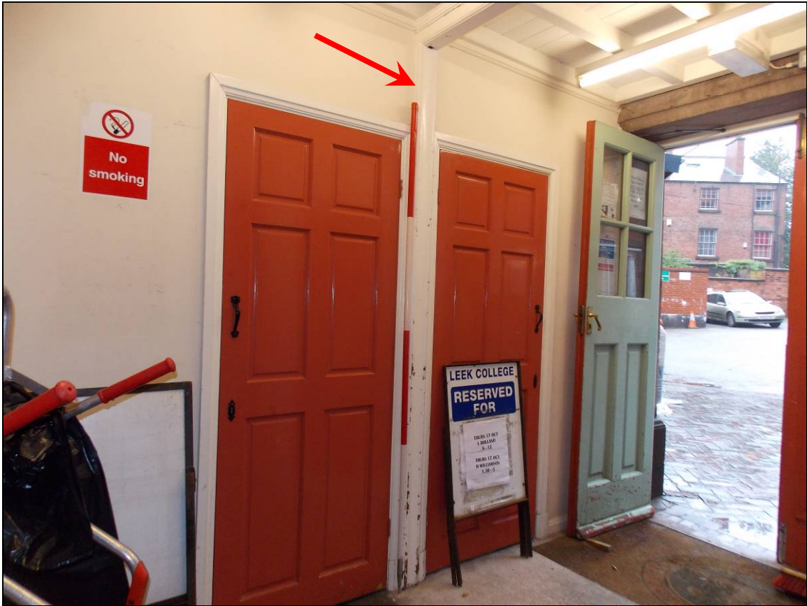
Plate 20: The lobby and doorway frame of a former swinging door (arrow), looking south (scale 2m).
