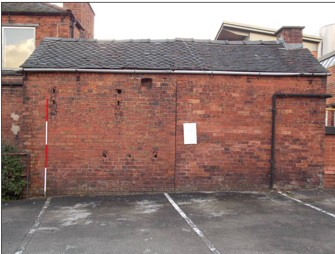
Plate 60: West elevation of the southern extension (scale 2m).
