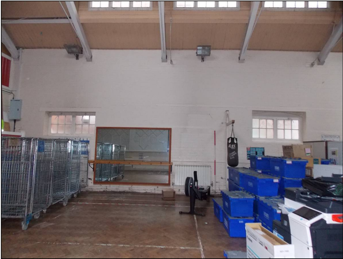
Plate 40: West wall (scale 2m).
