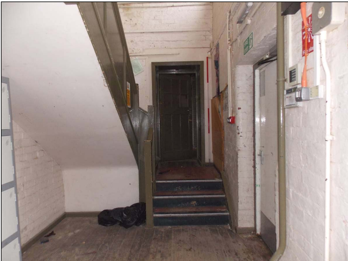
Plate 91: First floor's lobby, looking south (scale 2m).
