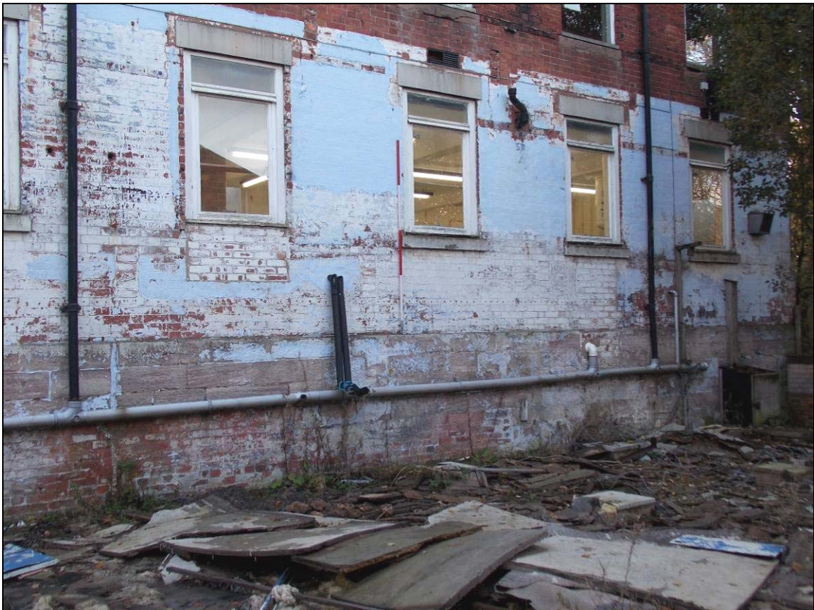
Plate 63: Detail of stone plinth and bricked-up openings, looking north-west (scale 2m).
