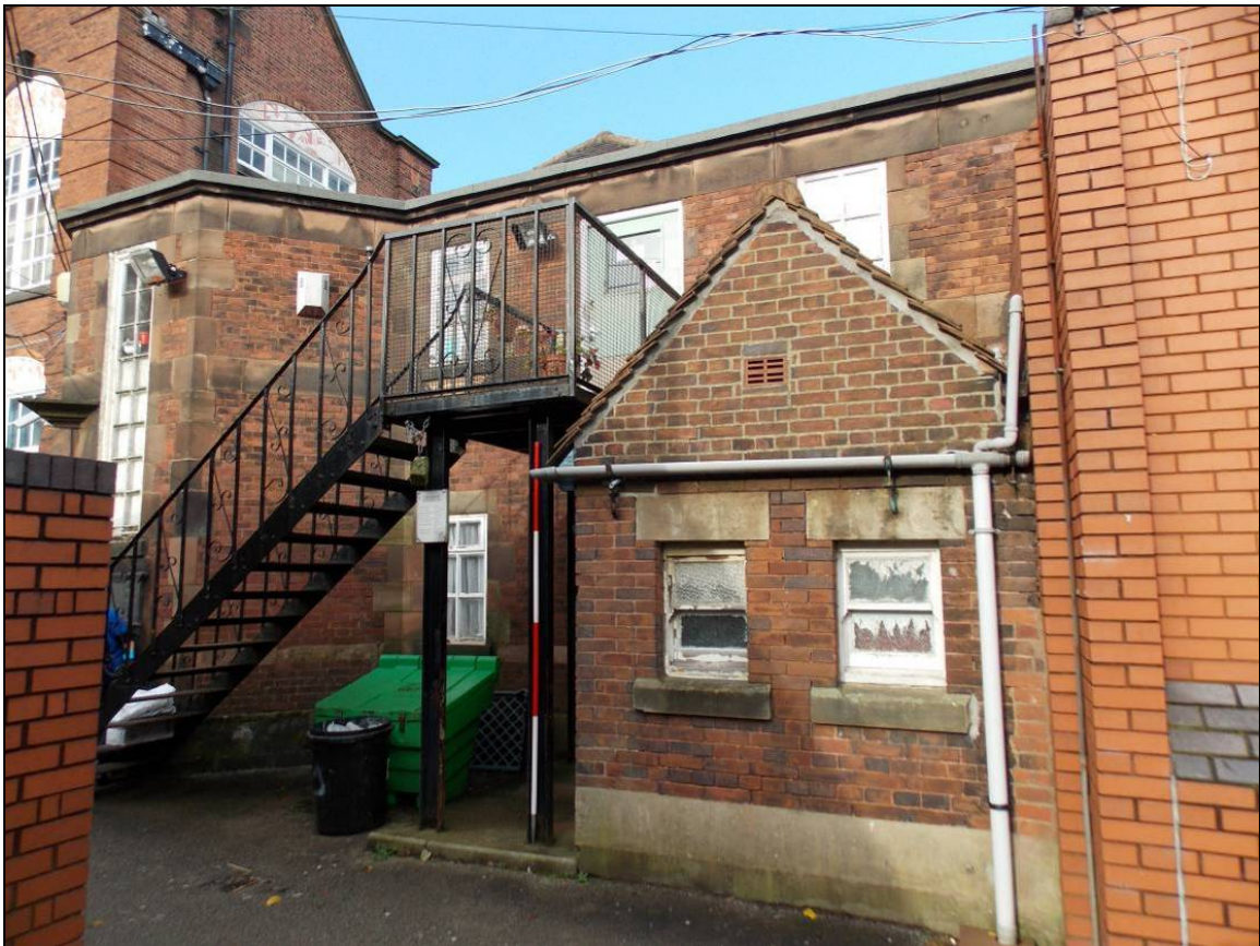
Plate 7: Later extension, looking north-west (scale 2m).
