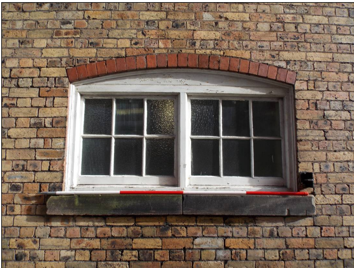
Plate 10: Detail of window openings (scale 2m).
