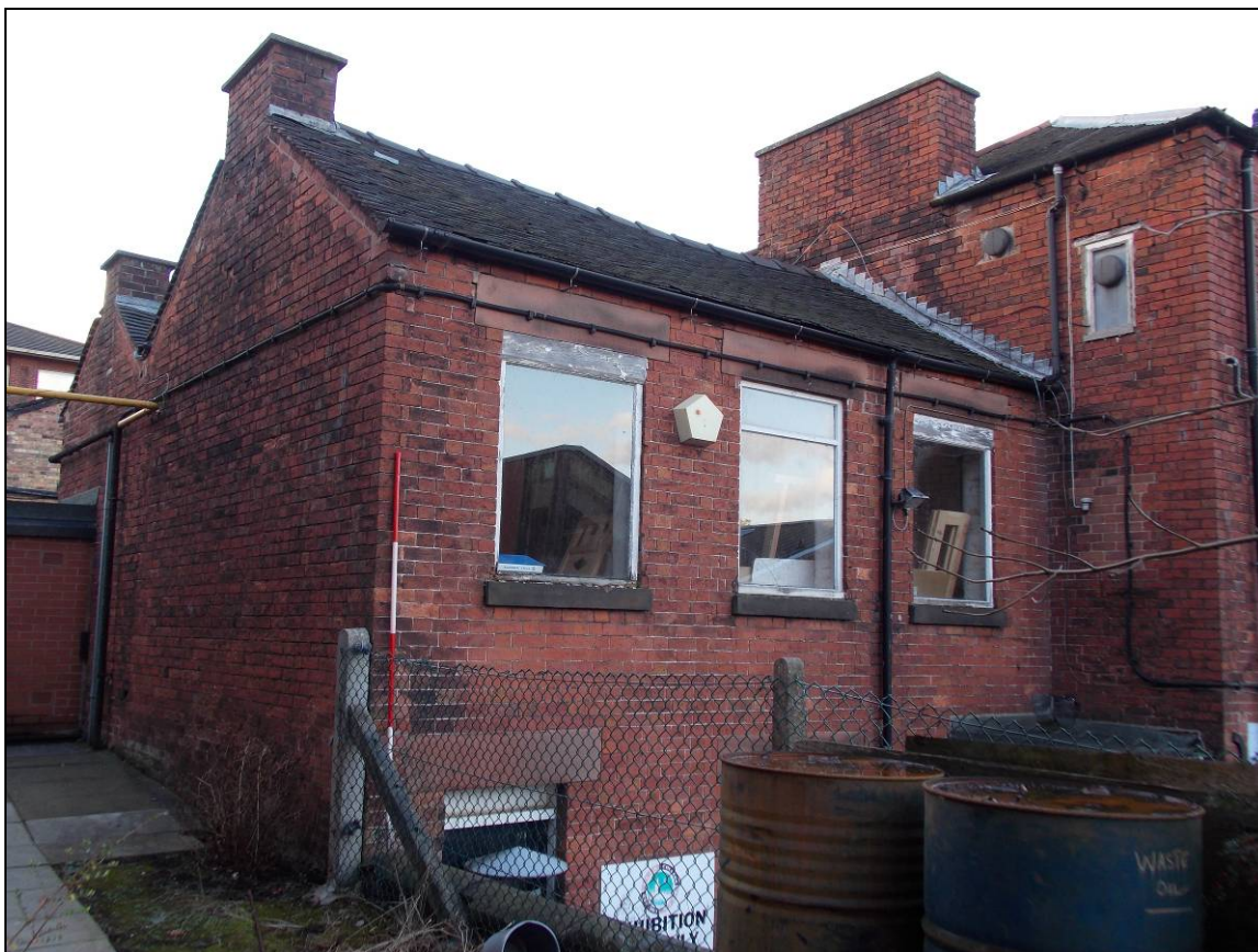
Plate 66: South elevation of the later extension abutting the Mill, looking north-west (scale 2m).
