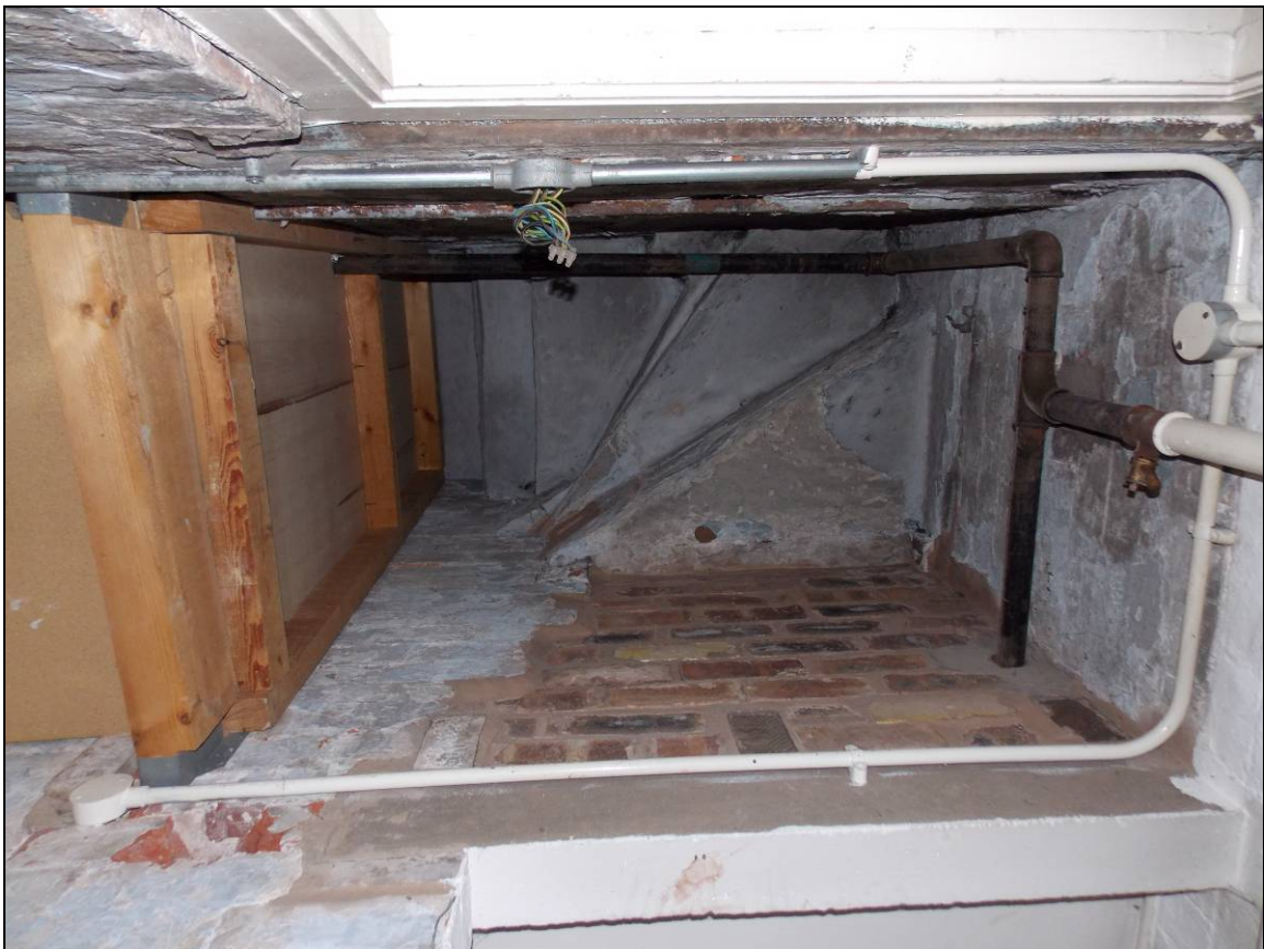
Plate 82: Stairwell with upper section of the original staircase.
