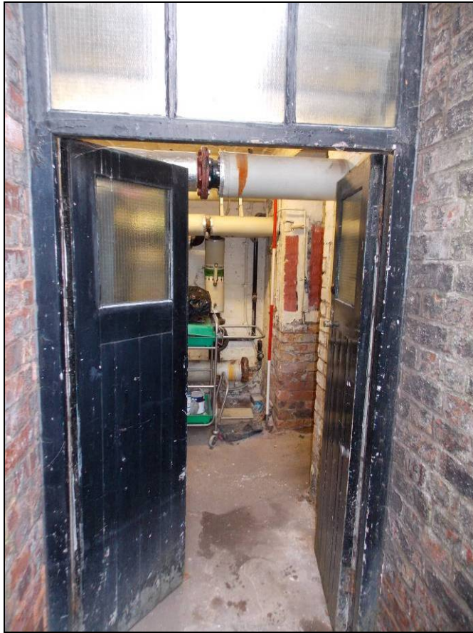
Plate 46: Doorway to the underground boiler room, looking south (scale 2m).
