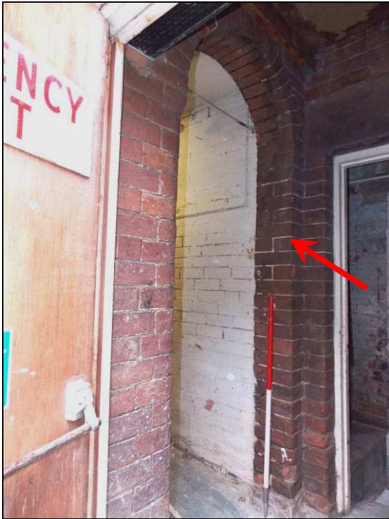
Plate 83: Arched doorway with mason's mark (arrow) along the brick jamb (scale 1m).
