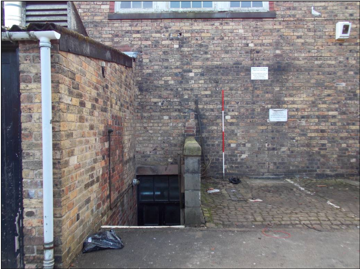
Plate 14: Staircase to the boiler room (scale 2m).
