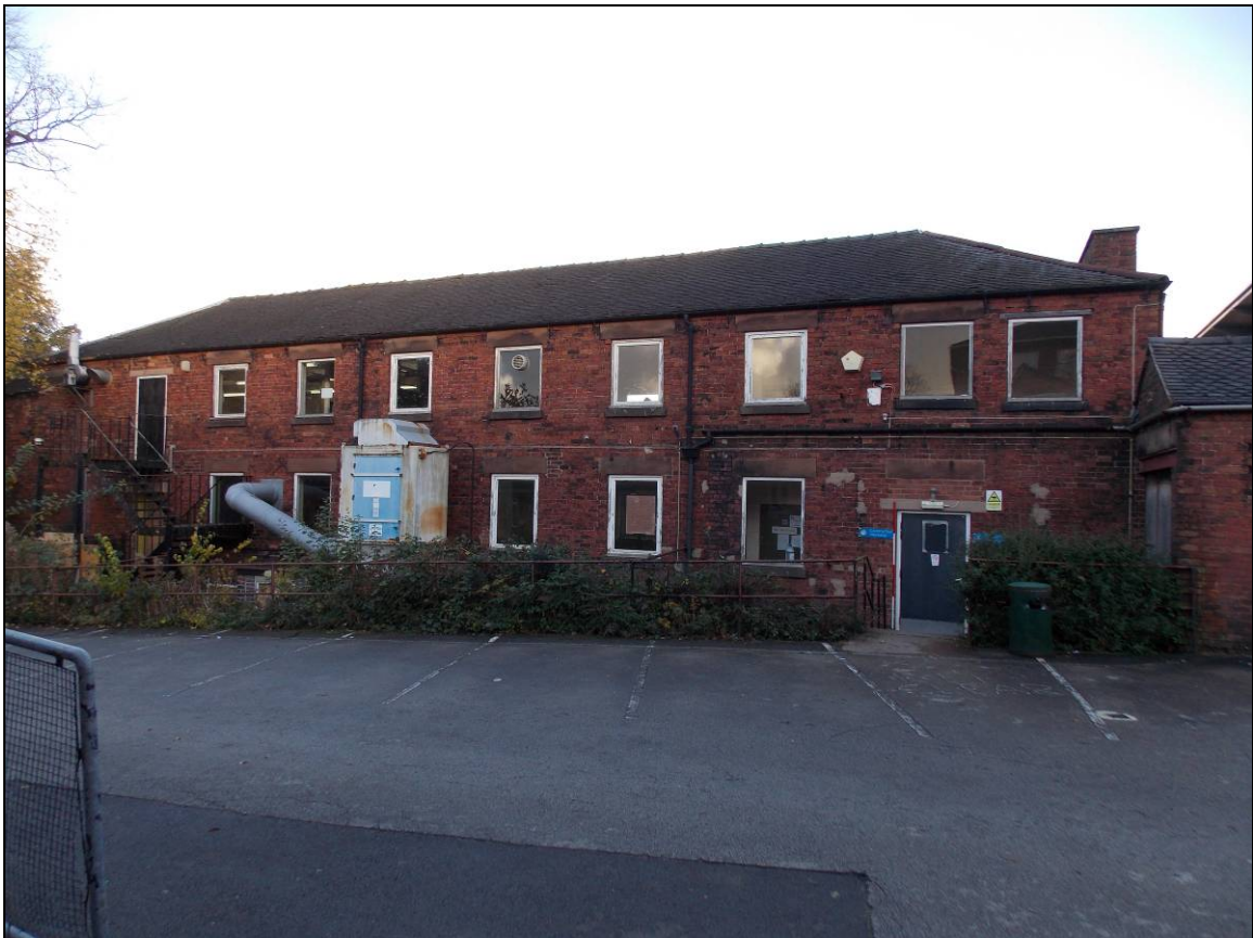
Plate 49: West elevation of the Mill (scale 2m).
