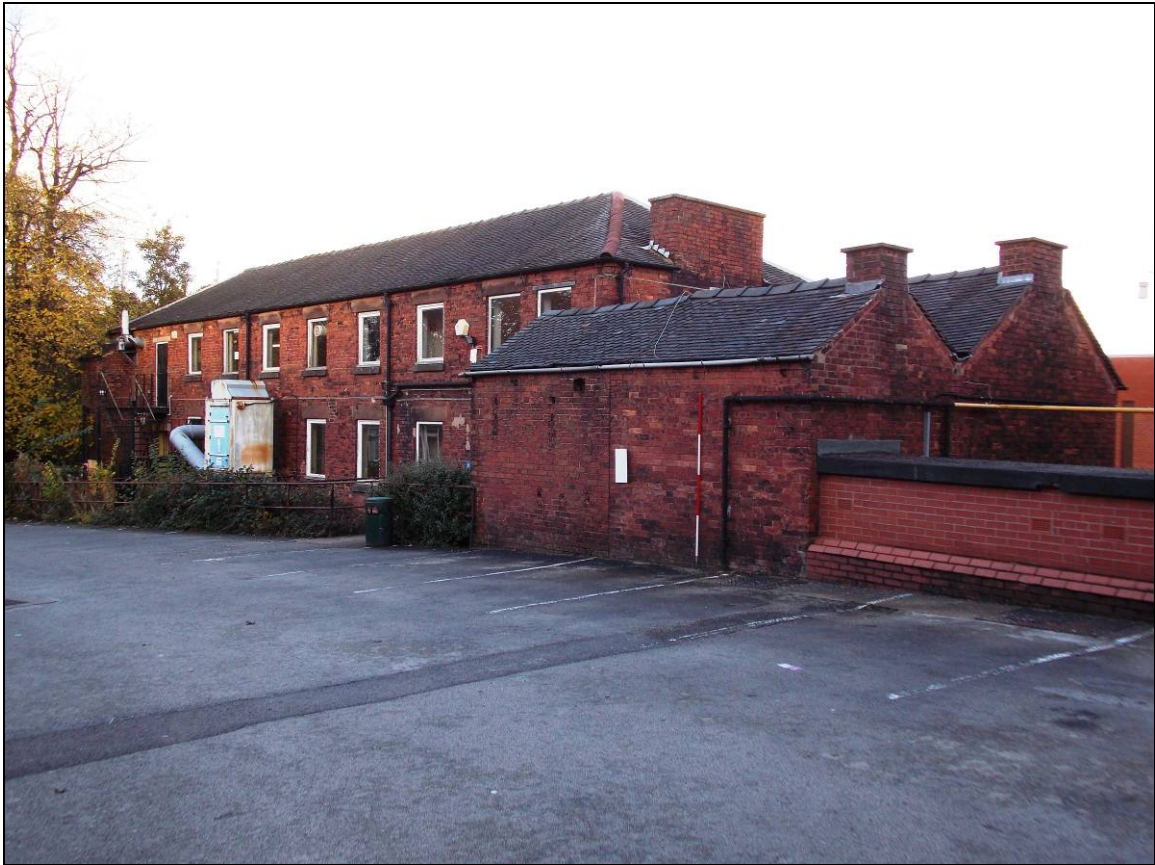
Plate 48: The Mill with a later southern extension on the foreground, looking north-east (scale 2m).
