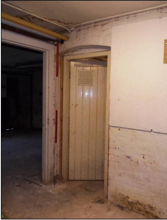
Plate 89: Doorway to the south-western room, looking south-east (scale 2m).
