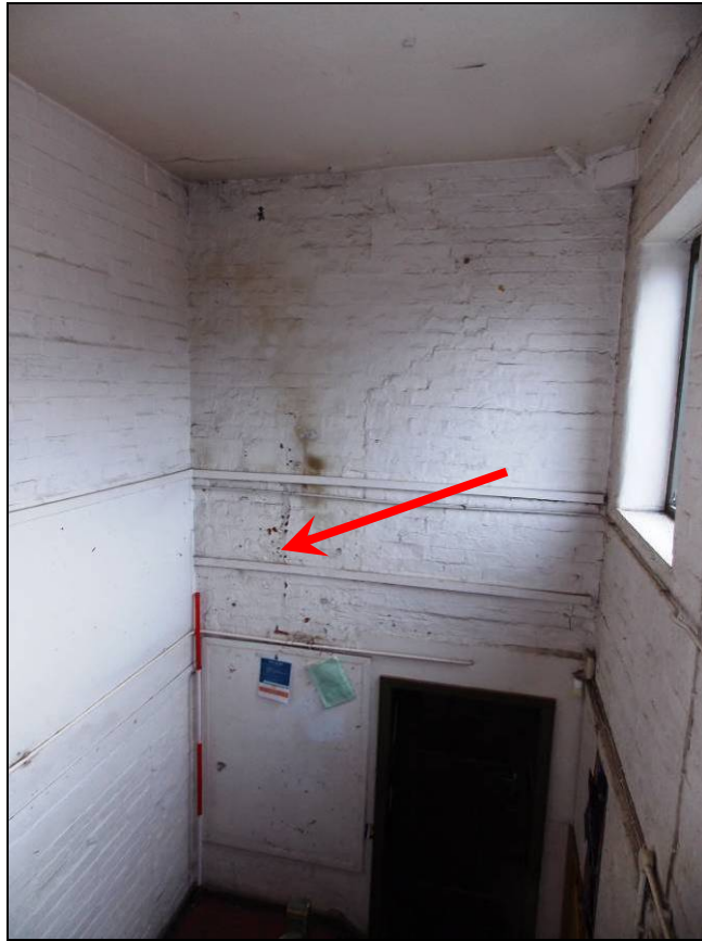
Plate 110: Inserted stairwell with blocked-up fire place (arrow) within the south wall, looking south (scale 2m).
