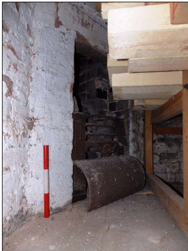
Plate 109: Cast-iron fire place within the south-west corner (scale 300mm).
