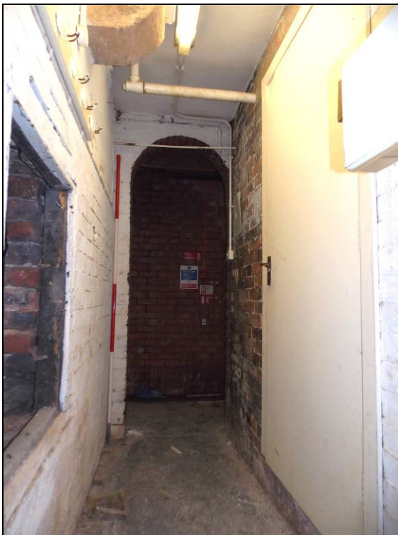
Plate 85: Arched doorway and narrow corridor, looking east (scale 2m).
