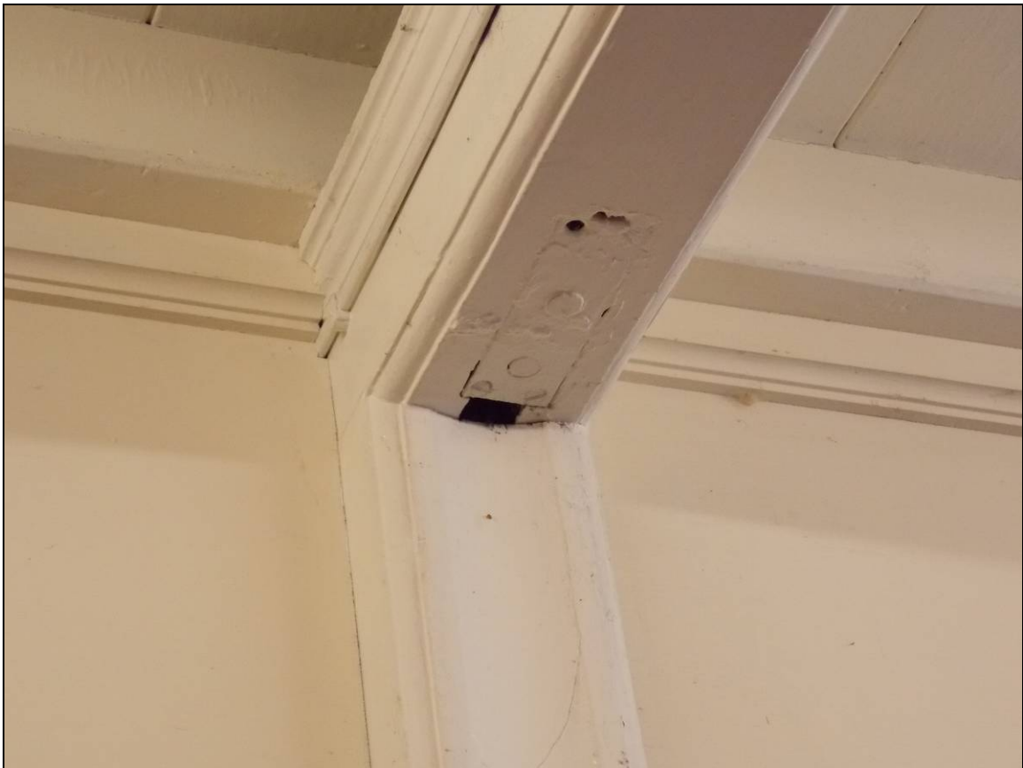
Plate 21: Detail of concave recessed frame and remains of pivoting hinge.
