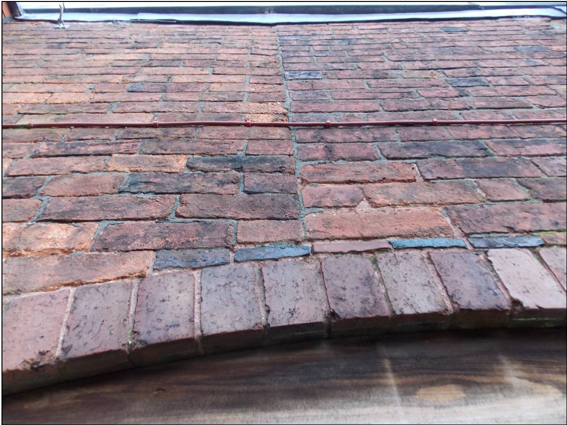
Plate 18: Construction break through the central window opening.
