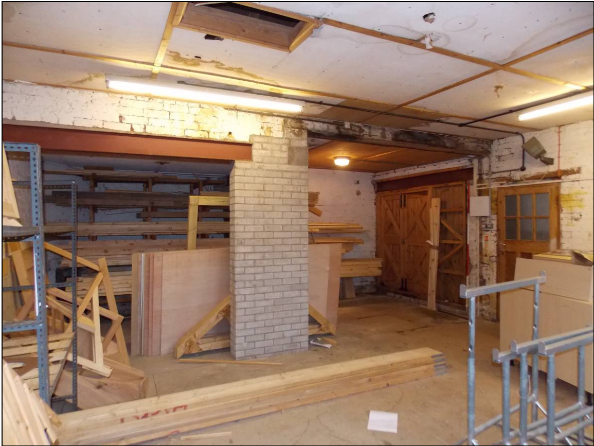
Plate 108: Western side with later insertions (scale 2m).
