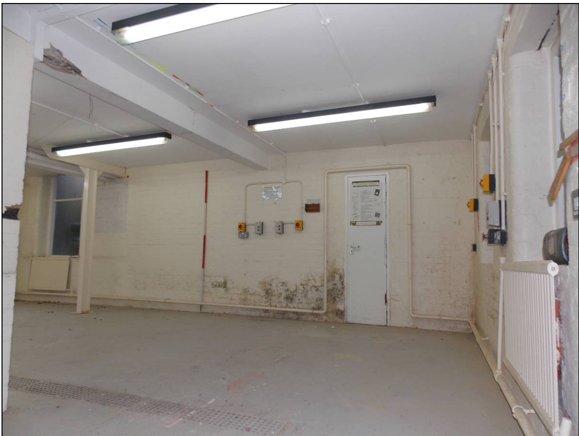
Plate 70: Inserted doorway to the projecting shaft block, looking west (scale 2m).
