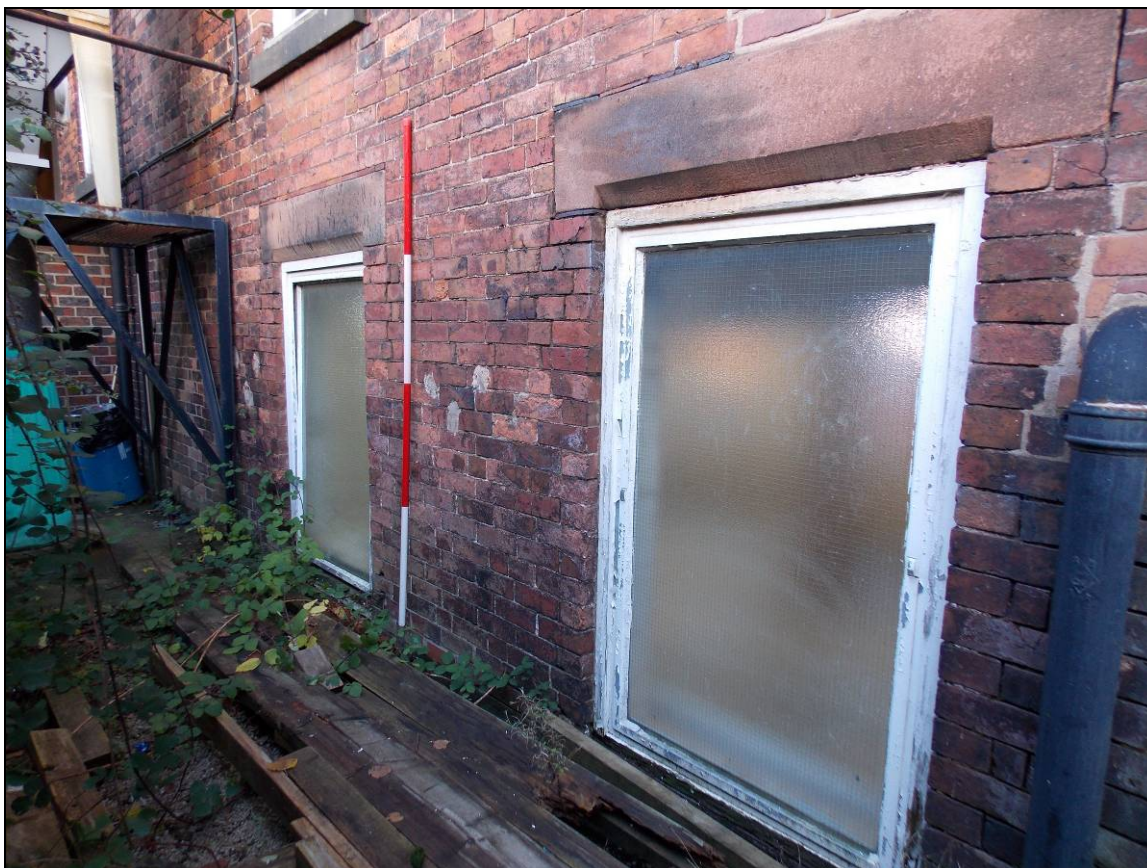
Plate 56: Detail of ground floor's window openings, looking north-east (scale 2m).
