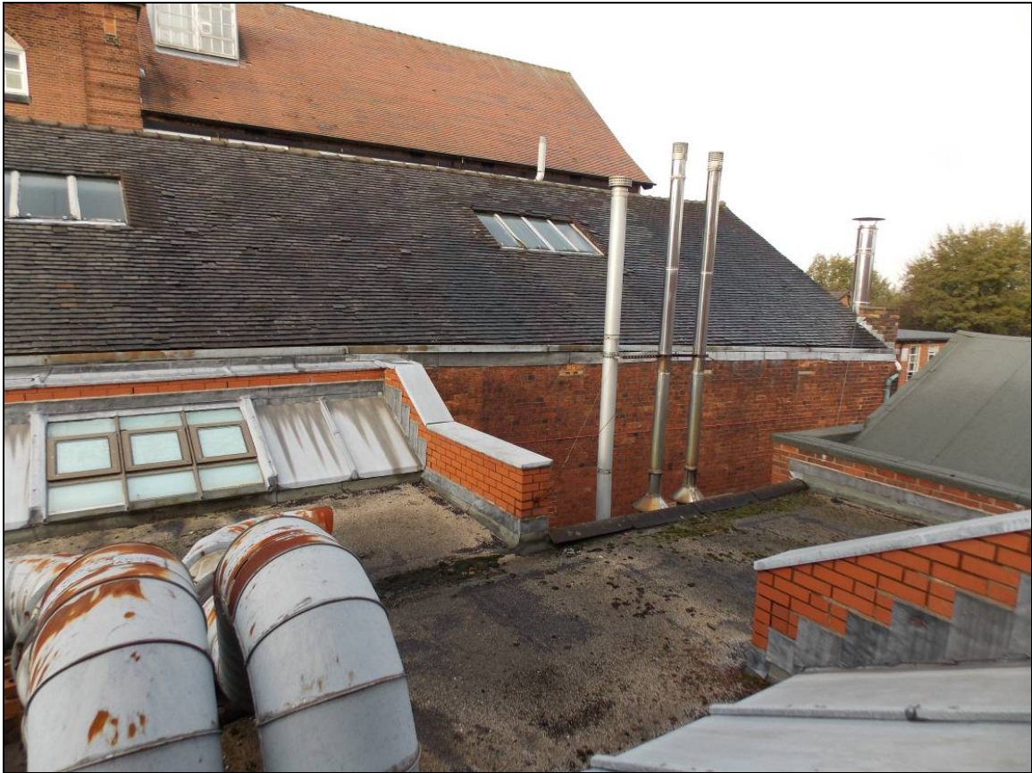
Plate 16: Northern side of the east elevation viewed from adjacent buildings.
