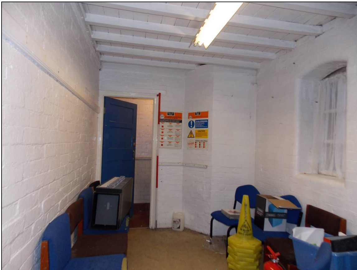
Plate 23: Principal room of the southern unit with a doorway to a lavatory block, looking east (scale 2m).
