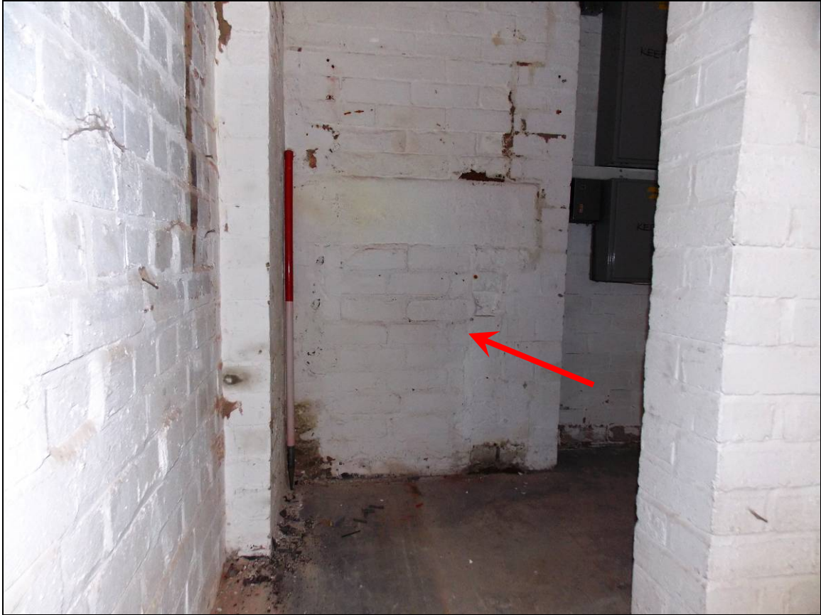
Plate 79: Chimney breast and concealed fire place (arrow) within the western side of the south wall (scale 1m).
