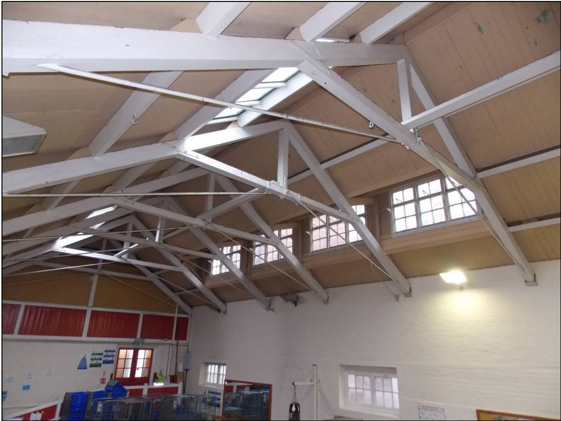
Plate 42: General view of the roof structure, looking south-west.
