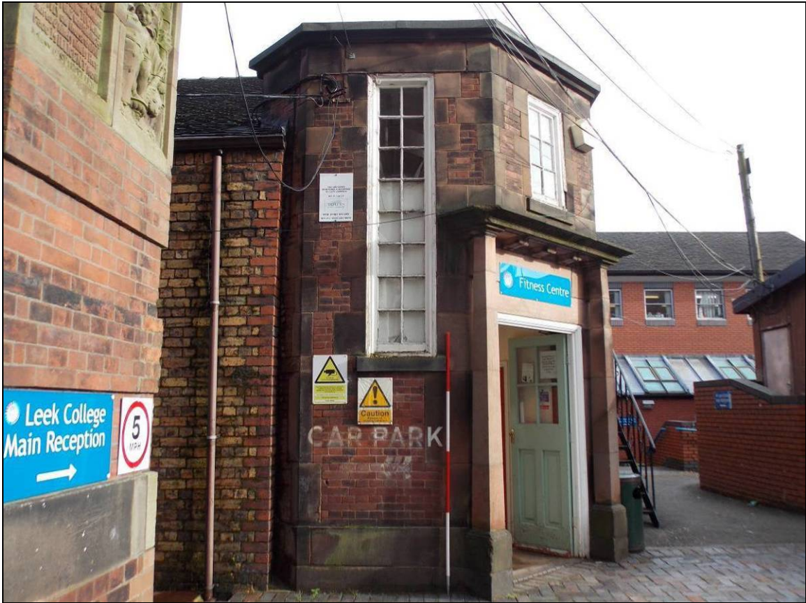
Plate 8: Southern end of the west elevation (scale 2m).
