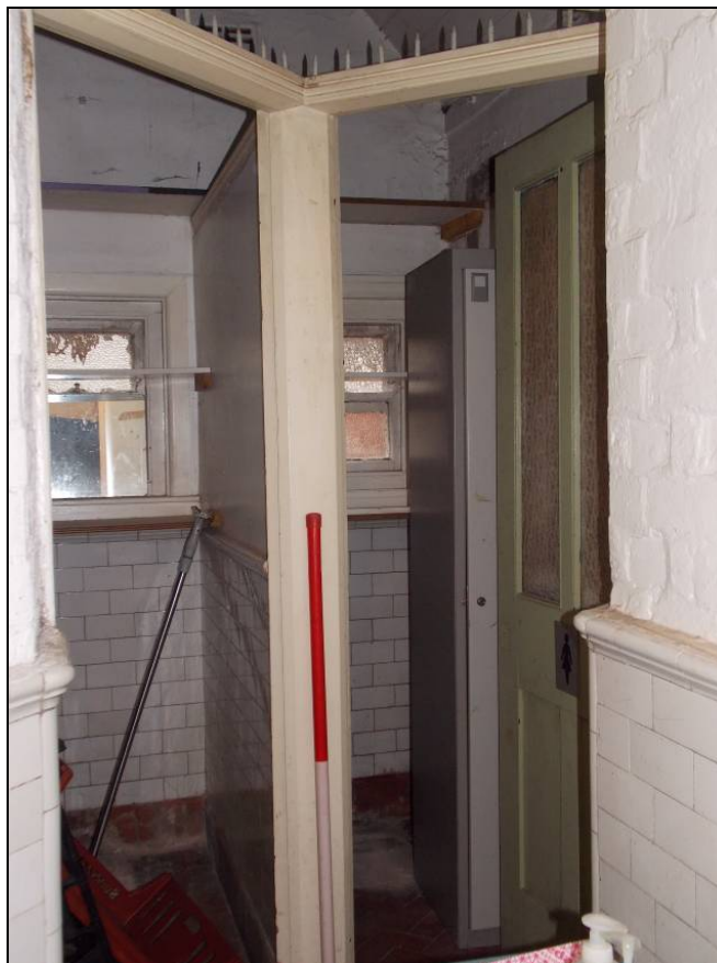
Plate 25: Dividing wall with doorway to the gents and ladies lavatories, looking south (scale 1m).
