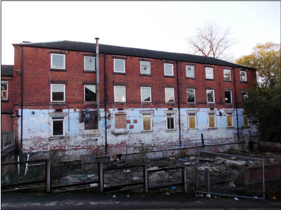
Plate 62: East elevation of the Mill (scale 2m).
