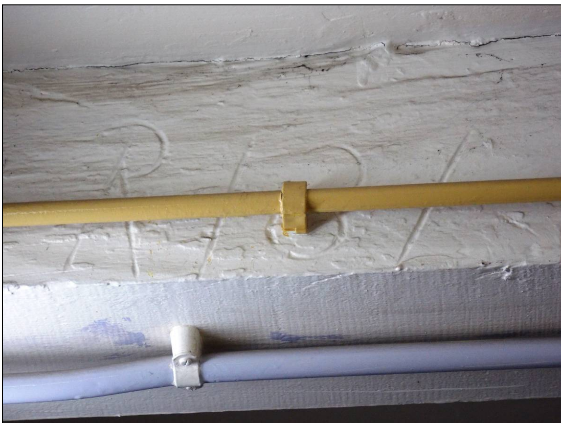
Plate 114: Carpenter's marks within the tie-beam of truss IIII.
