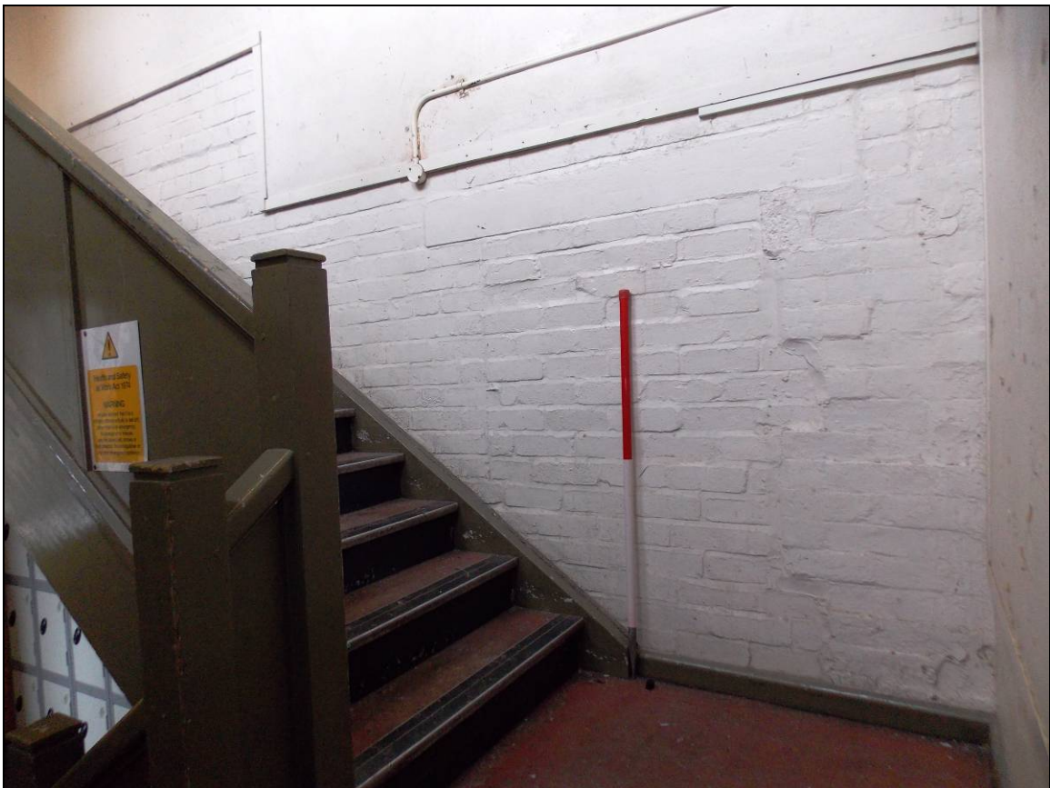
Plate 103: Blocked-up doorway to the southern room, looking east (scale 1m).
