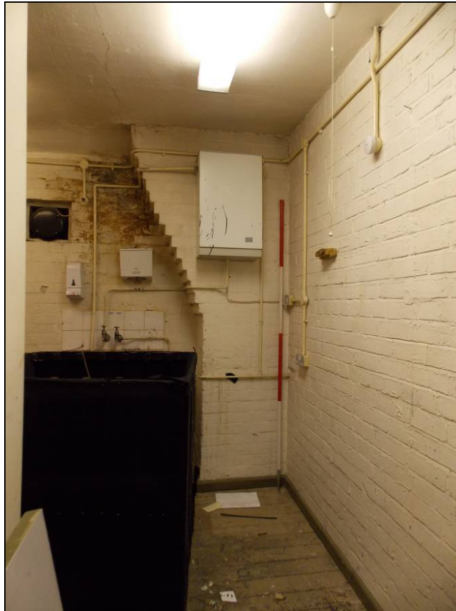
Plate 122: Chimney breast within the south wall (scale 2m).
