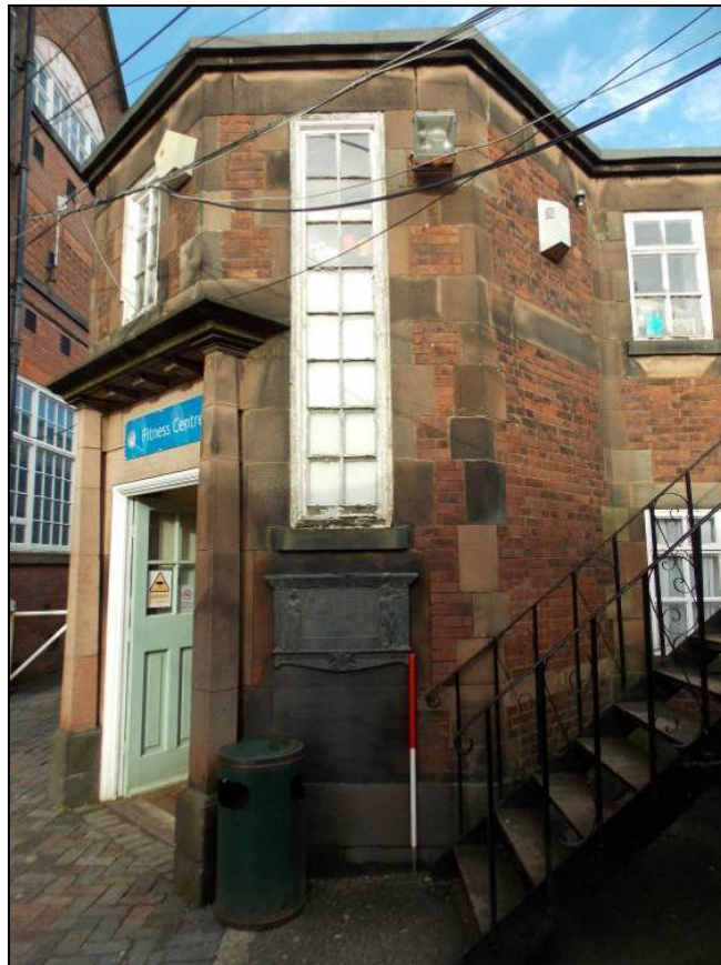
Plate 5: Plaque to the east of the doorway, looking north (scale 1m).
