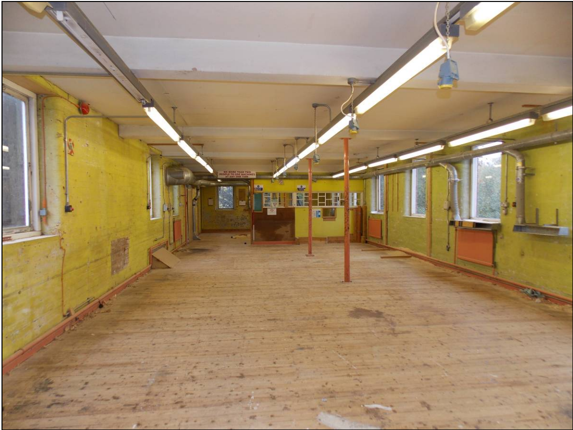
Plate 92: General view of the first floor, looking north (scale 2m).
