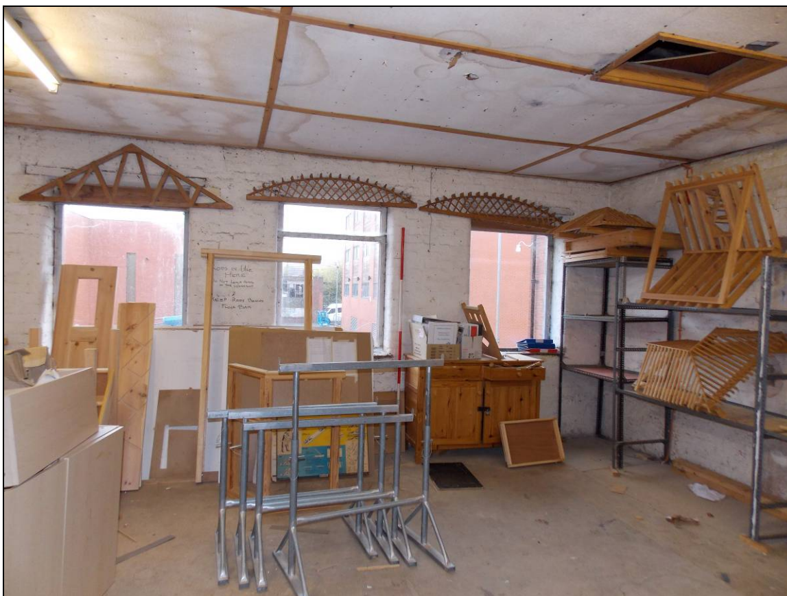
Plate 107: East wall with window openings (scale 2m).
