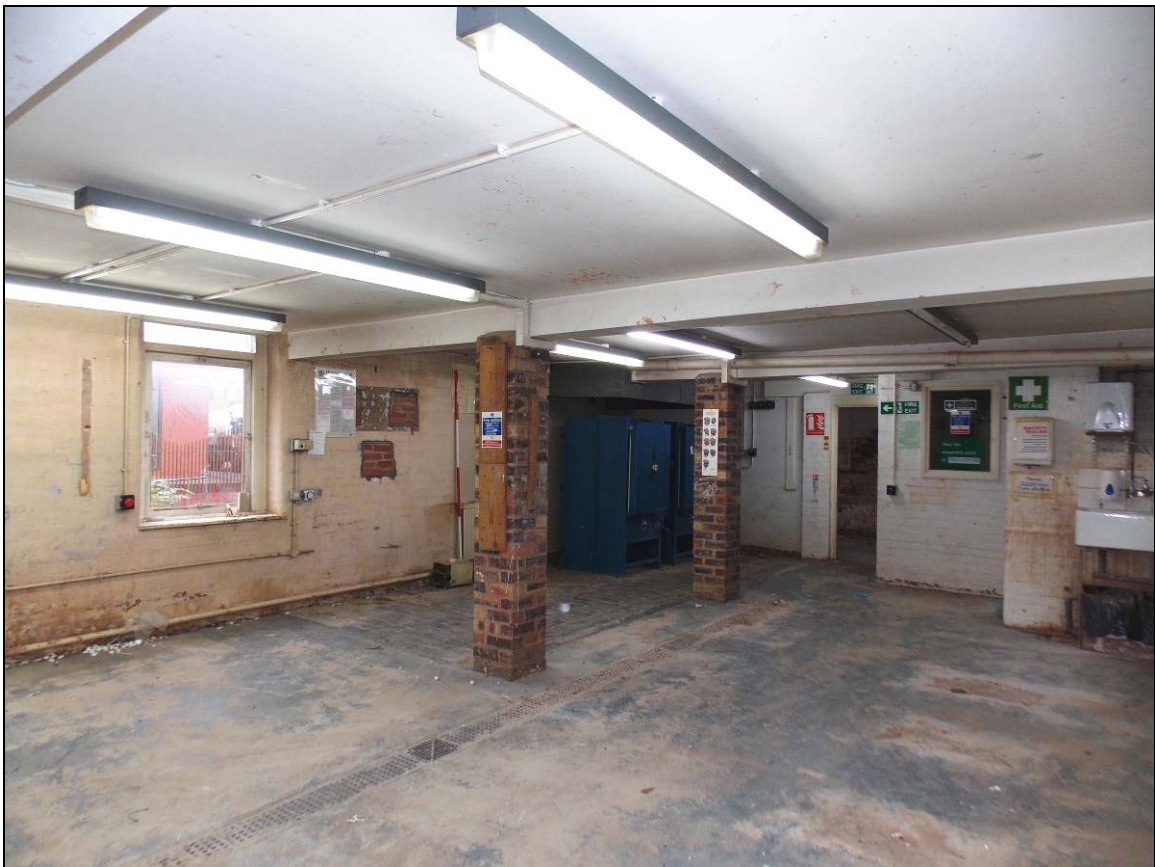
Plate 76: Southern side of the ground floor, looking south-east (scale 2m).
