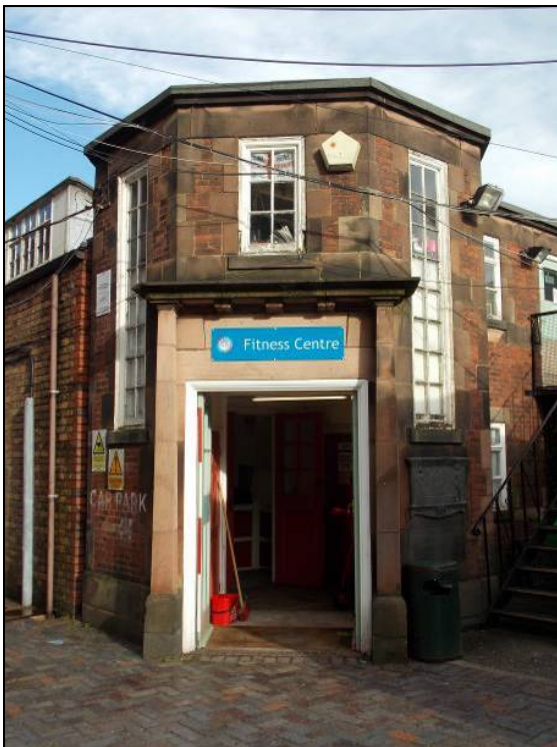
Plate 2: Canted bay with central doorway (scale 2m).
