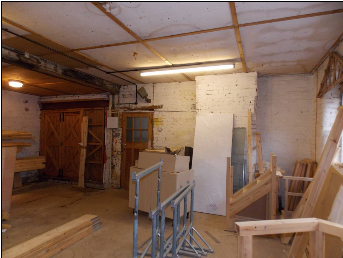
Plate 105: The southern extension with a chimney breast, looking north (scale 2m).
