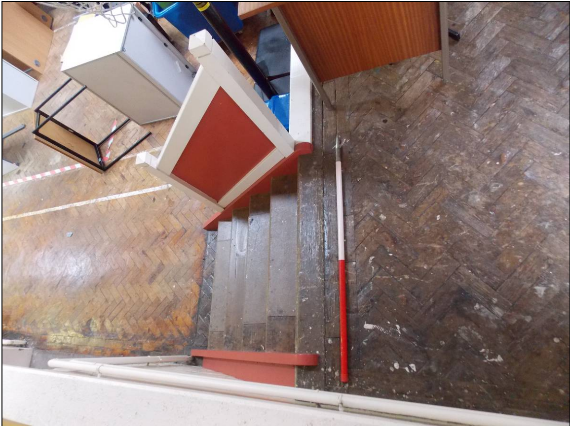
Plate 38: Staircase of the raised platform, looking west (scale 1m).
