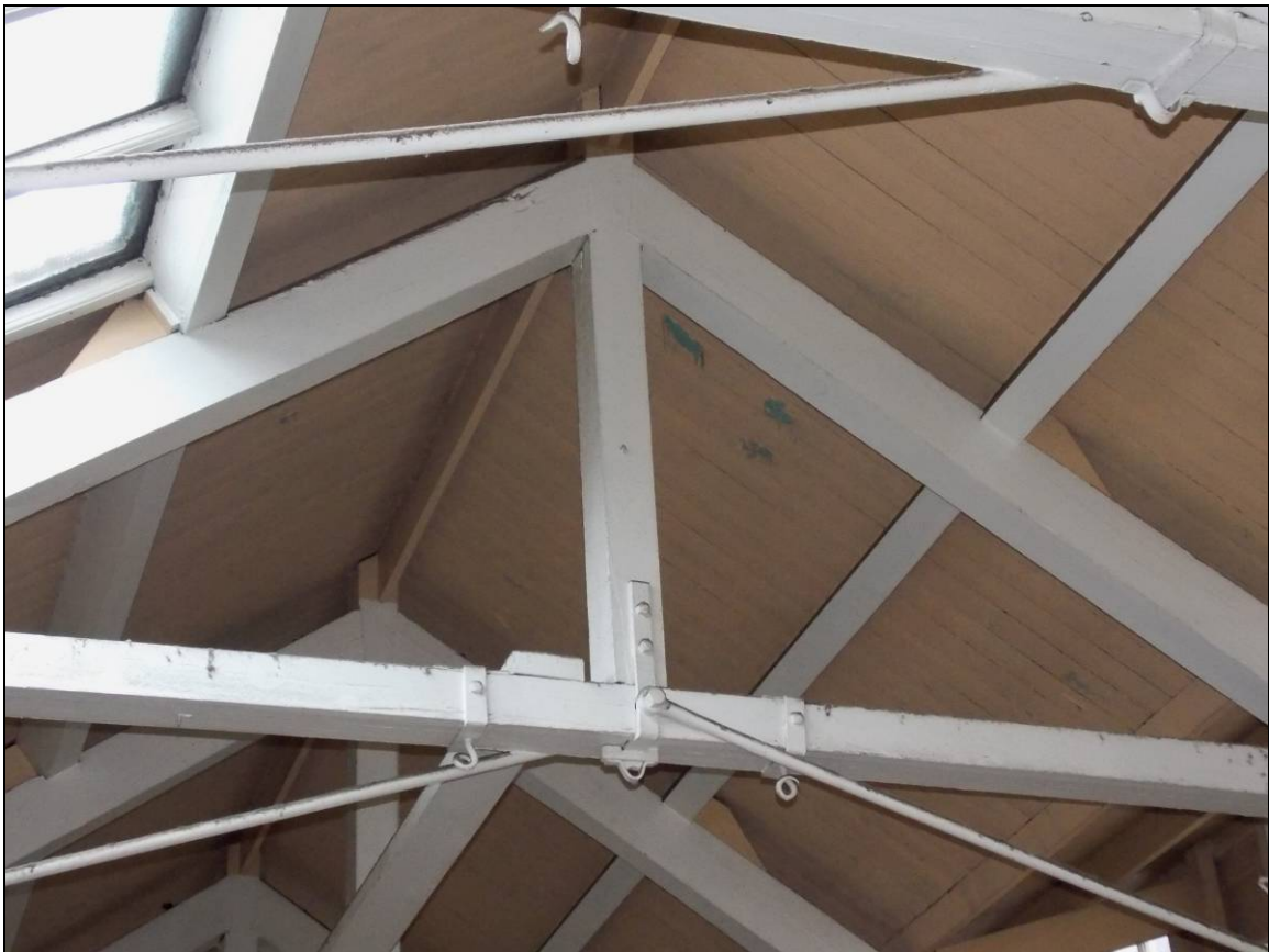
Plate 43: Plate attachment between timber king-post and wrought-iron tension raking struts.
