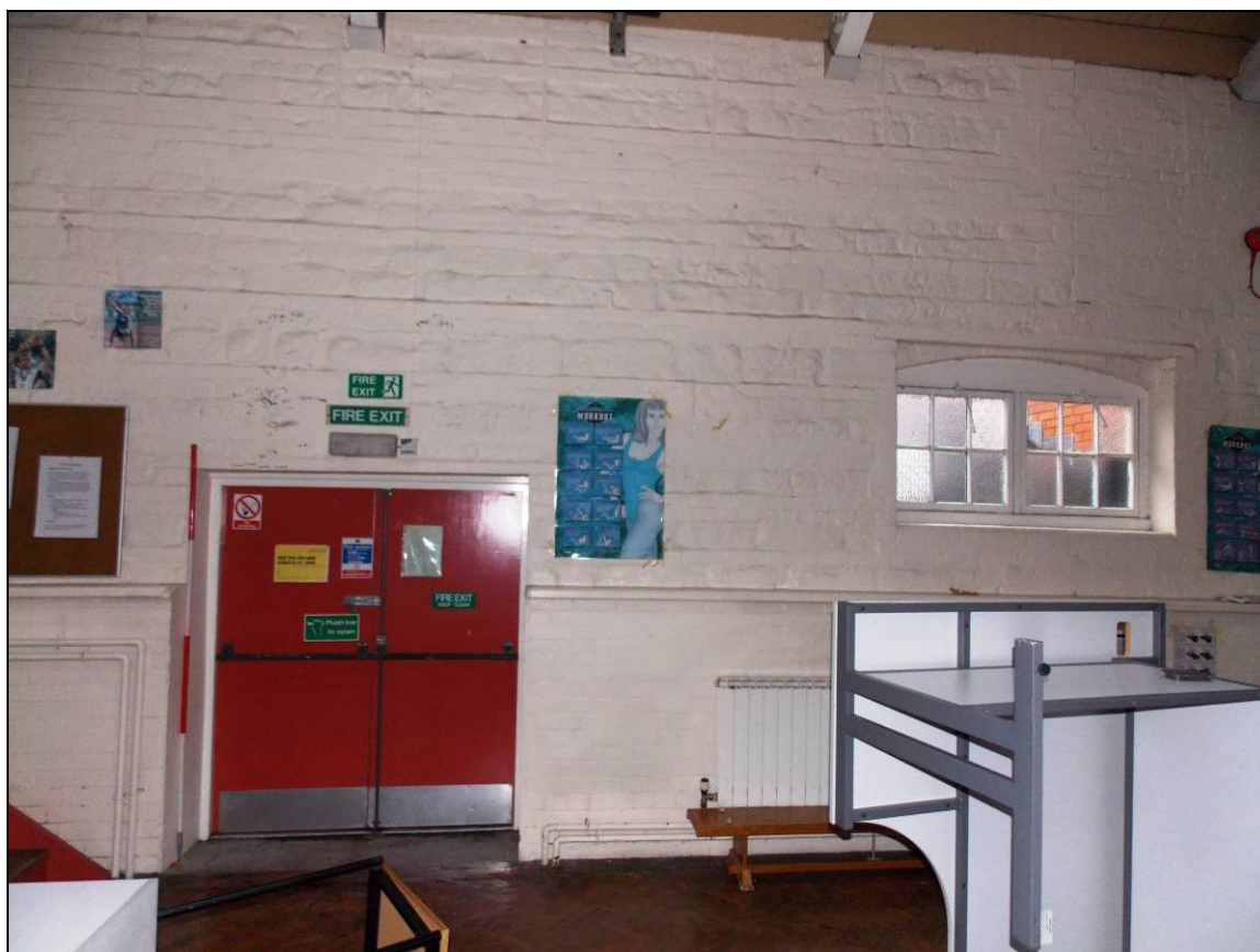
Plate 34: East wall with inserted doorway (scale 2m).
