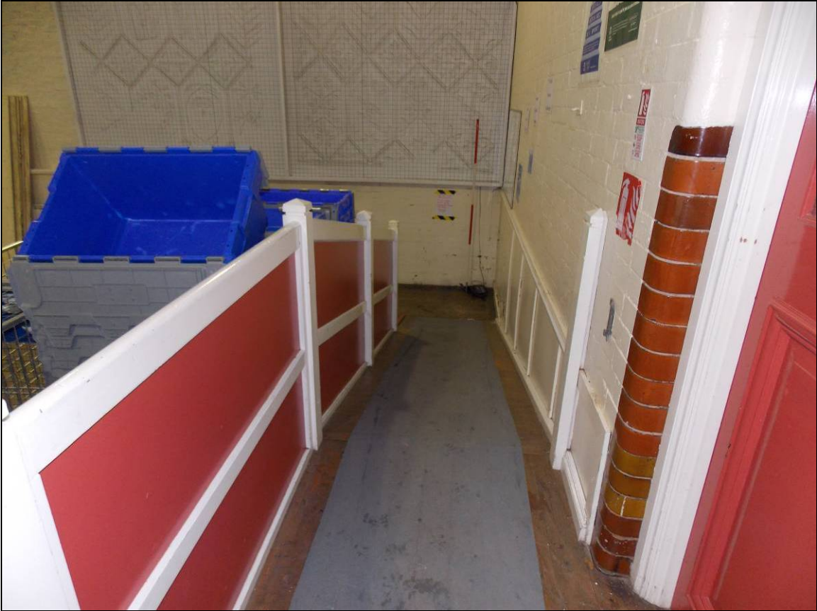
Plate 30: Later ramp along the main doorway, looking east (scale 2m).
