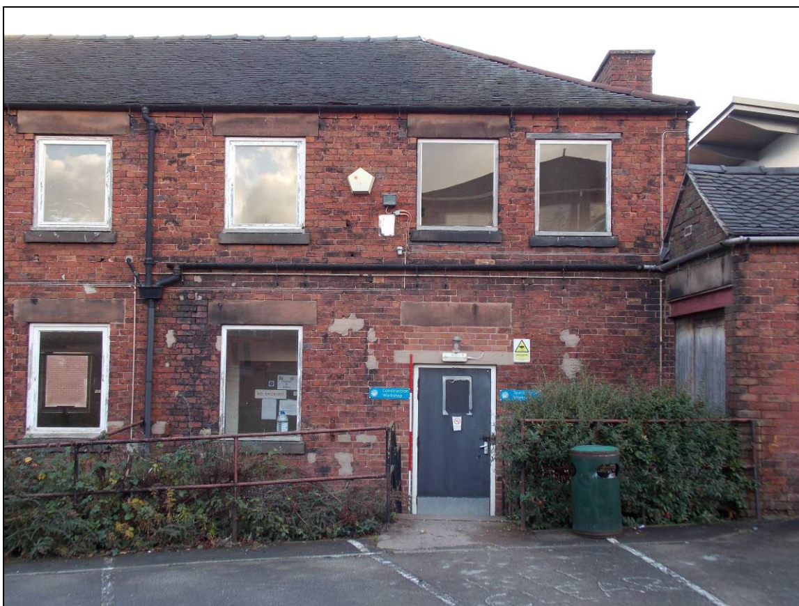
Plate 50: Southern end of the west elevation (scale 2m).
