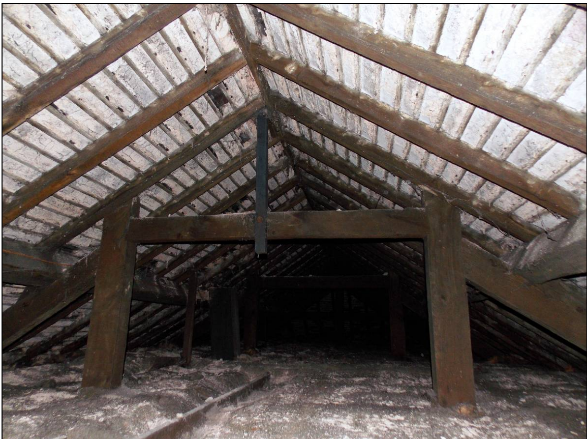
Plate 123: Detail of queen-post truss III, looking north.
