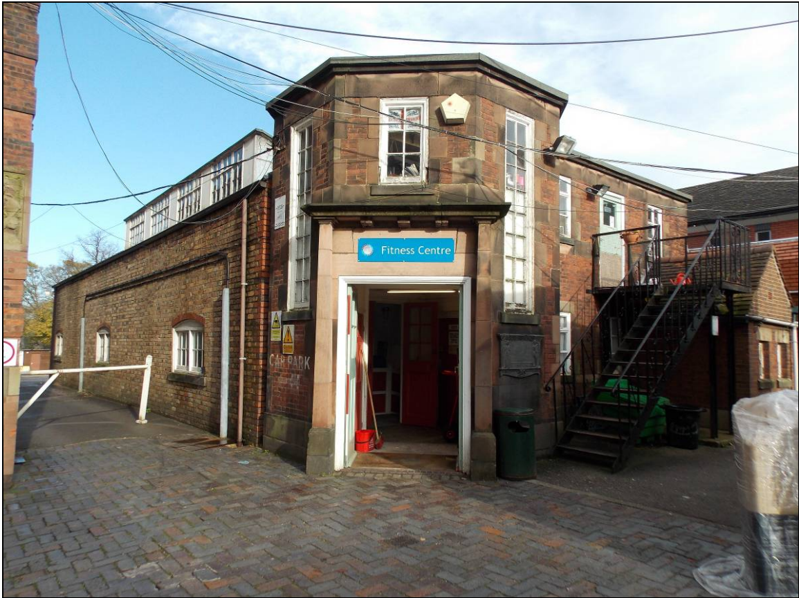
Plate 1: General view of the Carr Gymnasium (scale 2m).
