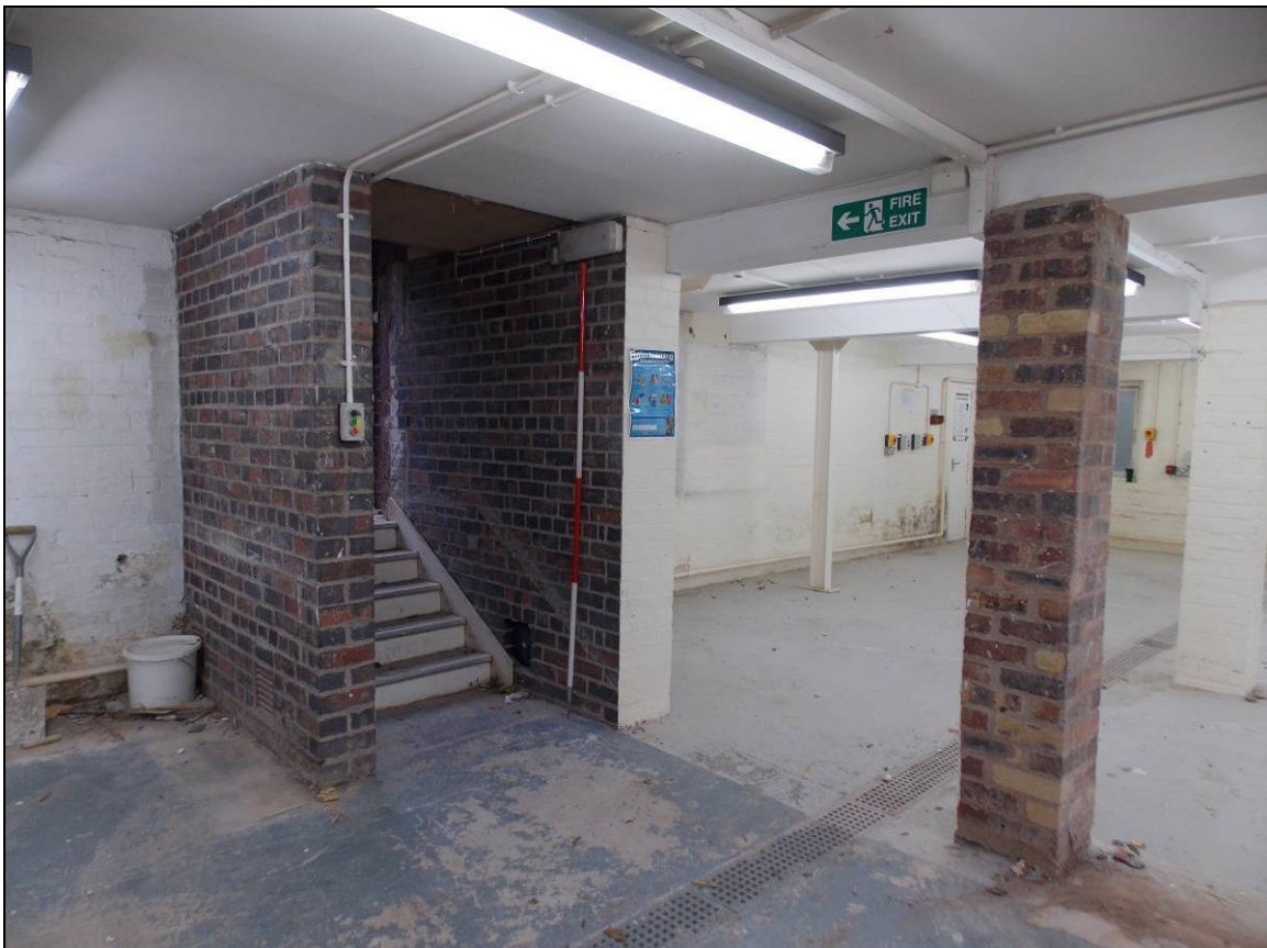
Plate 68: Inserted staircase down to the ground floor, looking north-west (scale 2m).
