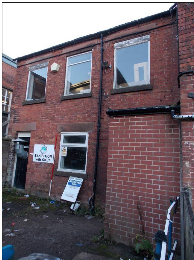
Plate 65: Detail of window openings and doorways, looking south-west (scale 2m).
