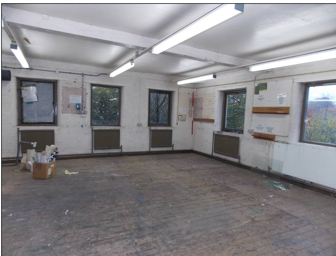
Plate 115: Northern end of the second floor with exposed tie-beam (truss I), looking north (scale 2m).
