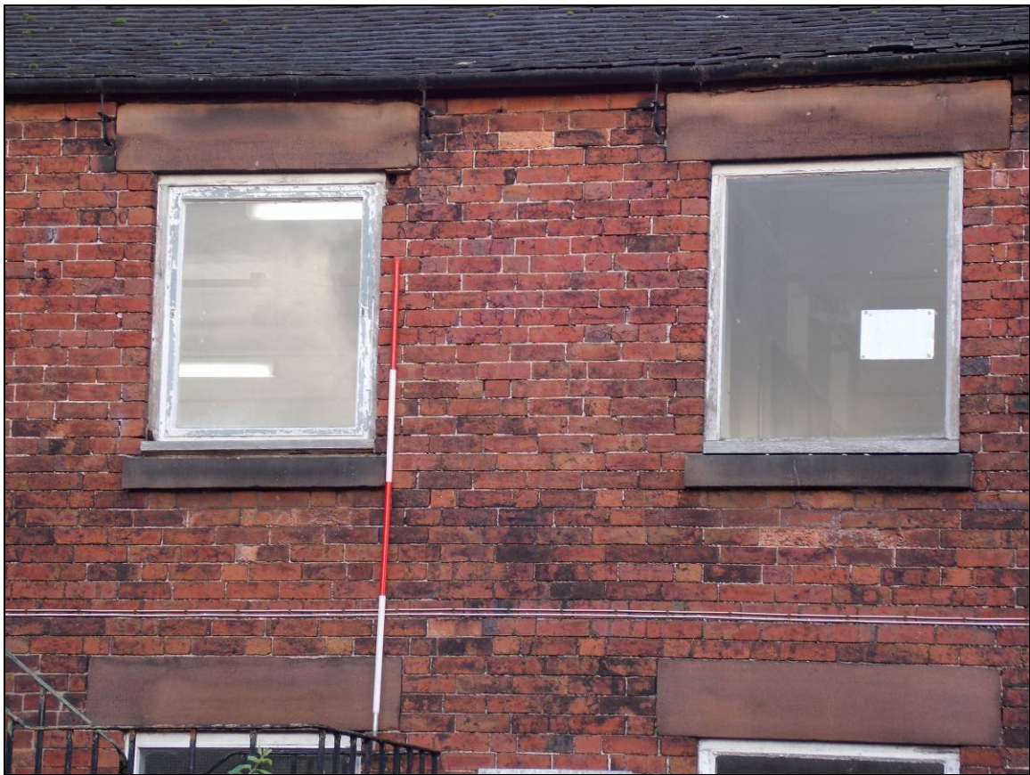
Plate 58: Detail of second floor's window openings (scale 2m).
