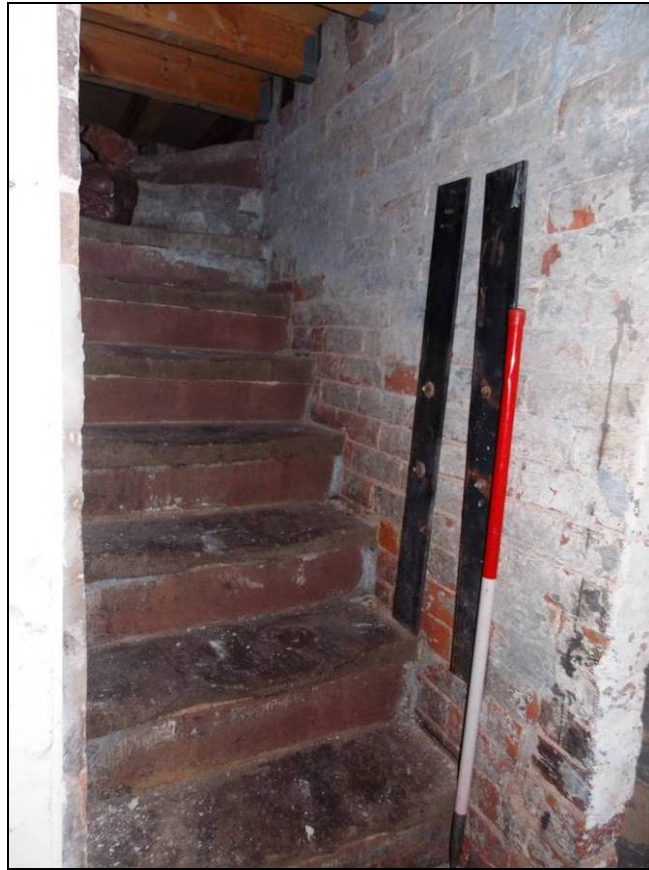
Plate 81: Lower section of the original staircase, looking west (scale 1m).
