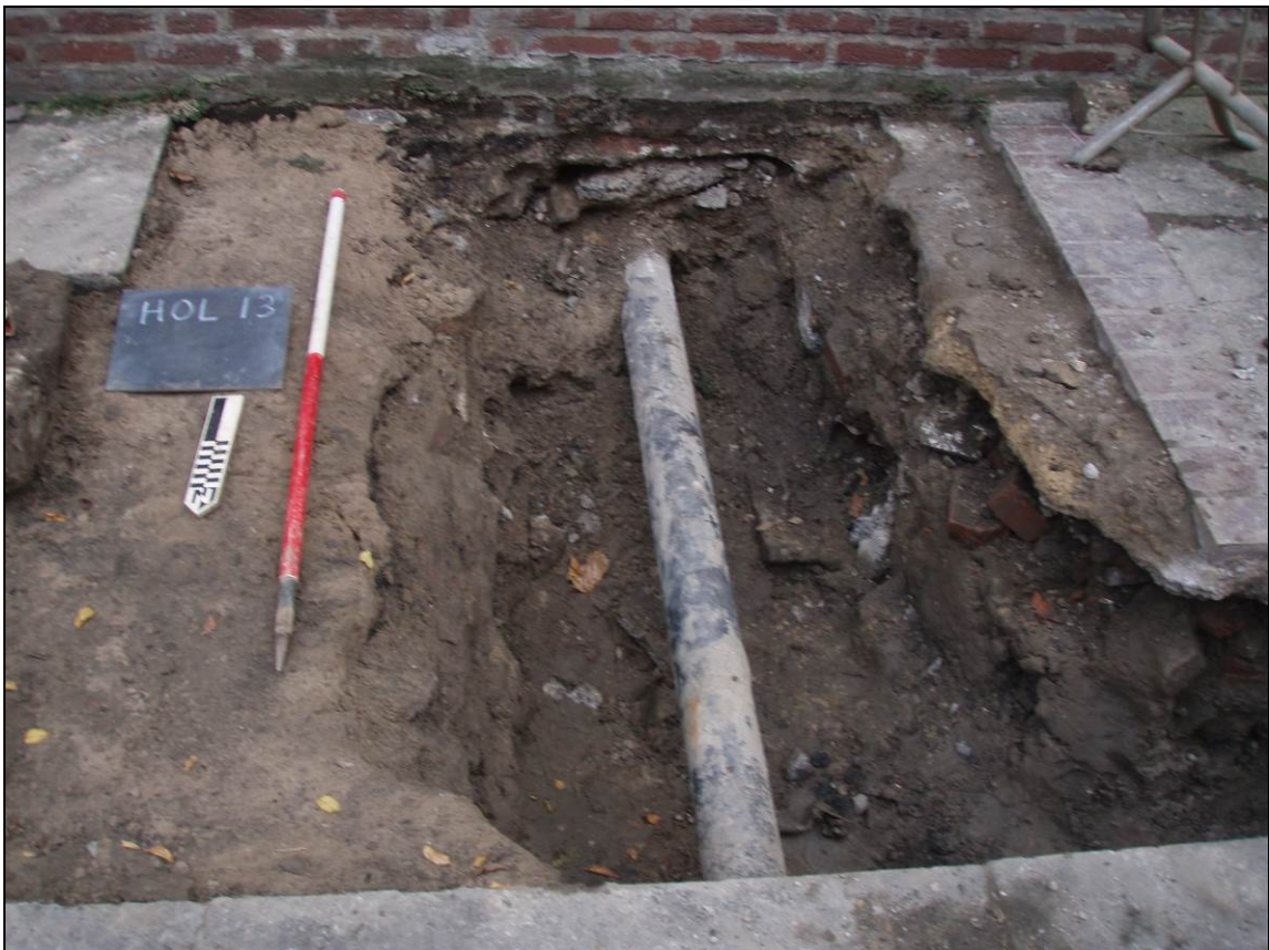
Figure 4. South facing view of Trench 1, showing exposed cast iron pipe. Scale = 1m
