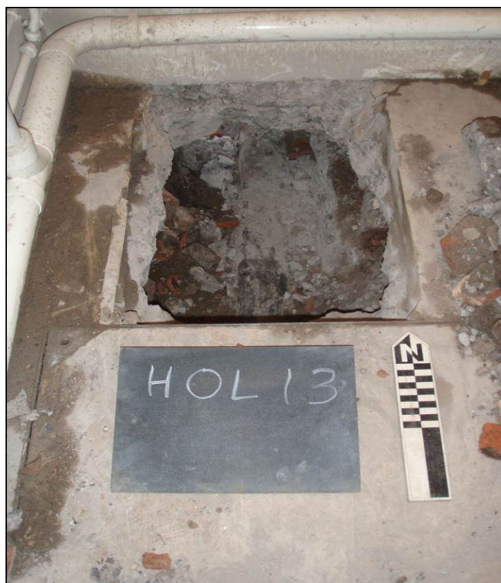
Figure 11. North facing view of Trench 2, showing exposed waste pipe (009).
