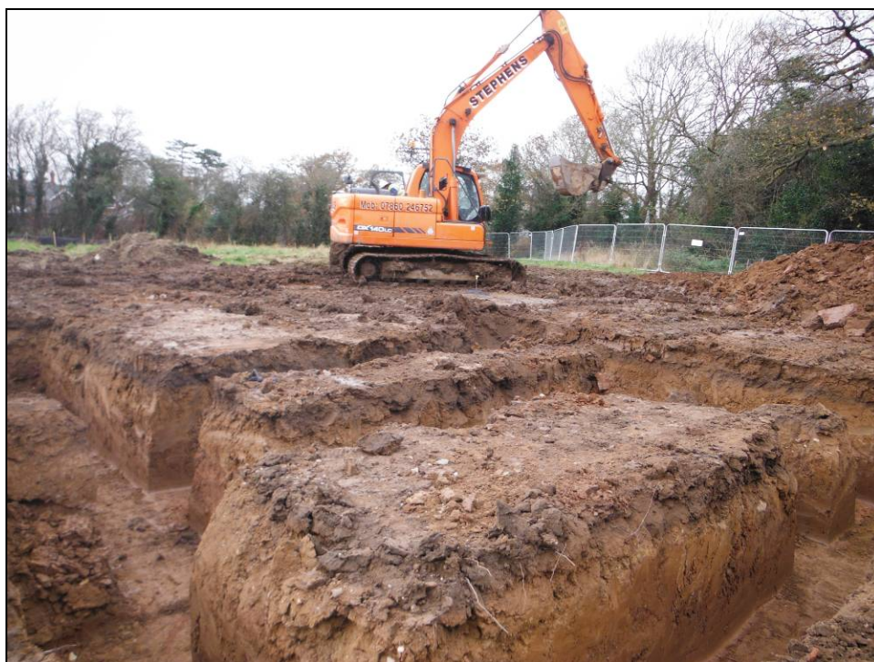
Figure 14. General shot of Plot 35 under excavation.
