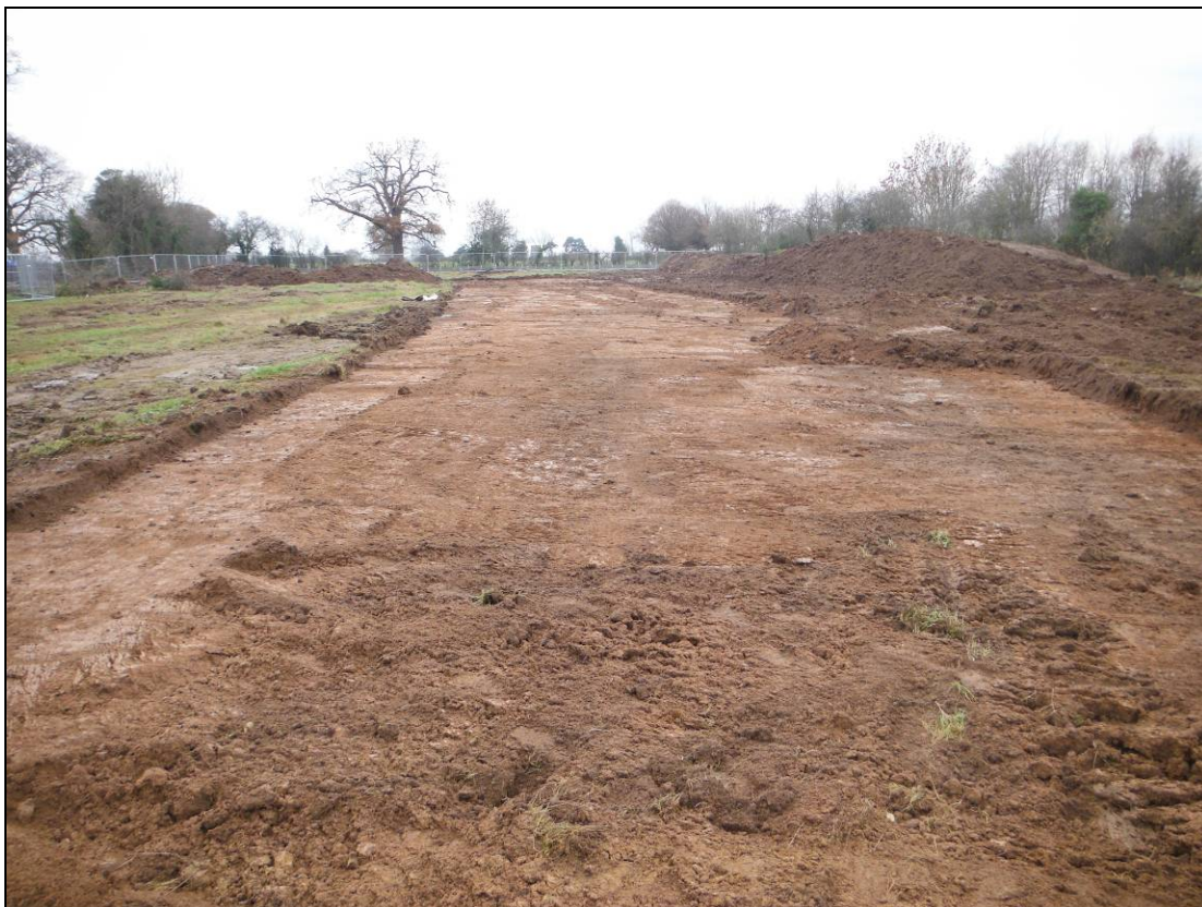
Figure 16. Initial topsoil strip of the access road.
