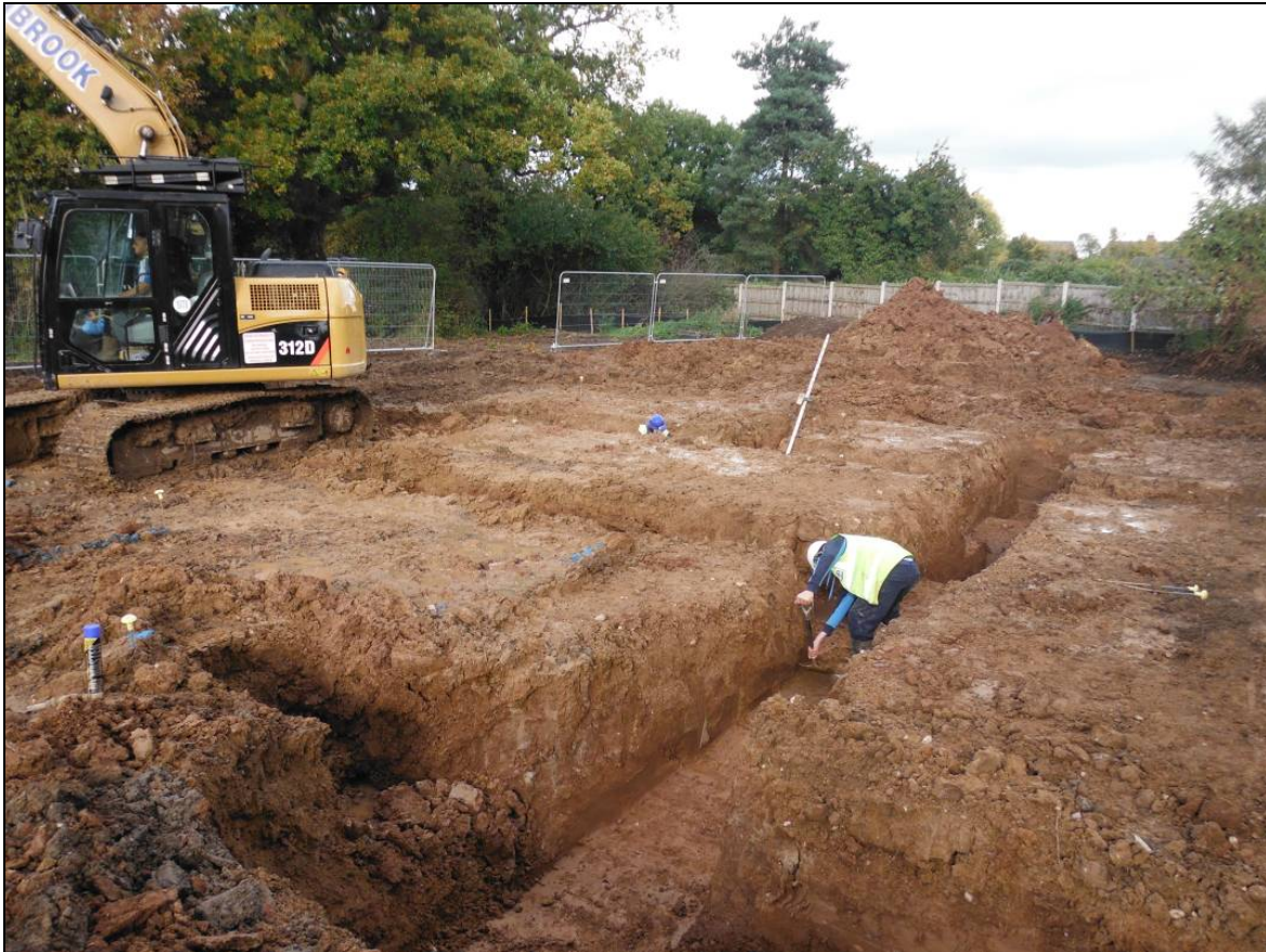
Figure 10. Excavation of the Plot 37 footings.
