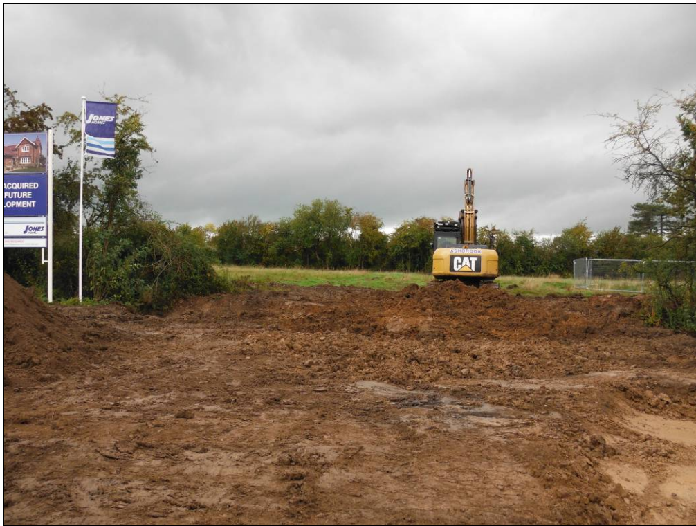
Figure 5. Initial topsoil and vegetation strip in progress.
