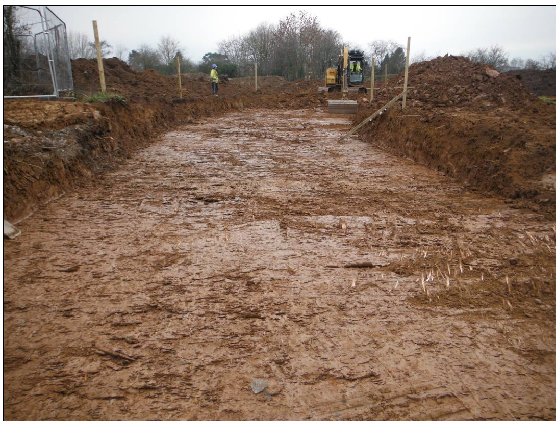
Figure 17. Stripping of the access road down to the natural substratum (003).
