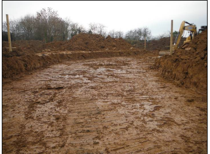
General view of the Access Road strip.
