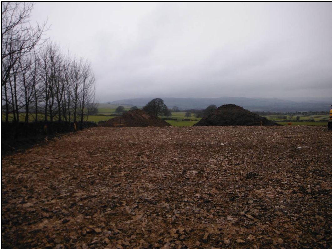
Figure 8. Build-up of the site after the initial topsoil strip.
