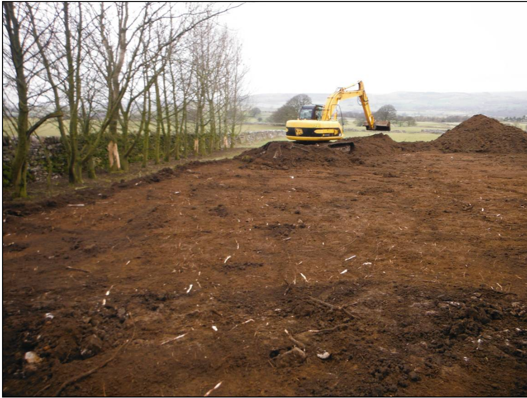
Figure 4. Initial topsoil strip of the site, looking north.
