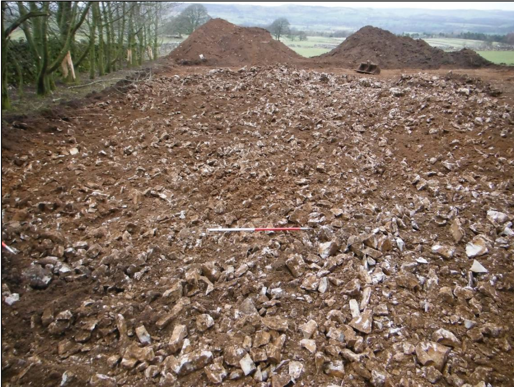
Figure 7. Strip at the south-western end of the site, excavated into the limestone bedrock. Scale = 1m.
