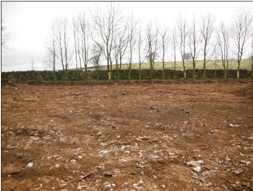
Figure 5. Subsoil at the north-eastern end of the site, looking north-west
