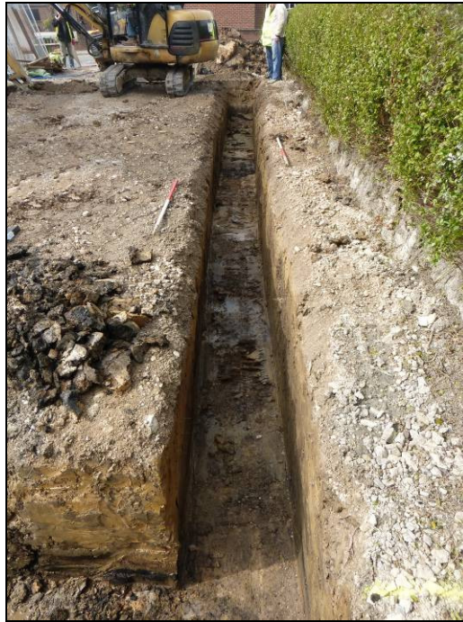
Figure 6. Footing at north of plot, looking west. Scale = 2 x 1m
