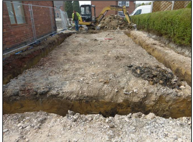
Footings at 10 Station Road, Denby, looking west
