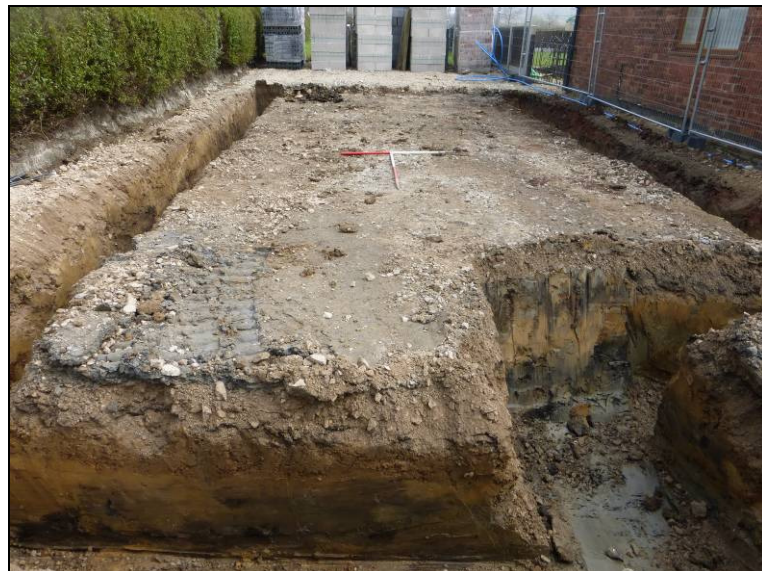
Figure 3. Denby building plot with footings, looking east. Scale = 2 x 1m
