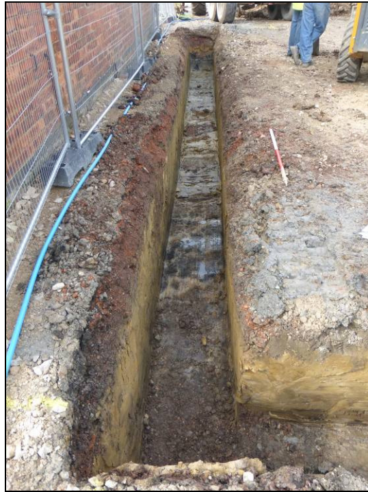
Figure 4. Footing at the south of plot, looking west. Scale = 1m
