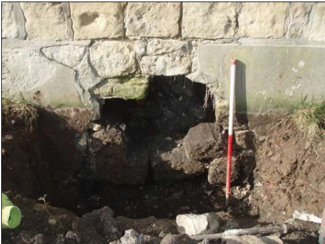
Figure 4: Test Pit 1 showing the blocked doorway.
