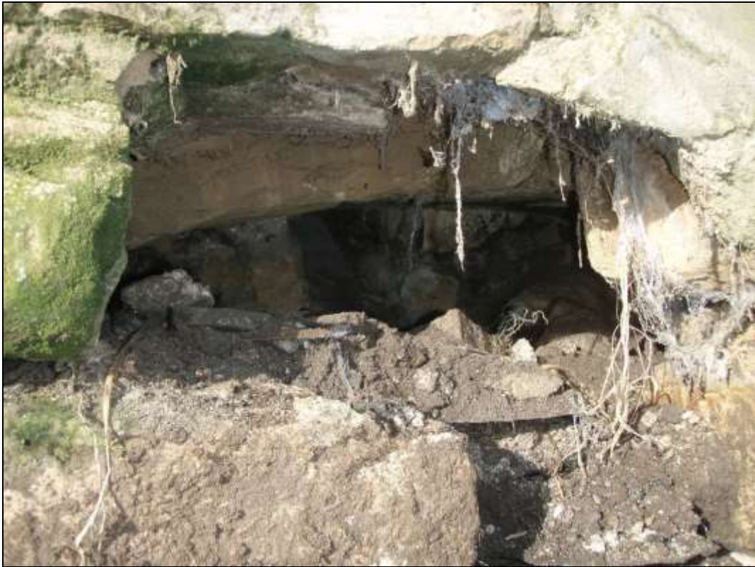
Figure 3: Looking through the blocked opening to the arch beyond.
