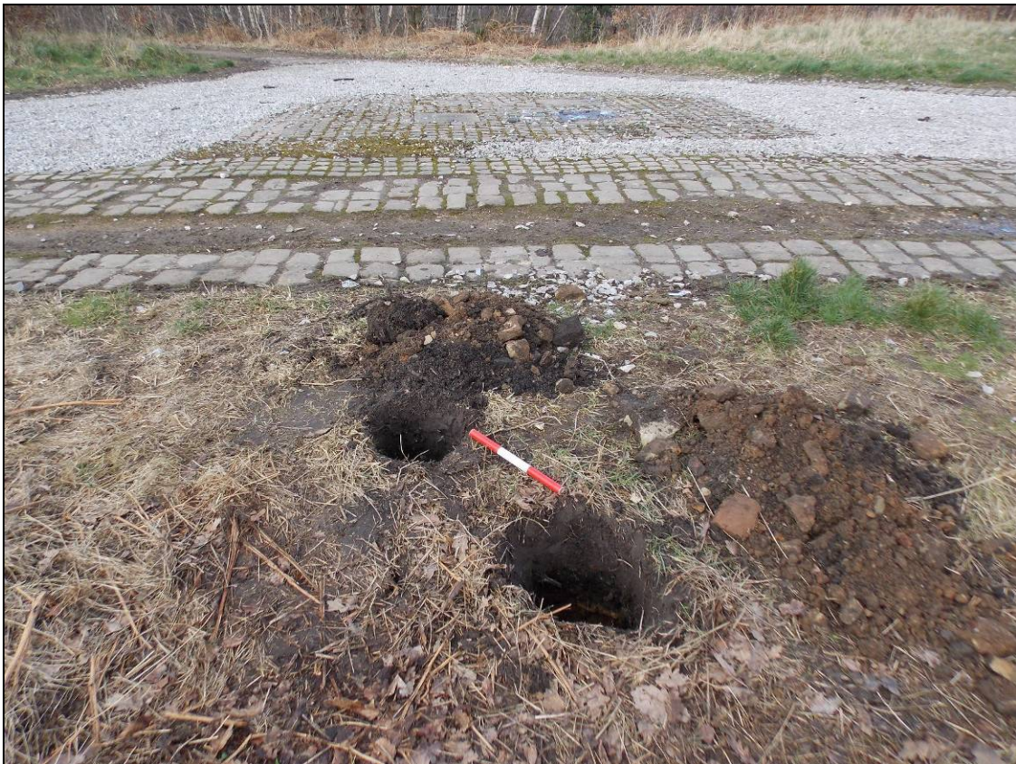
Figure 3: Excavated post holes adjacent to the confluence of footpath, looking north-west (scale 300mm).
