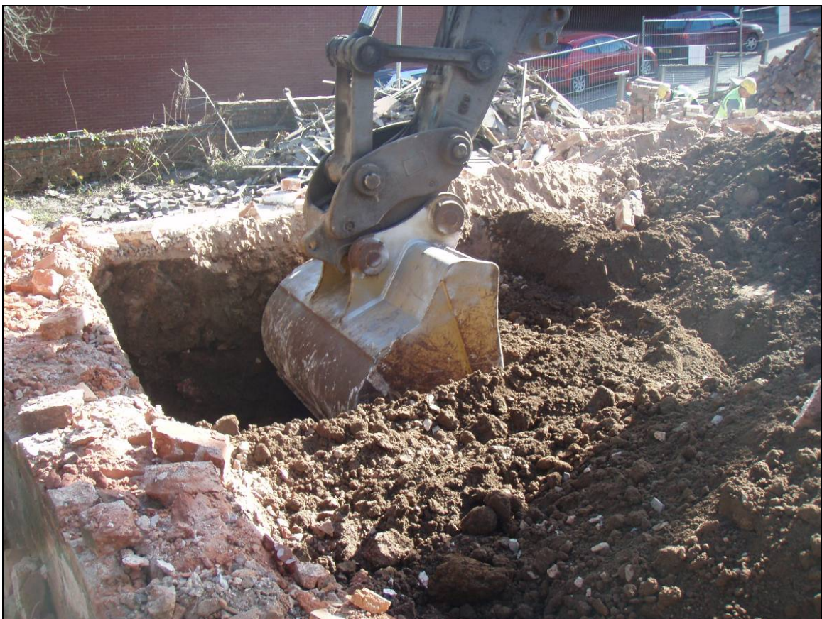
Figure 6: Excavation of the made ground layer, looking east.
