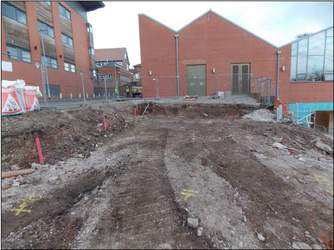
Figure 8: Excavation of Area 2, looking west.
