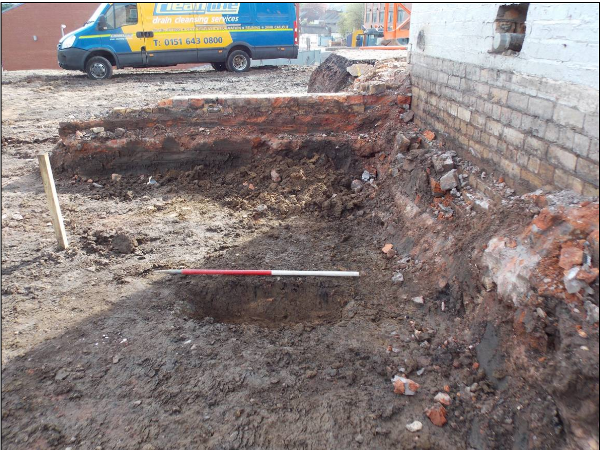
Figure 14: Sondage in close proximity to the 'Main Building' to the south, looking east (scale 1m).
