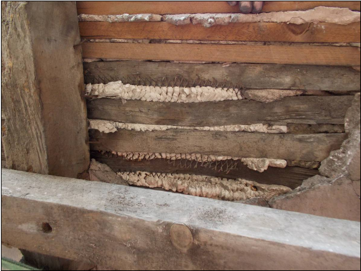
Figure 32: Repaired area with metal mesh.
