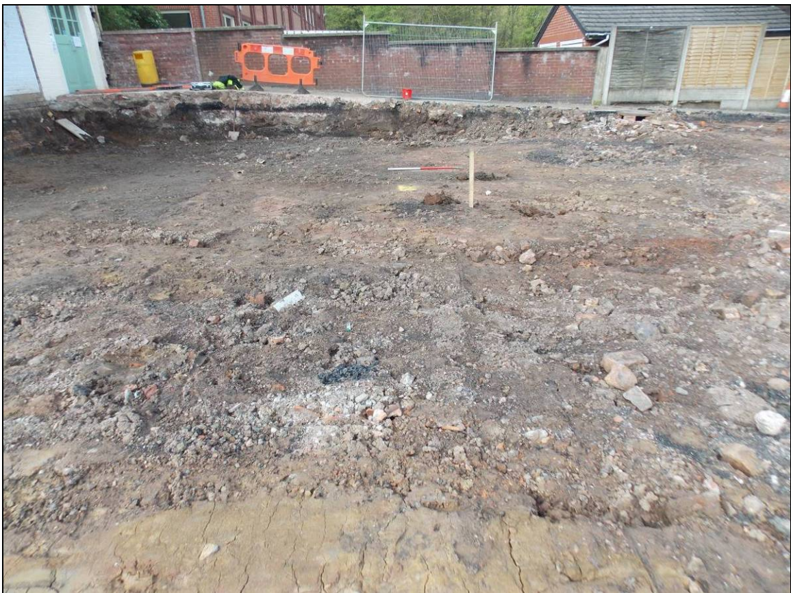
Figure 12: Excavated southern section of Area 3, looking west (scale 1m).
