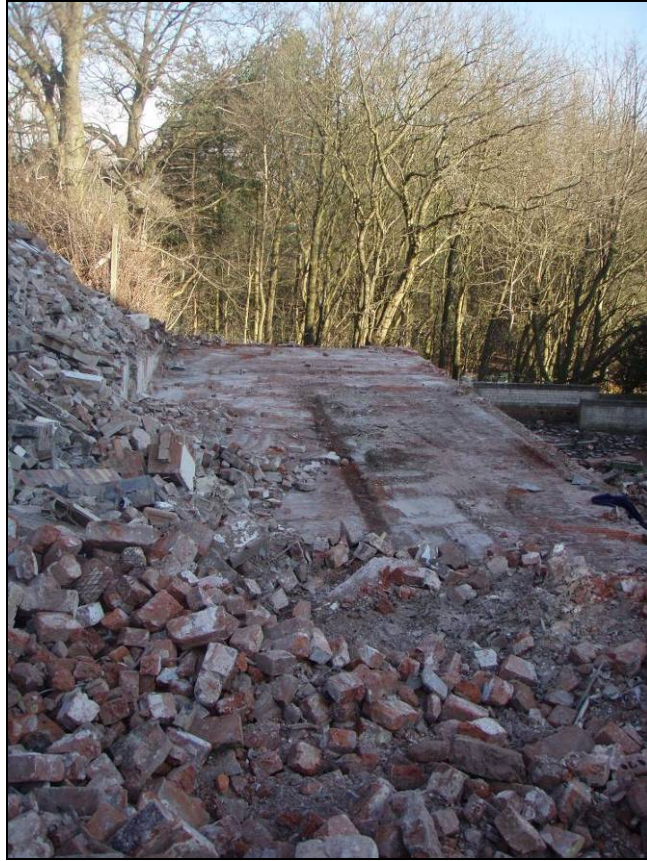
Figure 3: Concrete floor of the demolished Mill block, looking north.
