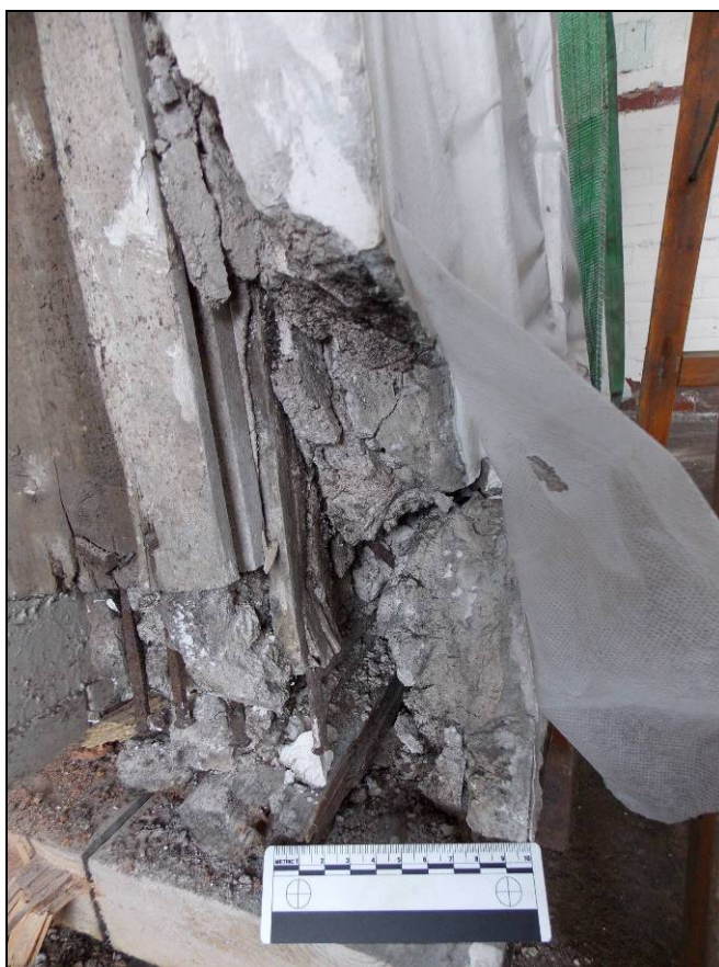
Figure 47: Detail of plaster coats and laths (scale 100mm).
