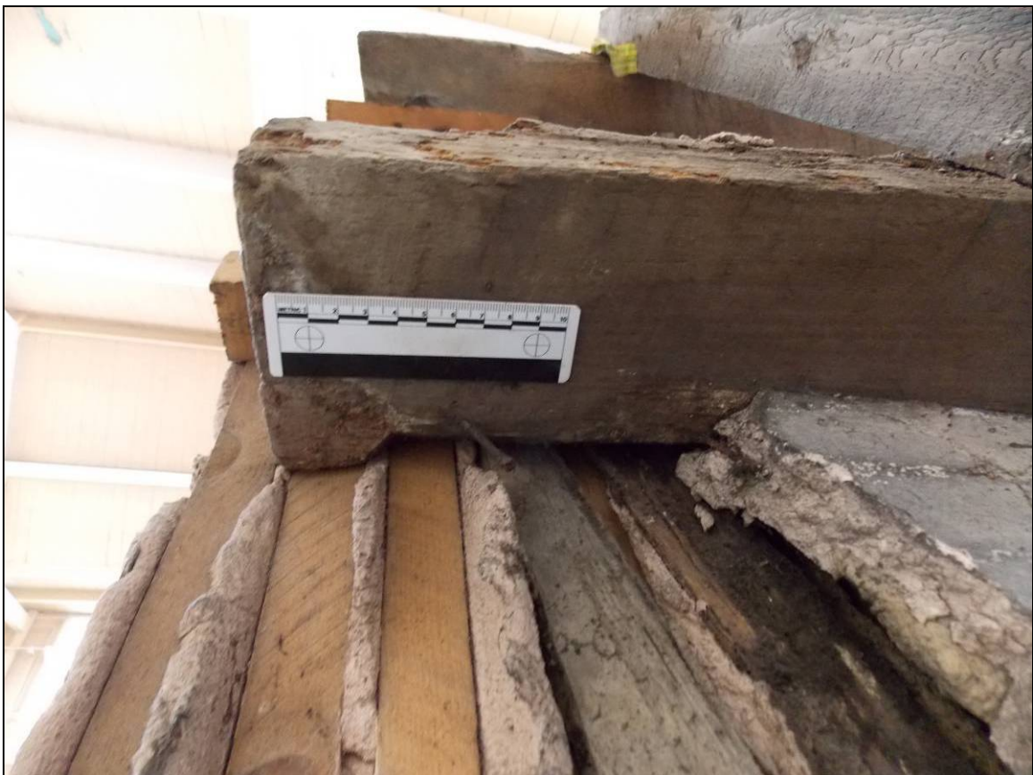
Figure 29: Ceiling joist with stop chamfer (scale 100mm).
