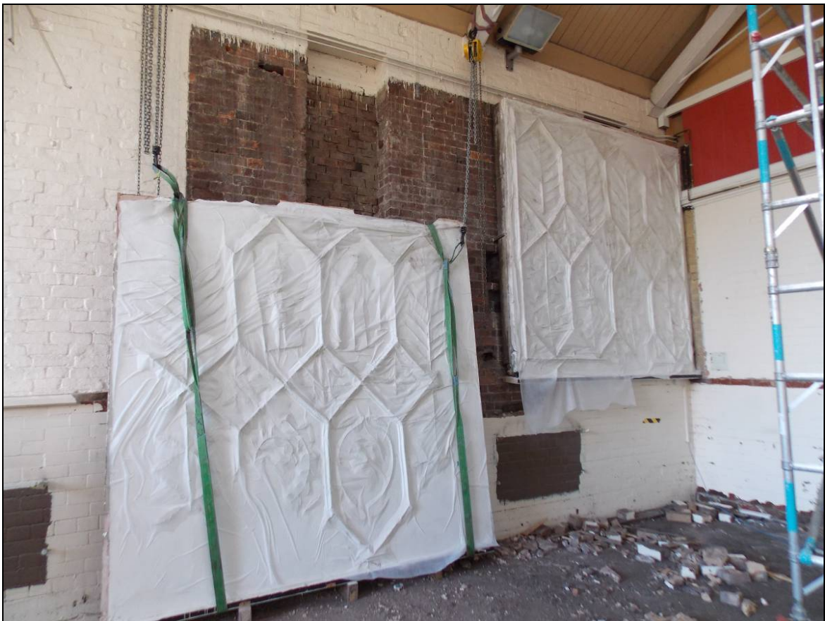
Figure 19: Panel 1 fully dismantled from the wall.
