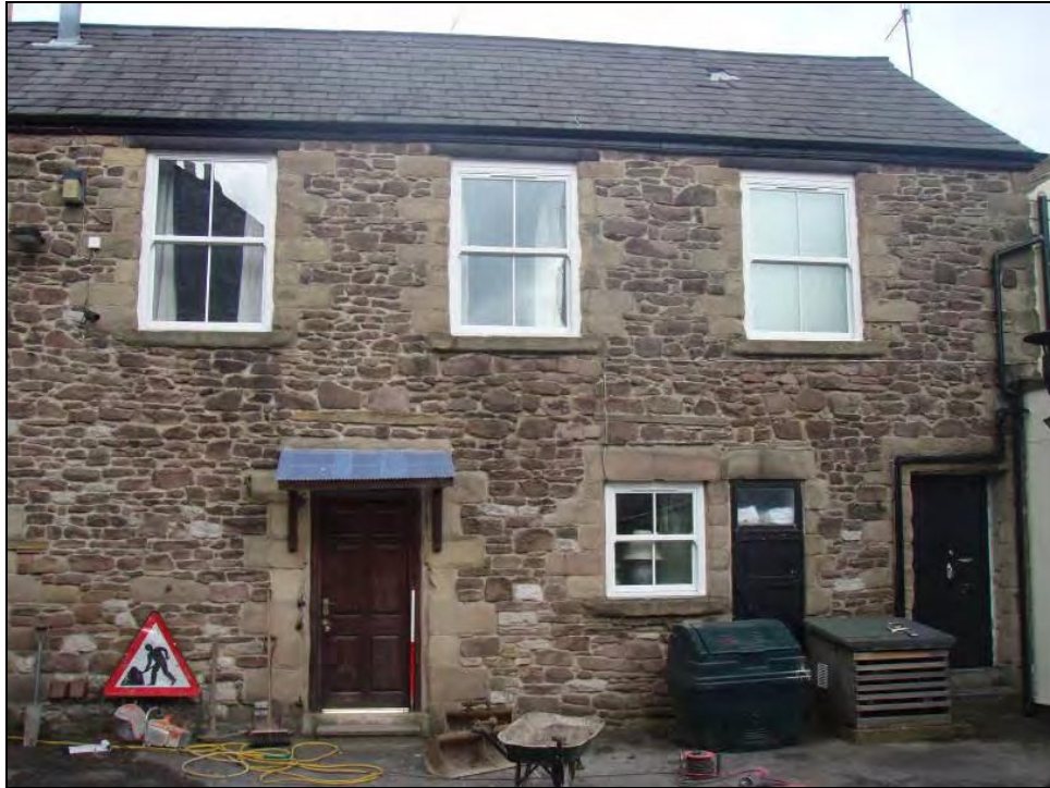
Figure 26. The existing stable in the Queen's Head car park. The walls identified during the watching brief are thought to belong to a perpendicular wing of this stable block that was demolished due to poor condition in the 1970s. Scale = 1m.
