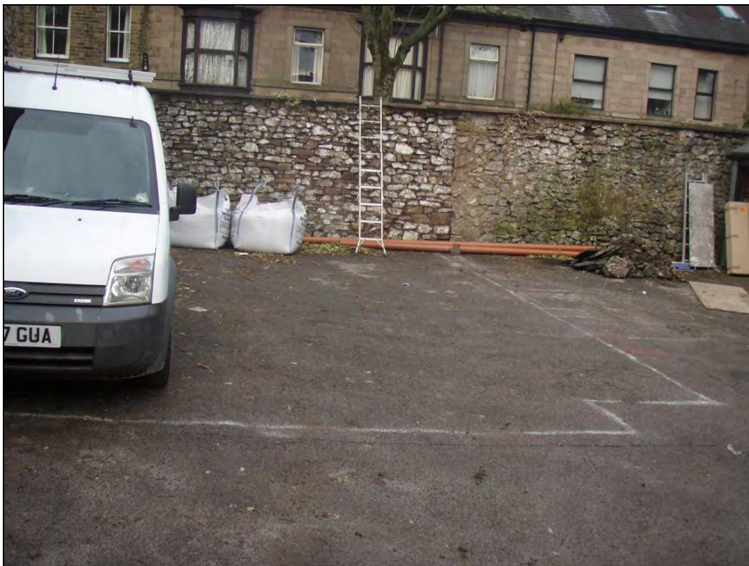
Figure 14. Wall (116) as observed intact before the commencement of ground works. The left hand side of the wall has clearly been subject to later repair/rebuilding works, however the foundations did not demonstrate any later alterations. Facing north-west.
