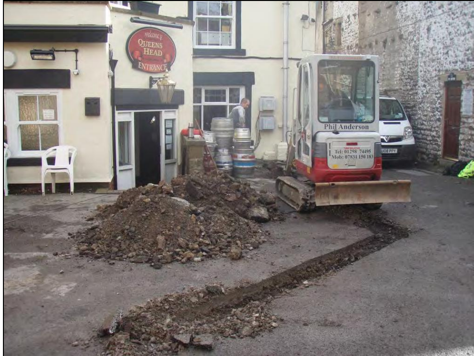
Figure 3. Trench 1 mid-excavation. Facing south-east.
