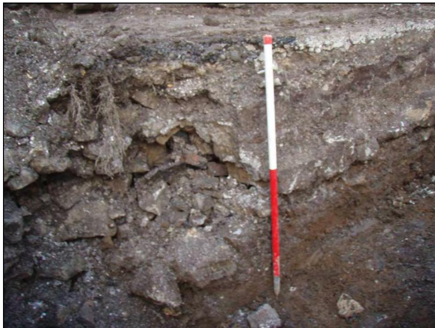
Figure 16. Intact wall (115) (right) abutting wall (116) (left), which continues beyond the confines of the trench, and runs up to the existing stable building as demonstrated in figure 13. Scale = 1m.
