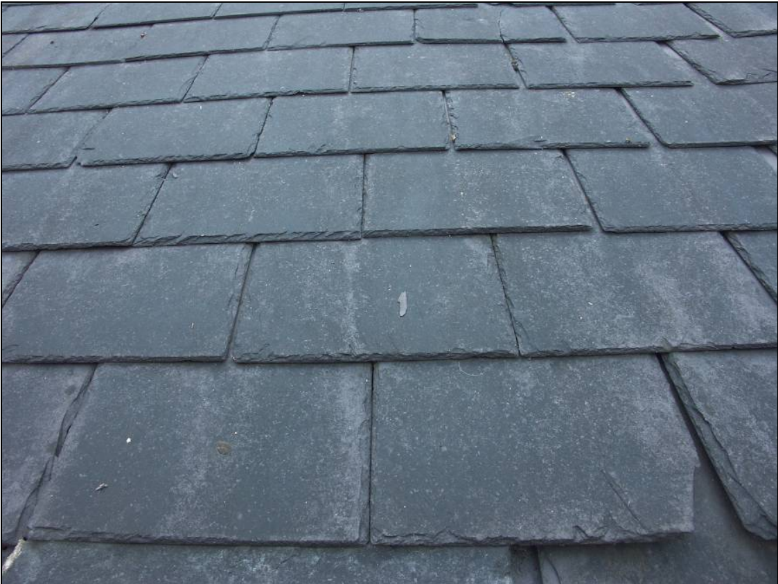
Figure 15: Detail of the slated roof of the small lean-to structure (Block 6)
