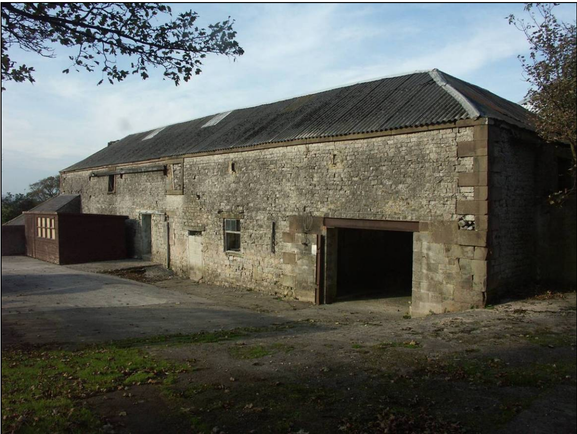
Figure 16: General view of the southern wing
