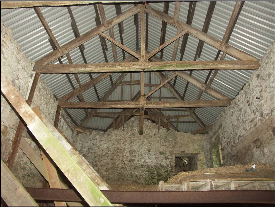
Figure 11: General view of the central roof structure of Block 2
