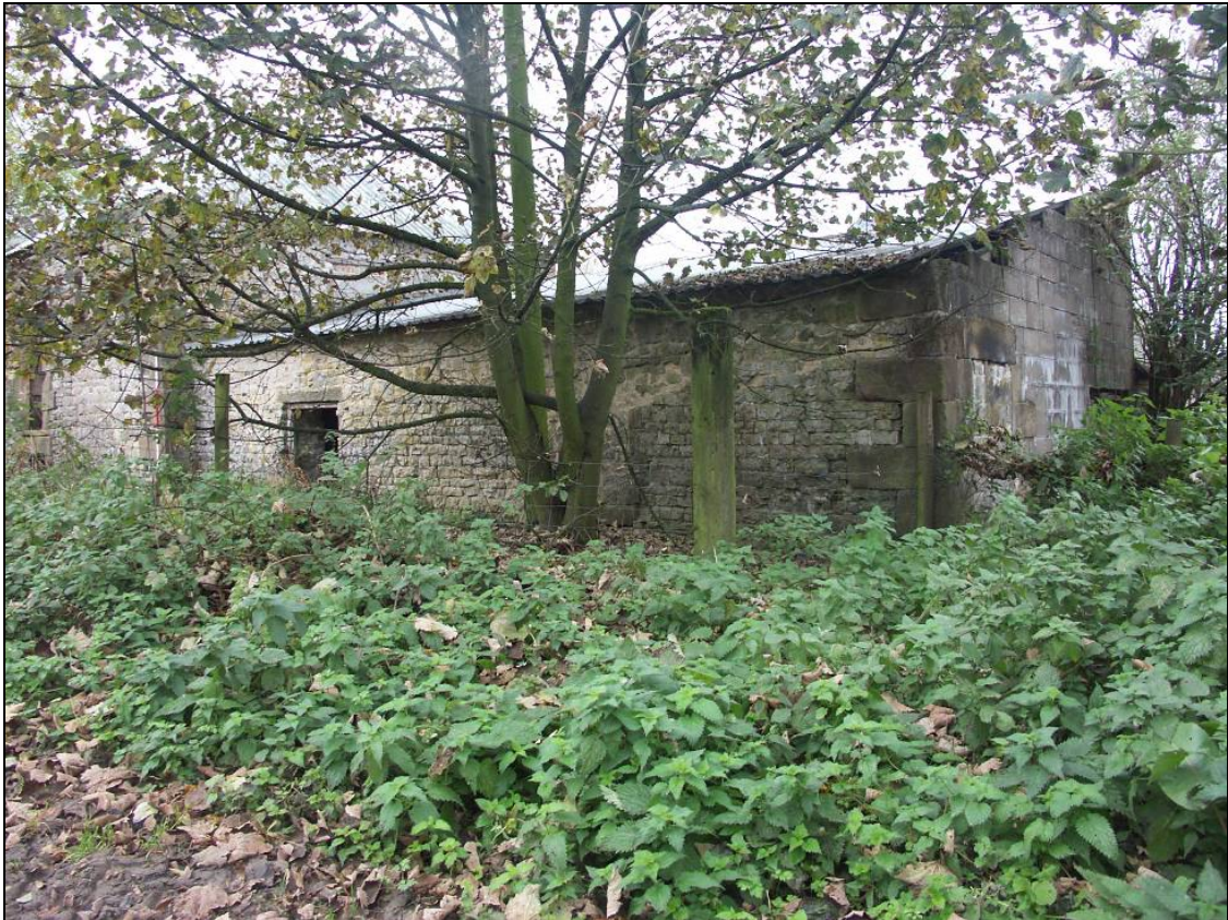
Figure 7: Modern alterations within the north section of the eastern wing (Block 1)
