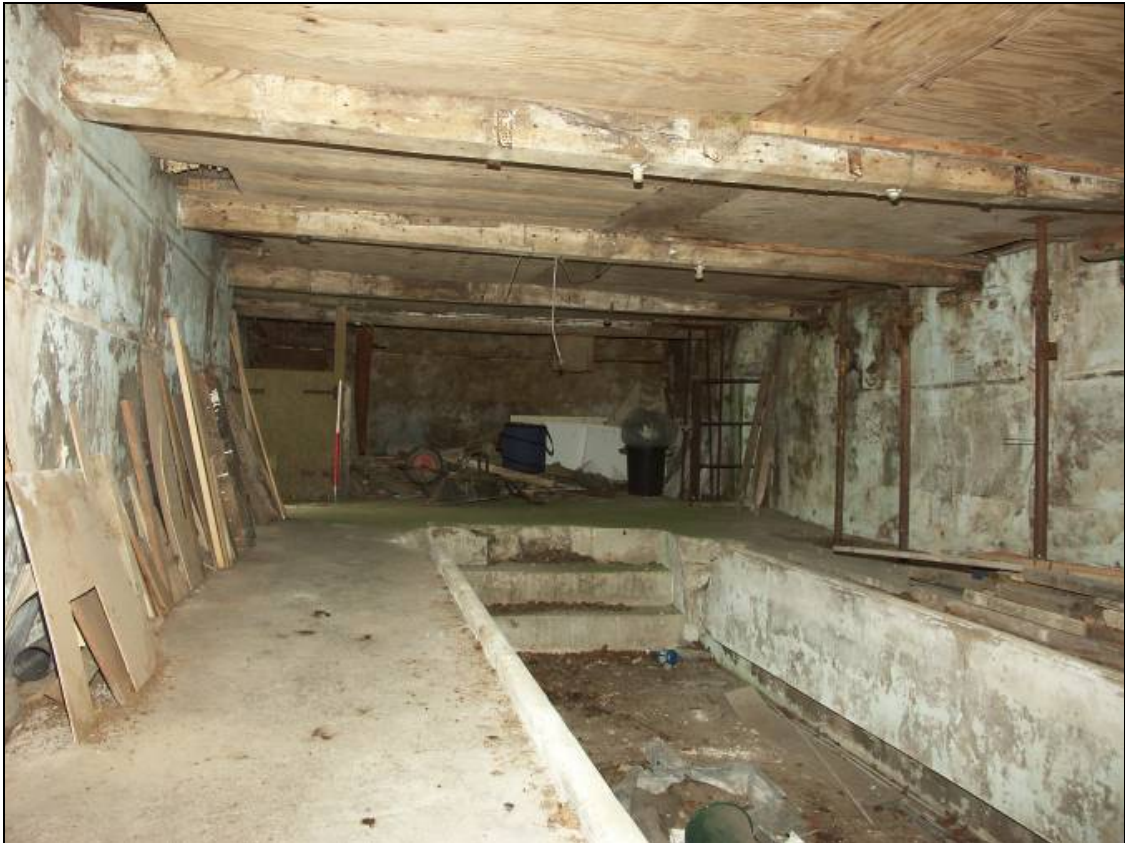
Figure 19: Internal view of the milking parlour (Block 4)
