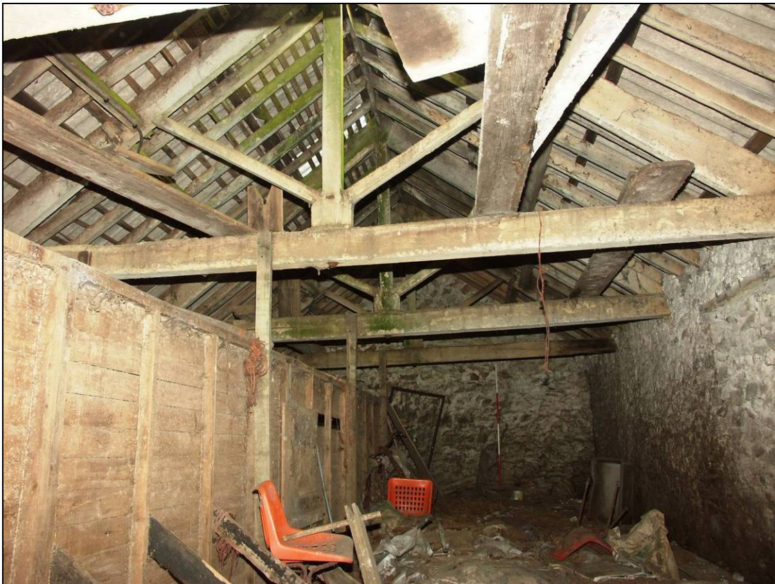
Figure 20: Roof structure of the southern wing (Block 4)
