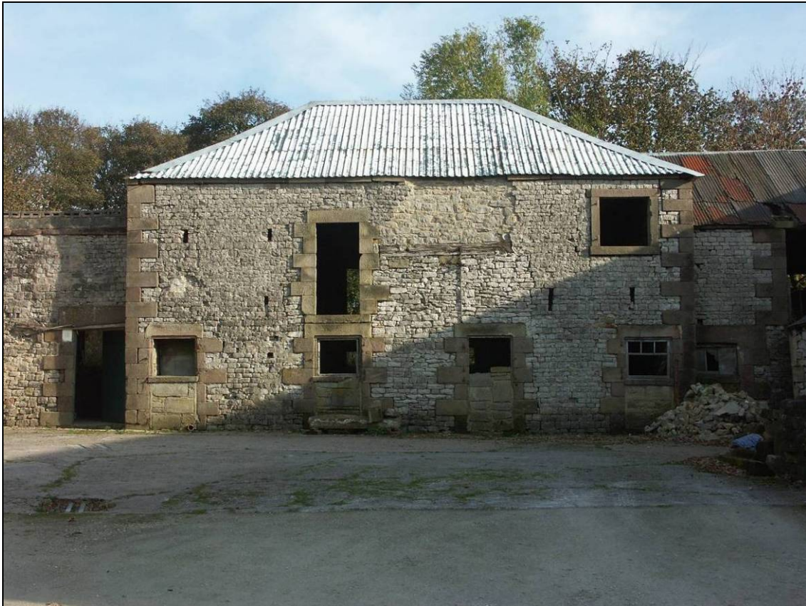
Figure 3: West elevation of the eastern wing with the central range (Block 2)
