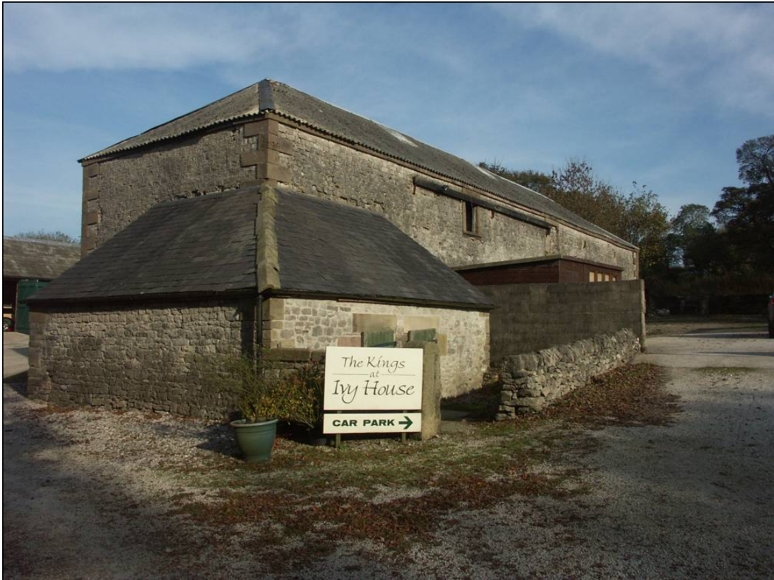
Figure 17: Southern wing with lean-to structure (Block 7) abutting the west and south elevations
