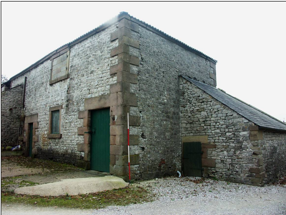
Figure 18: Detail of the west elevation of the southern wing (Block 5)
