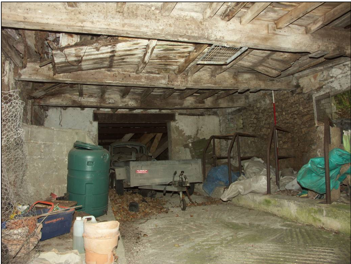
Figure 10: Southern ground floor of the eastern wing (Block 3)
