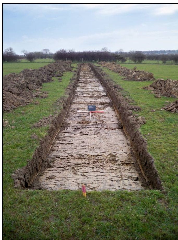
Figure. 30. ENE facing shot of Trench 10 (Scale: 2 x 1m)
