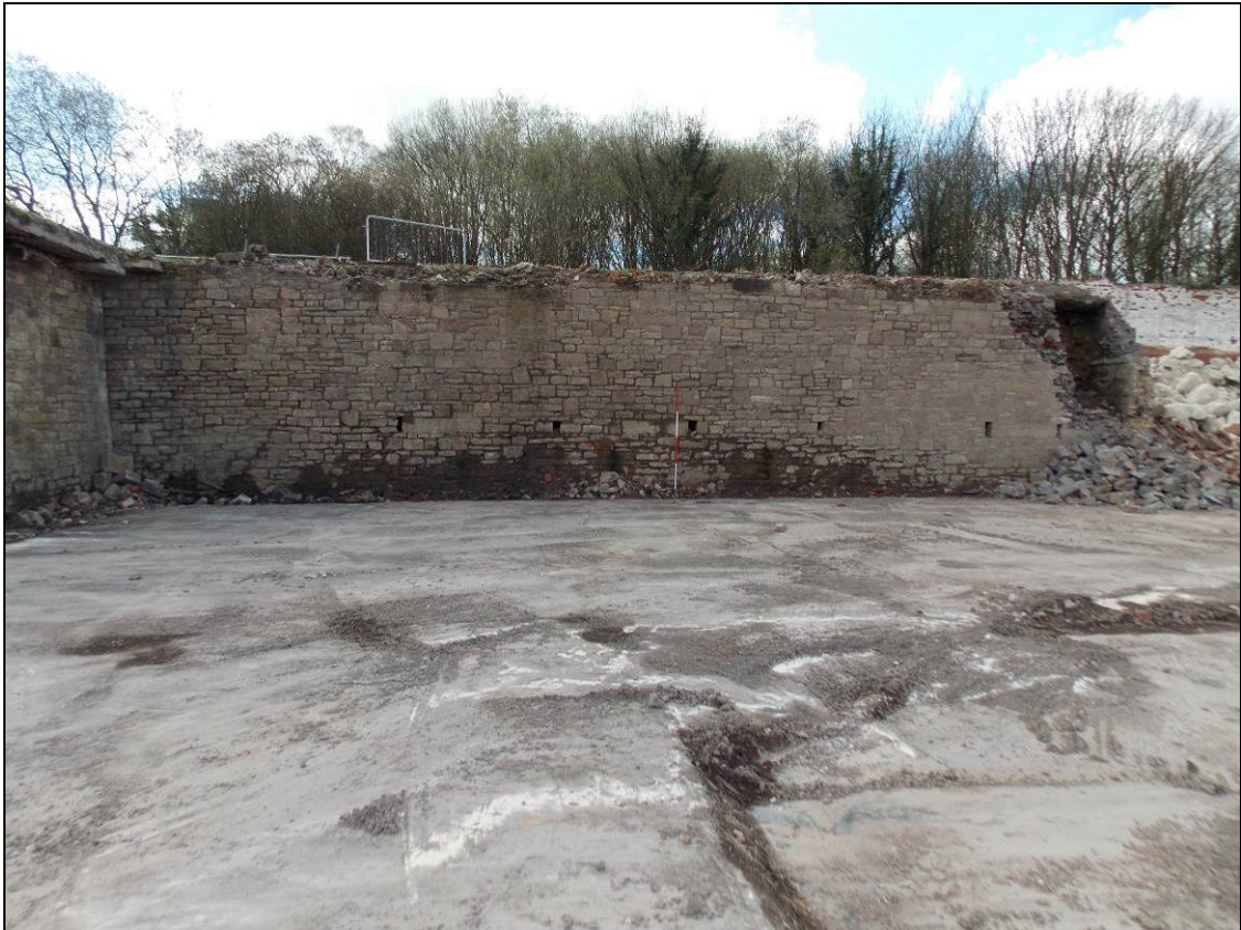
Figure 20: Southern retaining wall, looking south-west (scale 2m).
