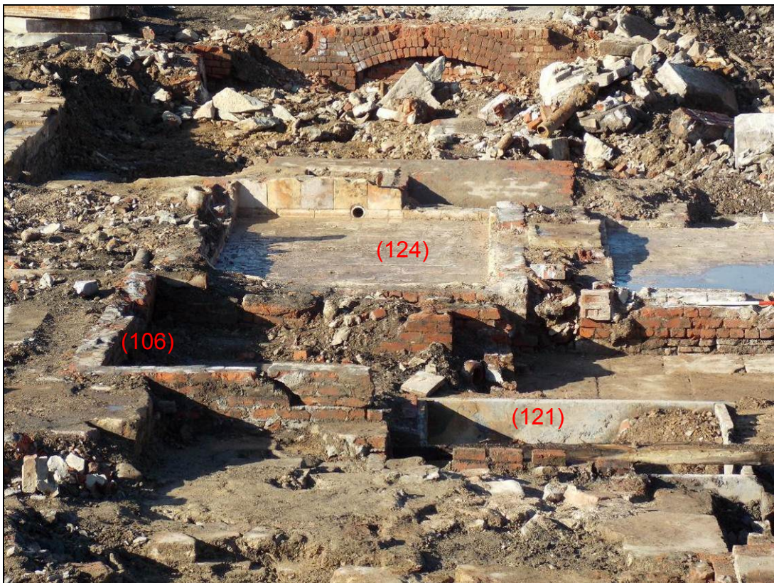
Figure 93: Southernmost tank (124) and adjacent structures, looking west (scale 1m).
