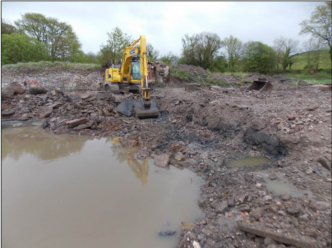
Figure 103: General view of the watching brief excavation.
