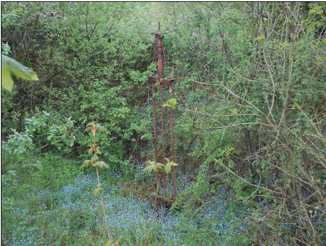
Figure 35: Detail of sluice gate mechanism, looking north.
