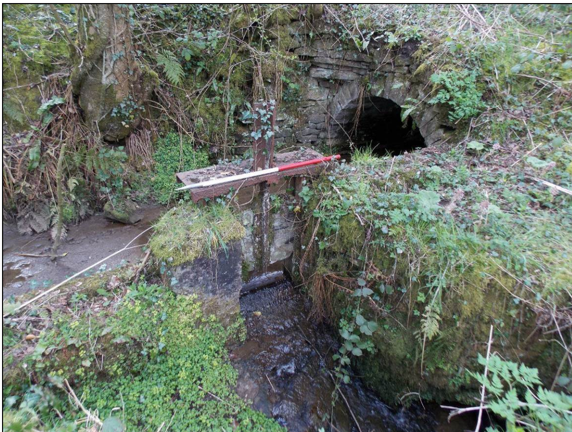
Figure 59: Sluice gate and spillway, looking south (scale 1m).
