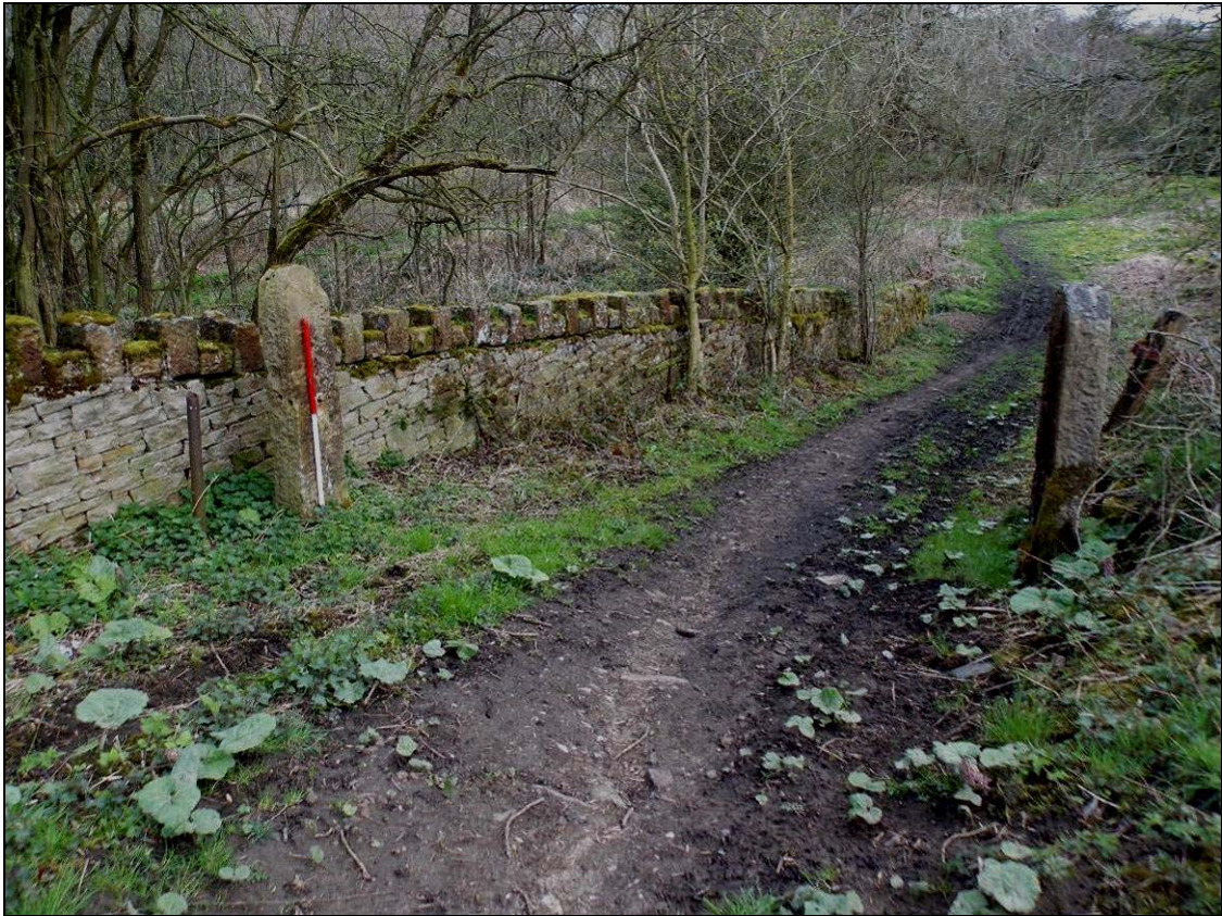
Figure 65: Structure N and boundary wall, looking north-east (scale 1m).
