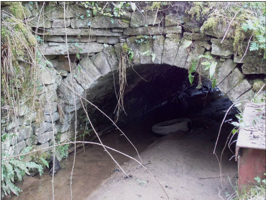
Figure 58: Detail of stone bridge, looking north-west.
