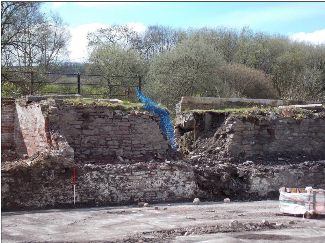
Figure 40: Terraced stone walls within the central area, looking south (scale 1m).
