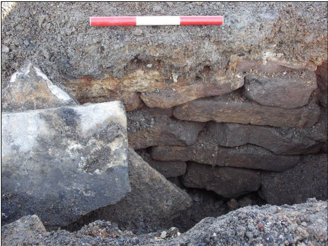
Figure 83: Stone-lined drain (135), looking north-west (scale 300mm).
