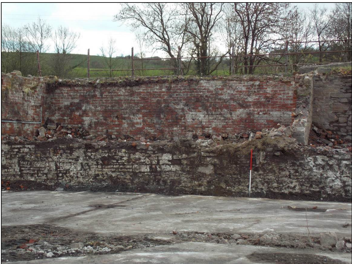
Figure 38: Brick-built extension to the south of the main southern stone wall, looking south (scale 1m).
