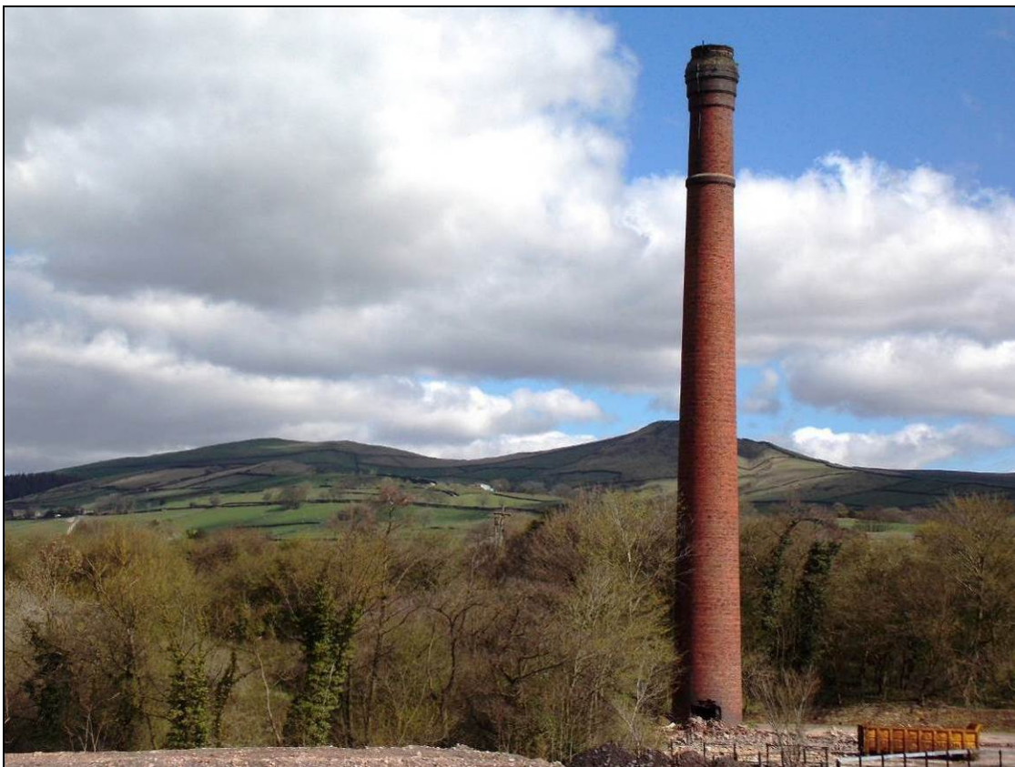
Figure 47: General view of the chimney, looking north.
