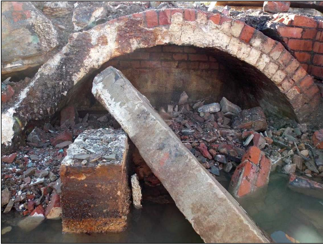
Figure 88: Detail of brick vaulted chamber (133), looking south.
