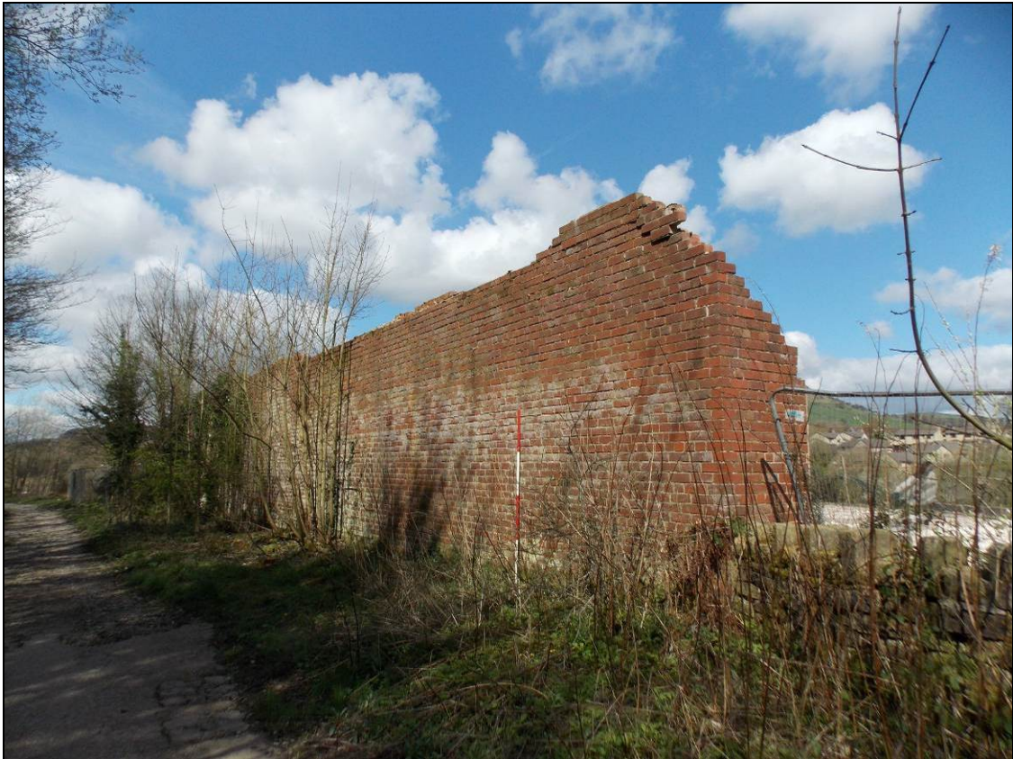
Figure 13: Structure D facing onto the disused tramway, looking north-west (scale 2m).
