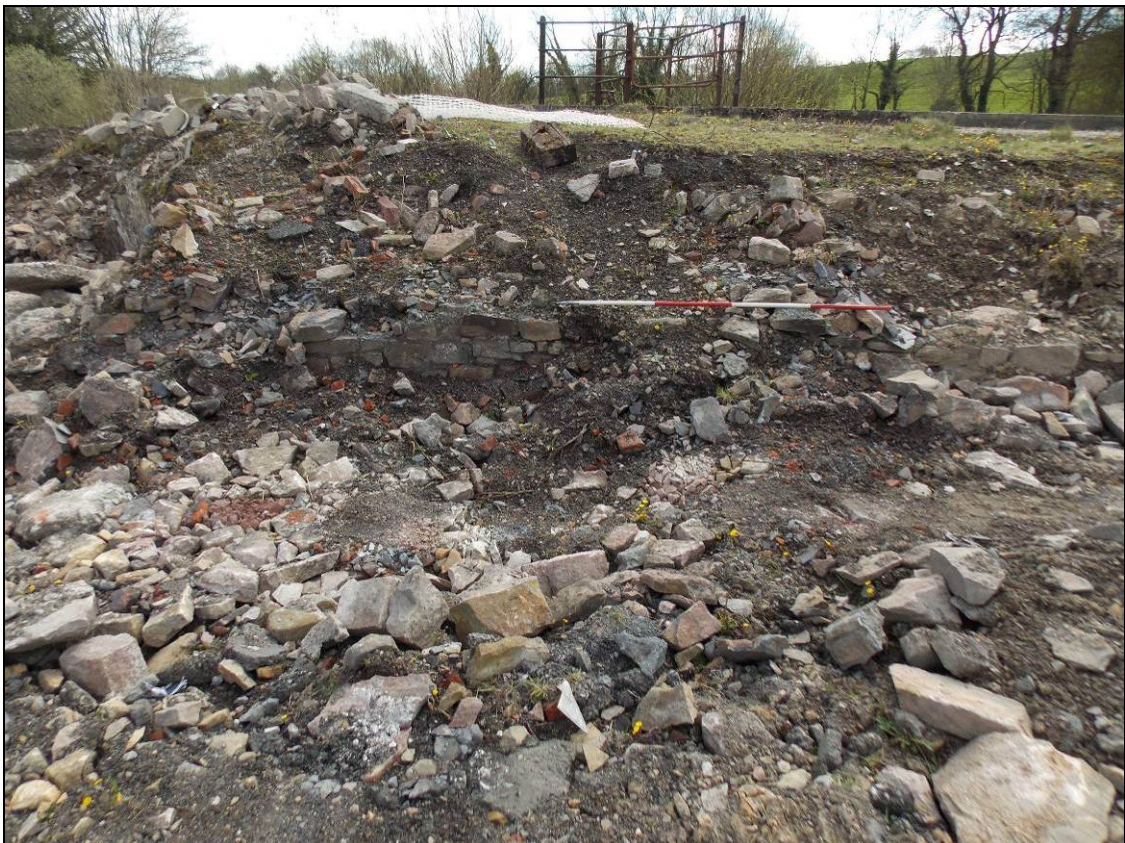
Figure 26: Surviving retaining wall of the trackway, looking east (scale 2m).
