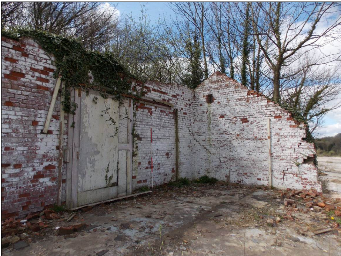
Figure 16: Western internal end of Structure D, looking north-west (scale 2m).
