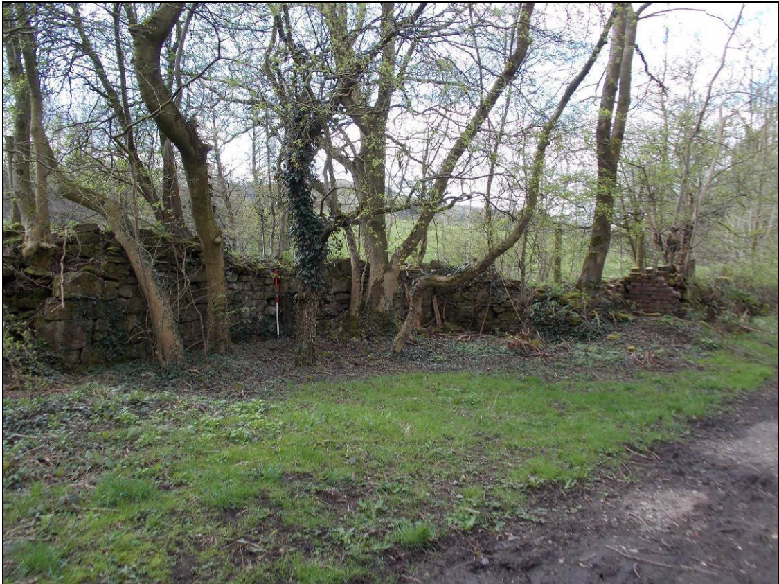
Figure 60: General view of Structure M, looking south-west (scale 1m).
