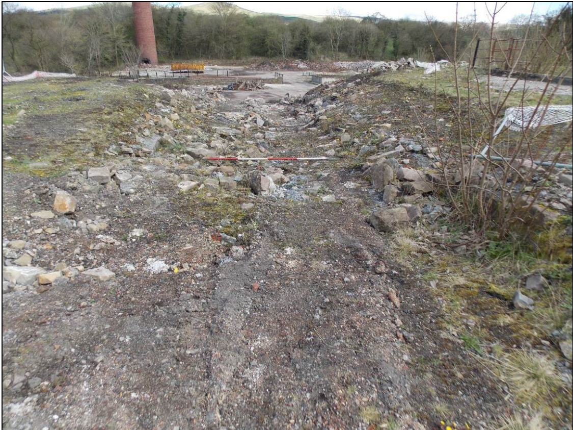
Figure 25: Structure F mostly backfilled with rubble, looking north (scale 2m).
