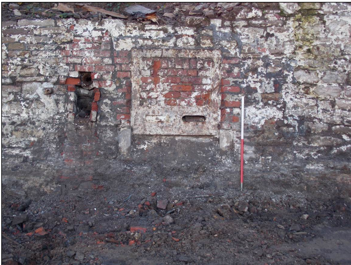
Figure 45: Detail of bricked-up bearing housing, looking south-east (scale 1m).
