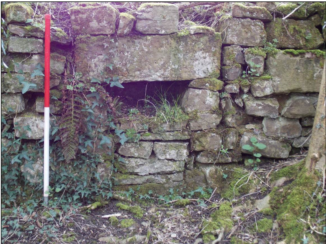
Figure 63: Detailed of blocked-up fire place, looking south (scale 1m).
