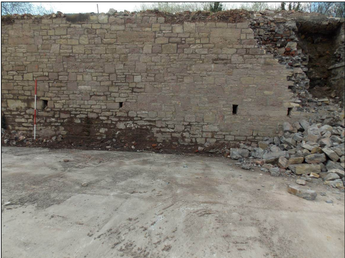
Figure 21: Detail of retaining wall with weep holes, looking south (scale 2m).
