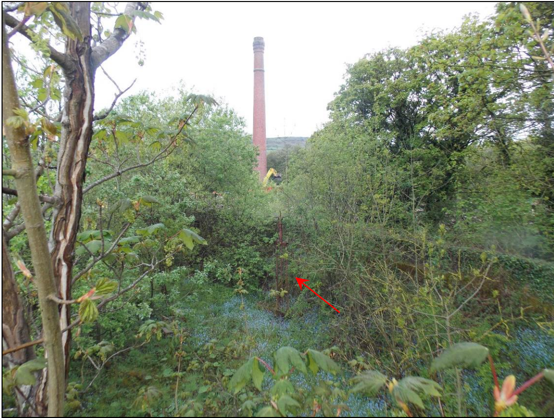
Figure 34: Small mill pond with a sluice gate mechanism (arrow), looking north.
