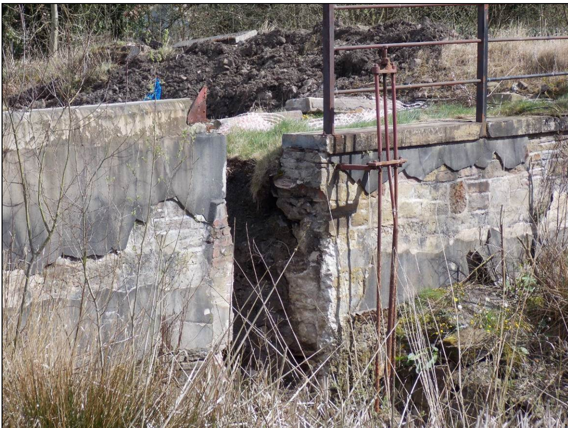
Figure 31: Remains of a sluice gate mechanism, looking south-east.
