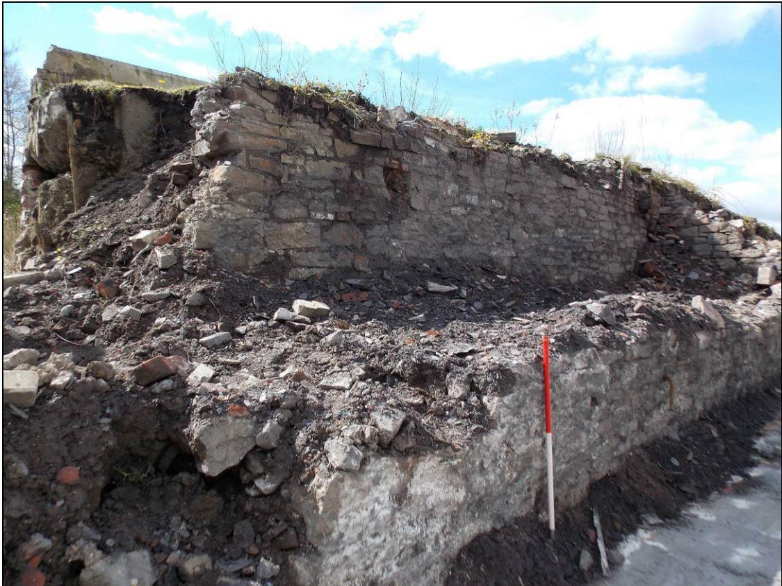
Figure 41: Detail of the terraced stepped walls, looking south-west (scale 1m).
