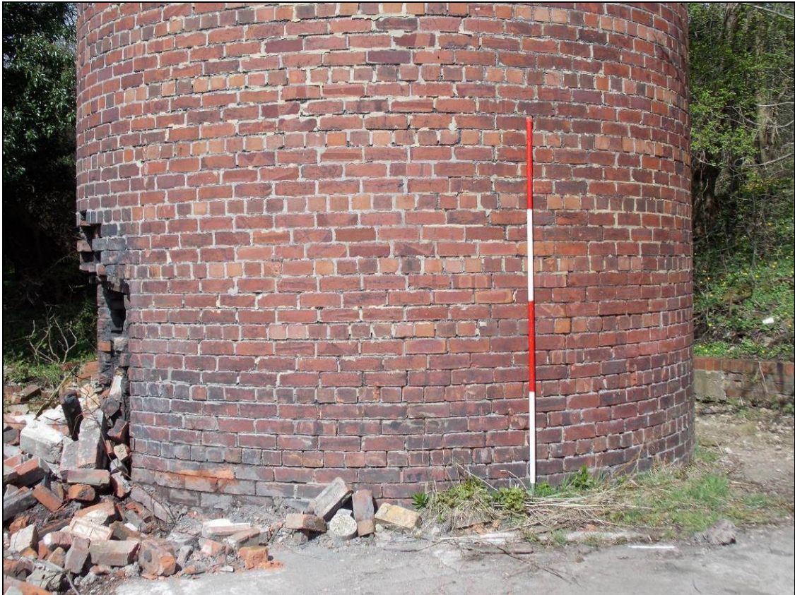
Figure 50: Detail of the brickwork, looking north-west (scale 2m).
