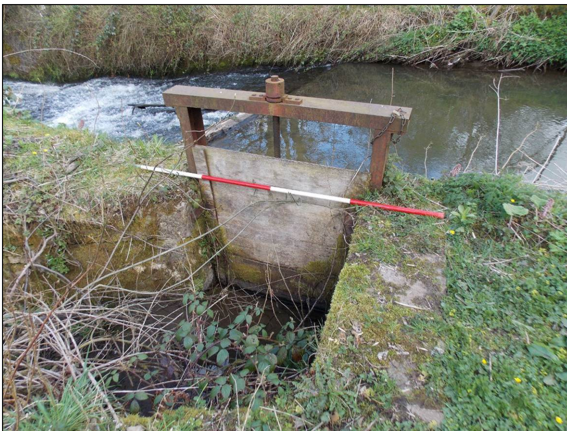
Figure 71: Structure P, looking north (scale 2m).
