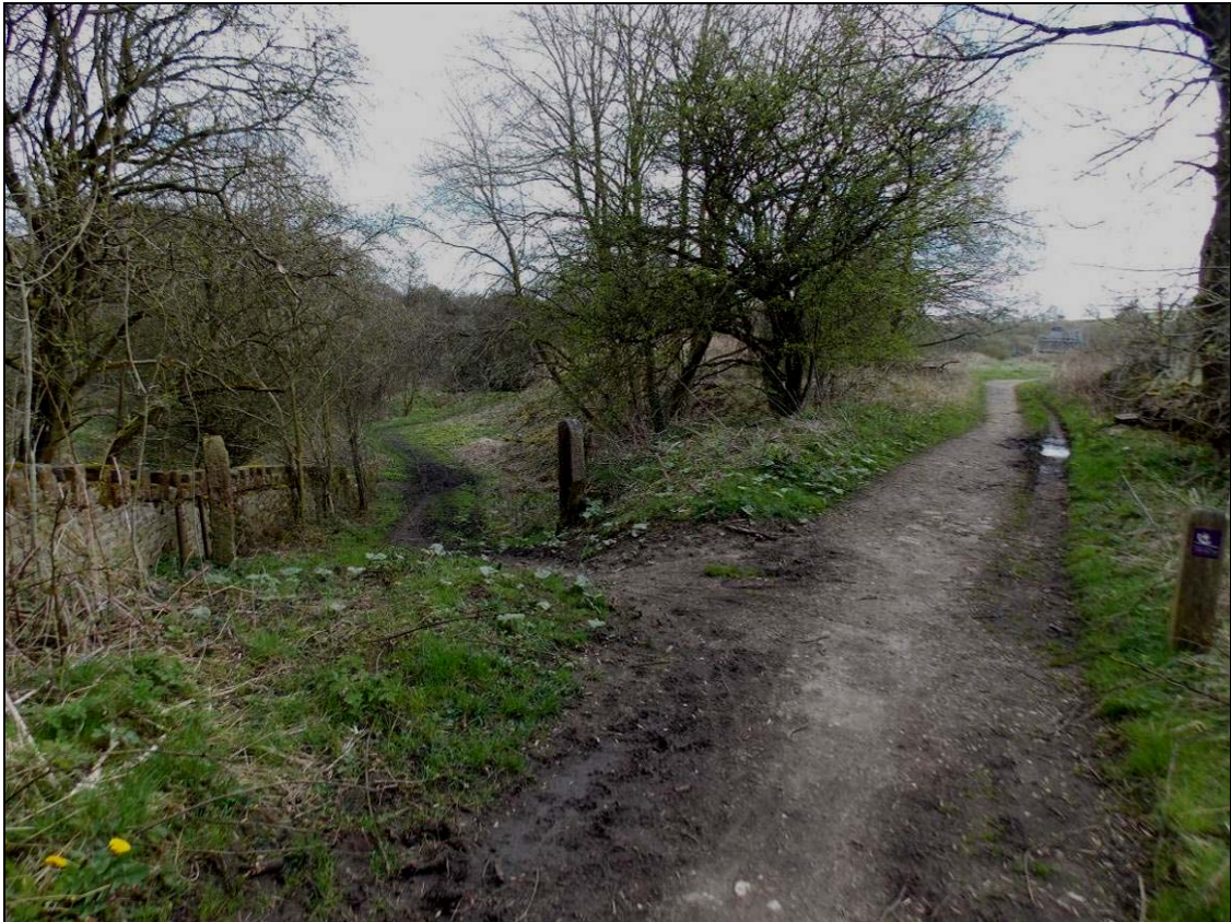
Figure 64: Structure N between the boundary wall and disused tramway, looking south-east.
