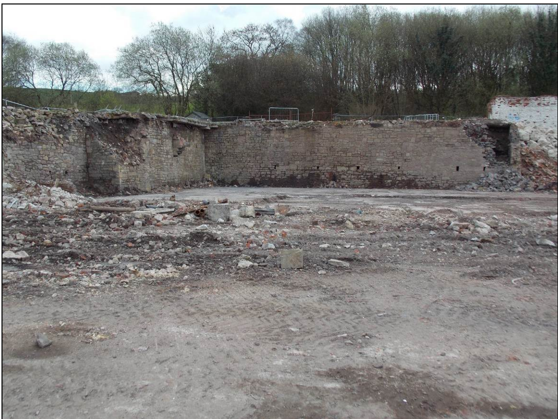
Figure 19: Internal corner of Structure E, looking south-west.
