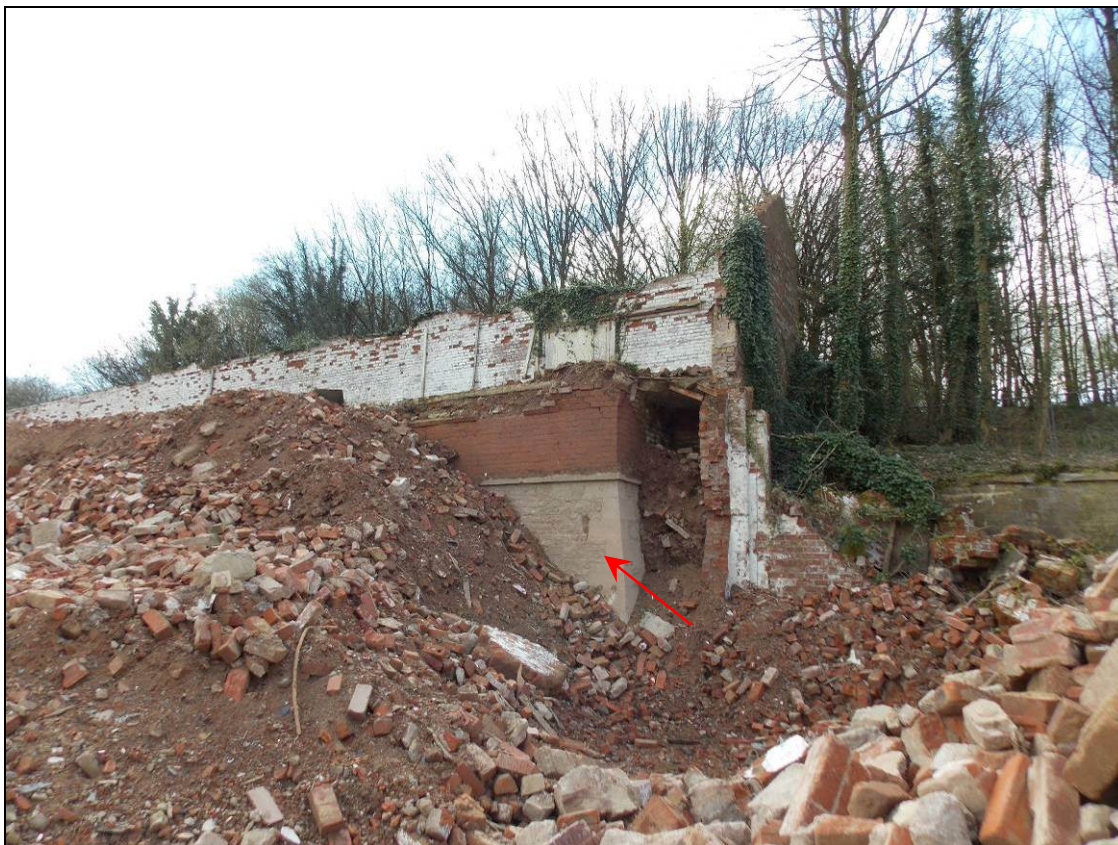
Figure 17: Detail of retaining wall with an earlier phase of construction (arrow), looking south.
