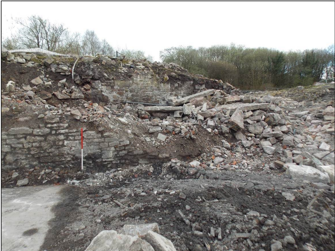
Figure 43: Westernmost end of the southern terraced wall, looking south (scale 1m).
