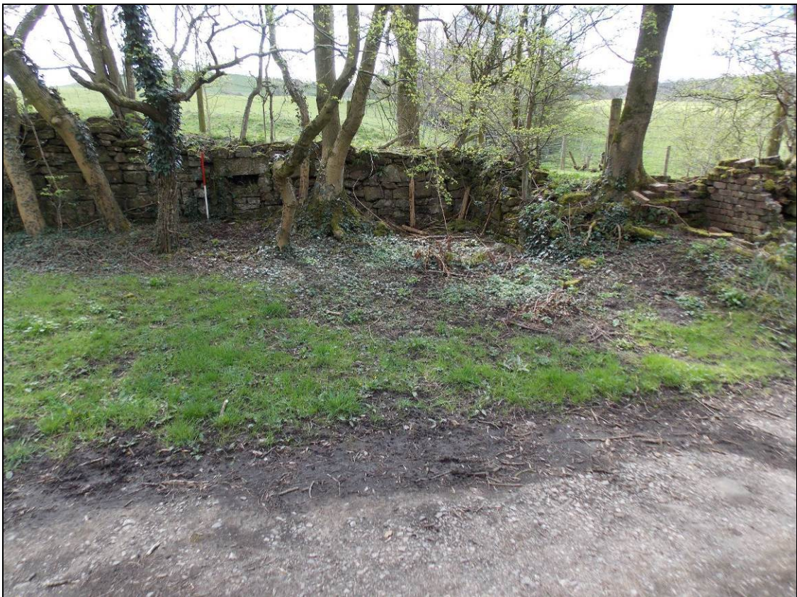
Figure 61: Southern wall with a central fire place, looking north (scale 2m).
