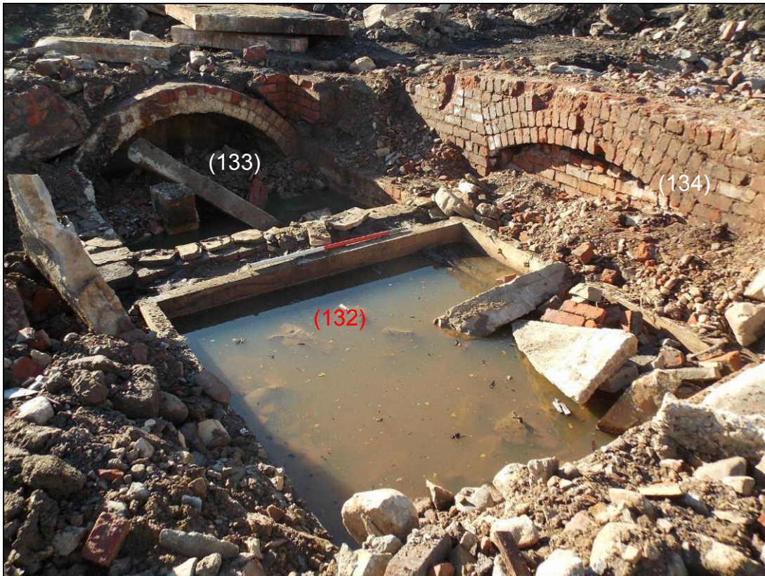
Figure 86: Cistern (132), vaulted chamber (133) and wall (134), looking south-west (scale 1m).
