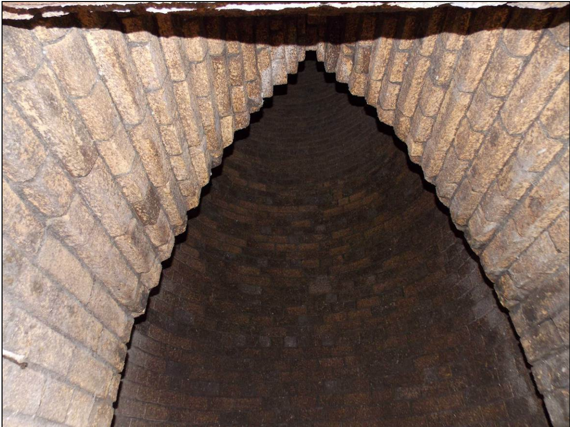
Figure 52: Fire bricks within the flue, looking north.
