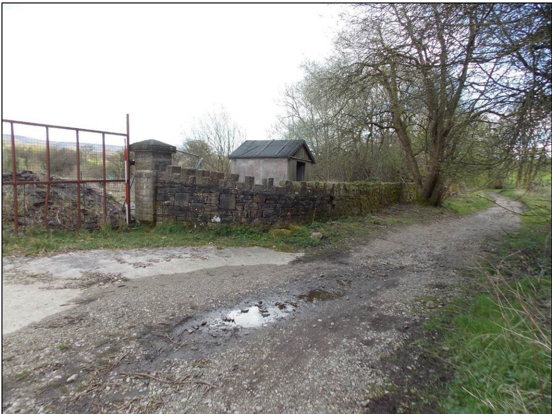
Figure 5: Eastern gatepost abutted by the wall along the disused tramway, looking south-east (scale 2m).
