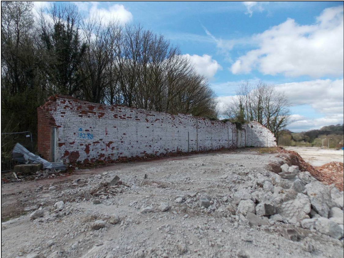
Figure 15: Internal view of Structure D, looking west (scale 2m).
