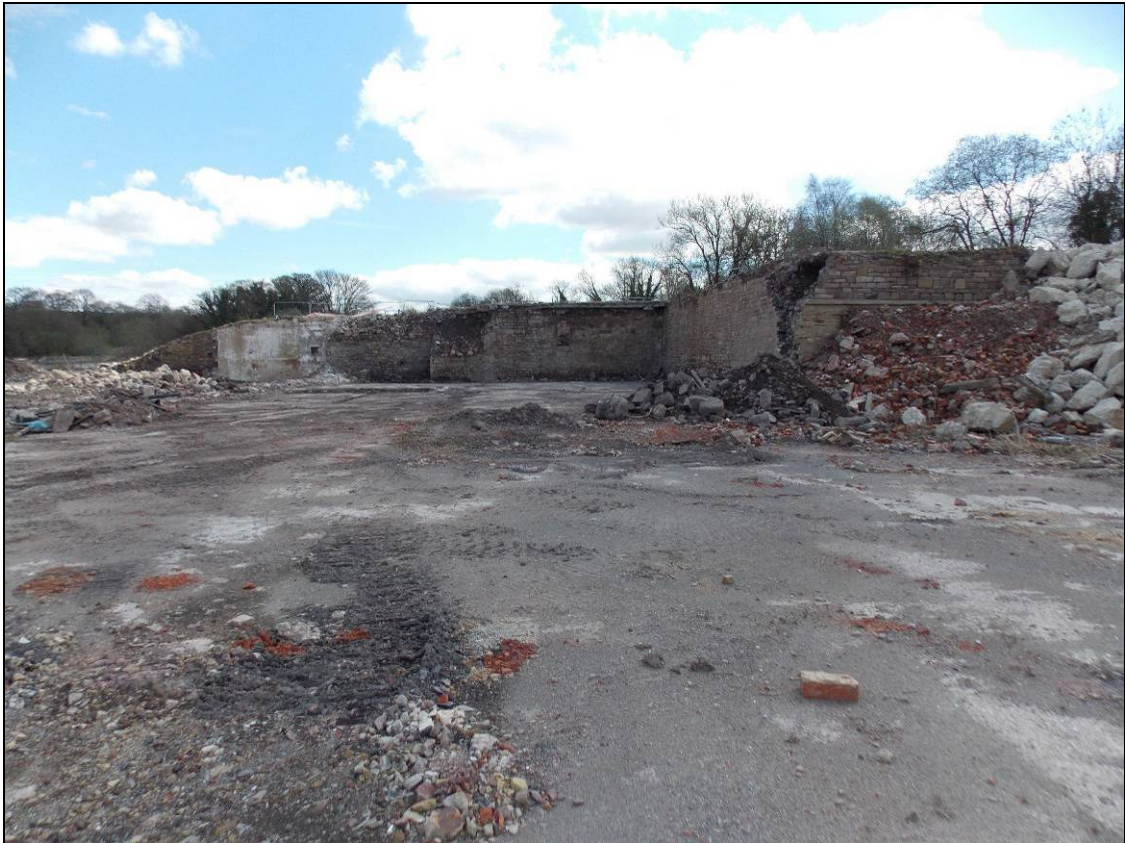
Figure 18: General view of Structure E, looking south-east.
