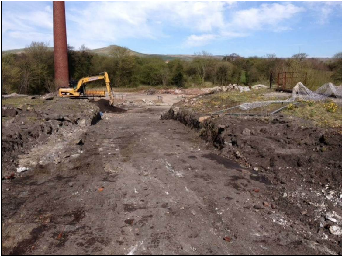
Figure 27: Trackway following the excavation of the backfilled rubble, looking north.
