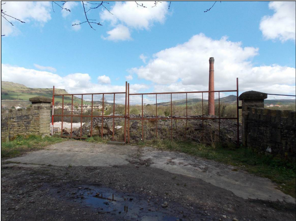
Figure 4: Structure A, looking north (scale 2m).
