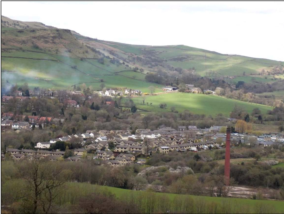
Figure 46: The tall chimney (Structure I) within its setting, looking north-west.
