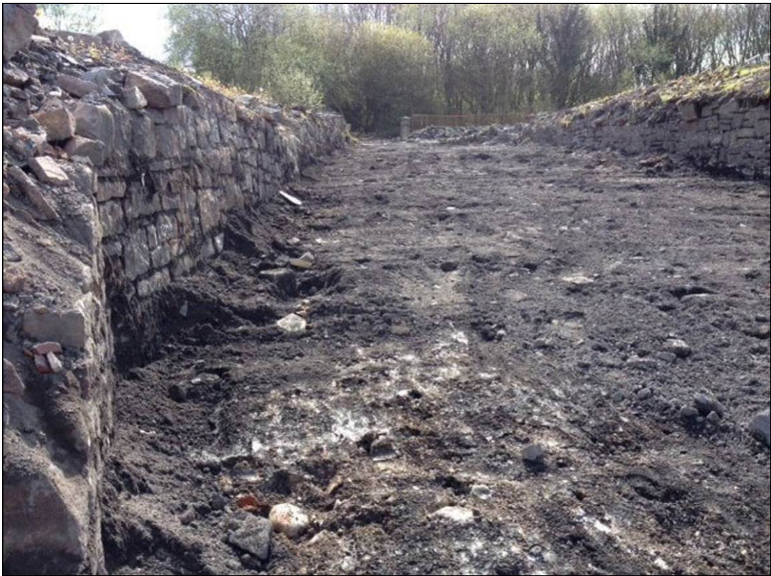
Figure 28: Excavated trackway flanked by retaining walls, looking south.
