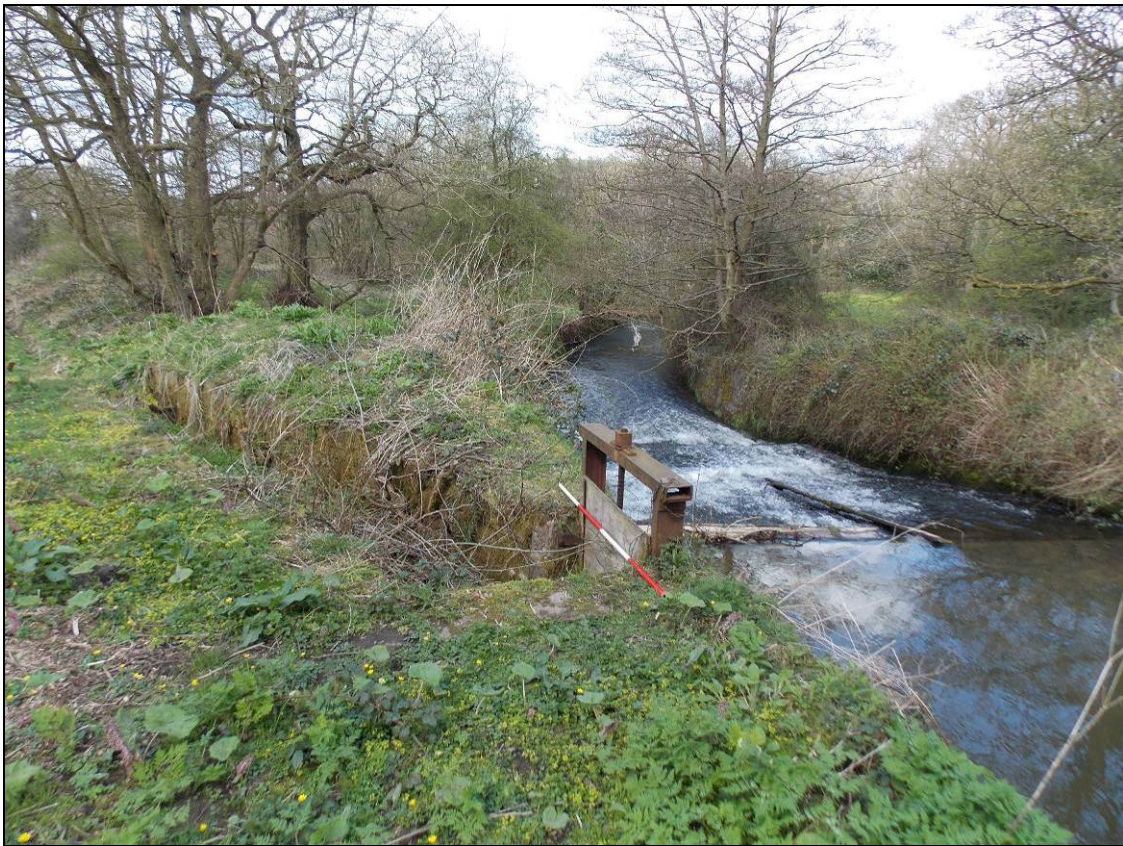
Figure 70: Structure P adjacent to Black Brook, looking north (scale 2m).
