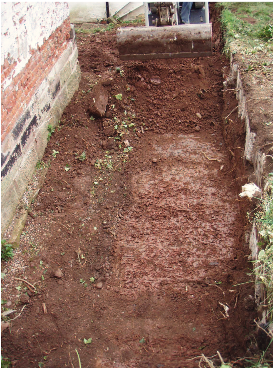
Photo 7 - Working shot – exposing top of natural substratum (104), looking east
