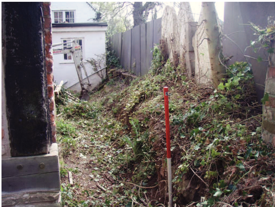
Photo 1 - Gravestones and wall prior to removal, looking east
