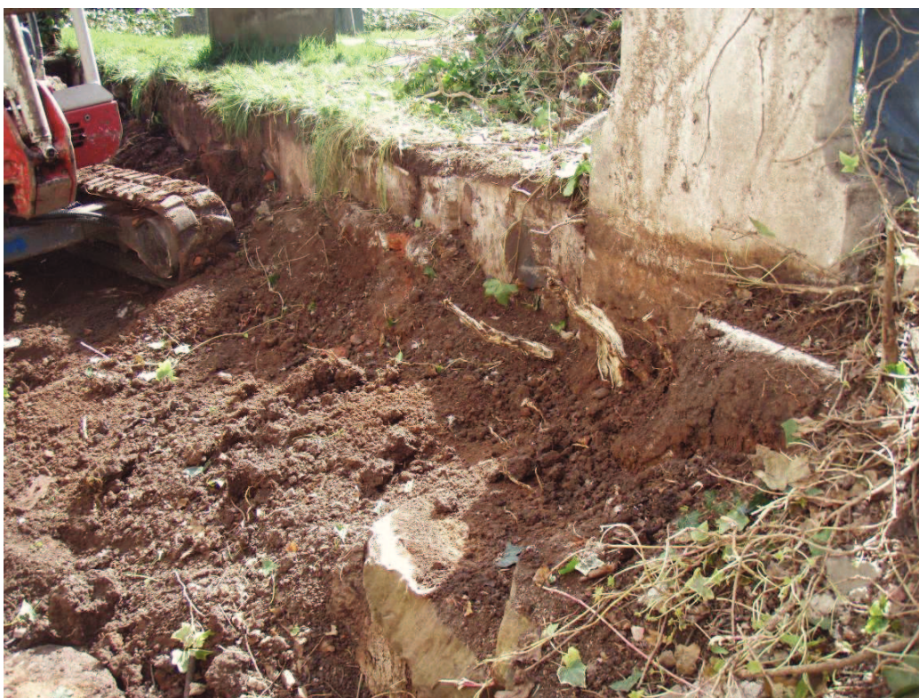
Photo 6 - Working shot - gravestone during removal exposing (102), looking south east
