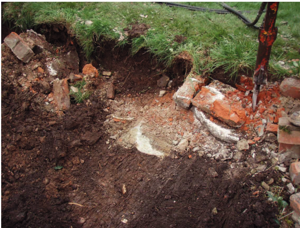
Photo 9 - Working shot – removal of western boundary wall footings, looking south
