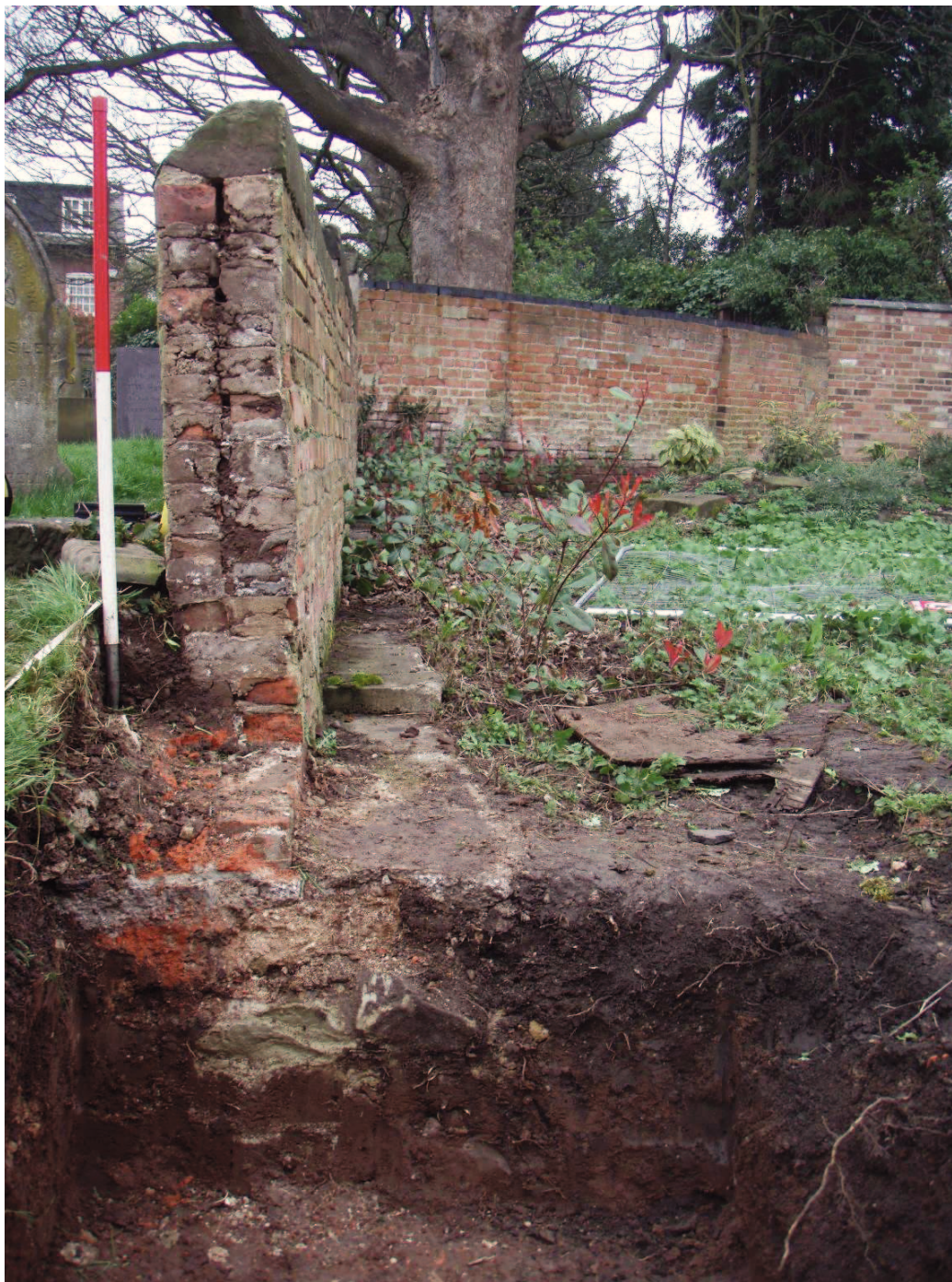
Photo 12 - East facing section through old boundary wall, looking west
