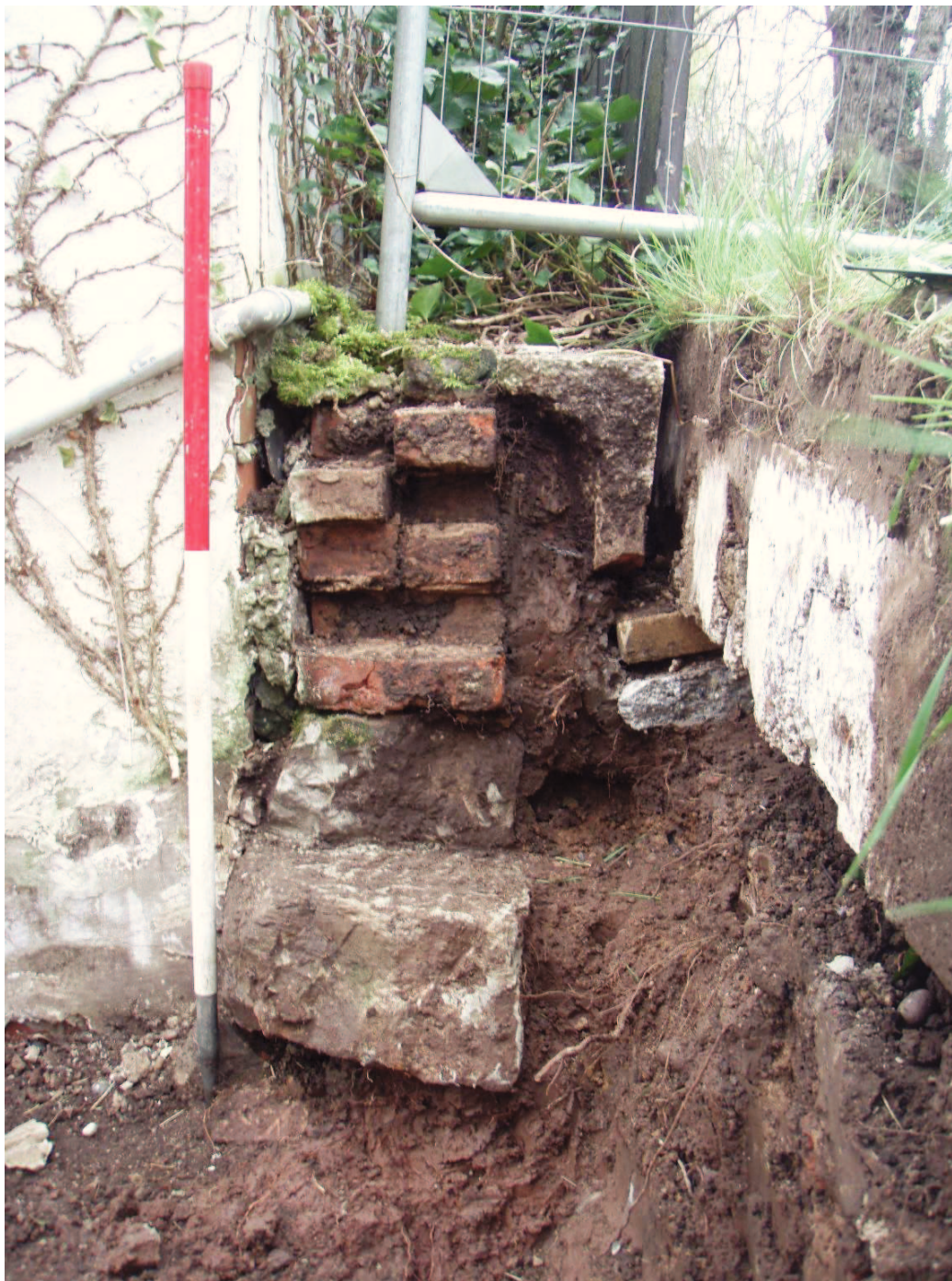
Photo 8 - West facing section through old boundary wall, looking east
