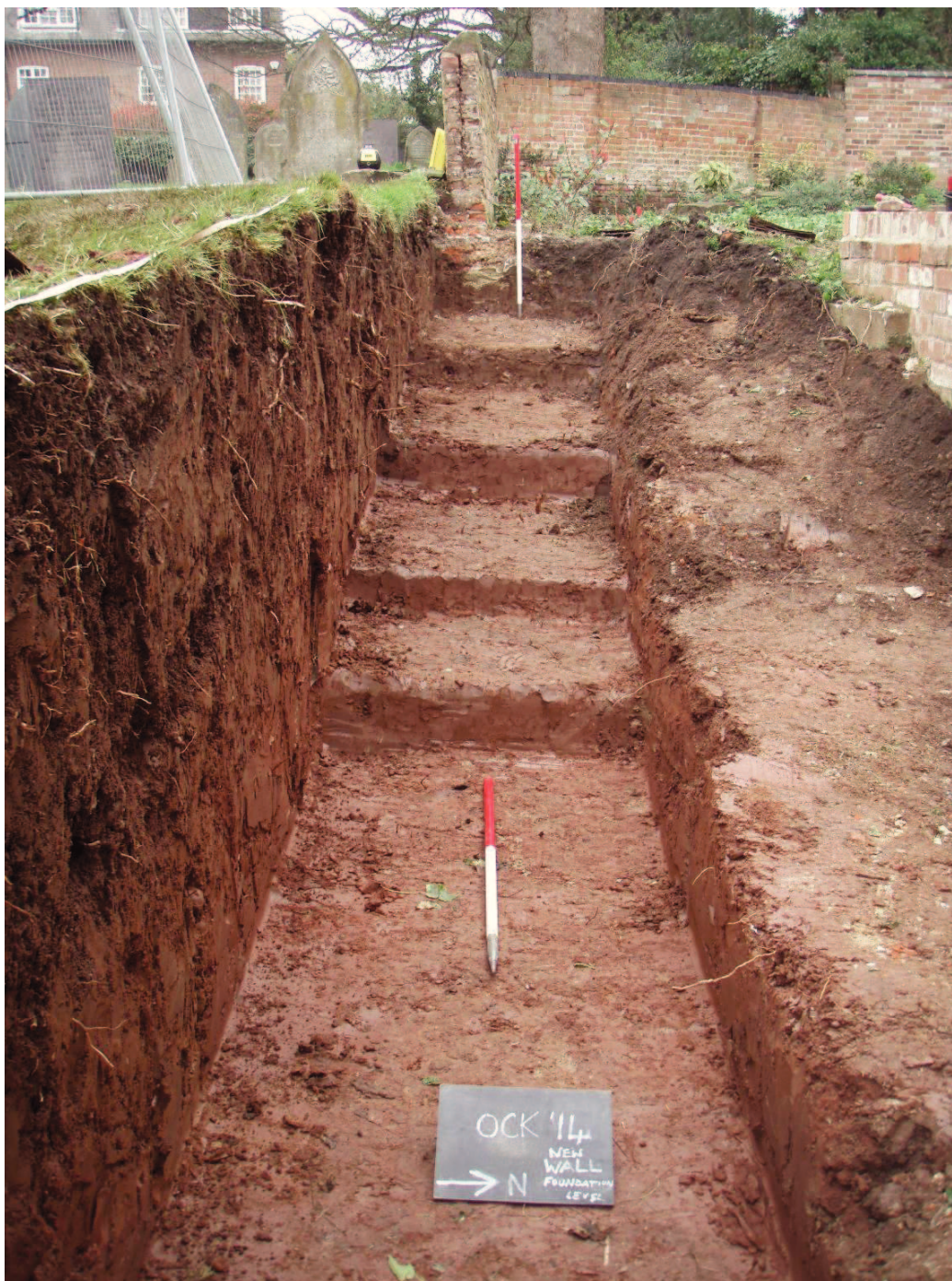
Photo 15 - Bottom of trench ready for footings of new wall, looking west
