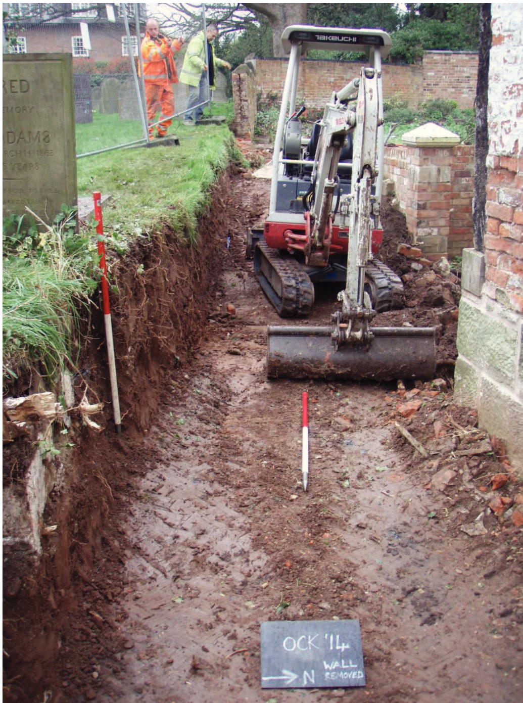
Photo 11 - Western end of site with wall removed, looking west
