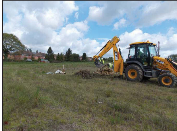
Working shot of the excavation of Trench 1.
