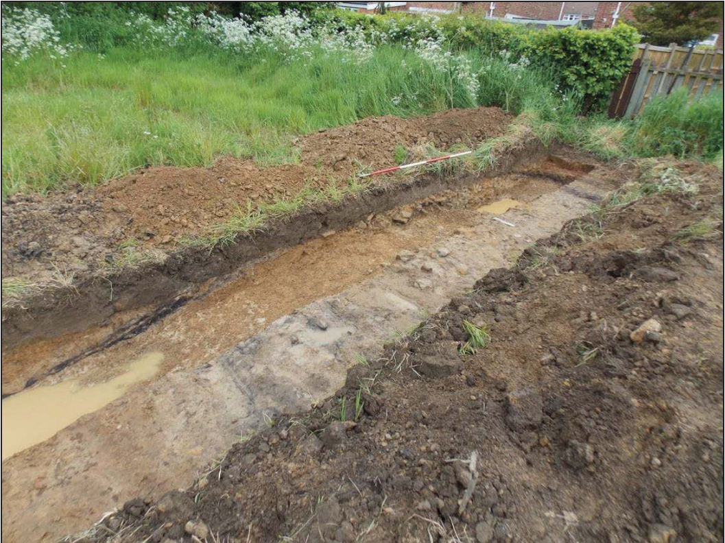
Figure 22. Investigation slot into the possible Roman road. Scale 2m.
