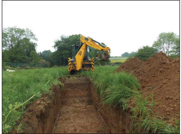
Working shot of the excavation of Trench 1.
