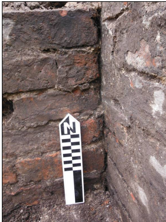
Figure 28. Internal partition wall (212) and 'front' wall (202), Trench 2. Note the mis-alignment of the courses of the walls, and the difference in bricks used. The implication is that wall (202) was constructed at an earlier date, before walls (212) were added. Scale = 0.25m.
