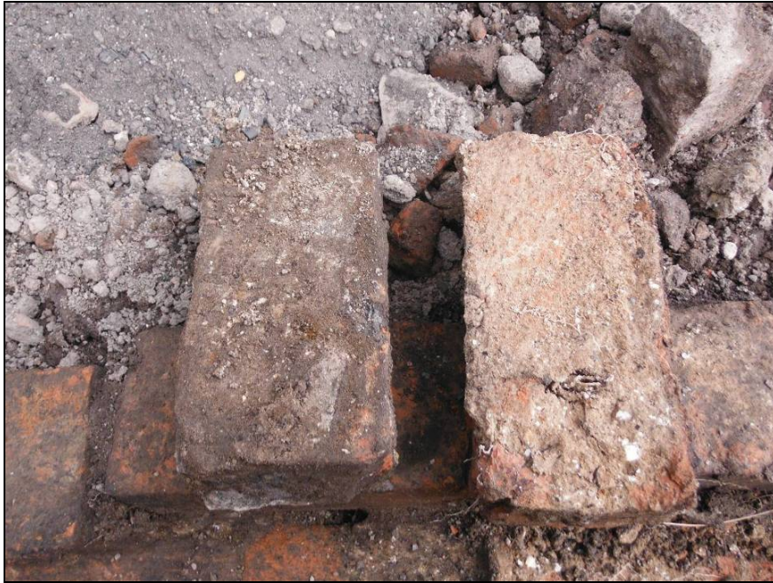
Figure 29. The brick on the left is taken from wall (202), whilst that on the right from internal partition walls (212), Trench 2. The difference in colour of both the bricks and the mortar suggest different construction events.
