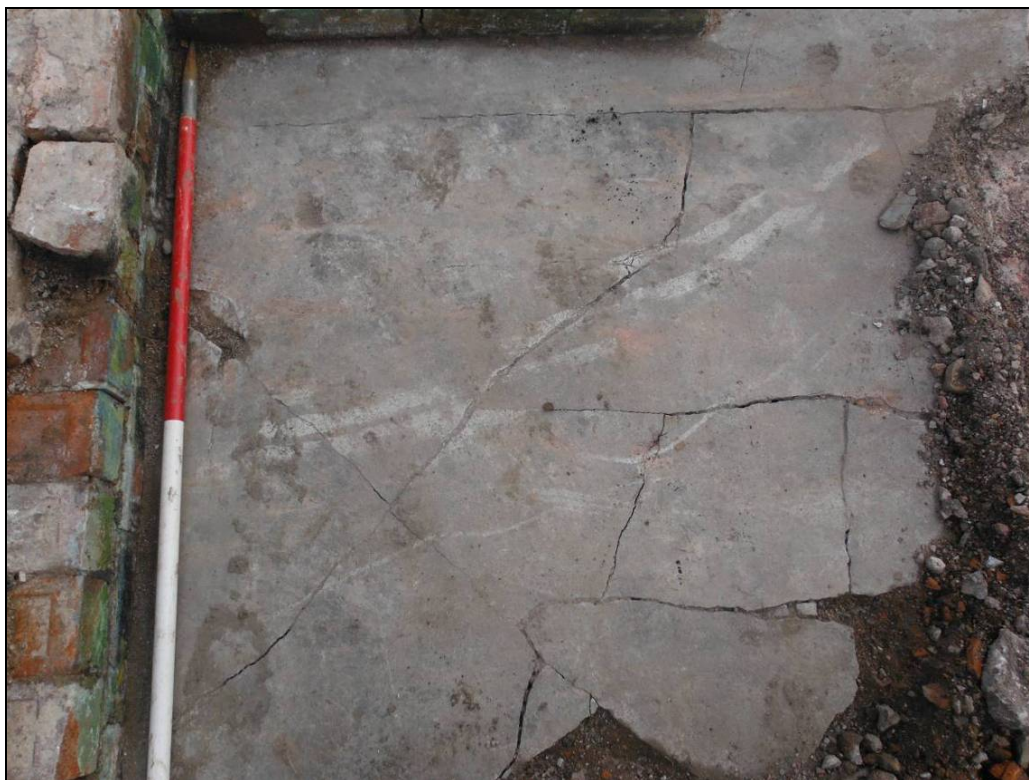
Figure 50. Evidence of a heavy door having existed over concrete floor (414), Trench 4. Scale = 1m.
