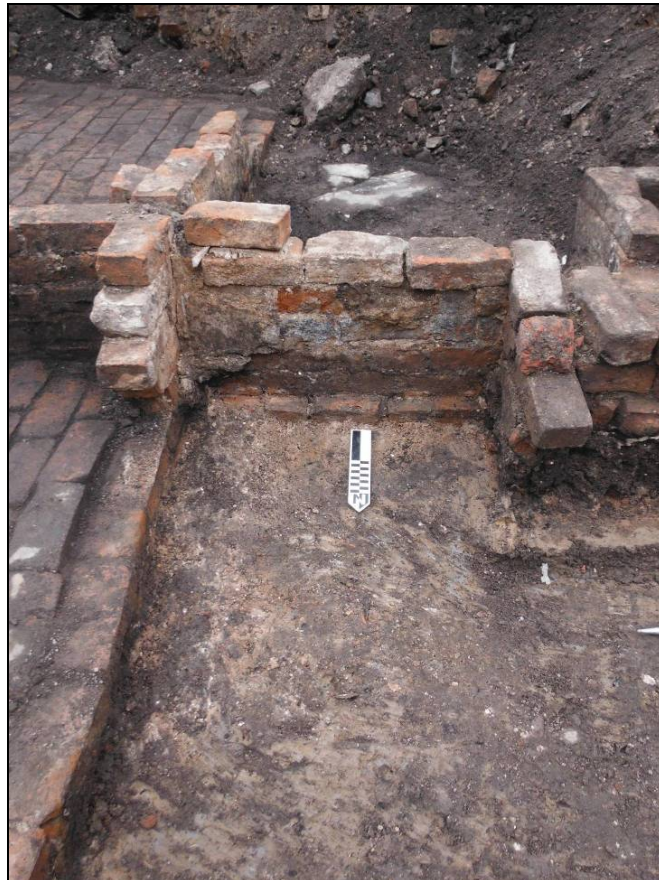
Figure 18. Internal partition walls (212) resting upon the natural clay, Trench 2. Scale = 0.25m.
