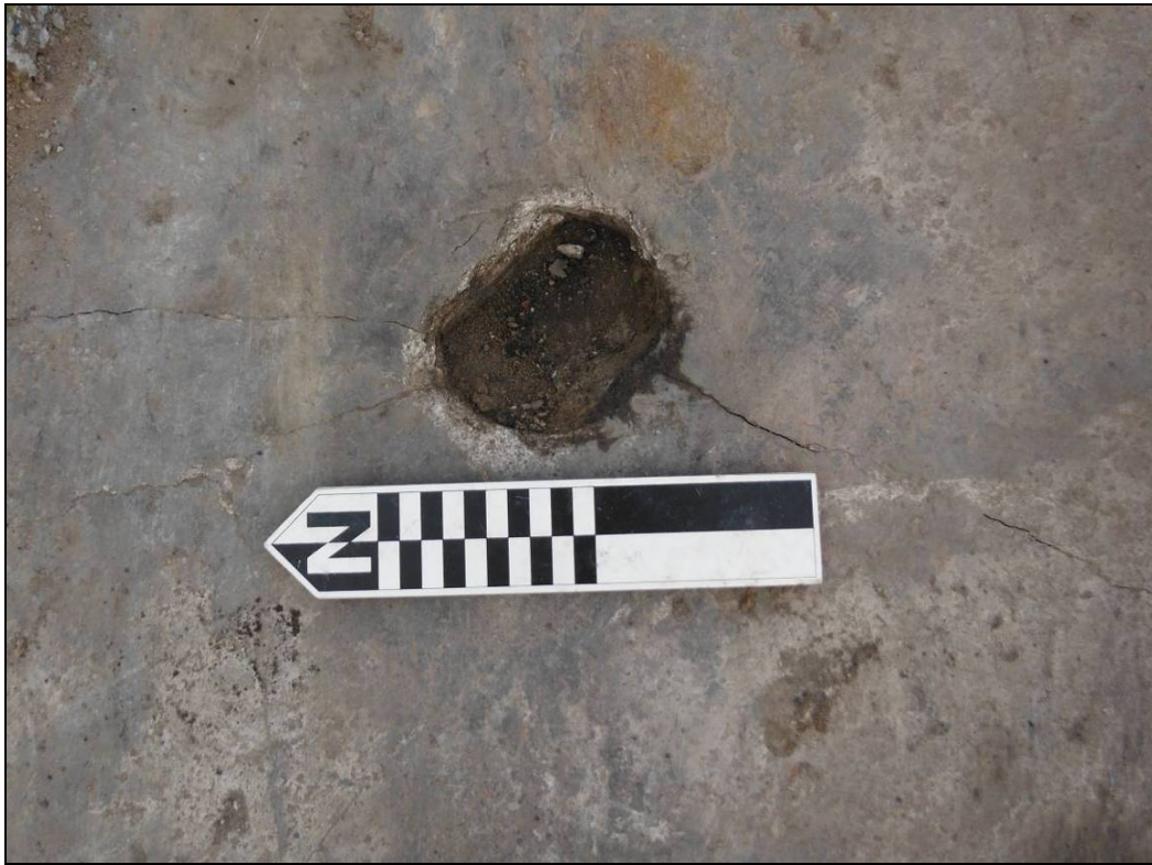
Figure 51. Possible fitting within concrete floor (414), Trench 4. Scale = 0.25m.
