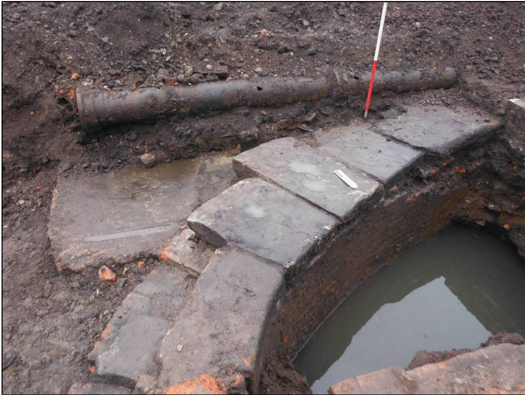
Figure 45. Wharf coping stones (404) with brick platform (402), Trench 4. Scale = 1m.
