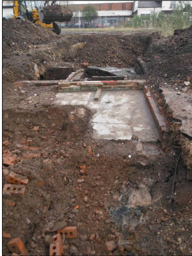
Figure 48. Walls (411) and (413) with concrete floor (414), Trench 4, post-exploratory sondage. Note that the curve of the canal wharf does not continue into this area. It is likely that the construction of the mill destroyed this area of the wharf – the area where the coping stones look as though they should continue was filled by Accrington Nori bricks, which post-date the construction of the wharf. Scale= 1m.
