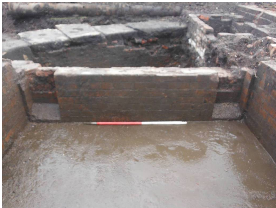
Figure 54. Southern end of structure (407) with the canal wharf coping stones (404) in the background, Trench 4. Scale = 1m.
