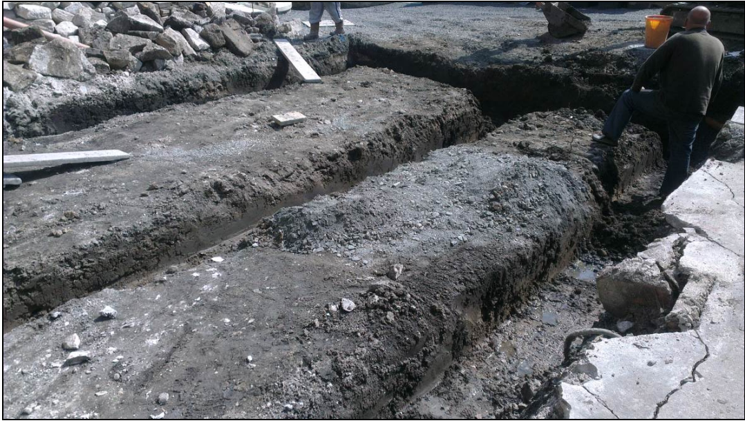
Figure 6. The excavation area and excavated foundation trenches, looking south.
