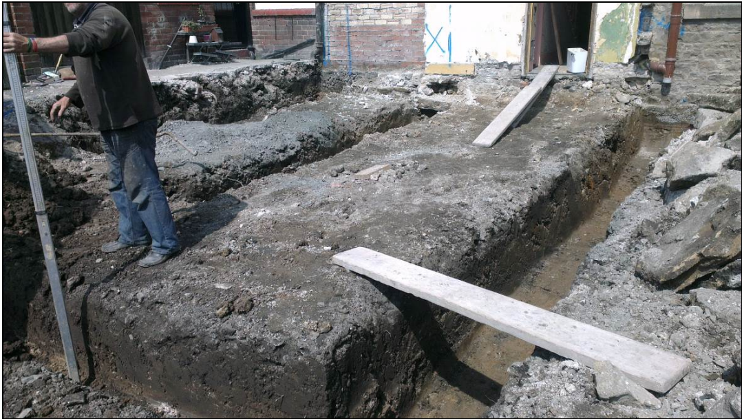
Figure 5. The excavation area and excavated foundation trenches, looking north.
