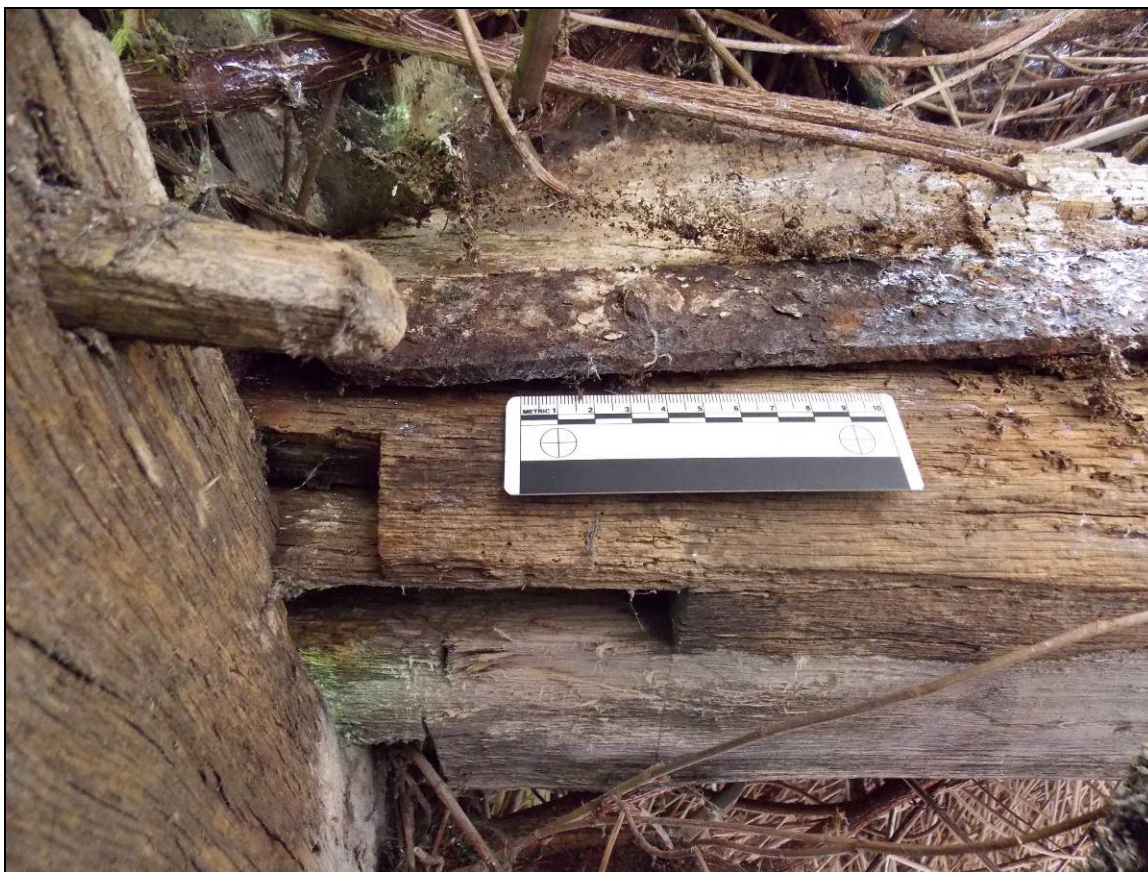
Plate 57: Eastern end of truss with vacant mortice, looking south (scale 300mm).
