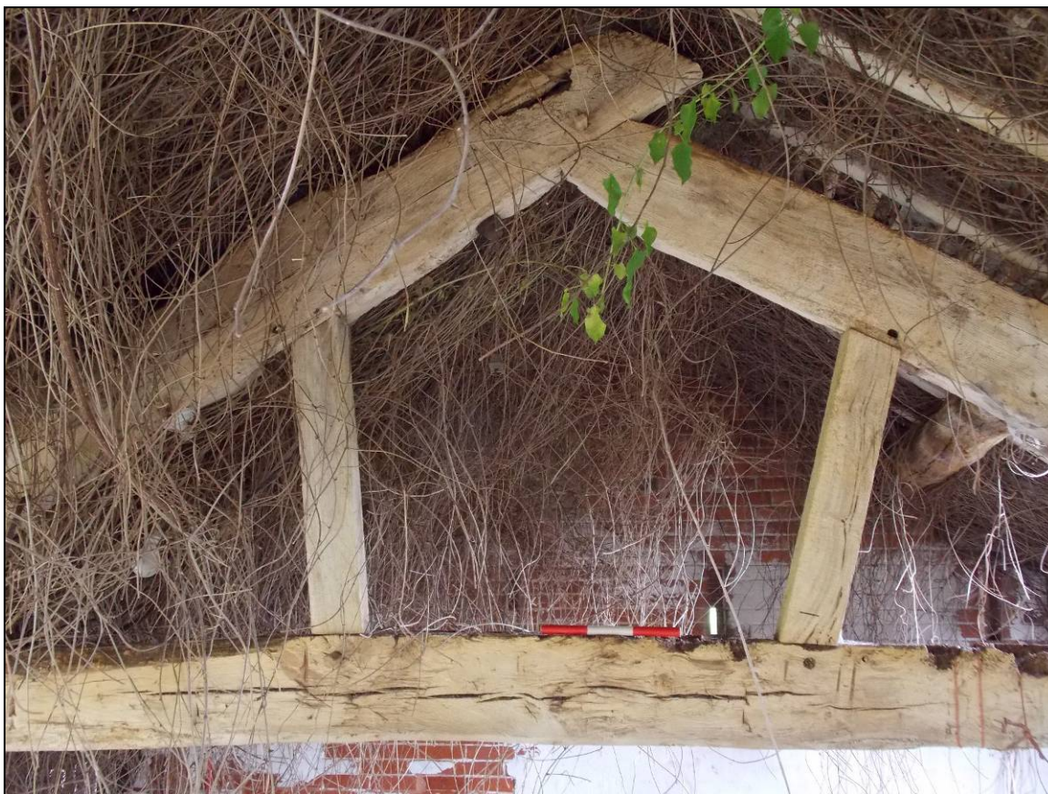
Plate 52: Detail of later raking struts, looking south (scale 300mm).
