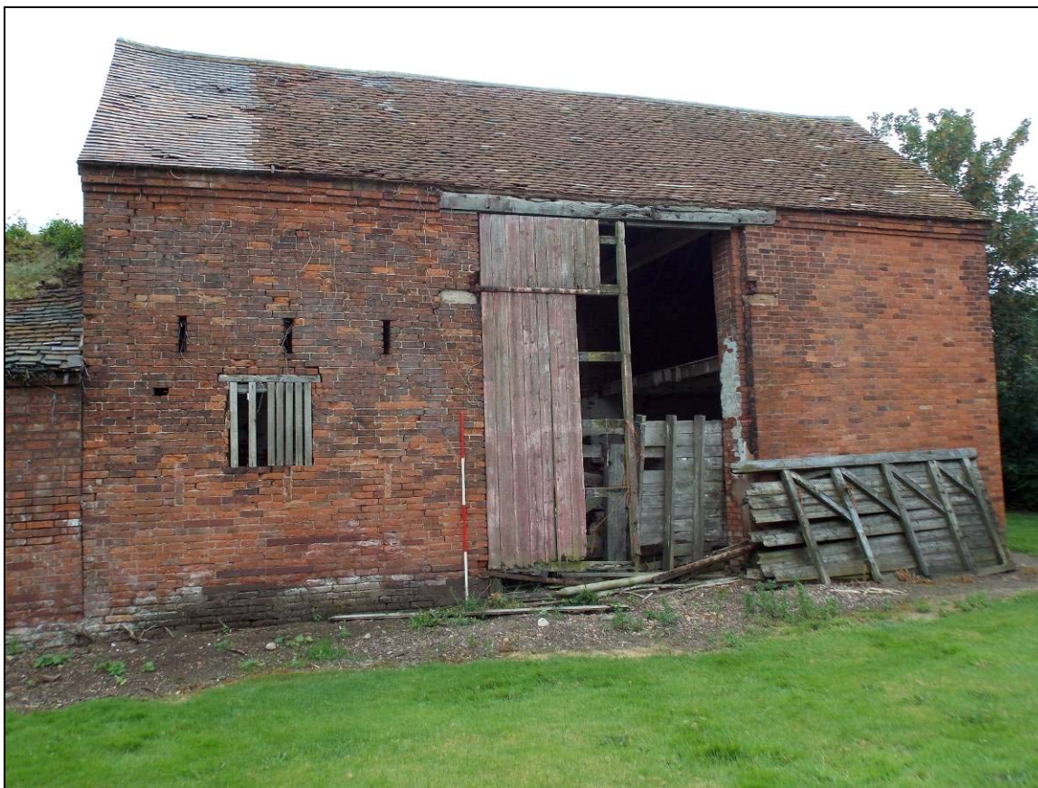
Plate 9: West elevation of Building A, looking east (scale 2m).
