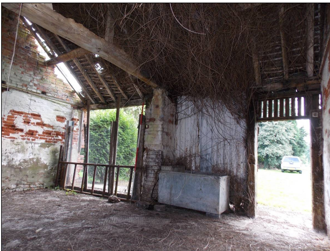
Plate 44: General view of the east wall, looking north-east (scale 2m).
