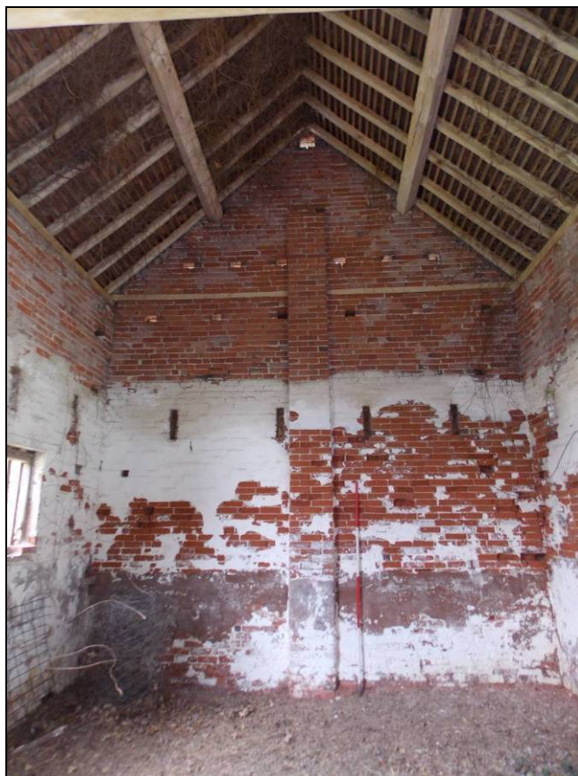
Plate 27: General view of the internal northern bay, looking north (scale 2m).
