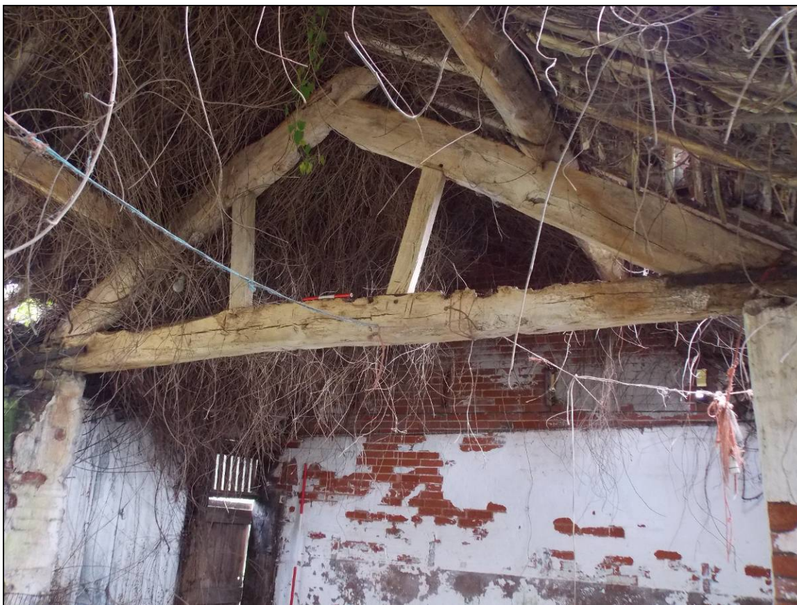
Plate 51: General view of the timber truss, looking south-east (scale 300mm).
