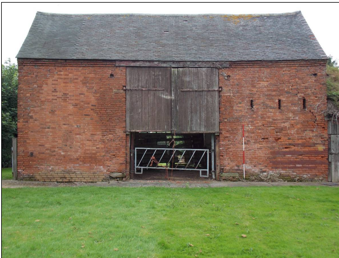
Plate 3: East elevation of Building A, looking west (scale 2m).
