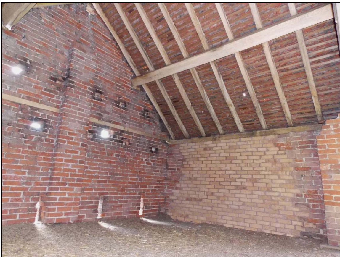
Plate 37: First floor of the internal southern bay, looking south-west.
