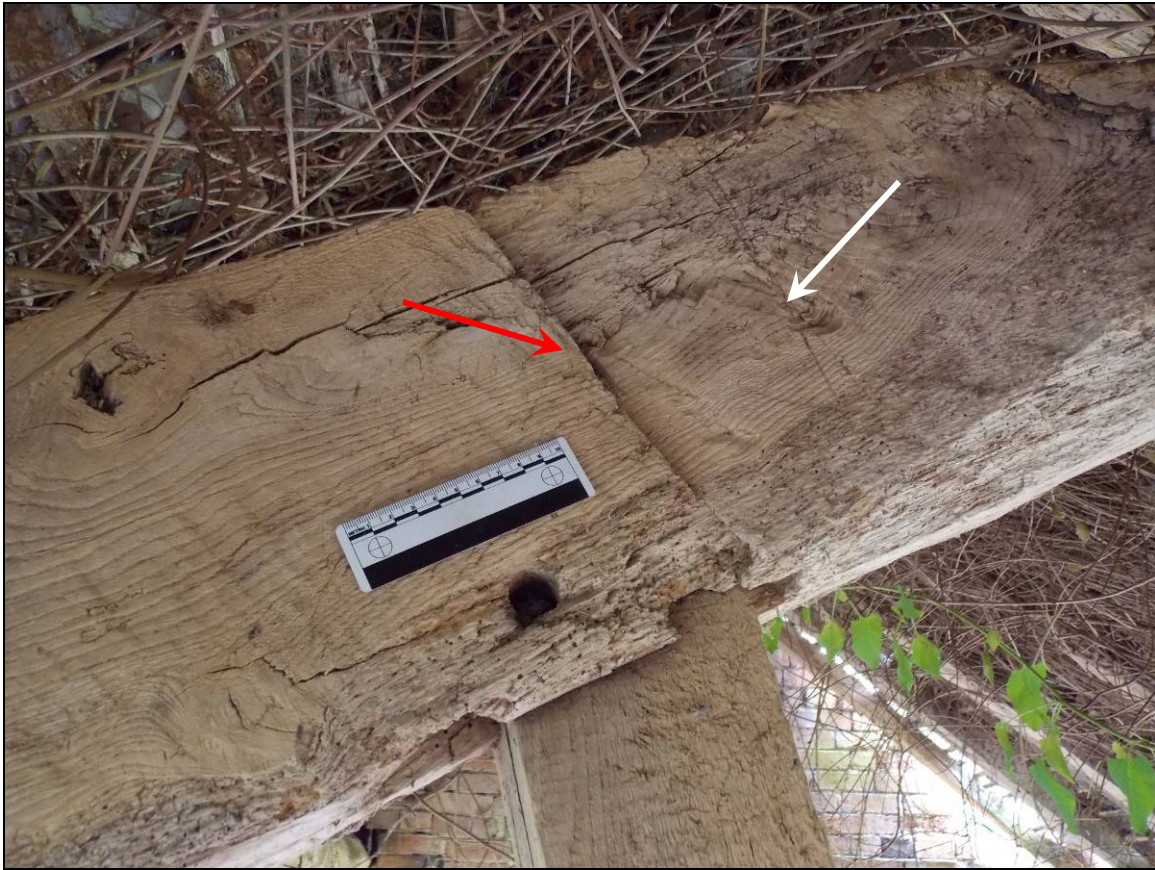
Plate 58: Detail of pit-sawn scar (red arrow) and levelling incised mark (white arrow) (scale 100mm).
