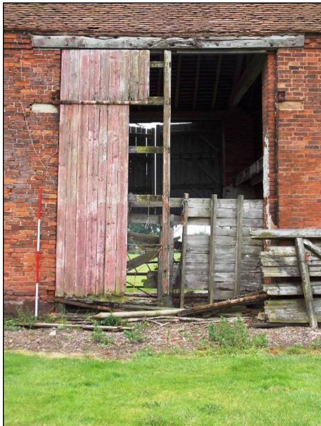
Plate 11: Central bay of the west elevation, looking east (scale 2m).
