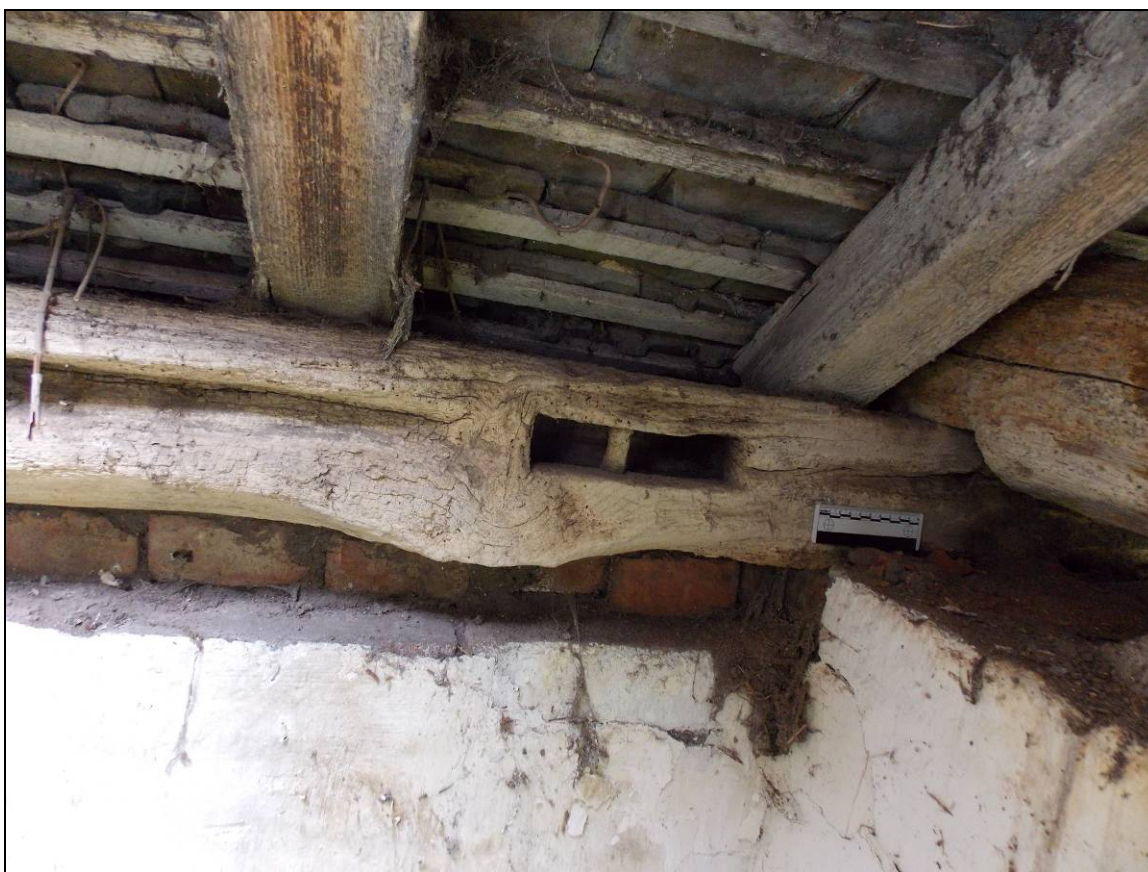
Plate 56: Reused wall plate with stave groove and empty mortice, looking west (scale 100mm).
