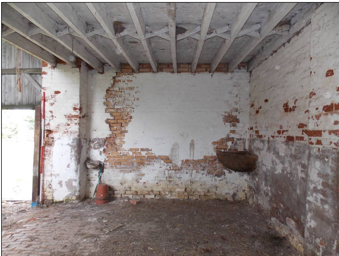
Plate 22: Southern side of the internal east wall, looking east (scale 2m).
