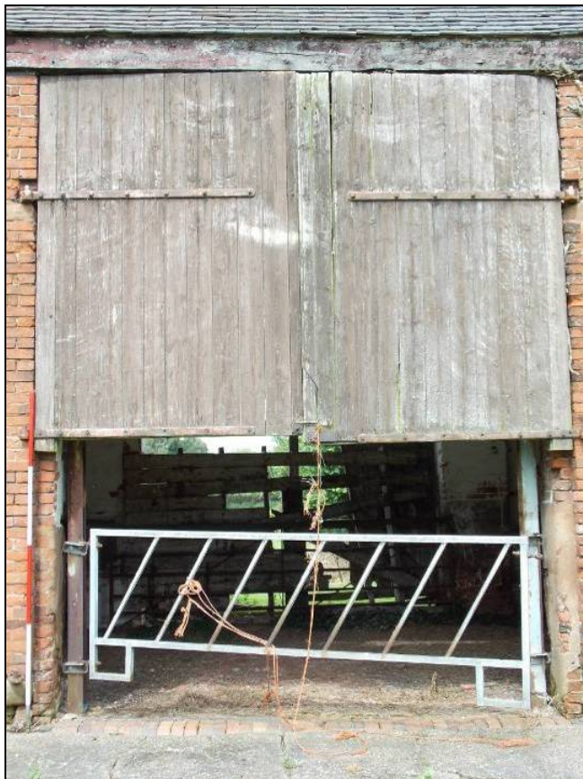
Plate 5: Central bay of the east elevation, looking west (scale 2m).
