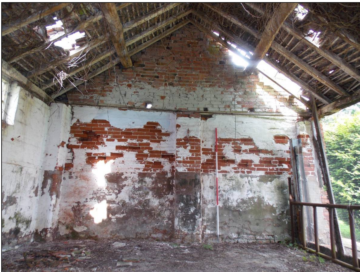
Plate 47: North wall with later brickwork within the gable (scale 2m).
