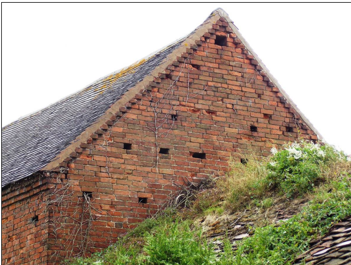
Plate 14: Gable wall of the north elevation, looking south-west.
