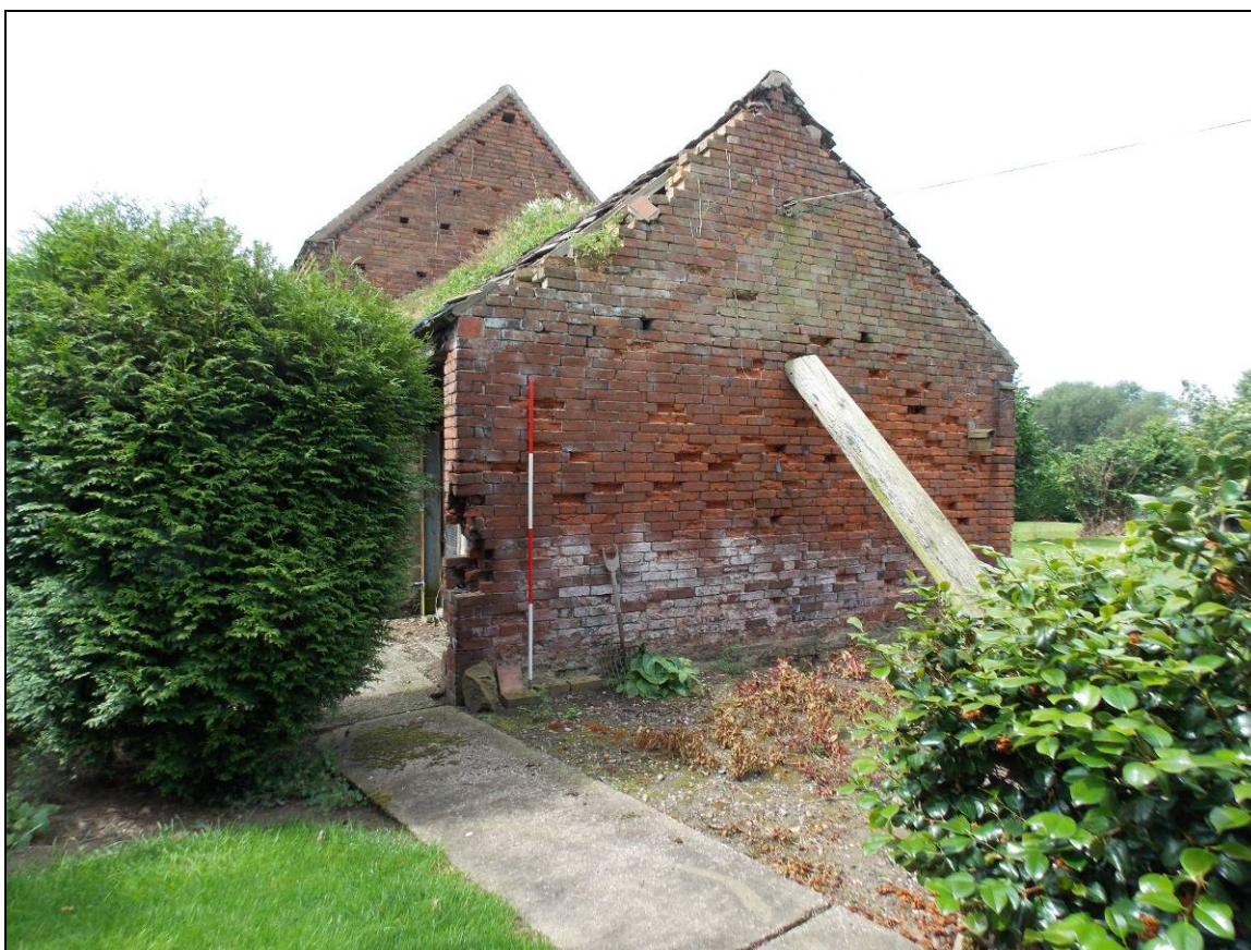
Plate 42: North elevation of Building B, looking south (scale 2m).
