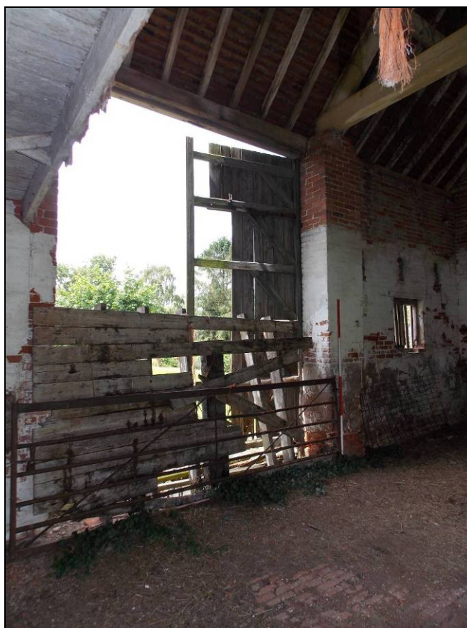
Plate 24: Central bay with western doorway, looking north-west (scale 2m).
