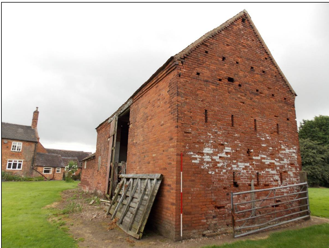
Plate 15: General view of the south elevation, looking north-east (scale 2m).
