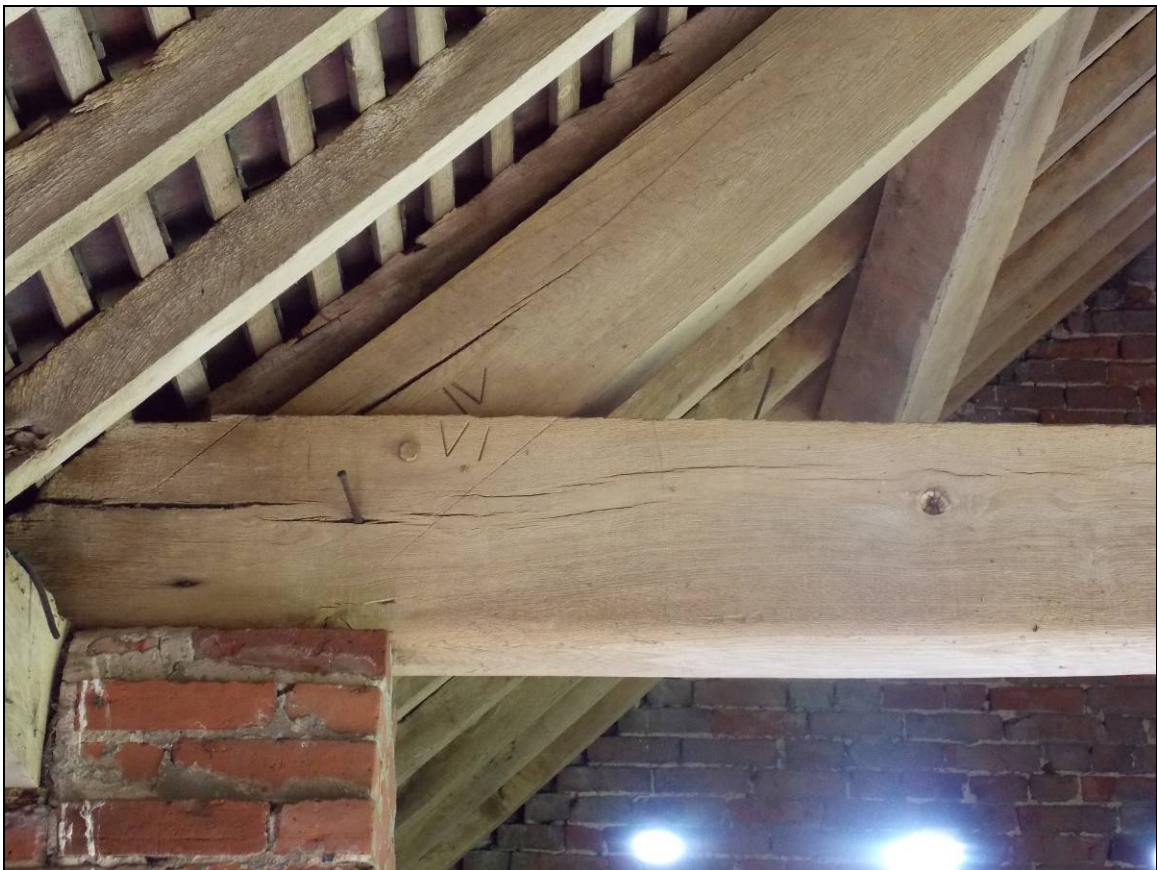
Plate 31: Carpenter's marks within the eastern end of the tie-beam and principal rafter of truss I, looking south.
