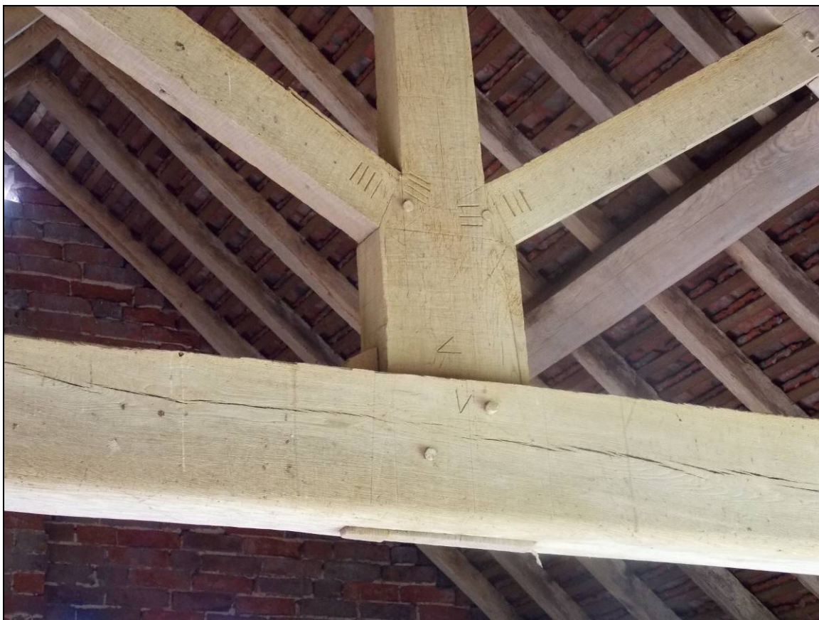
Plate 32: Truss I with several assembly carpenter's marks on the upper north face, looking south.
