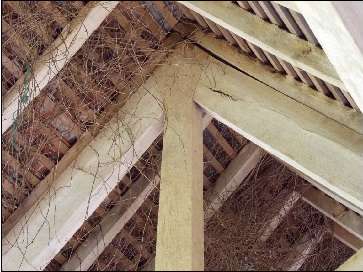
Plate 34: Detail of the upper section of truss II, looking north.
