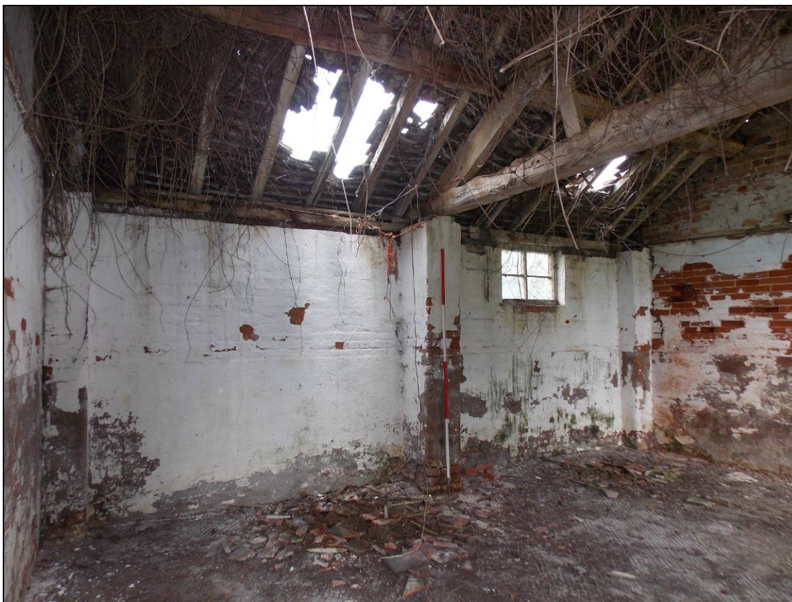
Plate 45: Internal west wall, looking north-west (scale 2m).
