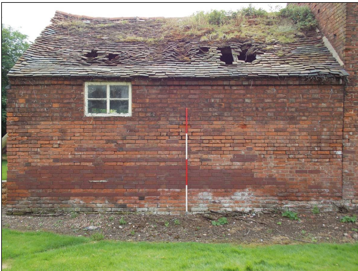
Plate 39: West elevation of Building B, looking east (scale 2m).
