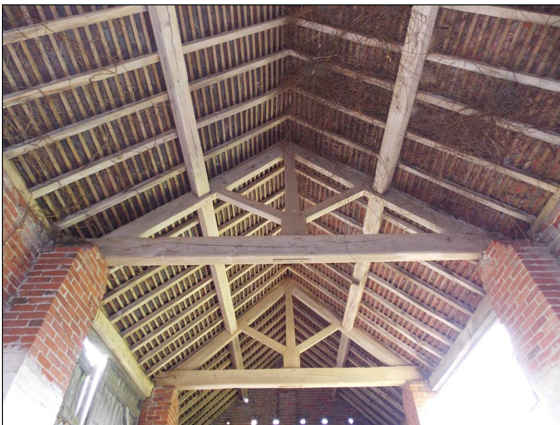
Plate 28: General view of the roof structure, looking south.
