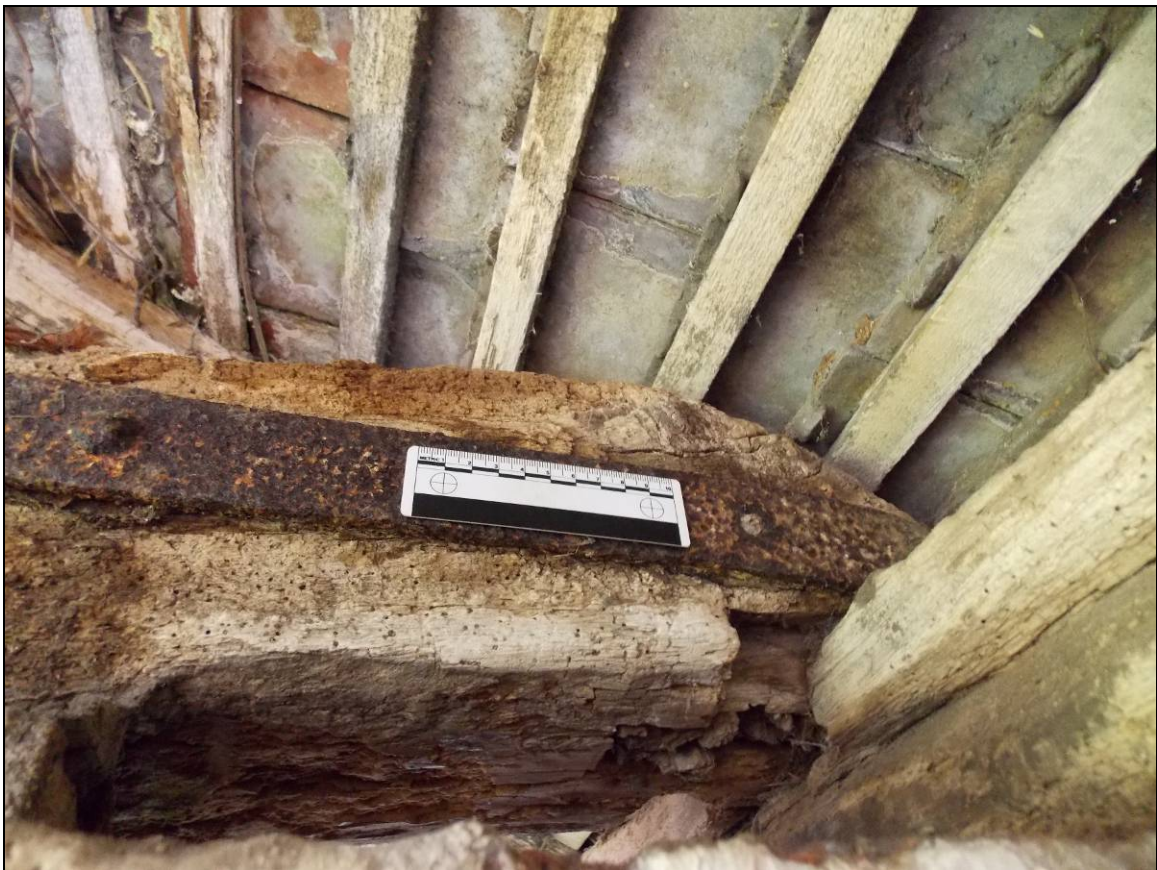
Plate 55: Detail of western mortice with partially decayed split tenon, looking south (scale 100mm).
