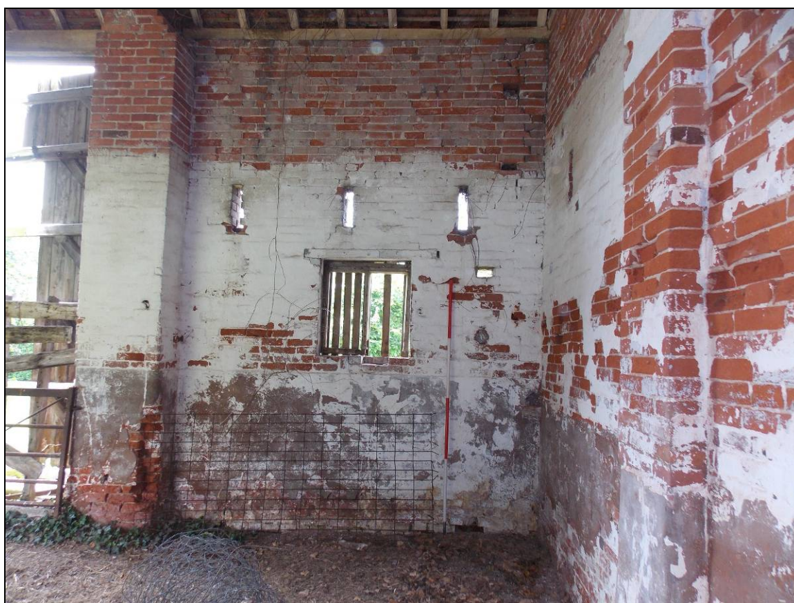
Plate 25: Northern side of the internal west wall, looking west (scale 2m).
