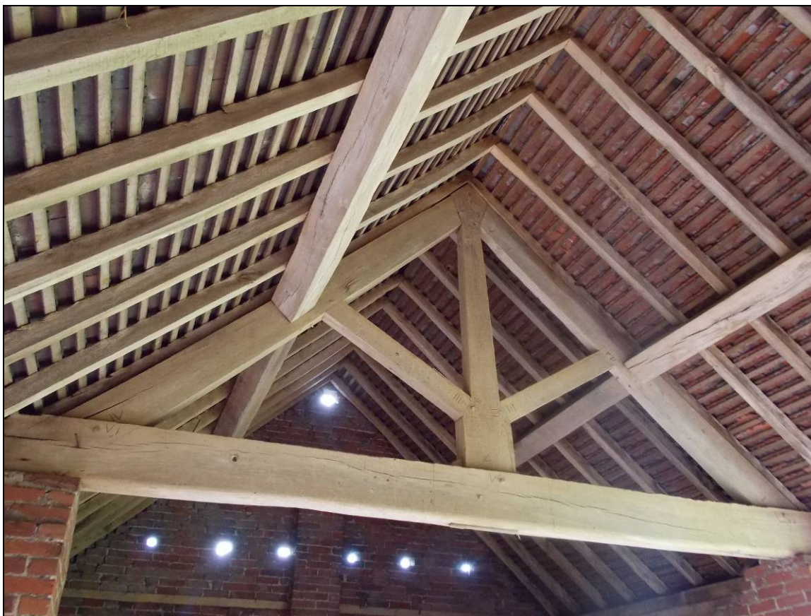
Plate 29: General view of truss I, looking south.
