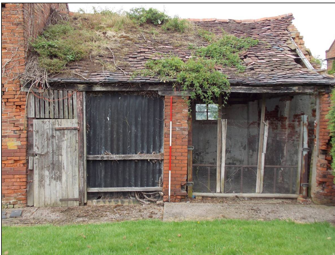
Plate 38: East elevation of Building B, looking west (scale 2m).
