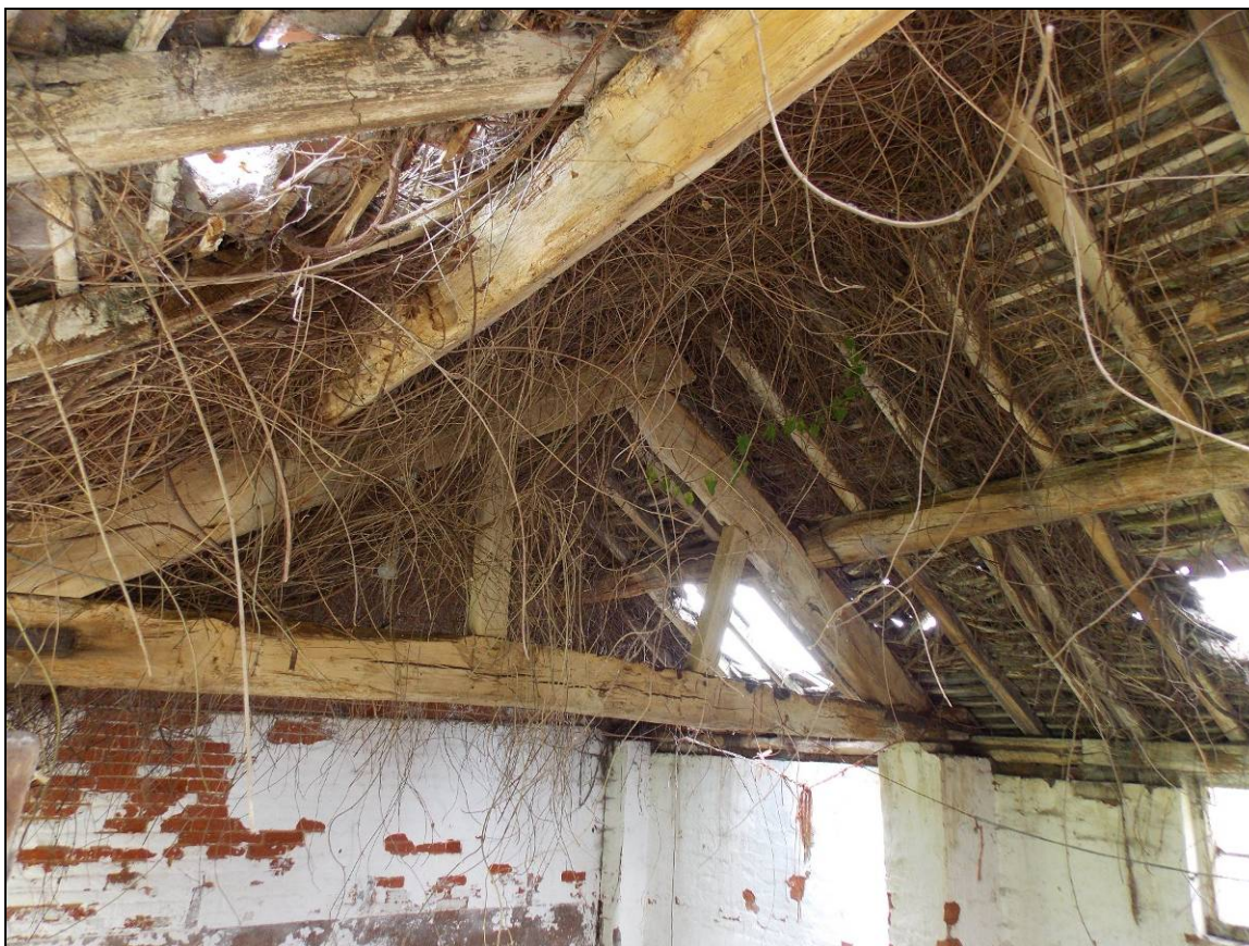
Plate 50: View of the roof structure, looking south-west.
