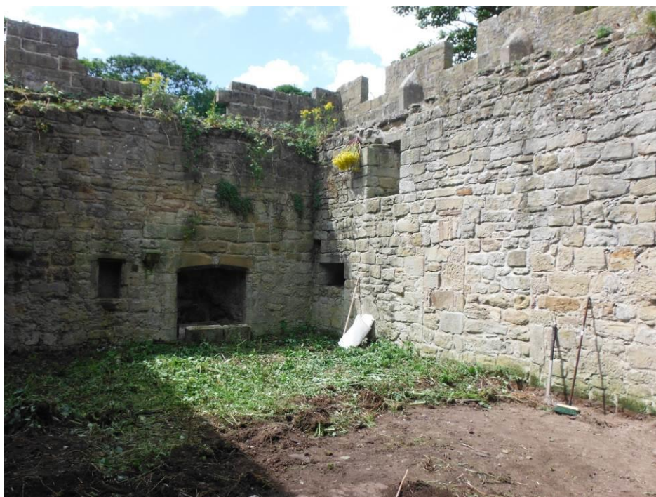
Figure 4: The first-floor during clearance of deposit (001), looking north-west.
