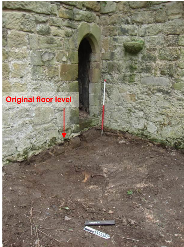
Figure 11: Rough rubble base to the west and south walls of the western chamber, marking the height of the previous floor level which must have been above the rubble section. Note also the height of the entrance to the latrine chamber. This floor level would have been higher than the level of the flag-stone floor in the eastern chamber (scale = 1m).
