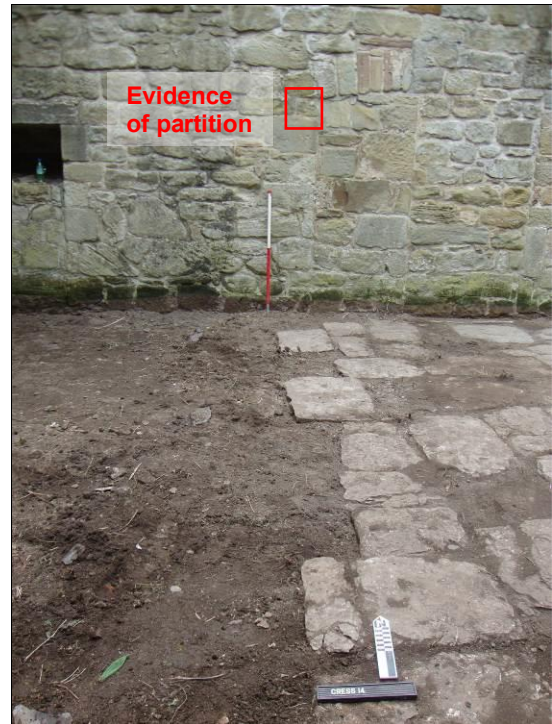
Figure 10: Extent of the surviving stone floor (002) in relation to the evidence in the north wall of a timber partition (scale = 1m).
