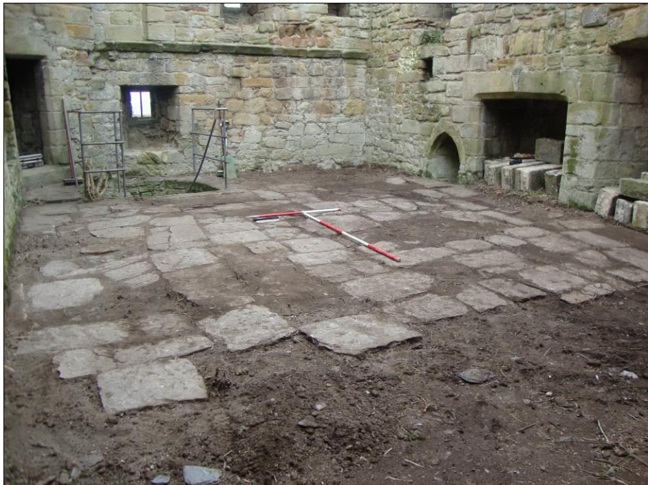
Figure 6: The first-floor level following clearance, showing the flag-stone surface (002), looking south-east (scale = 2m + 1m).
