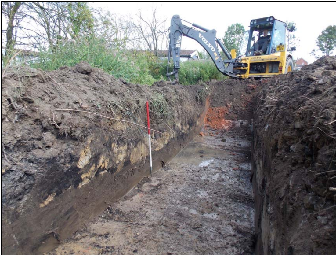
Figure 9: Eastern end of the trench (scale 1m).
