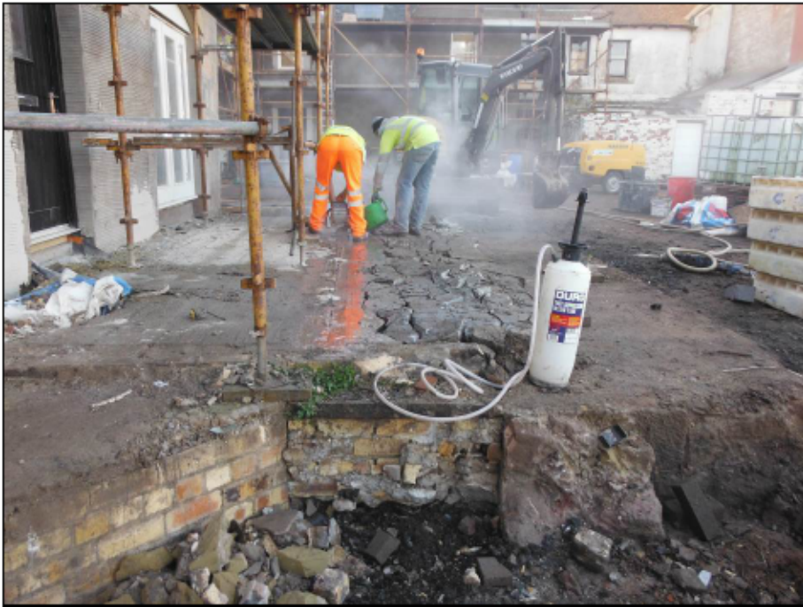
Figure 51 – Works in the vicinity of a previously identified 20 th century wall (215).
