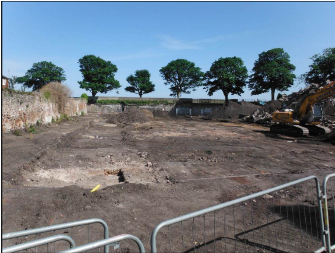
Figure 20 – Final stripped area to 49.325m OD.
