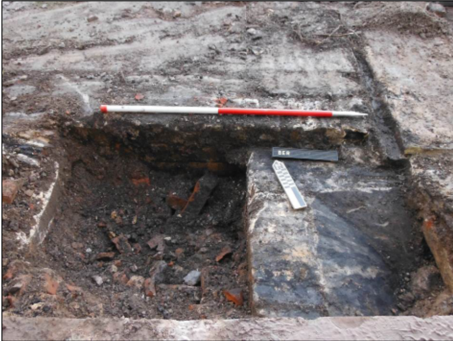
Figure 53 – 20 th century walling (215) on the right of the photograph with a concrete drainage gully behind feeding into a large stone drain. (Scale = 1m).
