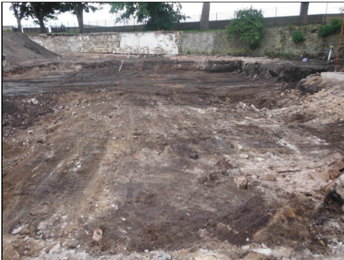
Figure 21 – 16x26m Stripped Area to South of Site.
