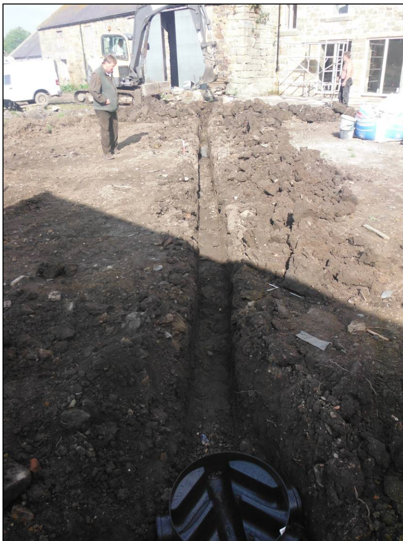
Figure 3. North-west facing view of pipe trench.
