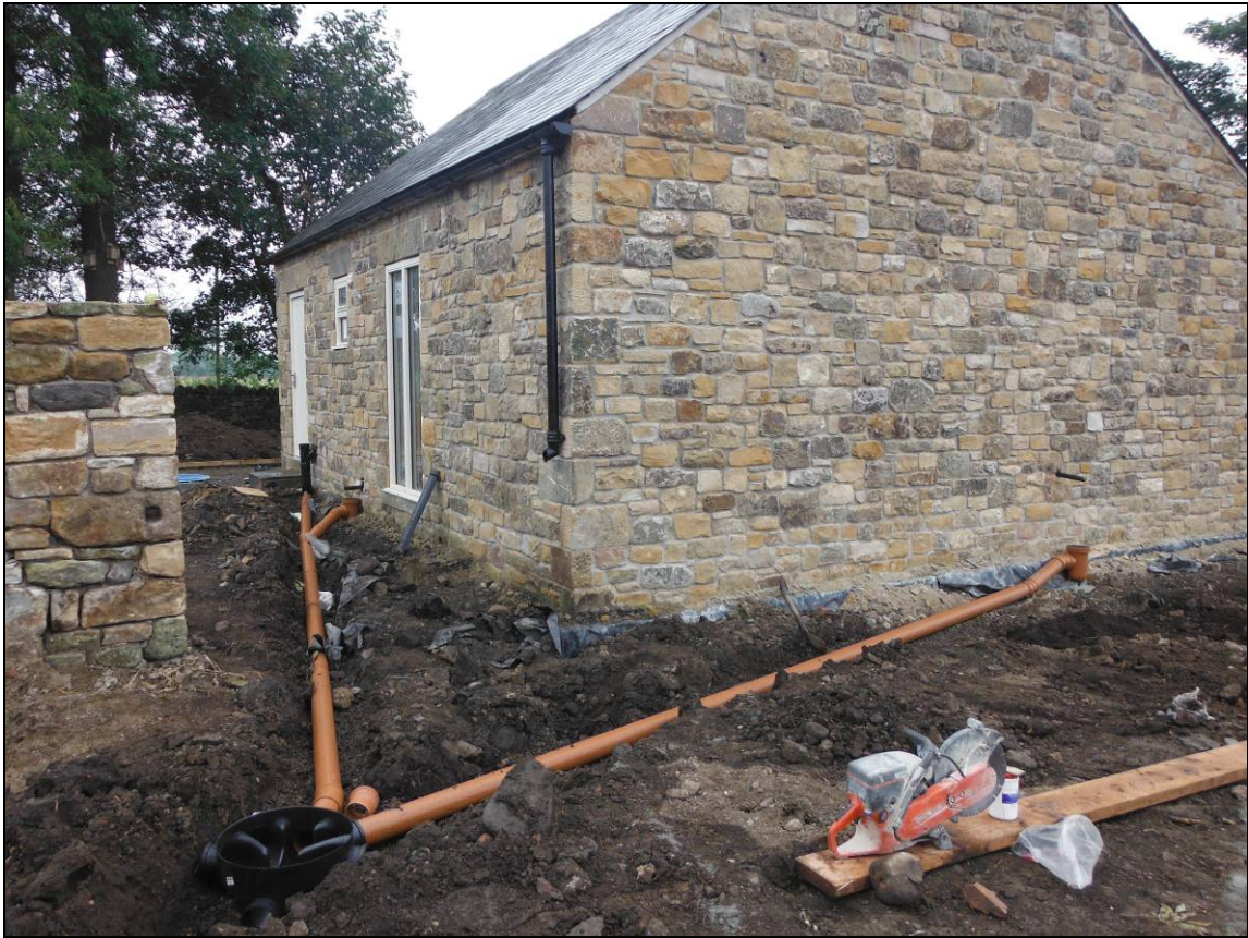
Figure 5. South-east facing view of in-situ pipe trenches.
