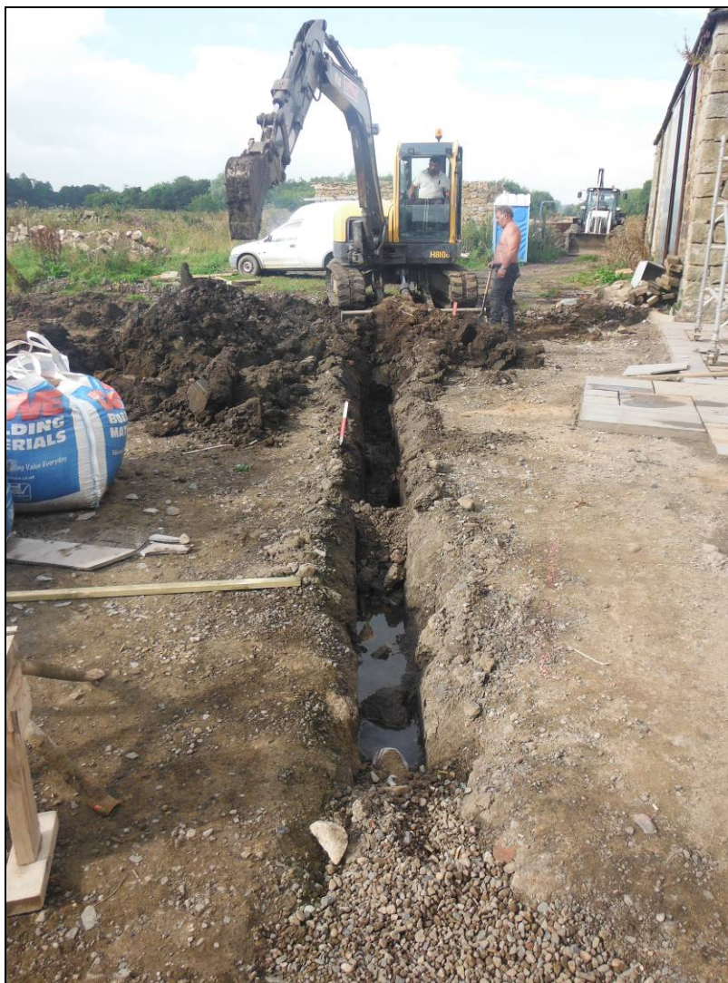
Figure 4. West facing view of pipe trench.
