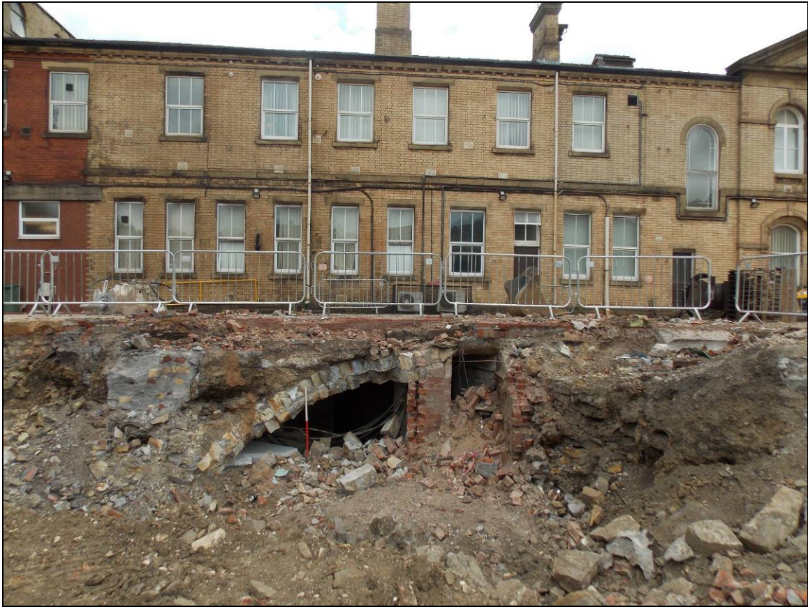
Figure 3: General view of the Air Raid Shelter, looking north-east (scale 1m).
