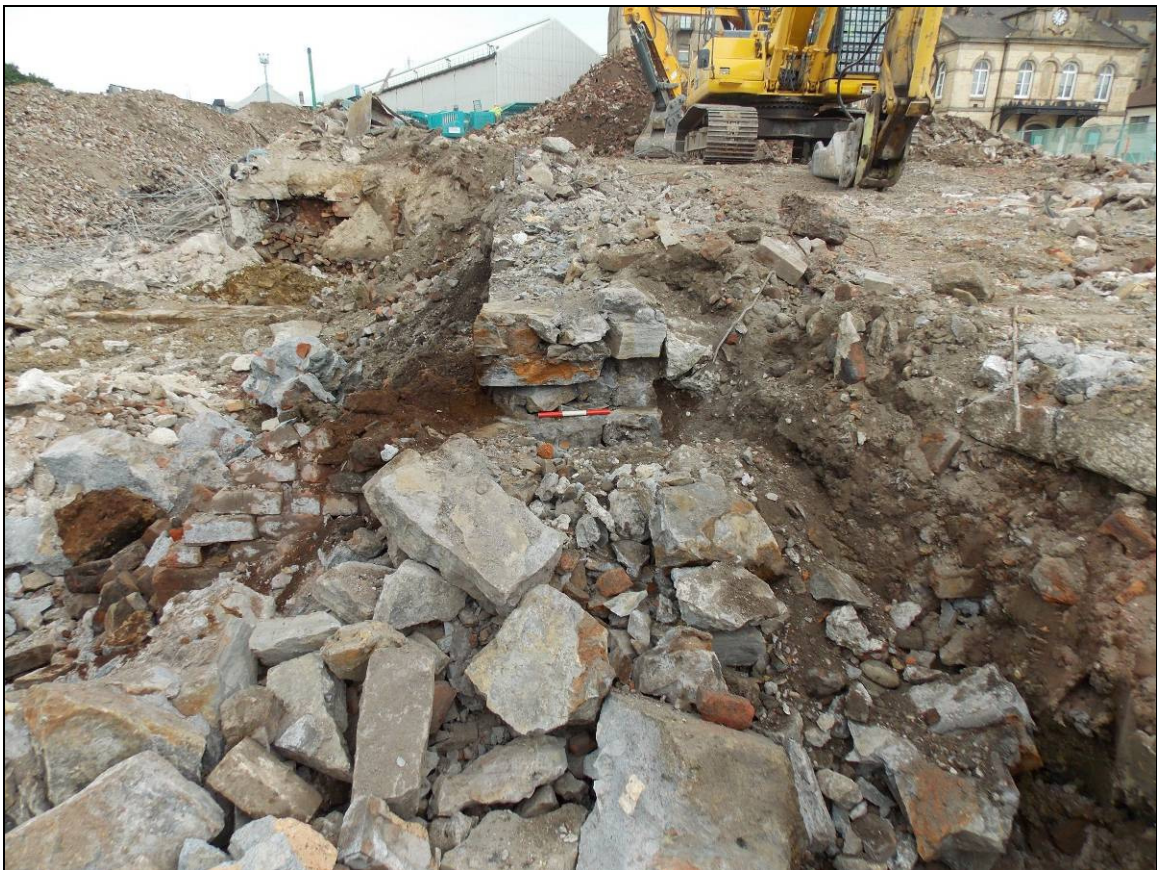
Figure 27: Sectional view of wall (119), looking north-west (scale 30mm).
