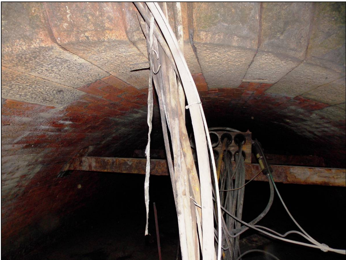
Figure 47: Arch's extrado and internal view of the vaulted chamber, looking west.
