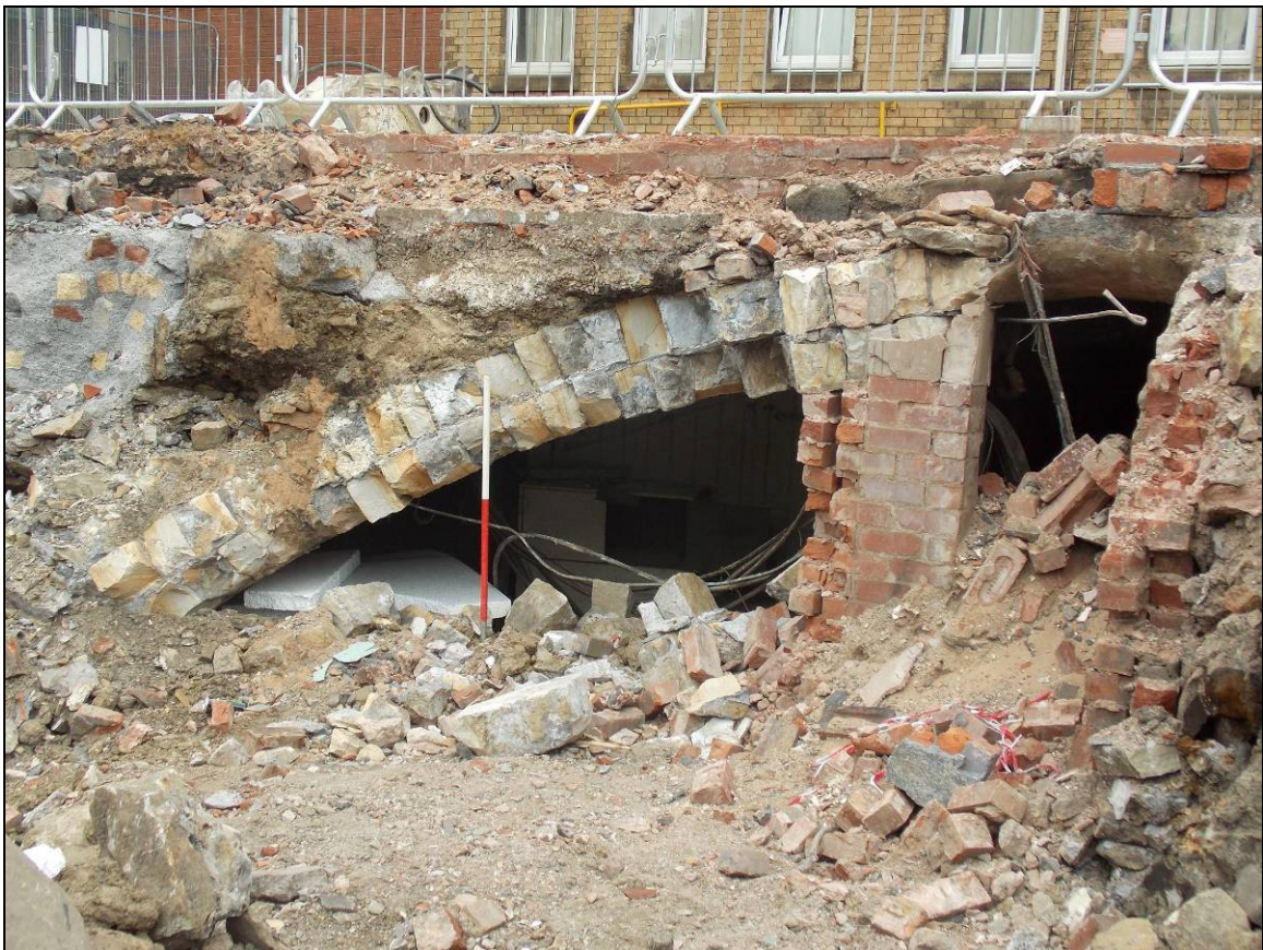
Figure 4: Vaulted stone chamber (101) and brick shaft (102), looking north-east (scale 1m).
