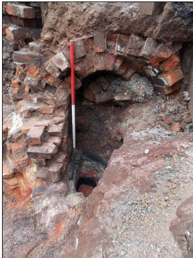
Figure 18: Arched chimney flue (113), looking east (scale 1m).
