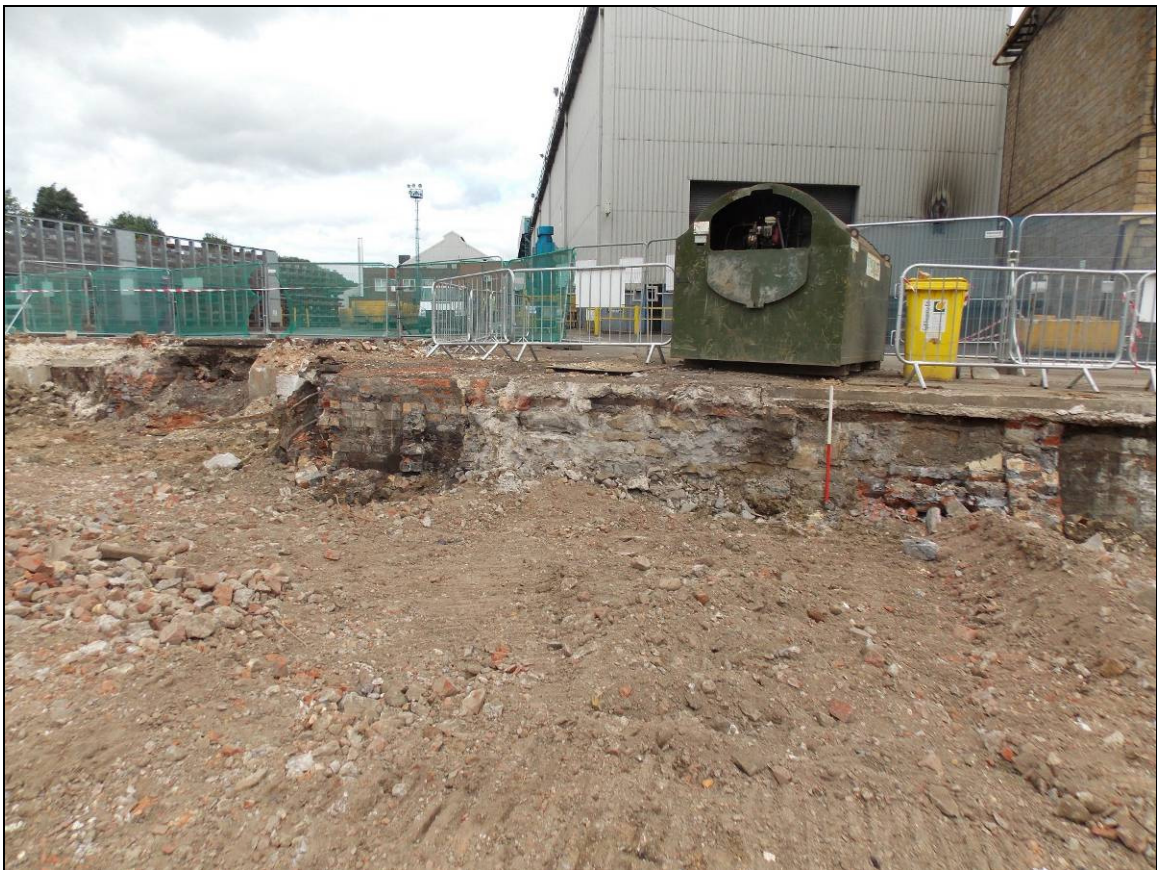
Figure 7: Sandstone wall (103) with truncated brick return (106), looking west (scale 1m).
