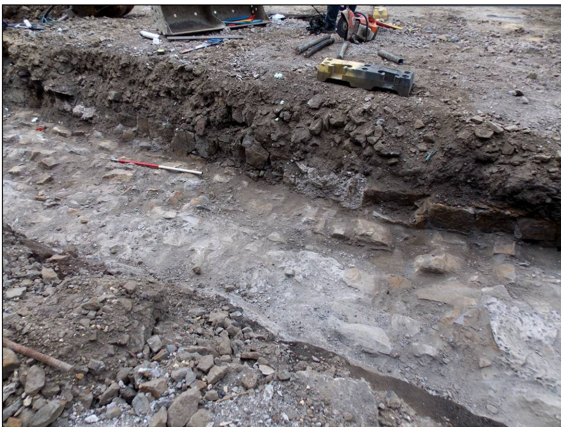
Figure 41: Detail of the culvert's masonry, looking north (scale 1m).
