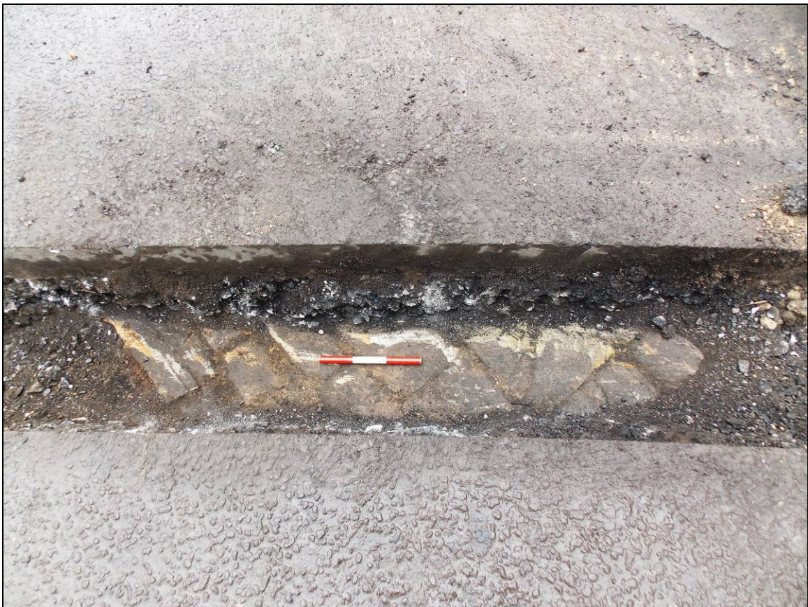
Figure 43: Remains of an earlier road surface, looking south-west (scale 300mm).
