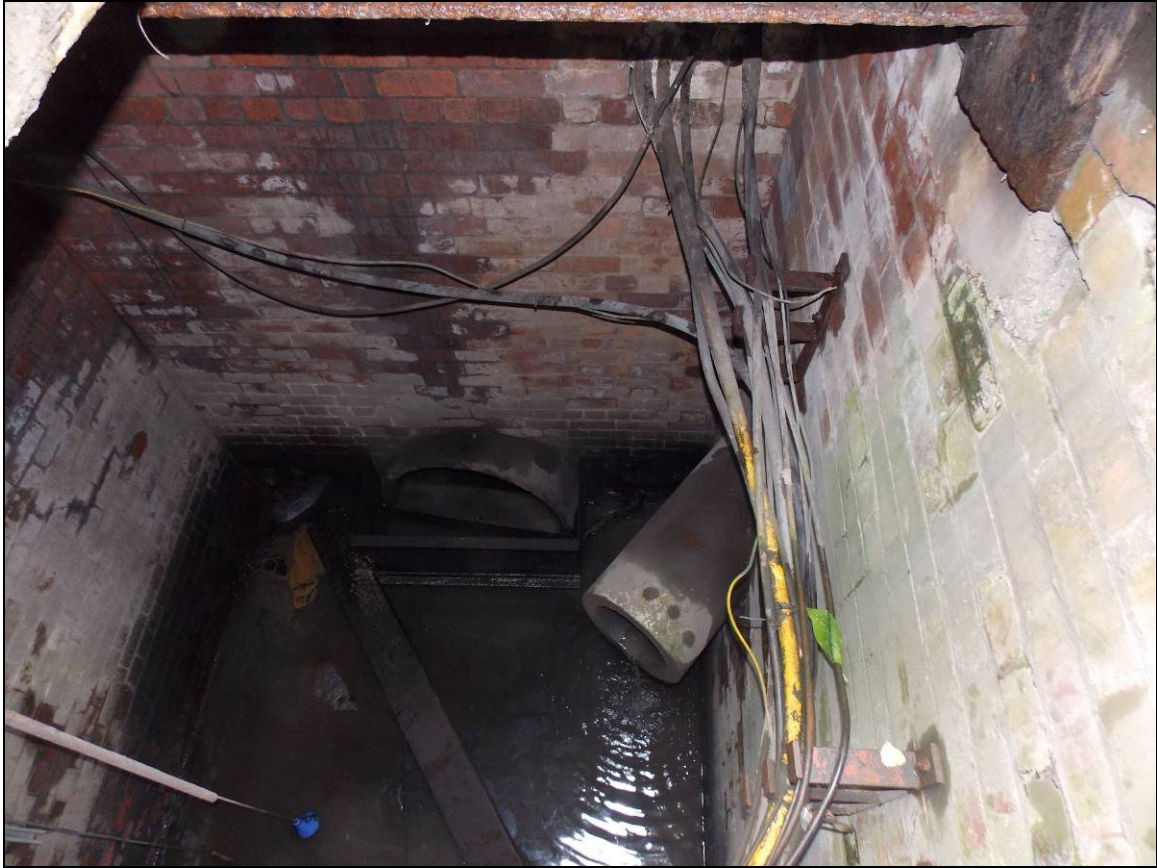
Figure 44: General view of the manhole, looking east.
