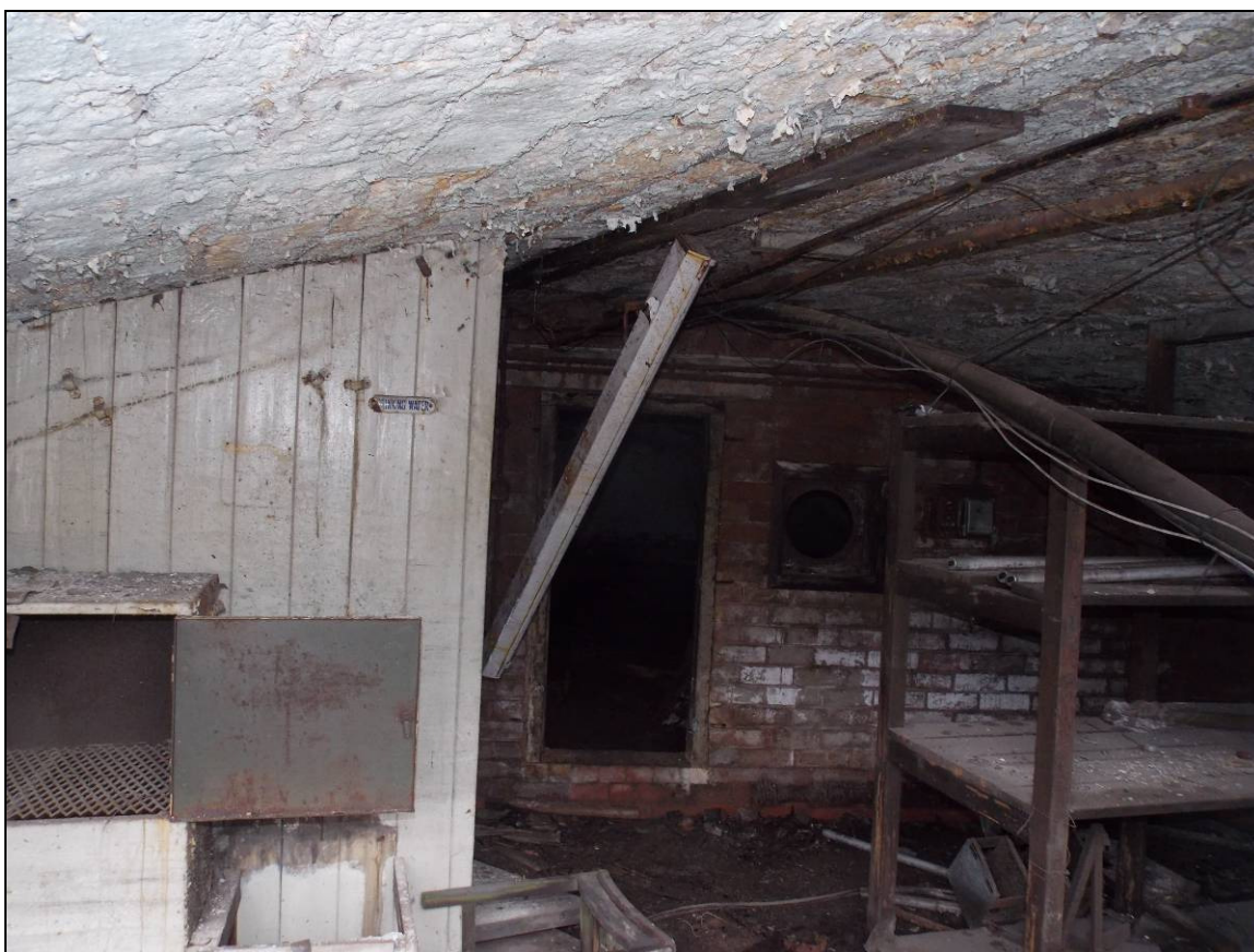
Figure 5: Detail of the interior, looking north-east.
