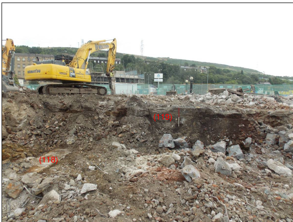
Figure 23: General view of sandstone wall (119) with a later partition wall (118), looking north-east (scale 1m).
