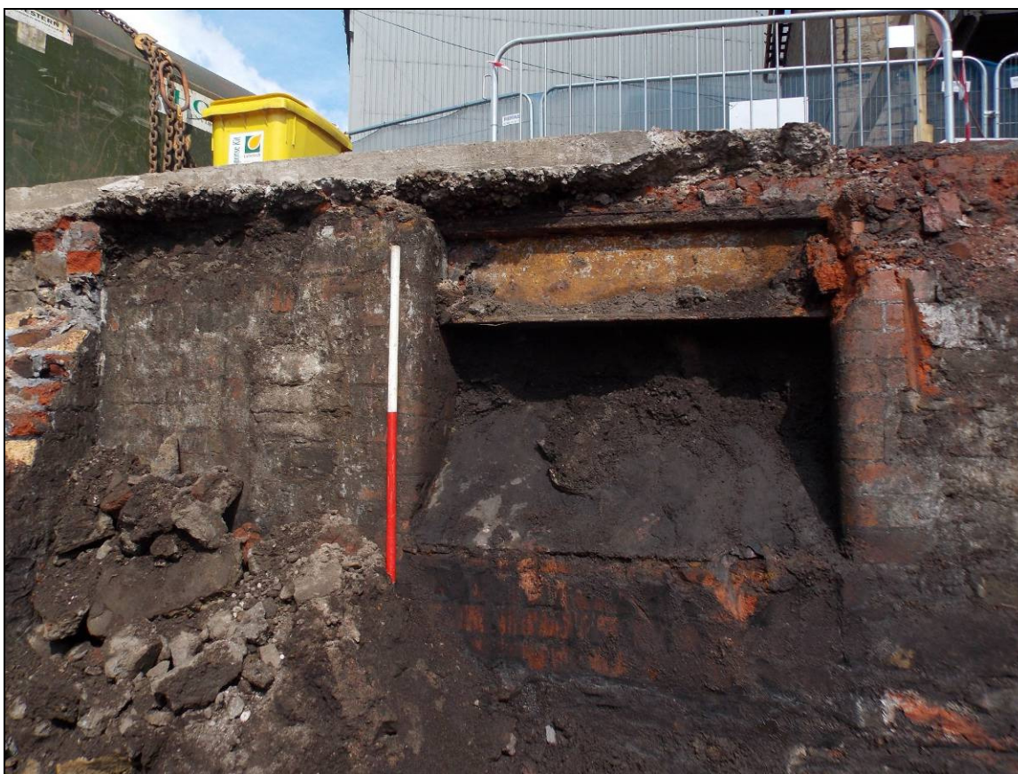
Figure 10: Detail of chute, looking north-west (scale 1m).
