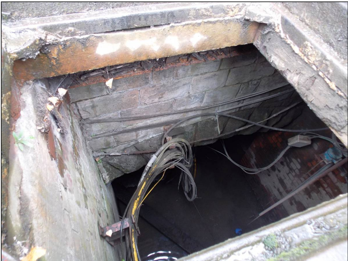
Figure 45: Manhole abutting an earlier stone-built arched structure, looking west.
