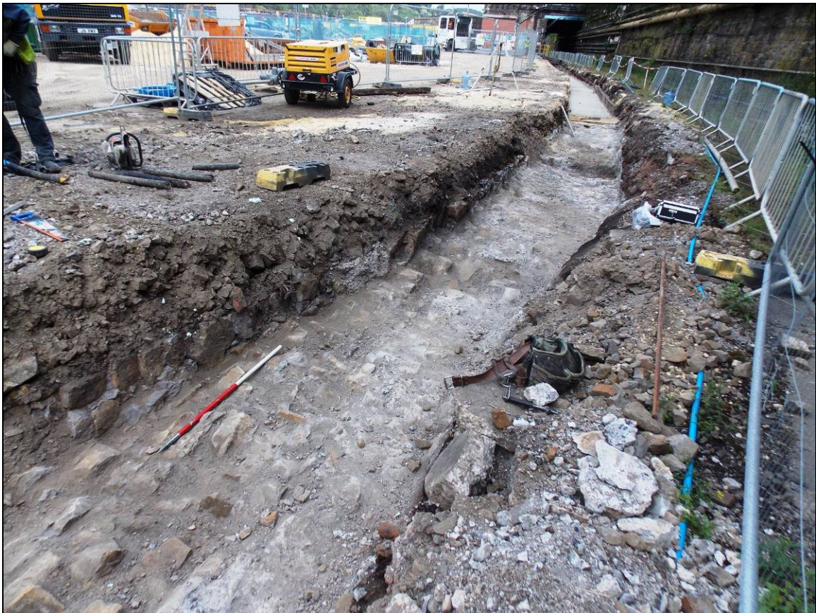
Figure 40: General view of the culvert, looking south-east (scale 1m).
