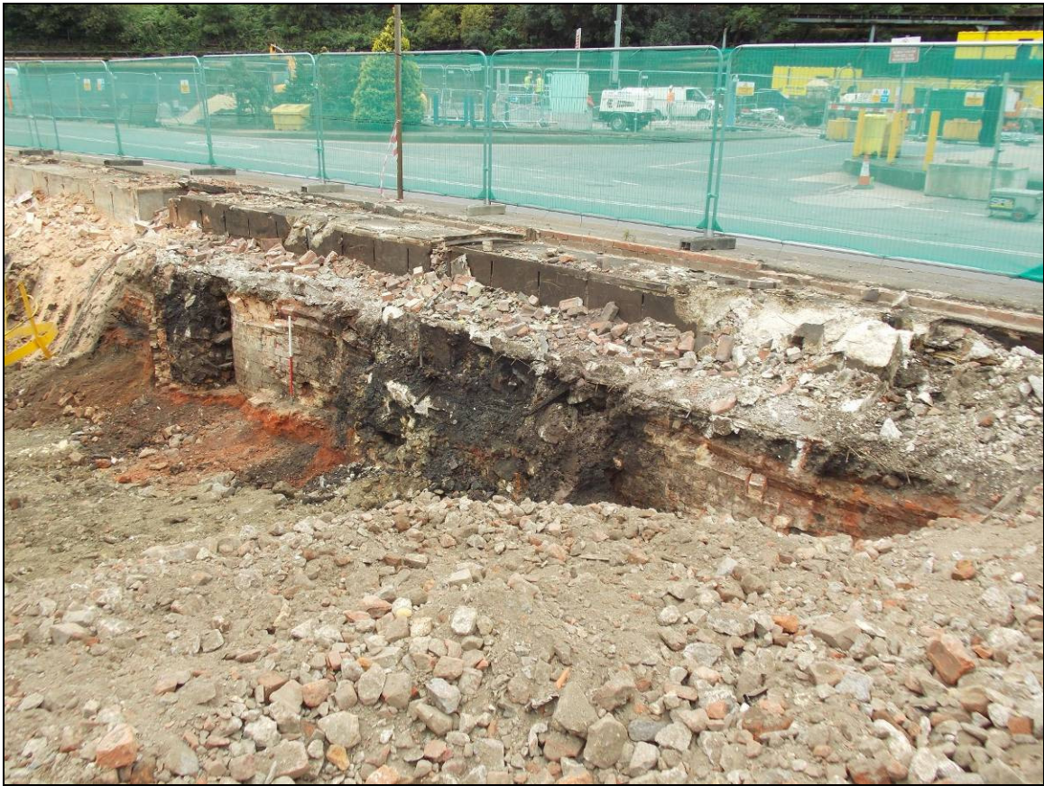
Figure 11: Location of furnace in Division A-3, looking south (scale 1m).
