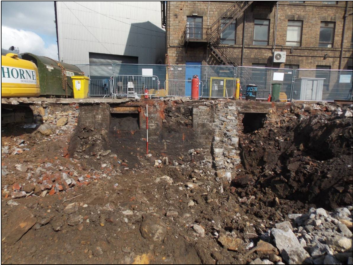
Figure 8: General view of the chutes, looking north-west (scale 2m).
