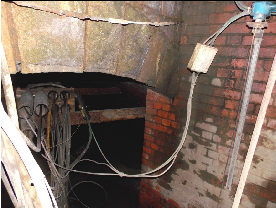
Figure 46: Detail of arch's keystone and voussoirs, looking west.
