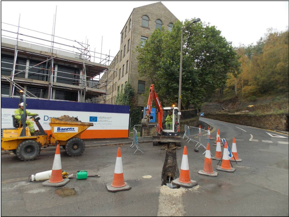
Figure 42: General view of service trench across Hunshelf Road, looking north-west.
