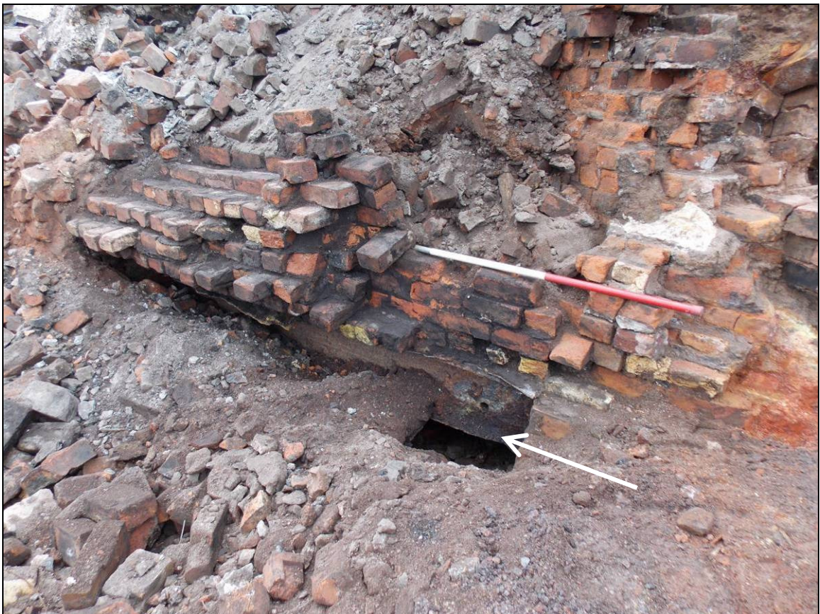
Figure 22: Detail of the RSJ beam with a void beneath (arrow), looking south-east (scale 1m).
