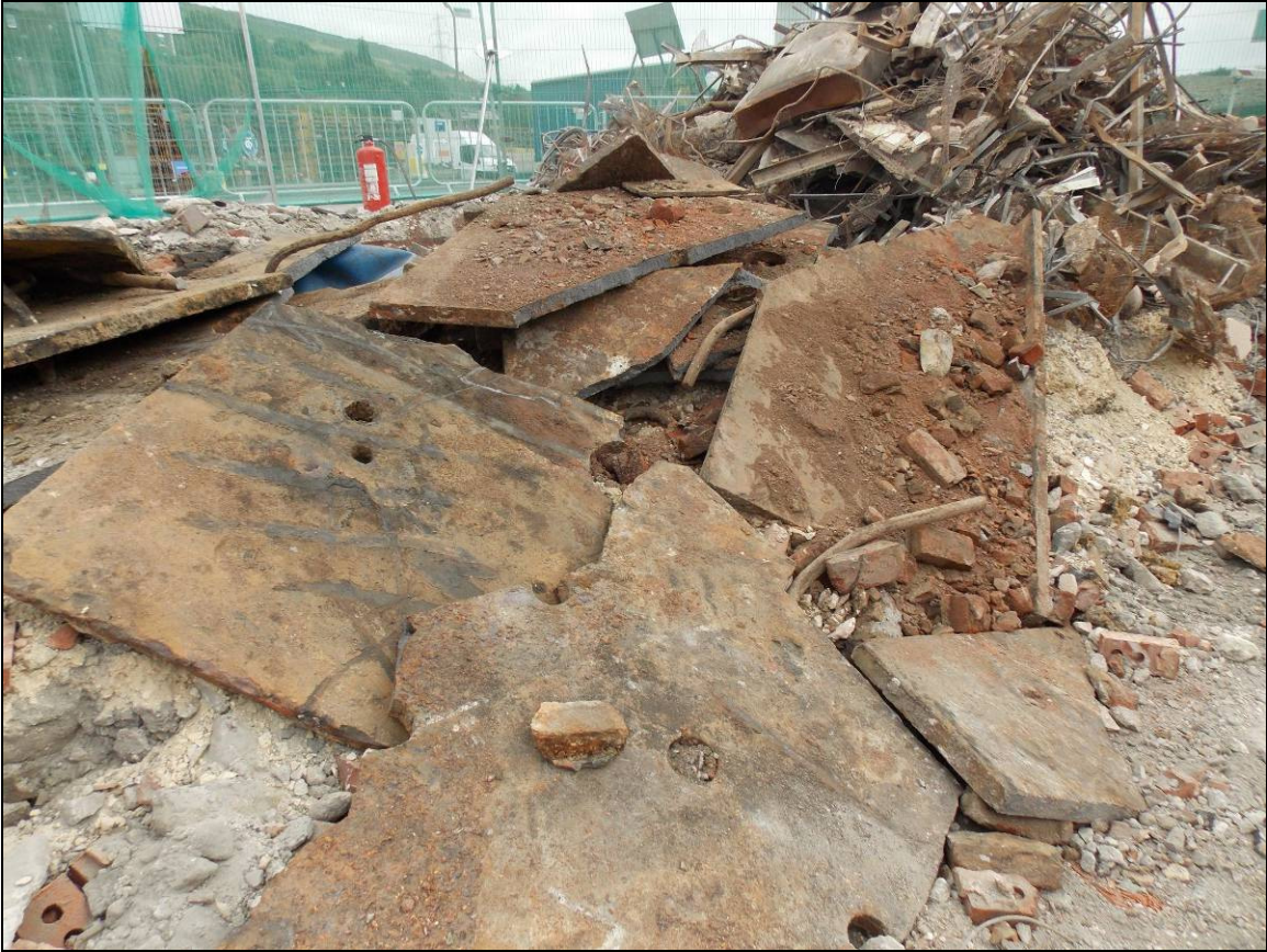
Figure 34: General view of dismantled steel sheets, looking east.
