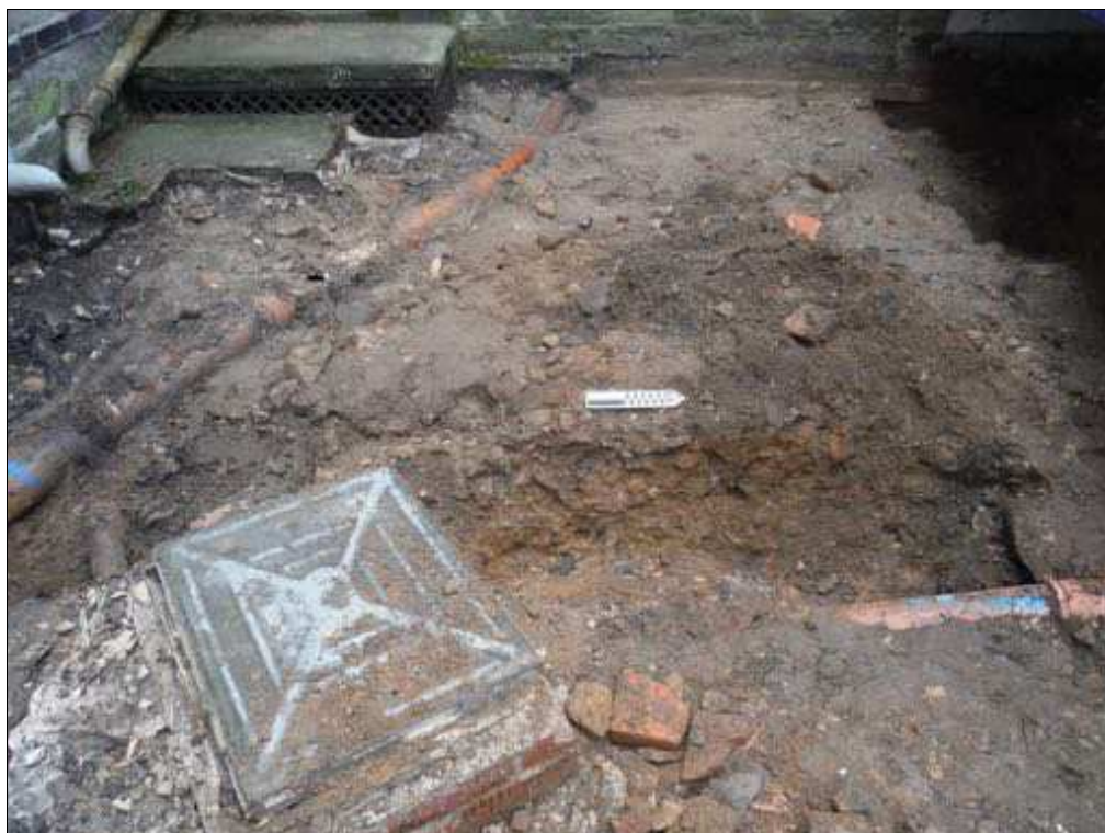
Figure 7. The foundation trenches for the garden room, looking west, excavated to the bedrock. Scale = 0.25m
