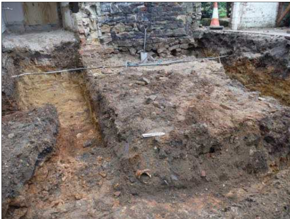
Figure 5. Dower House foundation trenches for north-west extension, looking north-west. The foundation trenches for the former outbuildings (which included a toilet) are visible in the centre of the image in front of the water pipe. Scale = 0.25m.
