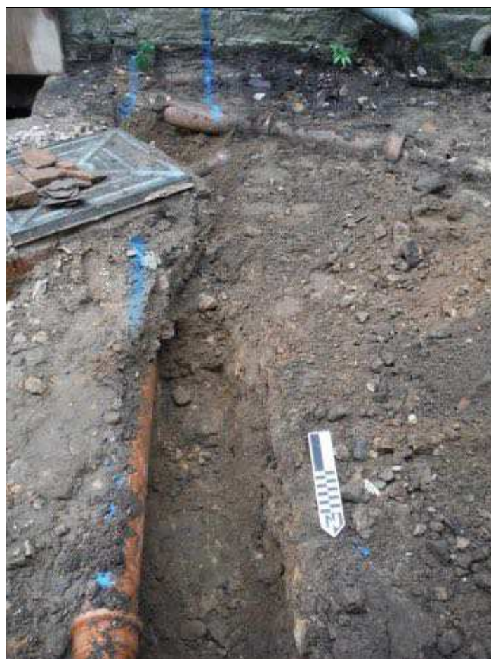
Figure 8. The foundation trenches for the garden room, looking south, excavated to bedrock. Scale = 0.25m
