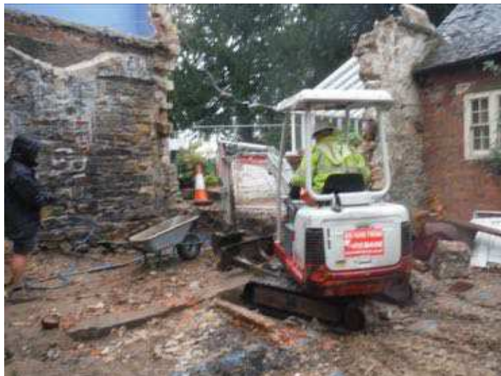
Excavating the footings for an extension at Dower House, Melbourne.
