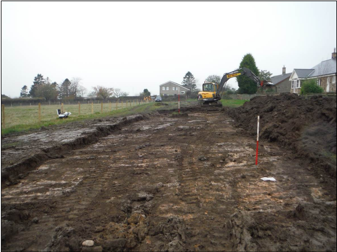
Figure 3: Topsoil strip, looking west. Scale = 1m.
