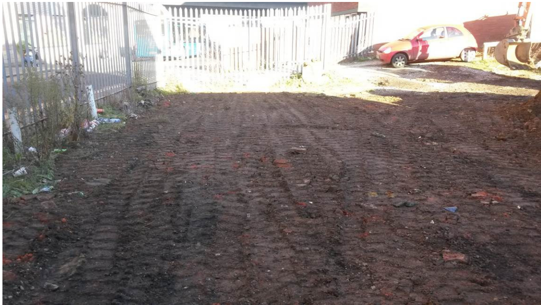
Figure 12: Trench 1 after backfilled. Looking north.
