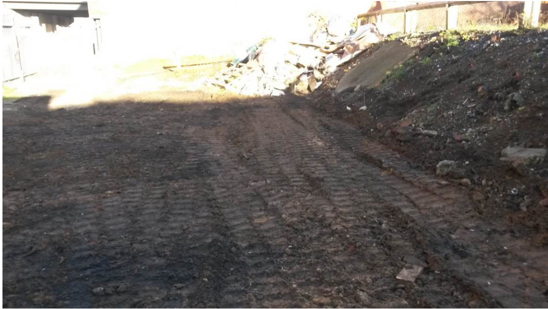
Figure 14: Trench 3 after backfilled. Looking north.
