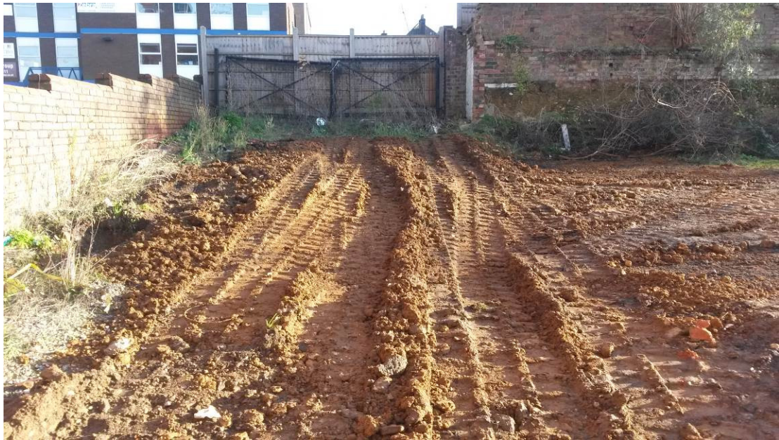
Figure 13: Trench 2 after backfilled. Looking east.
