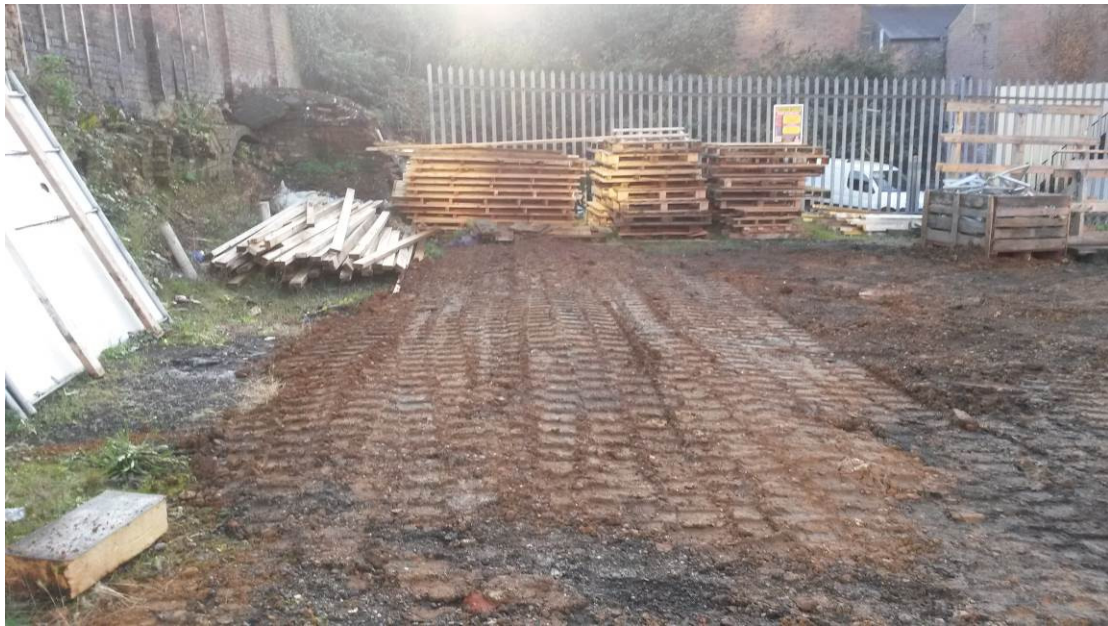
Figure 15: Trench 4 after backfilled. Looking south.
