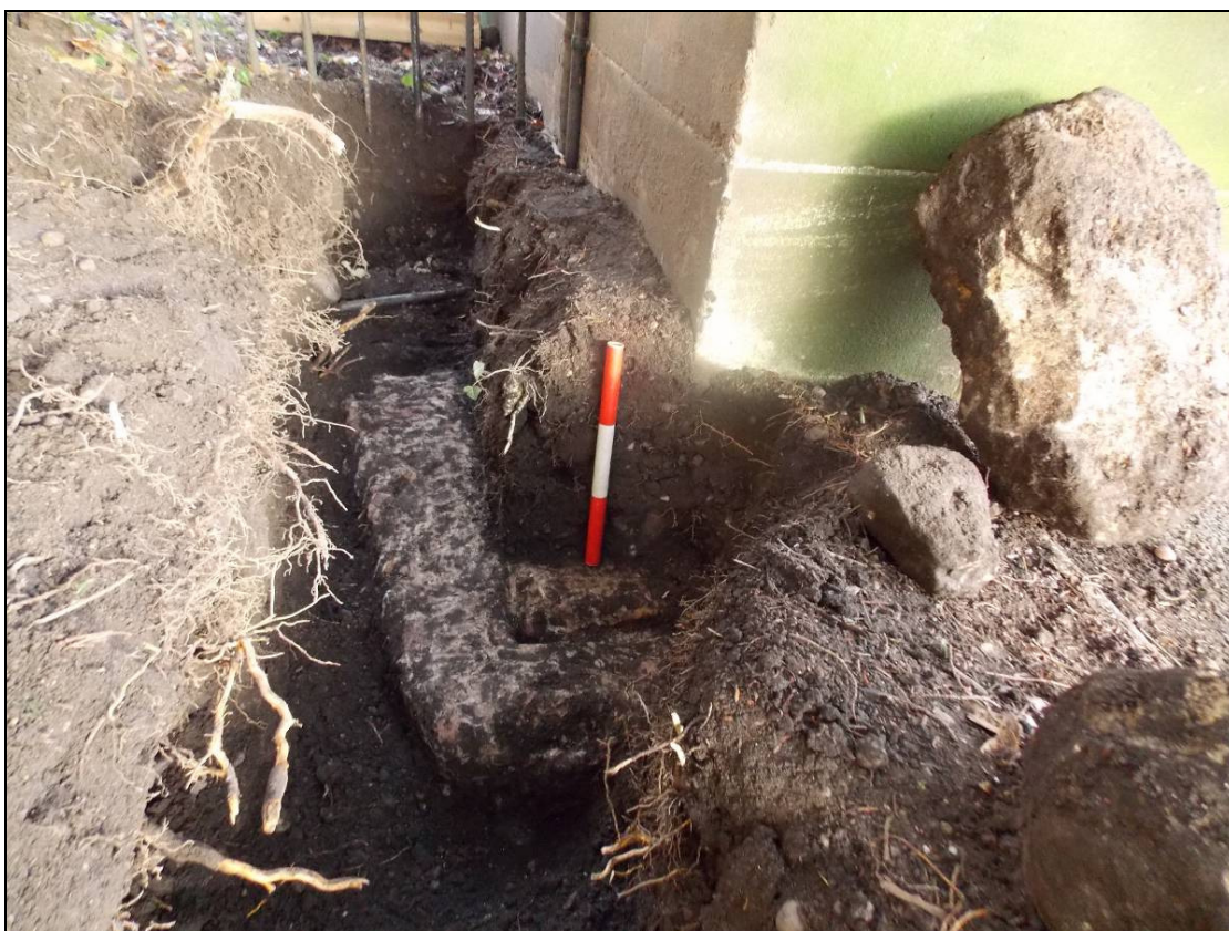
Figure 5: Mortar foundation of lychgate, looking north (scale 300mm).
