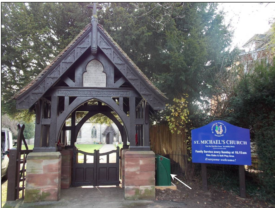
Figure 4: The lychgate and adjacent gas main (arrow).
