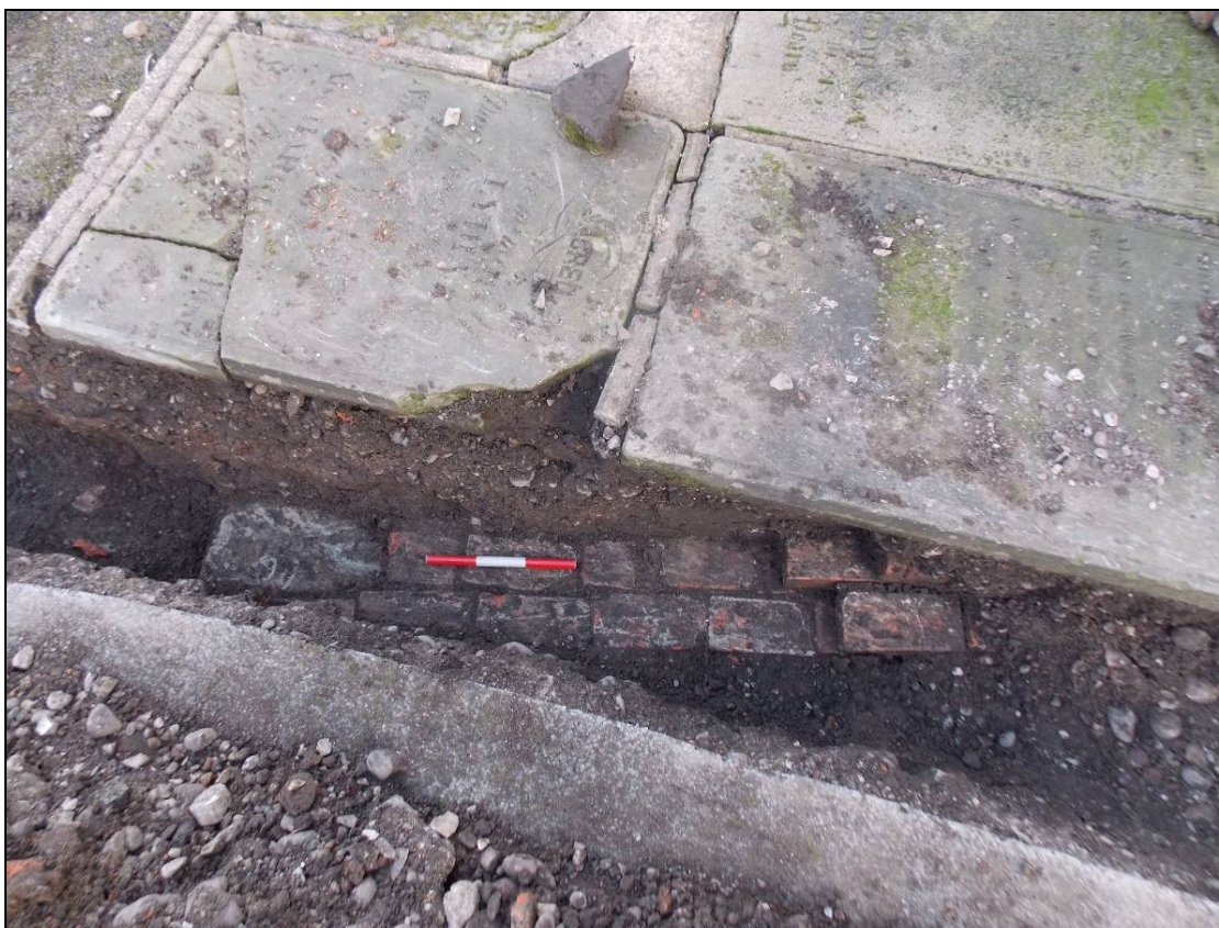
Figure 9: Brick wall (102), looking east (scale 300mm).
