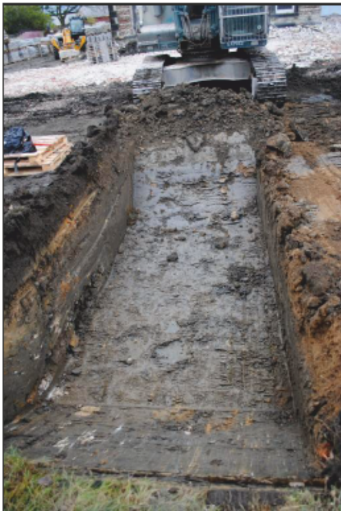
Figure 4: Phase 1 Trial pit during excavation, looking north.
