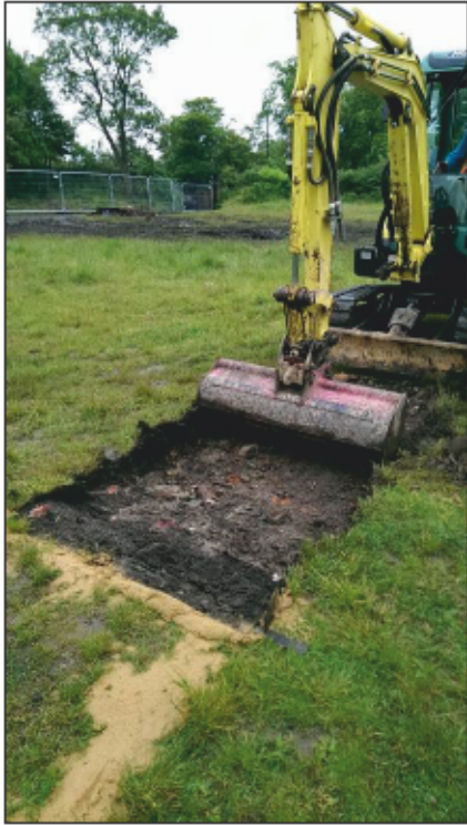
Figure 7: Phase 2 Trial pit during excavation, looking south-east showing deposit (202).
