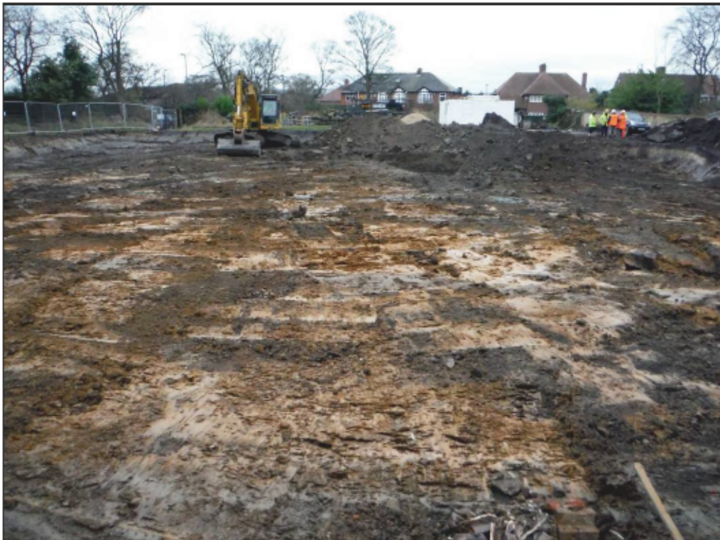
Figure 13 : Phase 3, looking south, re-deposited clay across site (414).
