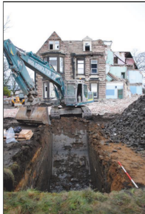
Figure 5: Phase 1 trial pit following excavation, looking north (scale = 2m).
