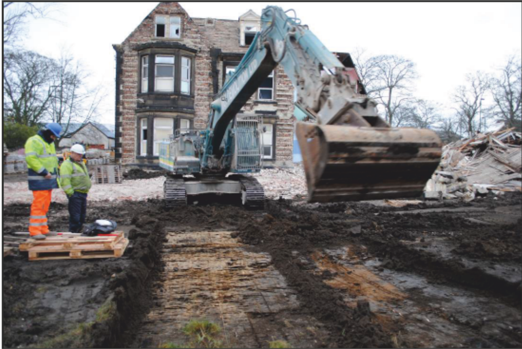
Figure 3: Phase 1 trial pit during excavation, looking north-east.
