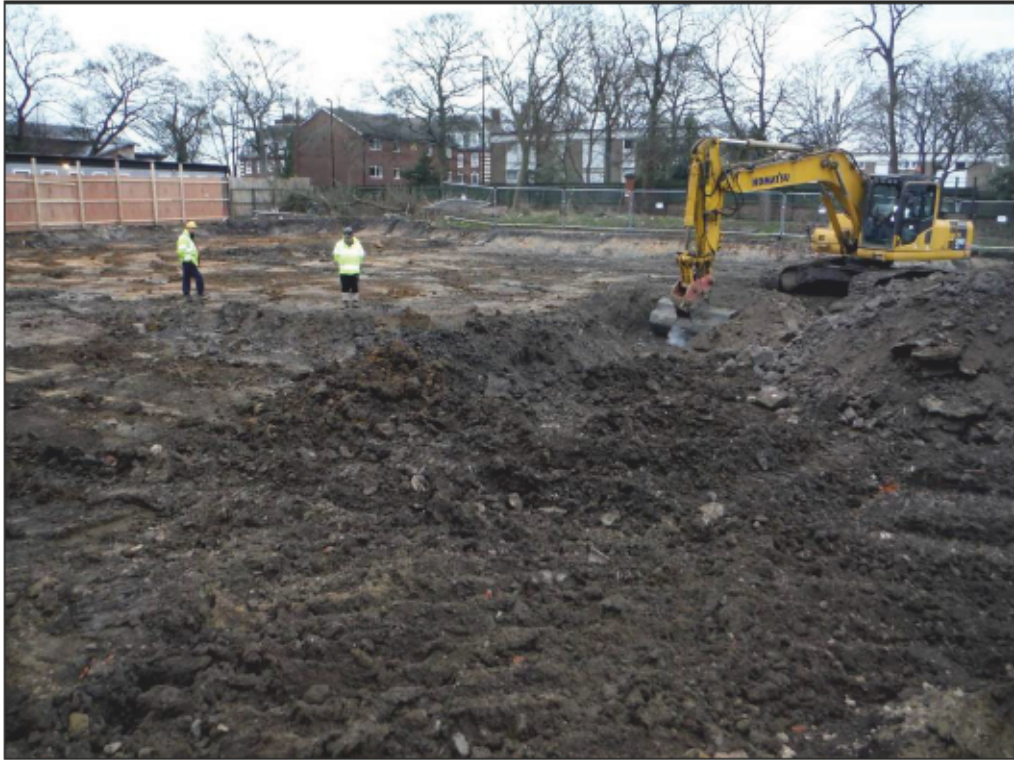
Figure 12: Phase 3, looking north-east, modern backfill deposits in foreground.
