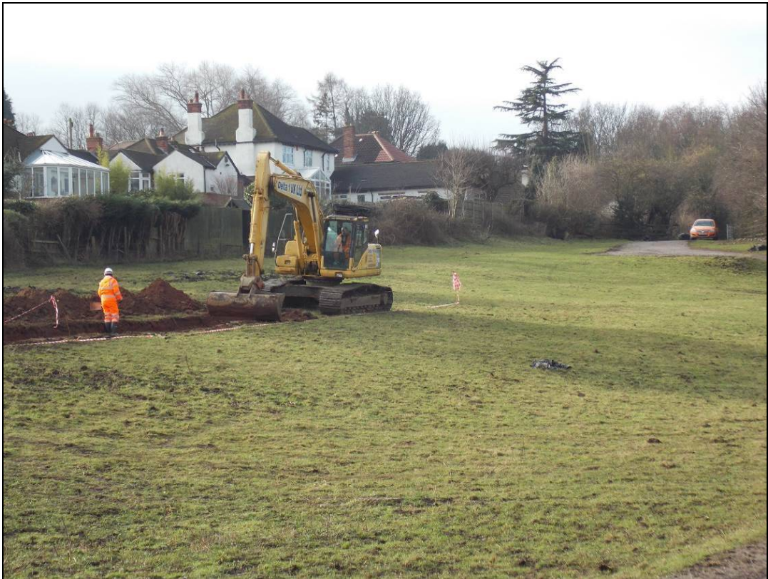
Figure 3: General view of trench 1 during excavation, looking south-west.
