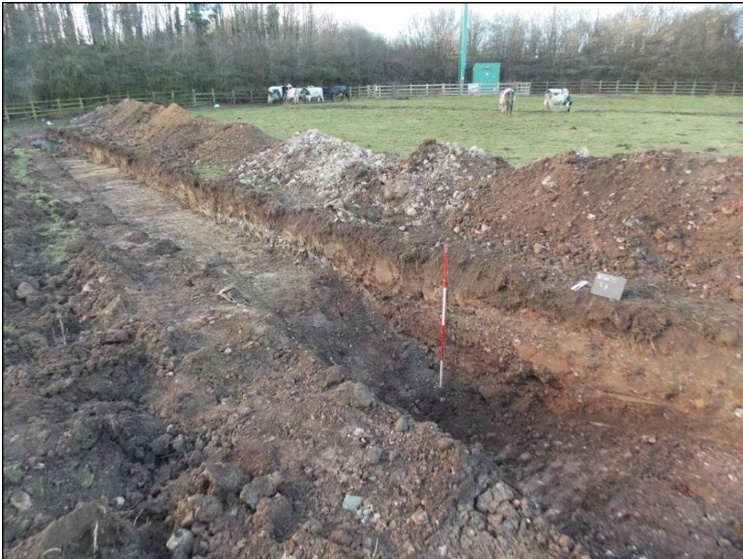
Figure 11: General view of trench 3 viewed from the eastern end (scale 2m).
