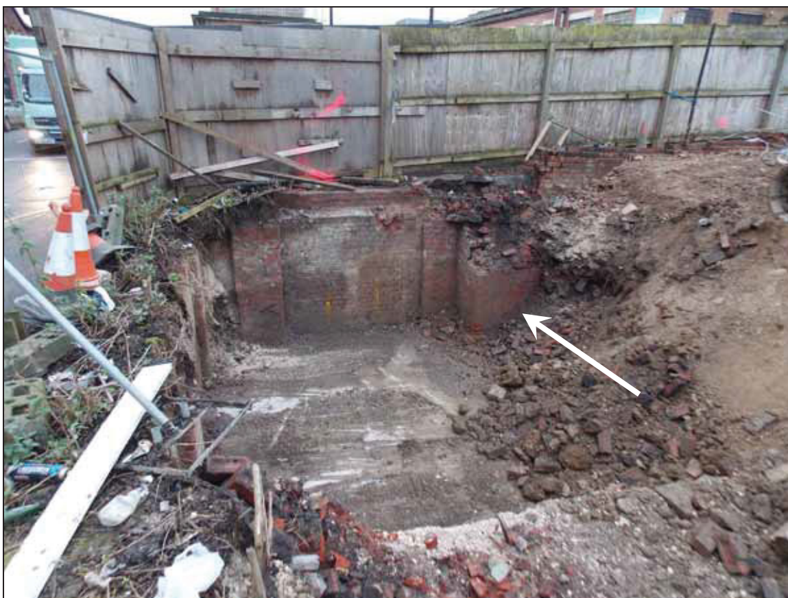
Figure 19: Cellar (111) with stairwell (114) (arrow), looking south-west.
