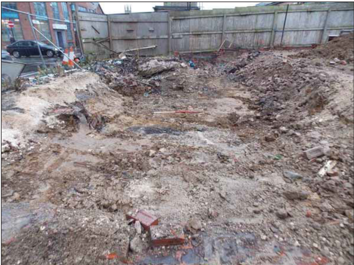
Figure 14: Southern area of the site, looking south-west.
