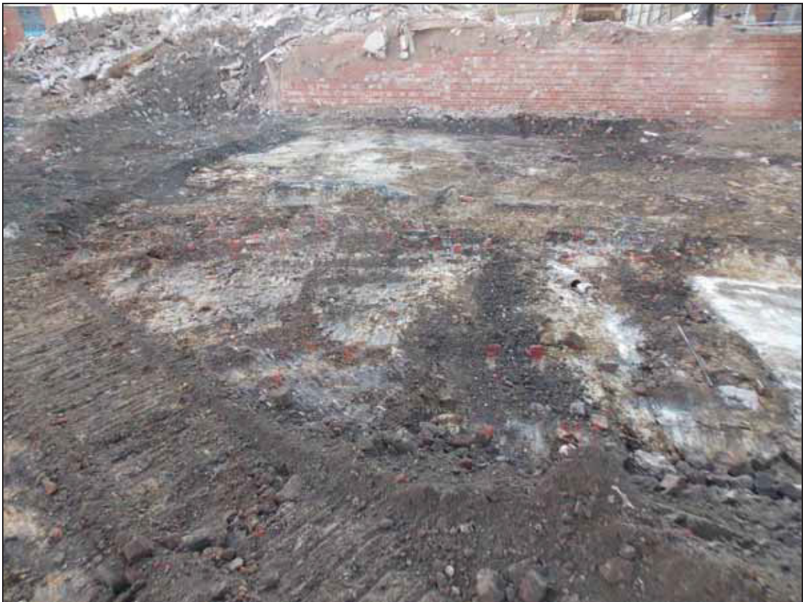
Figure 4: General view of the north-western area, looking south-west.
