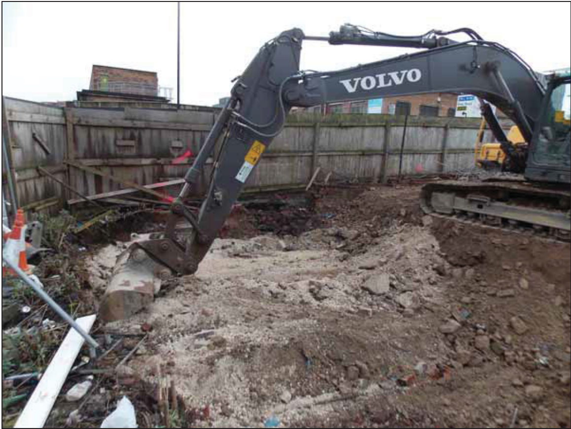
Figure 15: Excavation of the southern area of the site, looking south-west.
