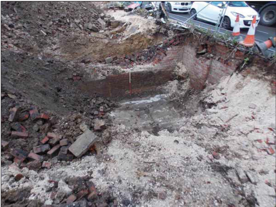
Figure 18: Partially excavated cellar (111) revealing concrete floor (112), looking north-east (scale 1m).
