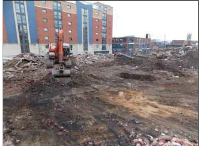
Excavation on land at 102 – 112 Arundel Street, Sheffield.
