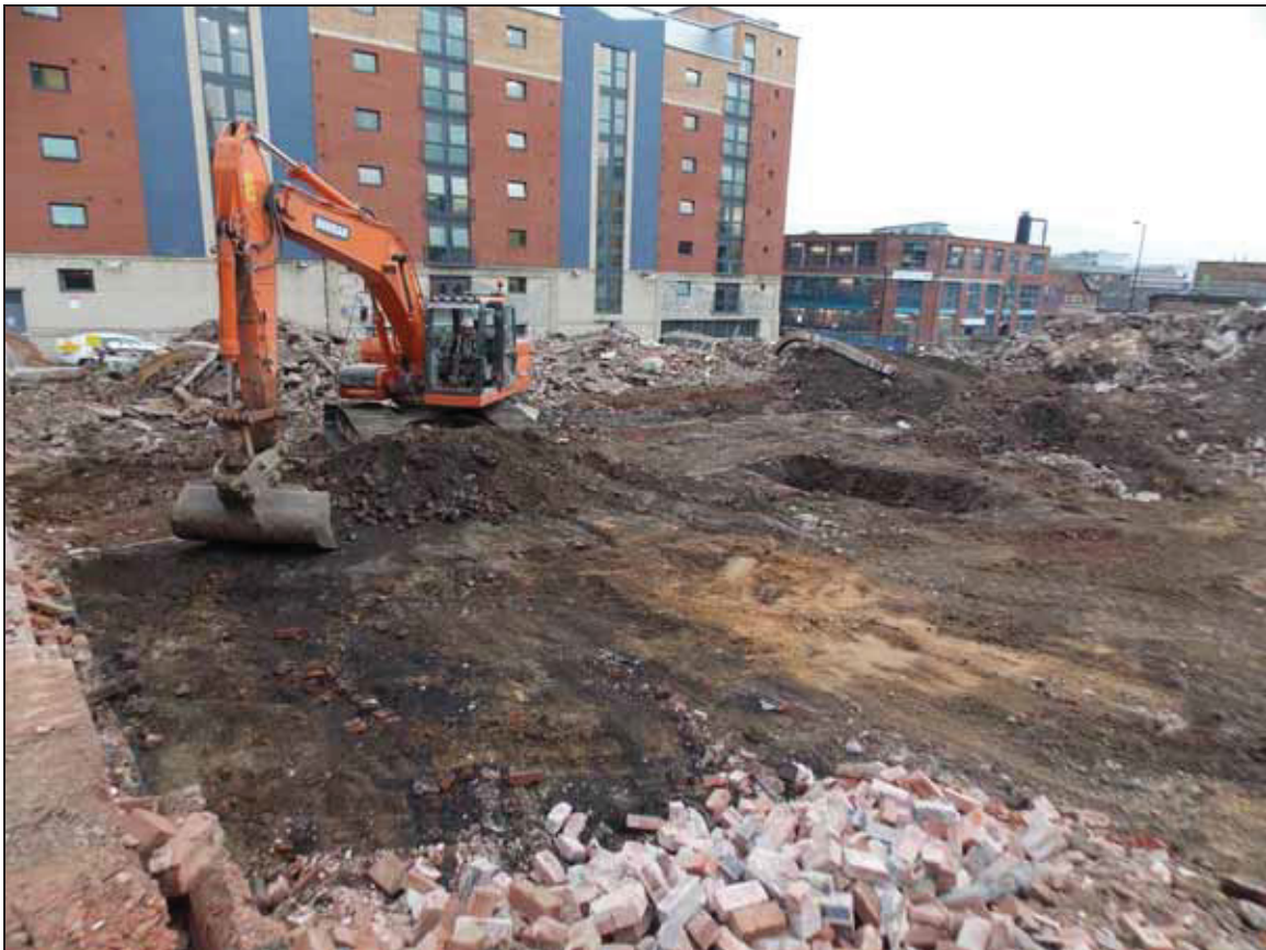
Figure 2: Initial stripping of the northern area of the site, looking south.
