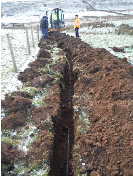
Figure 13: Trench 9 looking south (scale =1m).
