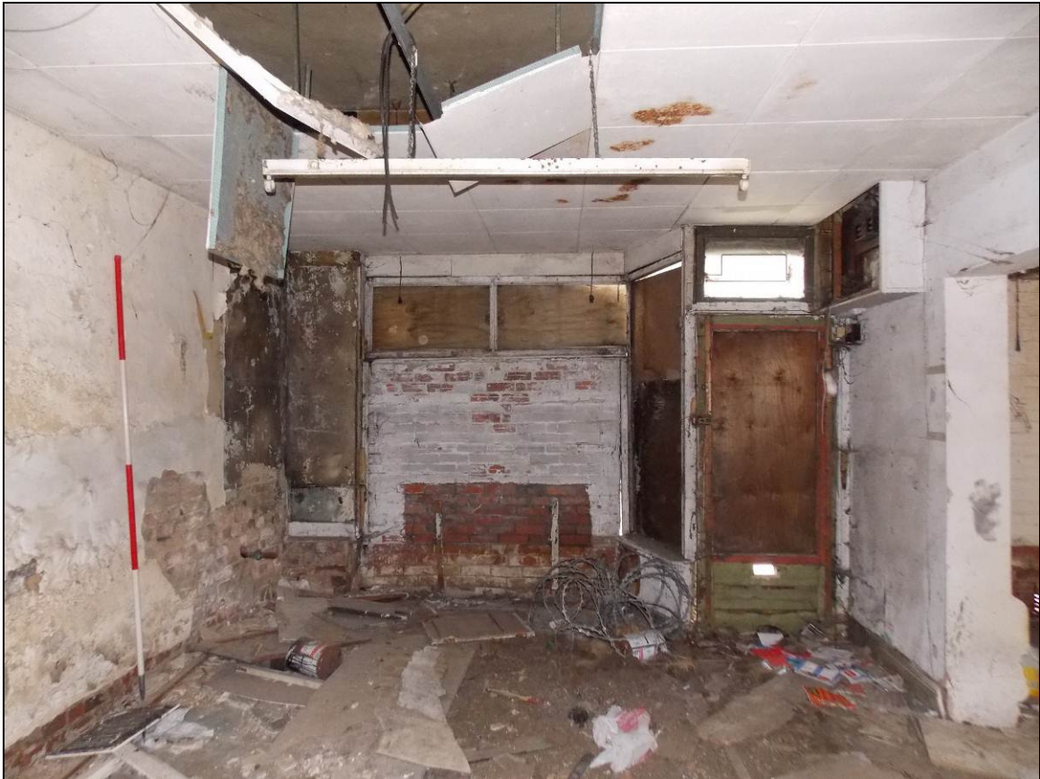
Plate 19: North-eastern room within the ground floor, looking south-east (scale 2m).
