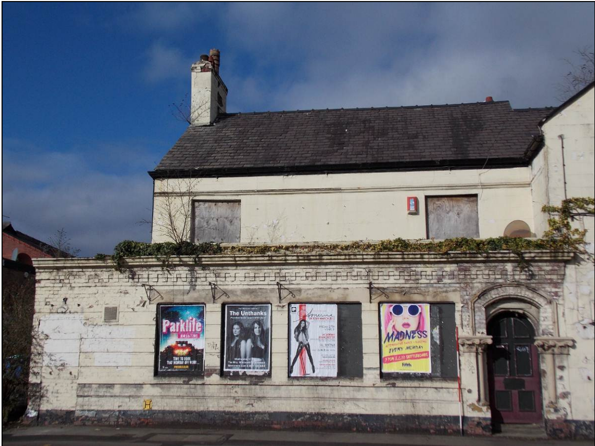
Plate 2: Rusticated brick wall with principal doorway, looking north-west (scale 2m).
