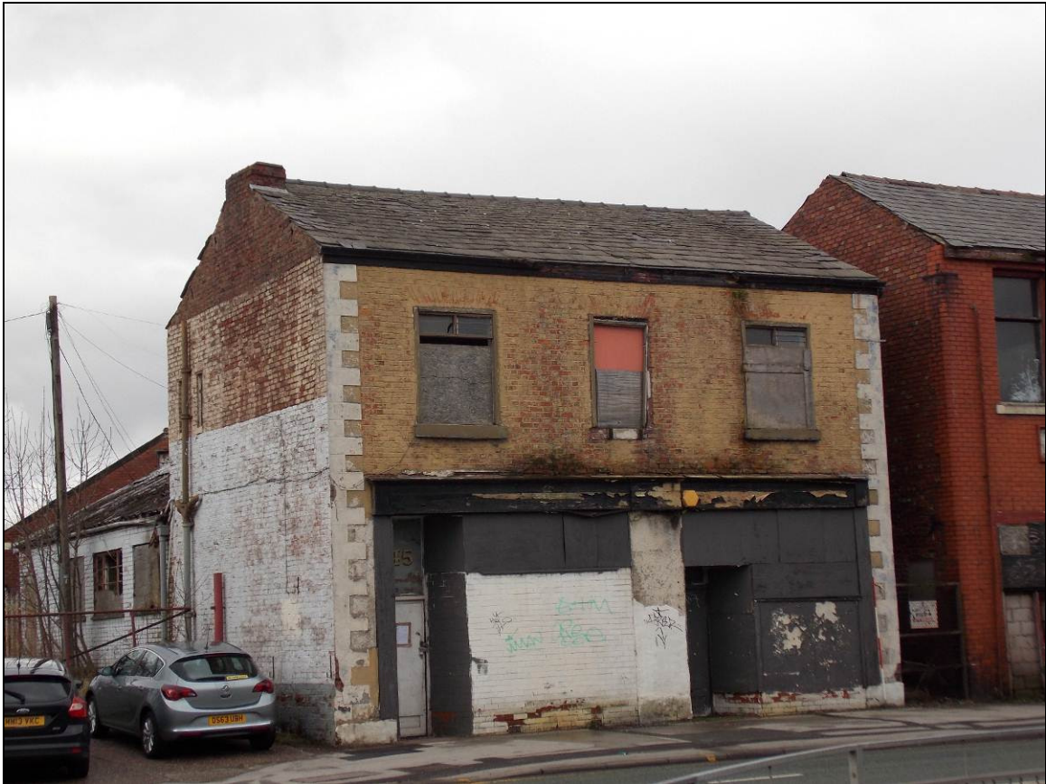
Plate 13: South-west gable wall with reduced chimney stack, looking north (scale 2m).
