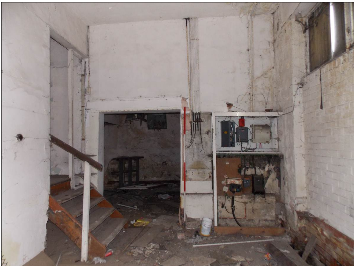
Plate 18: South-western room within the ground floor, looking north-east (scale 2m).
