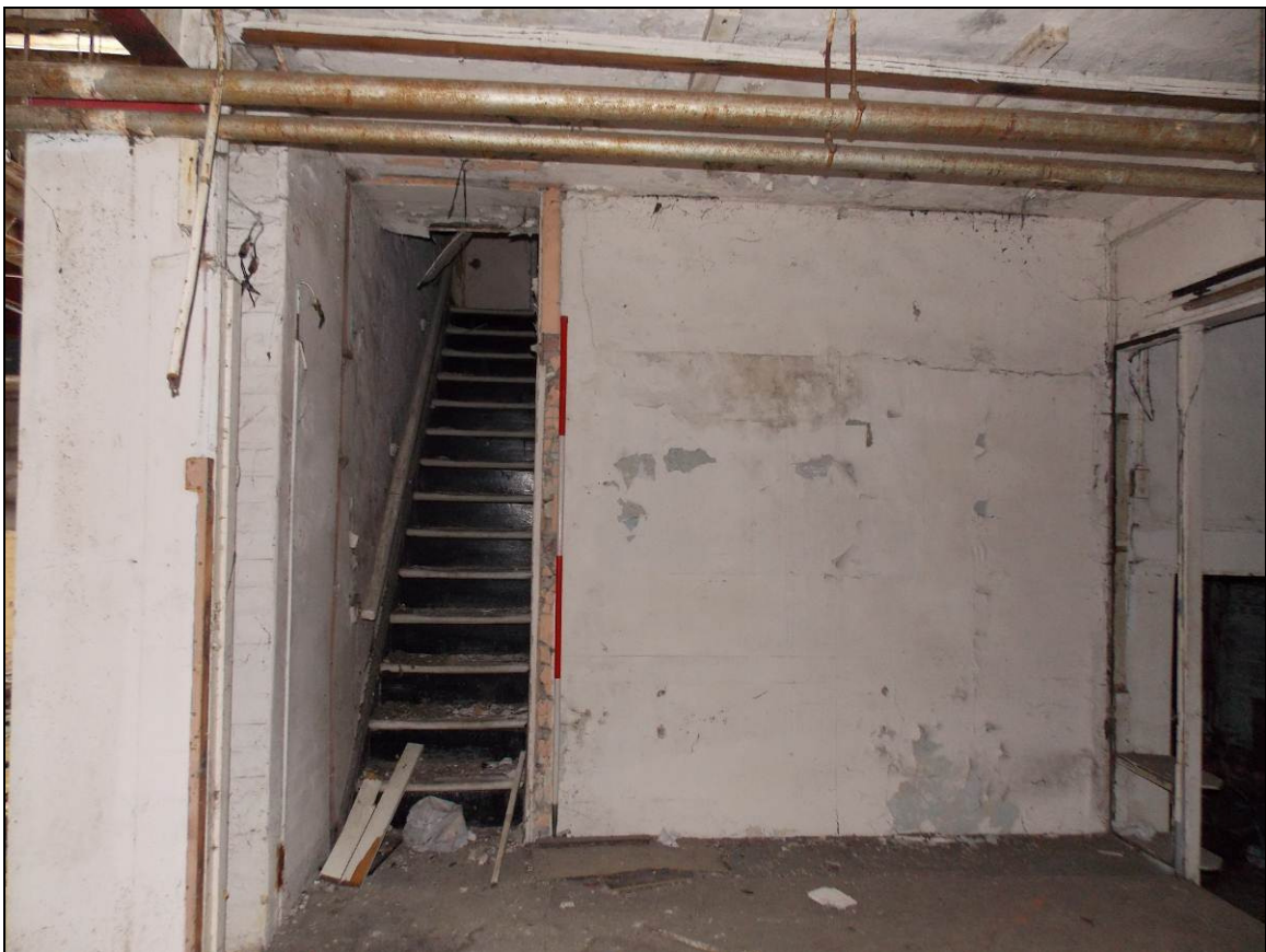
Plate 22: Staircase to the first floor, looking north-east (scale 2m).
