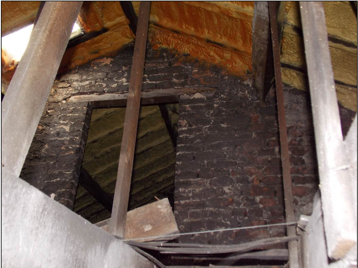
Plate 27: Loft area with a brick partition wall, looking north-east.
