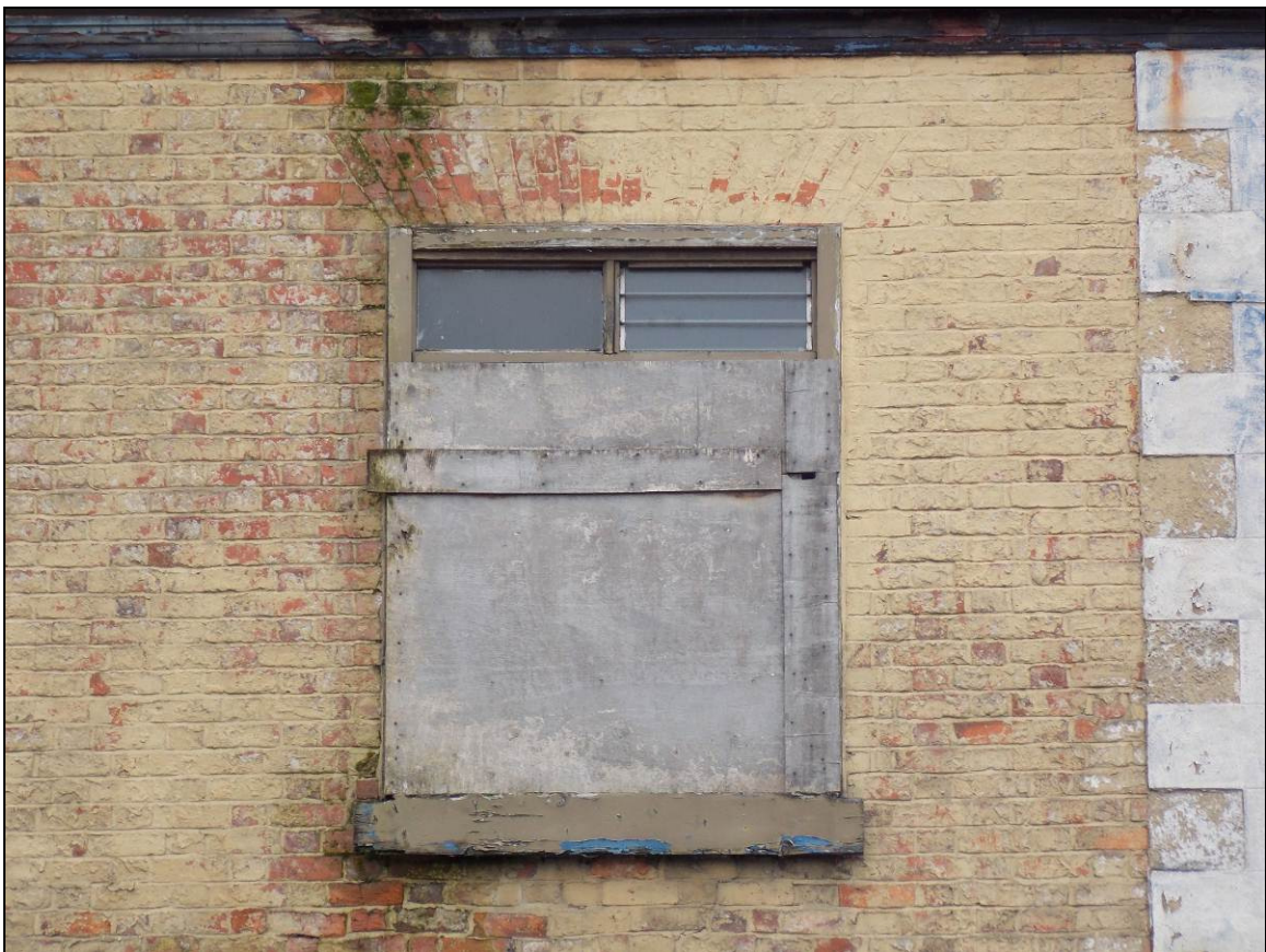
Plate 12: Detail of window opening within the first floor, looking north-west.
