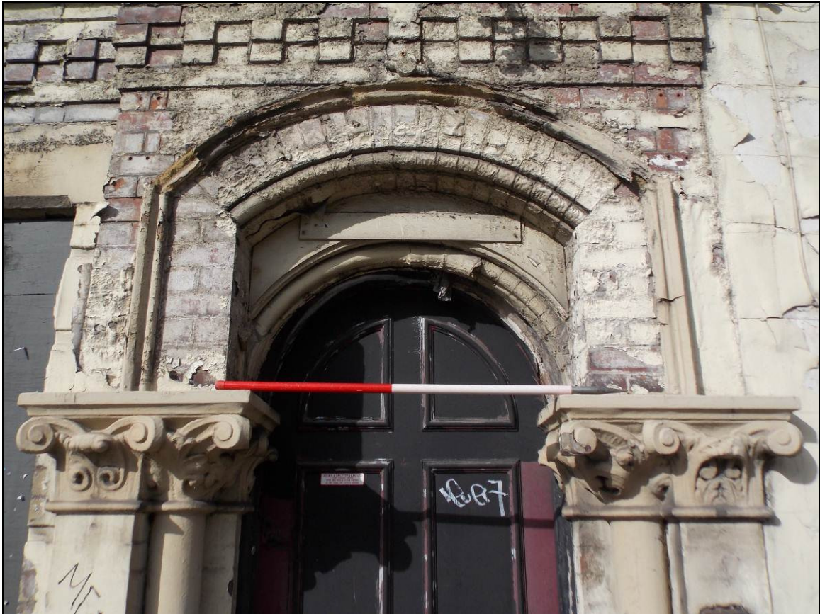
Plate 4: Detail of capitals and arched head, looking north-west (scale 1m).
