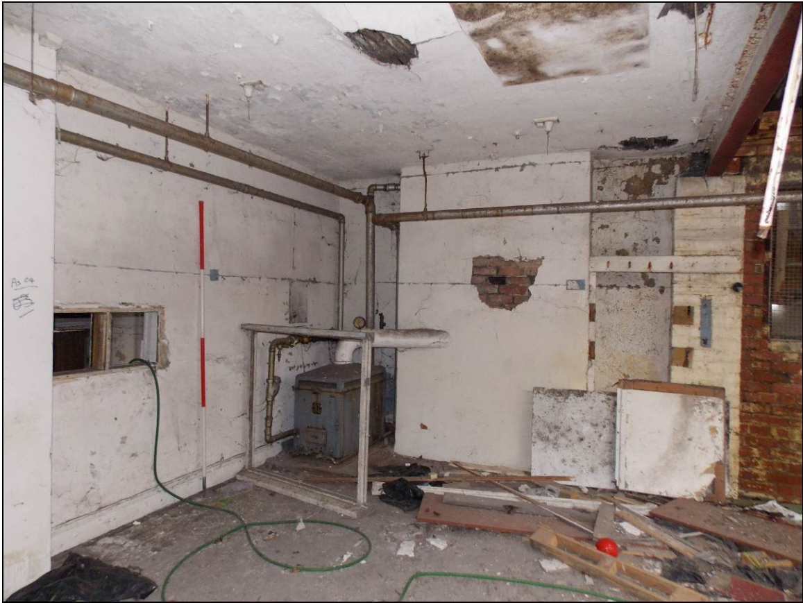
Plate 21: South-western room within the ground floor, looking south-west (scale 2m).
