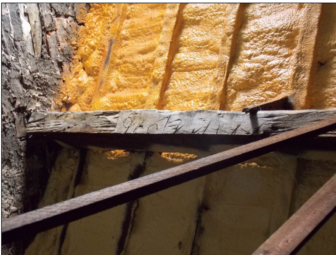
Plate 29: Sawn purlin with Baltic shipping mark.
