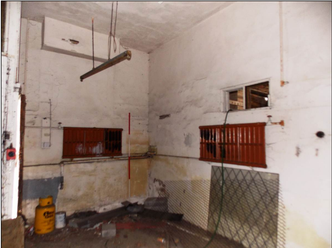
Plate 17: South-western room within the ground floor, looking south-west (scale 2m).
