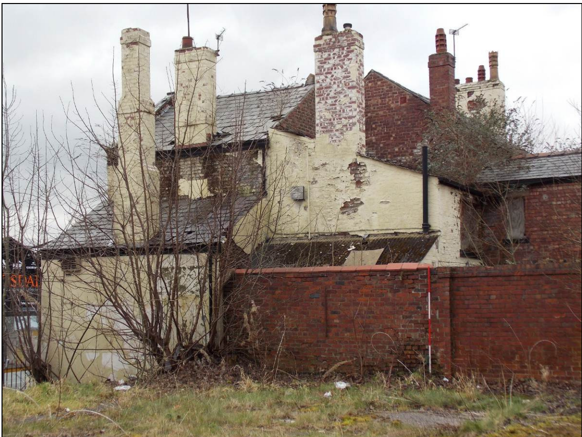
Plate 9: North-east elevation, looking south-west (scale 2m).
