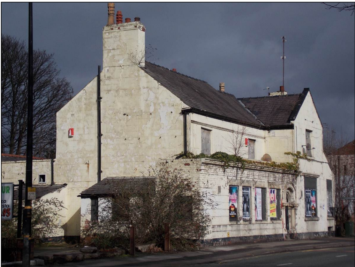
Plate 5: South-west gable wall, looking north (scale 2m).
