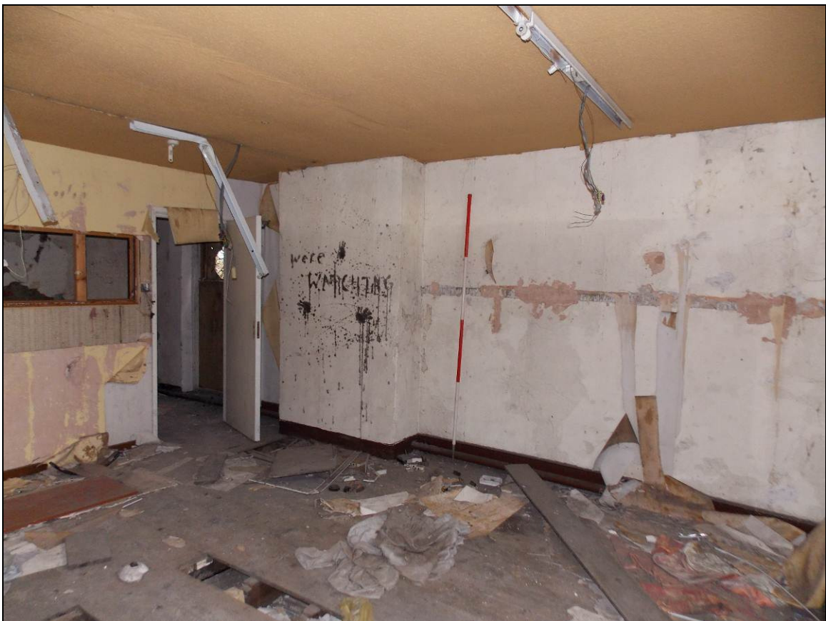
Plate 24: Northern room within the first floor, looking north (scale 2m).
