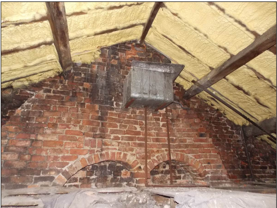
Plate 28: Upper section of the converging chimney breast along the south-west wall.
