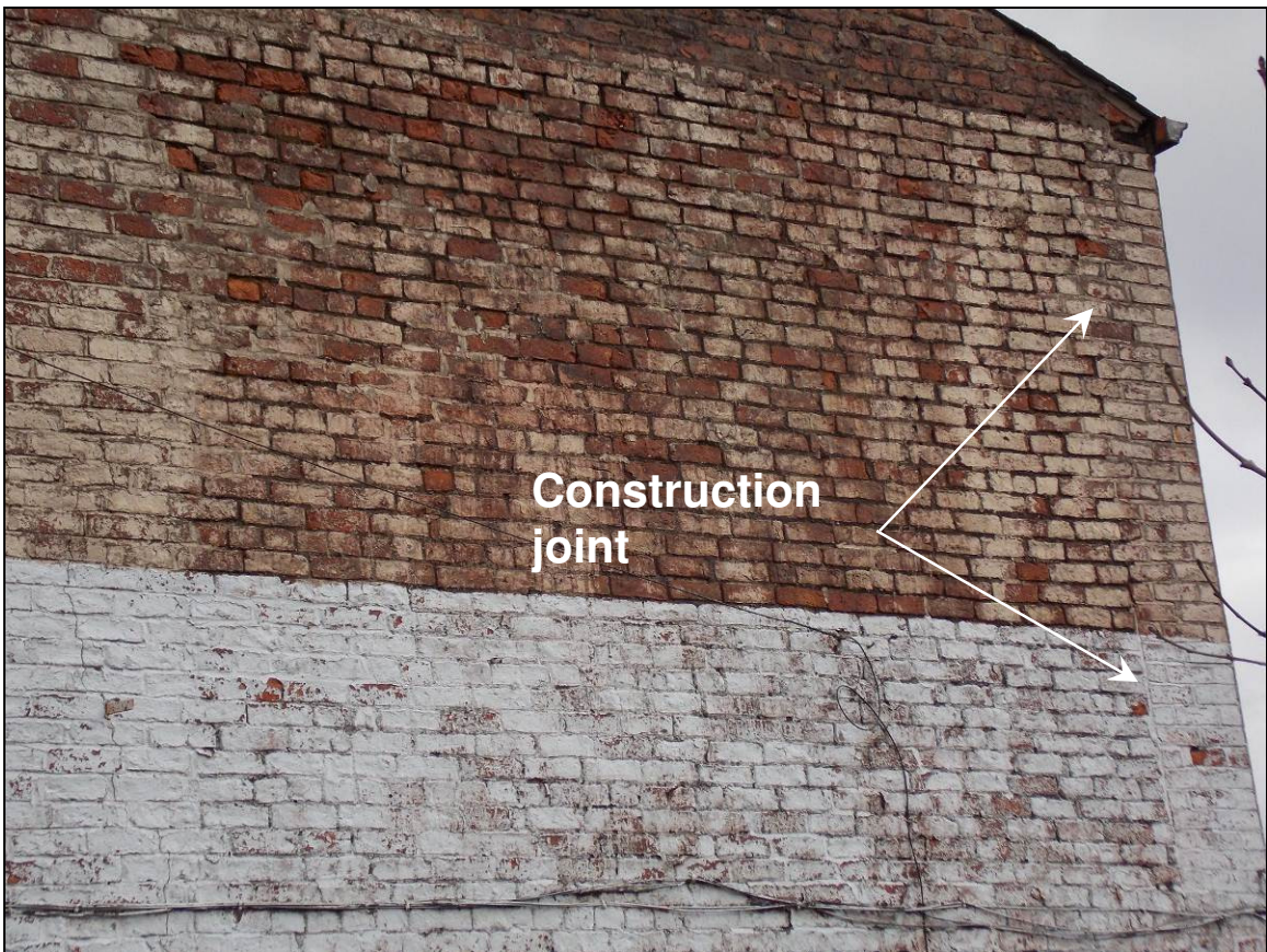
Plate 14: Detail of construction joint, looking north-east.
