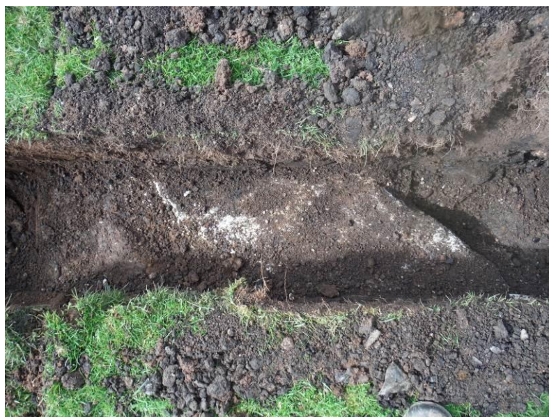
Figure 8. Concrete possible foundation uncovered during excavation.
